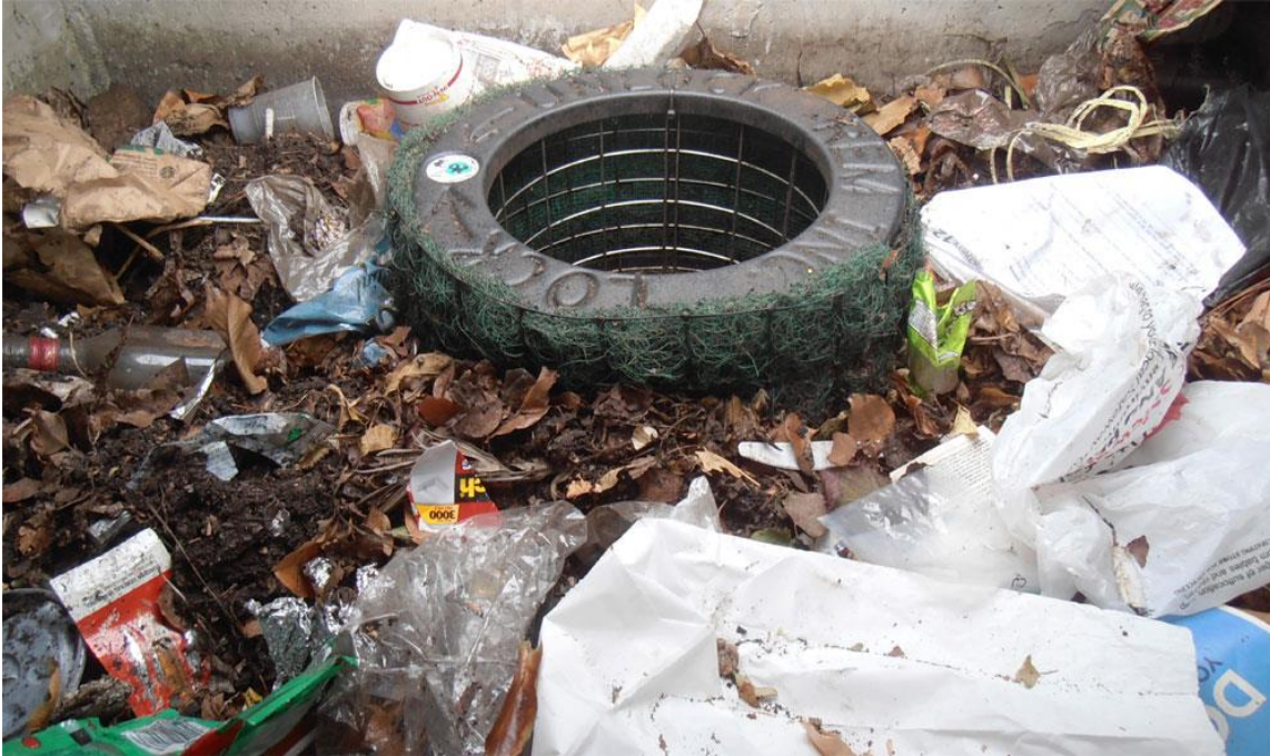
Trash capture device in a catch basin. Credits: https://remfilters.com/triton-full-trash-capture/
