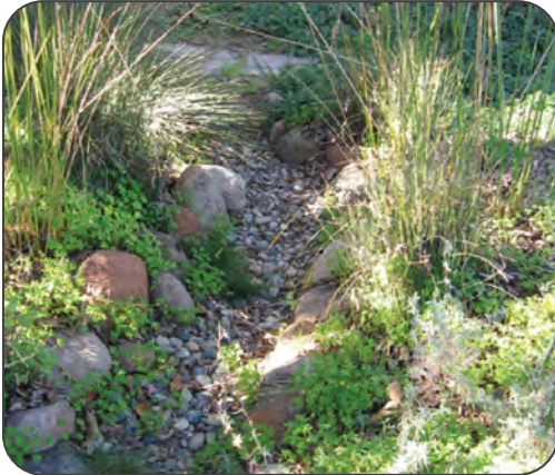
Dry creek infiltrates and conveys runoff.
