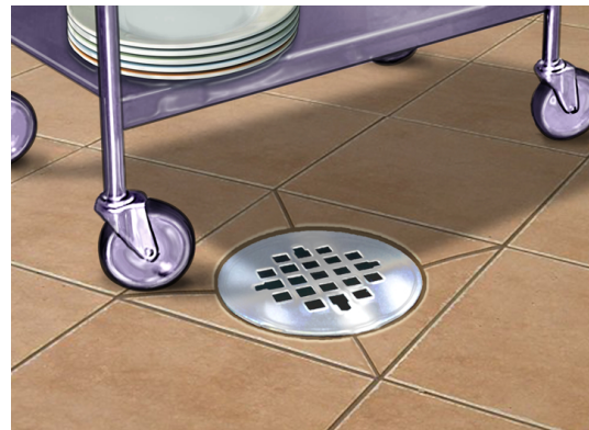
Sanitary Sewer Drain: An indoor drain that flows to the sewage treatment plant.
