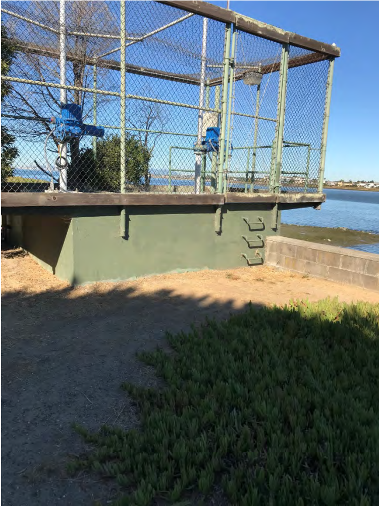
Figure 2B – Bay Farm Island Gate Structure
