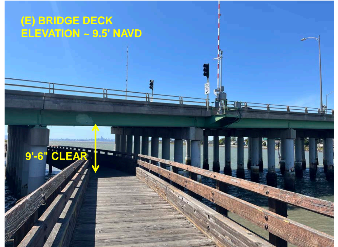
EAST SIDE (looking west)
