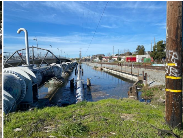
Embarcadero West Bridge over Lake Merritt Channel
