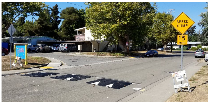
Figure 2: Speed cushions on Orion St, installed in 2023
