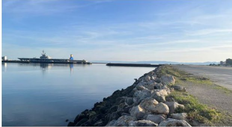
Seaplane Lagoon Armored Shoreline
