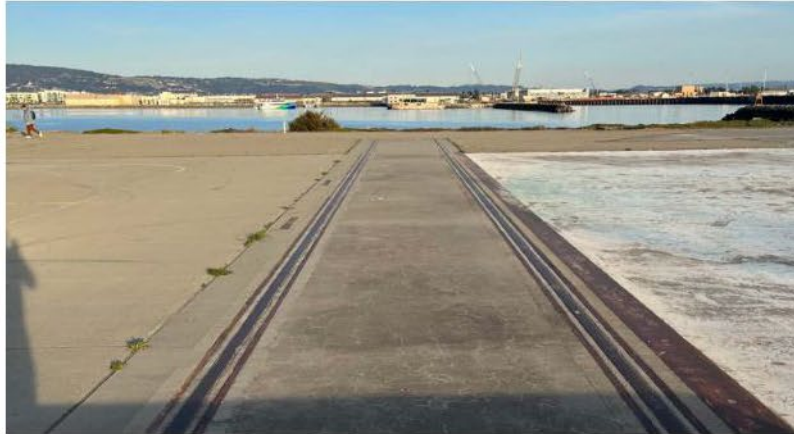
Rails Embedded in Concrete
