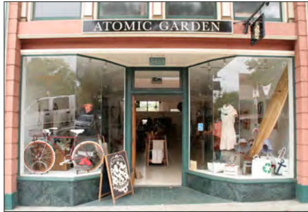
Storefront elements should include a bulkhead, display windows, recessed entry, transom windows, and awnings or overhangs.
