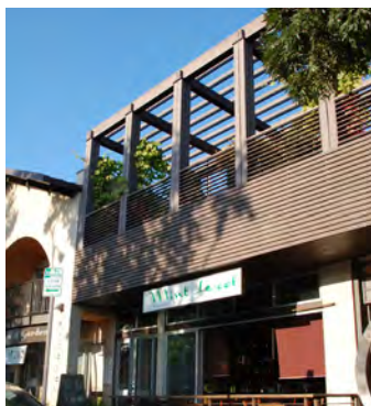
Second floor terrace with horizontal wood railings.
