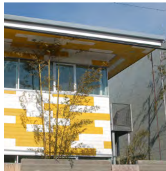
Large roof overhangs minimize heat gain.
