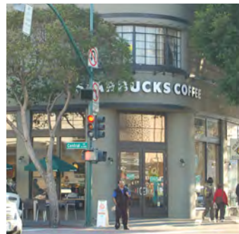
Stucco wall with horizontal lines.
