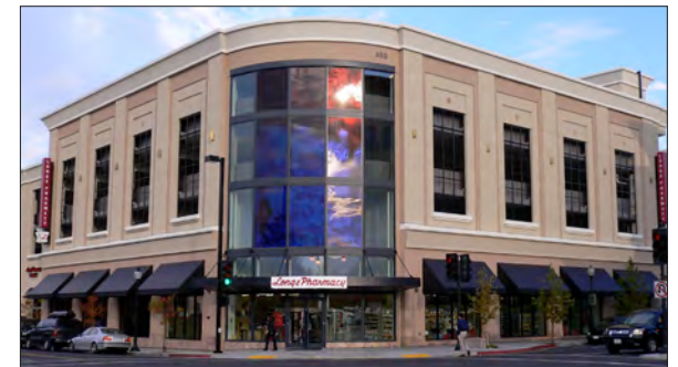
A retail anchor with prominent corner entry occupies the ground floor of this parking structure.
