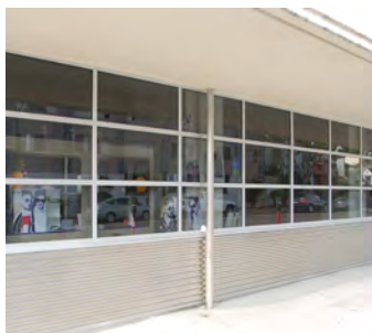
Metal cladding is used as a secondary material at building base.
