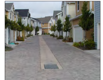
Pervious concrete pavers in alley can be used to decrease run-off.
