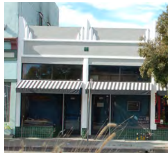
Smooth stucco is an appropriate material for Art Deco buildings.
