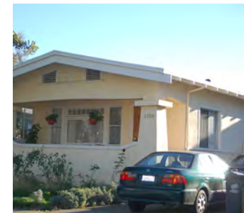
Downspout is located on side of house.
