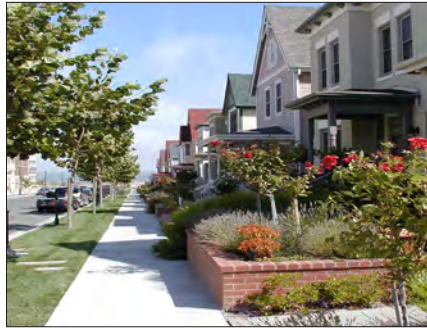
Single family homes with terraced front yard retained by decorative wall.
