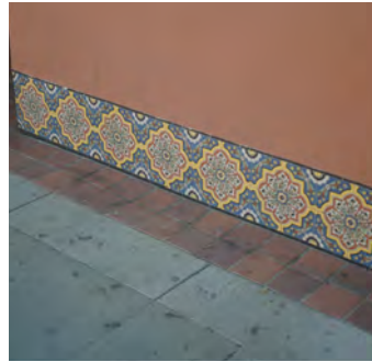
Base treatment with decorative Spanish tile.
