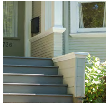
Raised entry with lap siding base treatment.
