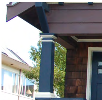
Entry porch column detail.
