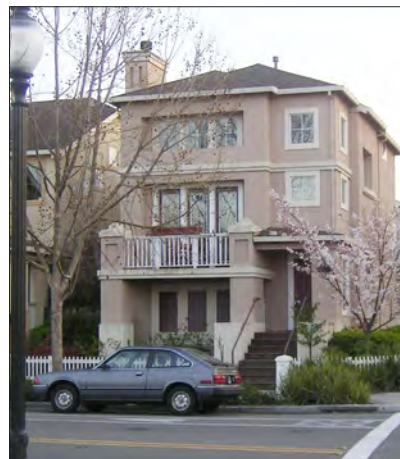
Duplex with ground floor garden unit and two story apartment above.
