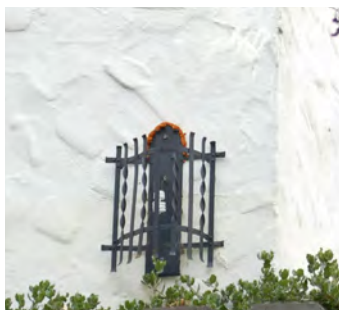
Mediterranean Revival decorative wrought iron light fixture.
