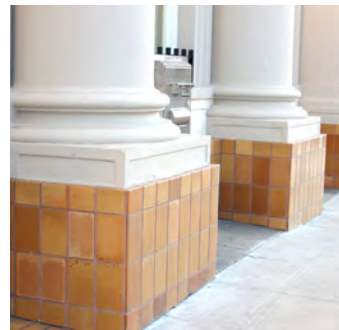
Column base treatment with tile plinths.
