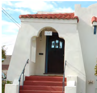
Raised entry porch with tapered walls.
