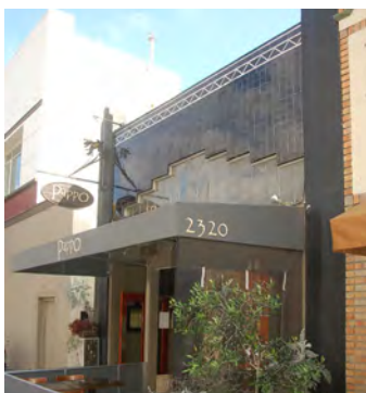
Ceramic tile is used for primary cladding material.
