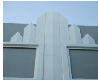
Smooth stucco wall surface with decorative pilaster.
