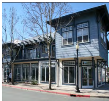
Contemporary workplace commercial with divided-lite transom windows.
