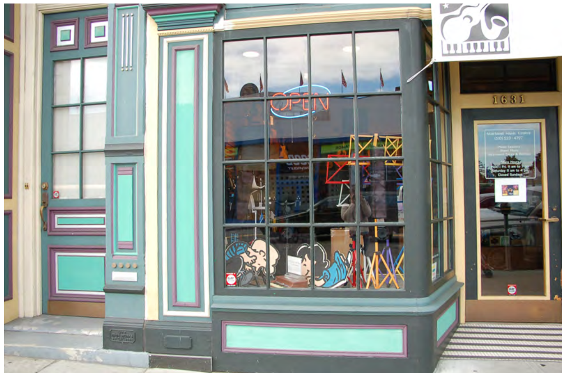
Storefront windows are framed in wood and contain wood sills. Bulkhead contains decorative painted wood panels. Secondary colors are used to accentuate architectural details.
