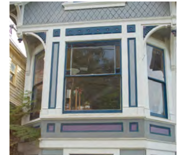
Single hung window with ornamental window surround.
