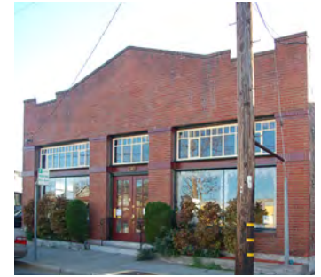
Early 20th century workplace commercial building with divided lite clerestory windows.
