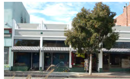
Commercial store fronts.
