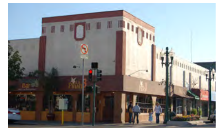
Commercial block building.
