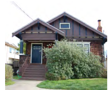
Roof overhangs on a craftsman bungalow reduce solar gain.
