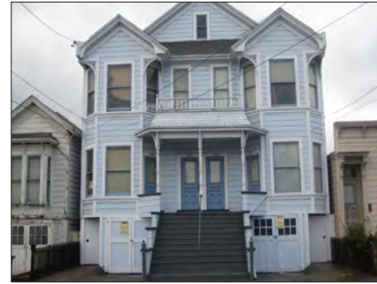
Shared stoop and porch on a multiplex building having four dwelling units.
