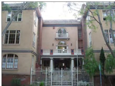
Forecourt serves as shared garden and patio for residents of this villa.
