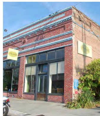
Flat roof with parapet.
