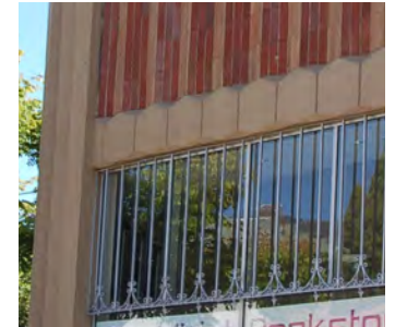
Steel sash window detail.
