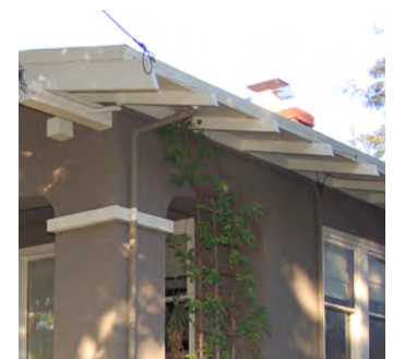
Large eave overhang with exposed rafter tails.
