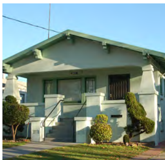
Raised entry porch.
