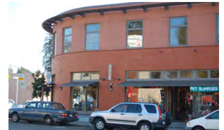
Commercial block building.
