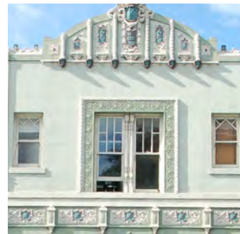
Ornamented window surround and parapet.
