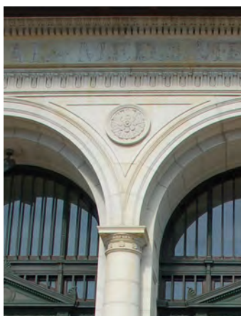
Cast stone medallion in spandrel.
