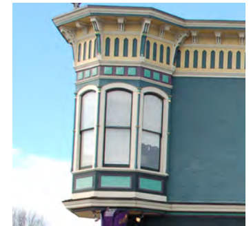
Secondary colors are used to accentuate architectural details.
