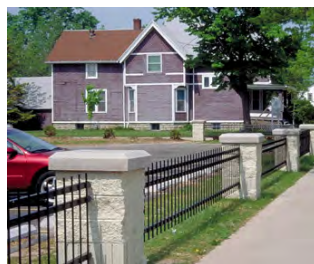
Masonry piers, caps, and ironwork.
