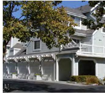
Multiplex building with group of single loaded garage doors.
