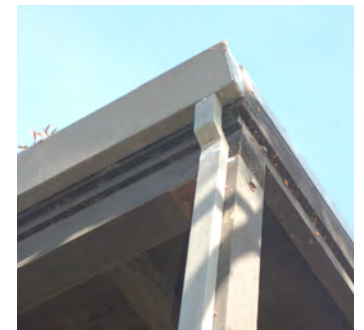
Squared metal gutter and downspout.
