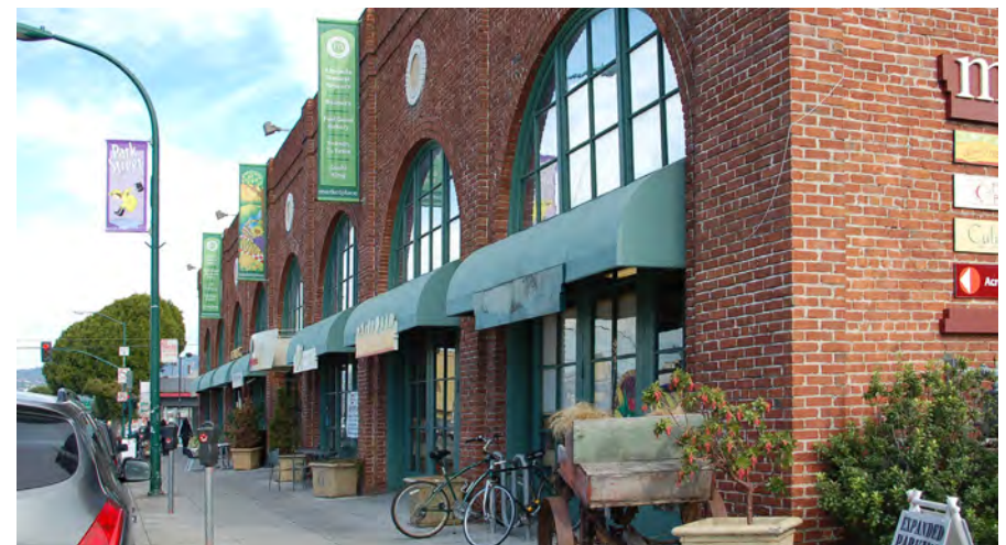
Banner sign is consistent with building articulation and massing.
