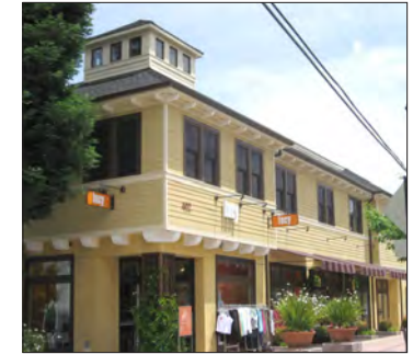
Contemporary building with prominent corner volume.
