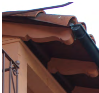
Eave overhang with exposed rafter tails and decorative gutter.
