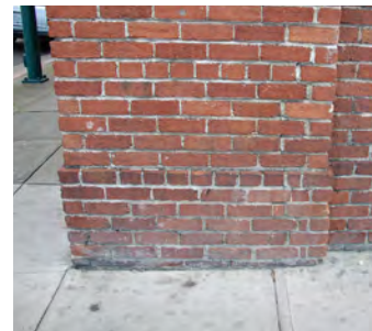
Brick extends to building base.
