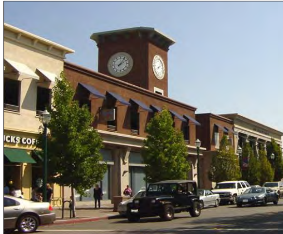
Parking structure with ground floor storefronts. Second story opening are vertically proportioned and include decorative grille-work and shade devices. A combination of brick and stucco accentuates building articulation and creates an attractive setting in a downtown environment.
