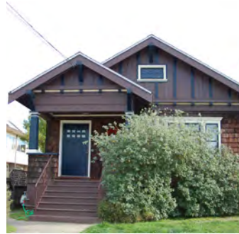
Board and batten used as a secondary material at gable ends.
