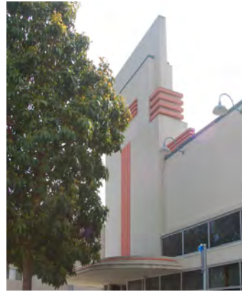
Vertical marquee signage at building corner.
