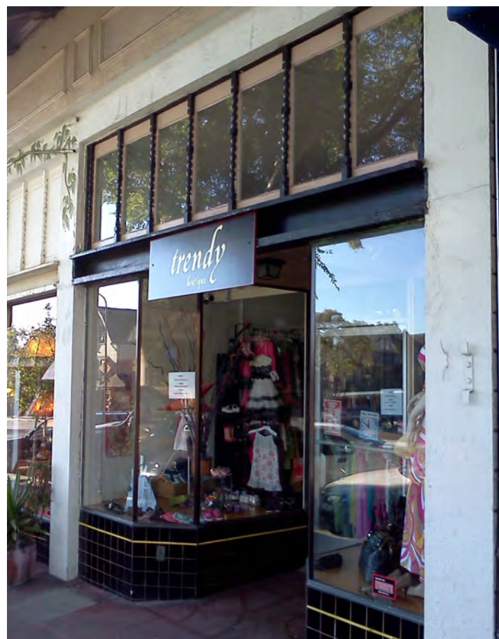
Storefront includes recessed area. Bulkhead treatment includes ceramic tiles.
