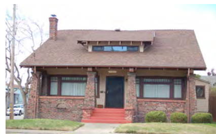
Brick base and shed dormer.
