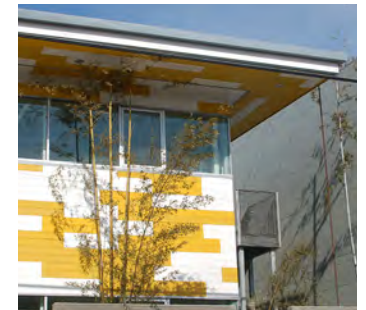
Modern building with fiber cement siding.
