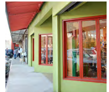
Façade colors used to accentuate storefront windows.
