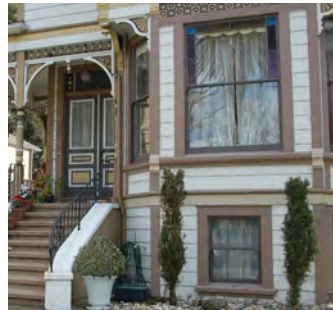
Painted wood siding extends to base.
