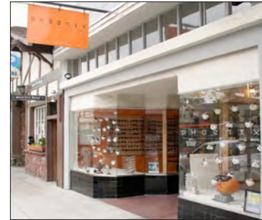
Bulkhead, display windows, transom windows, and blade sign.
