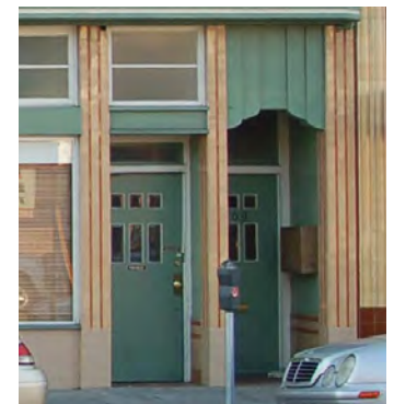
Pilasters frame building entries.
