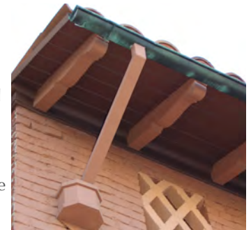
Half round copper gutter and decorative conductor head.
