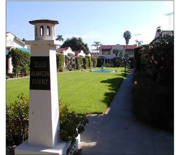
Primary pedestrian entry to this bungalow court is treated with formal landscaping and accented with a pedestrian-scale gateway monument.
