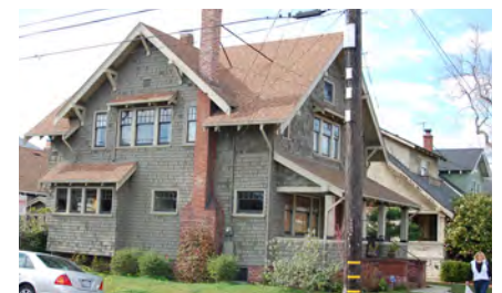
Multiplex with grouped windows.
