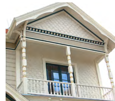
Balcony railing detail with turned wood balusters.
