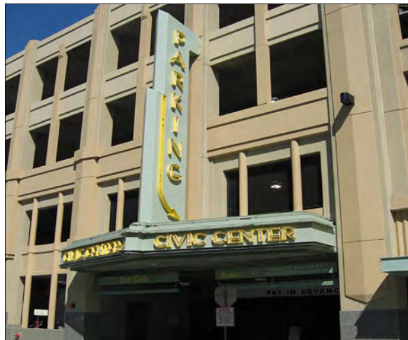
A marquee sign announces entry to Alameda's downtown parking structure. Vertically oriented recesses and voids mimic existing buildings in the historic downtown.
