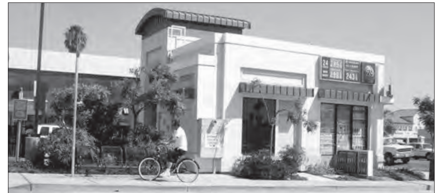
Retail building located at back-of-sidewalk. Fuel pumps located within lot interior.
