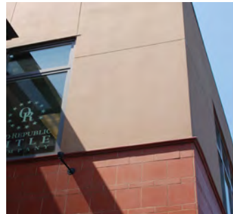
Smooth stucco and terracotta tiles applied to a modern building.
