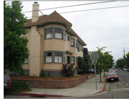
Multiplex building with terraced frontyard retained by decorative wall.
