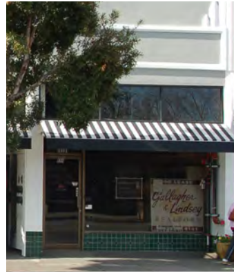
Stucco wall surface with ceramic glazed tile base treatment.
