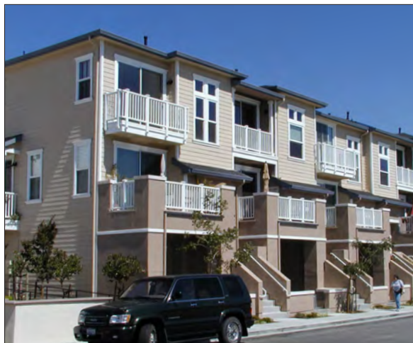
Modern rowhouses with stoops. Upper story terraces enhance neighborhood character.
