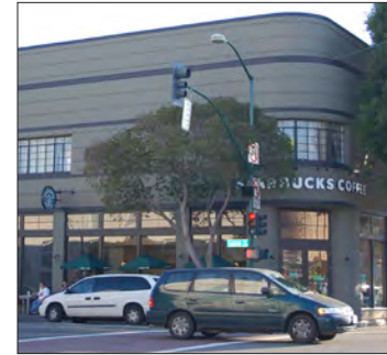
Traditional commercial block building with corner entry.
