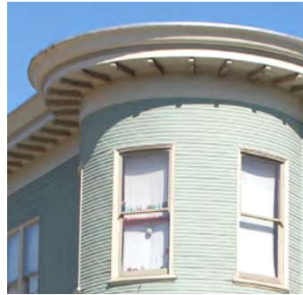
Eave overhang with decorative brackets.
