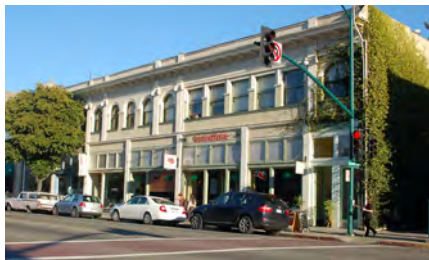
Commercial block building.
