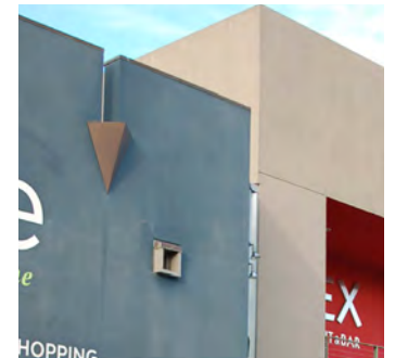
Parapet roof with geometric shaped conductor head.
