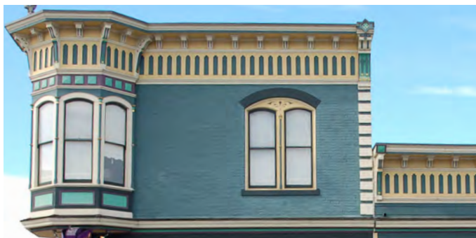
Ornamental relief and cornice detail.
