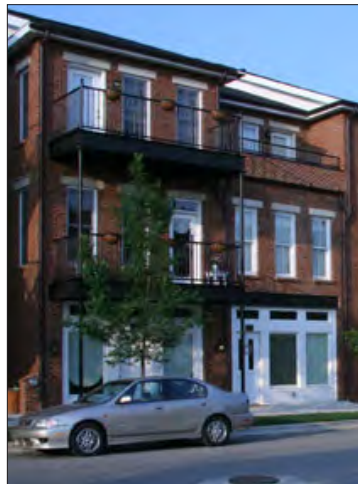
Three-story live-work units with ground floor commercial space.
