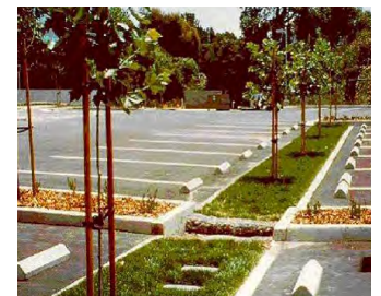
Curbsless bioswale water infiltration and detention system internal to parking lot.
