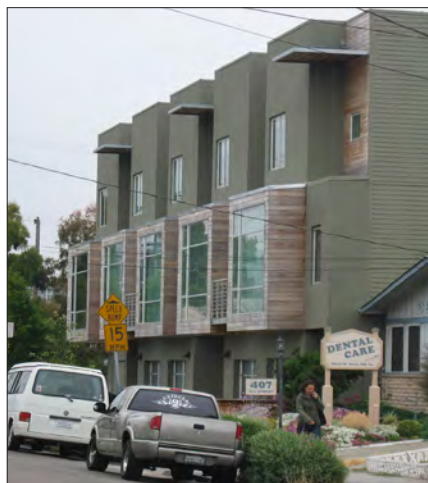
Rowhouses containing residential lofts. Gardens at rear of building provide a mix of private and shared open space.
