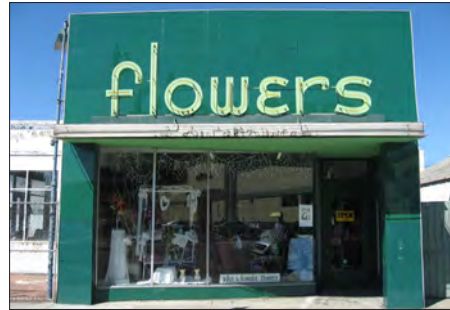
Bulkhead omitted on Deco building in favor of enlarged display windows, minimal base treatment, and recessed entry.
