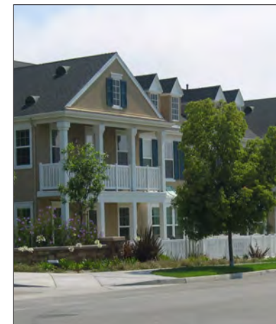
Colonial Revival multiplex with frontyard and decorative fence.
