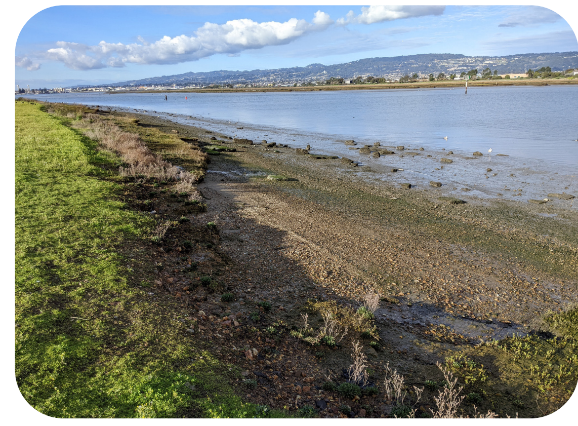
Erosion of fringe marsh at Sea View Park
