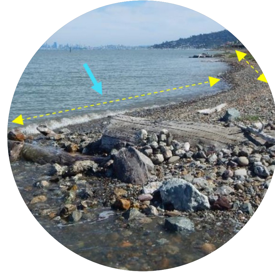
Rock and Wood Groins: Rock, cobble, and large woody debris shaped into 'groins' help to catch drifting beach material at Aramburu Island in Richardson Bay.
