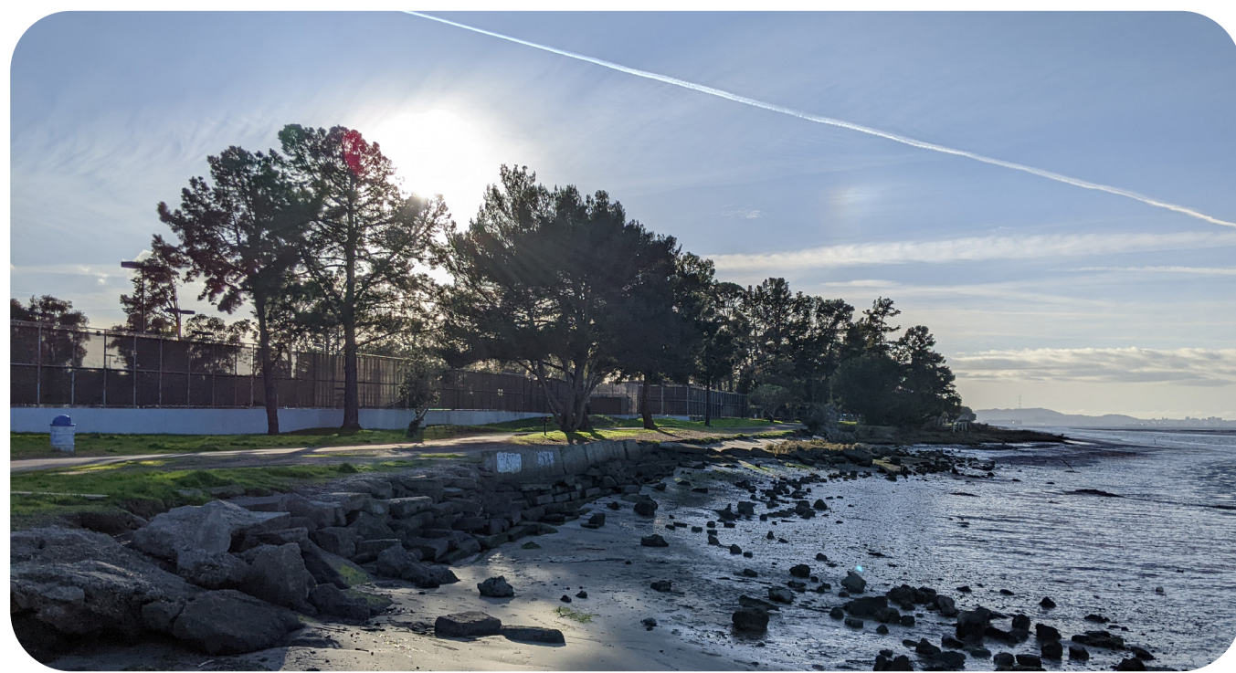
Erosion in front of Harbor Bay Club
