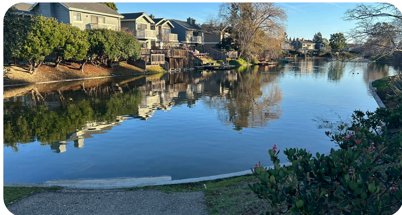
Bay Farm Island lagoon at pump station
