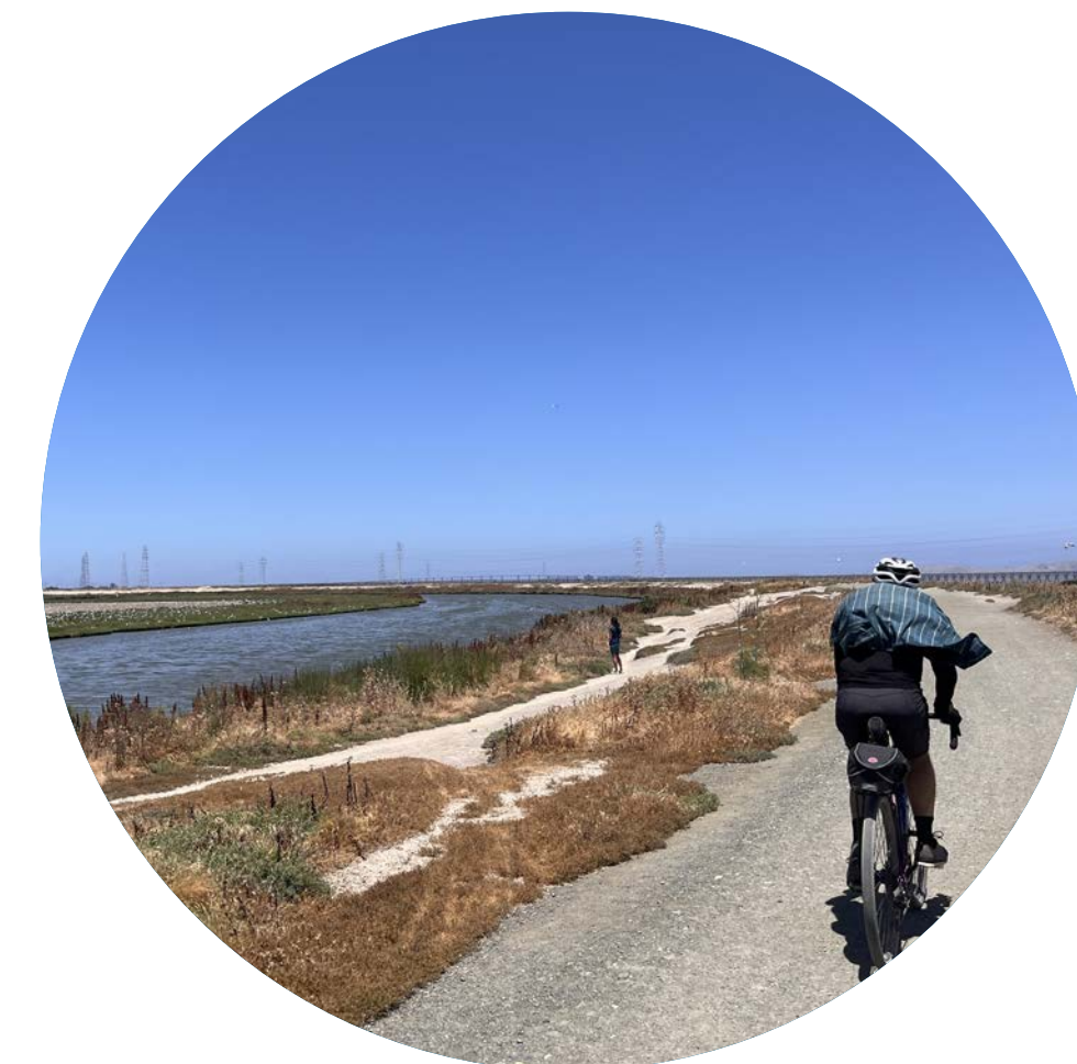
Levee with Public Access SF Bay Trail
