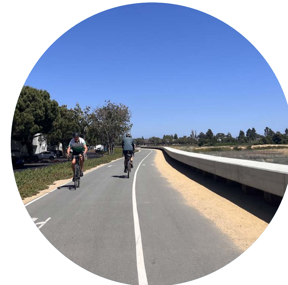
Seawall at Foster City
