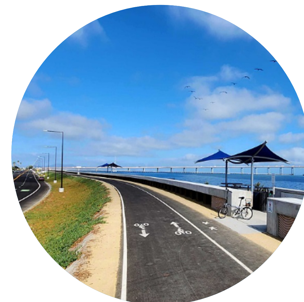
Levee with Seawall Foster City
