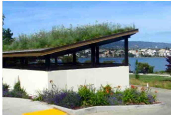
Pump Station Building Precedent
