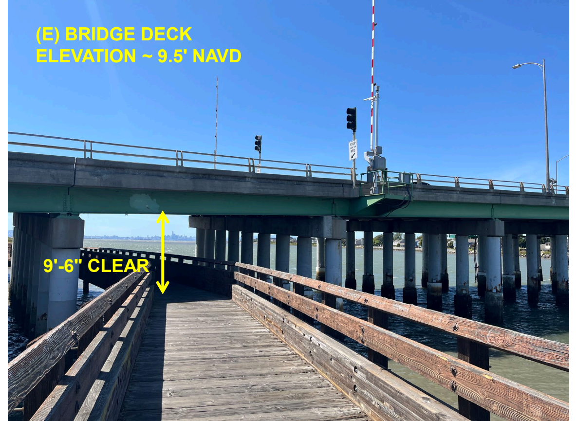
EAST SIDE (looking west)
