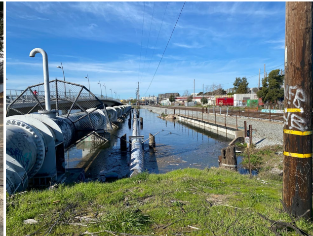
Embarcadero West Bridge over Lake Merritt Channel
