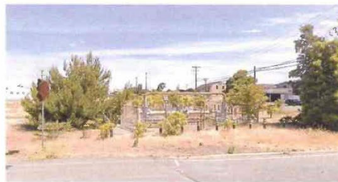
2. PG&E GAS FACILITY
