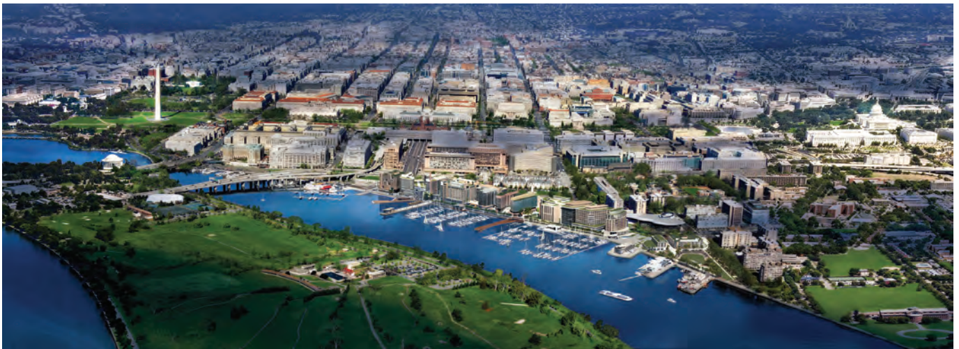
Madison Marquette’s The Wharf project in Washington D.C. This project has similar qualities to Alameda Point’s waterfront.
