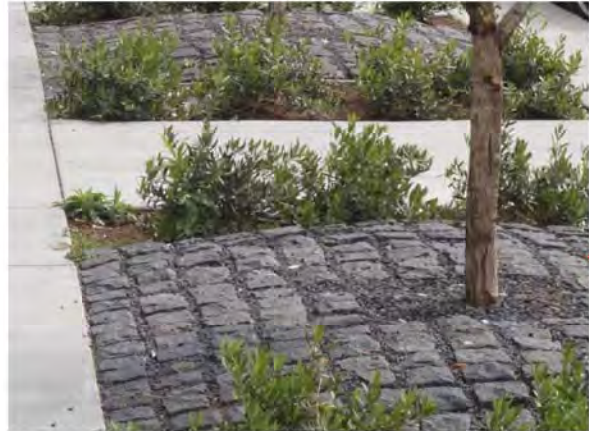
STONE COBBLES AT TREE WELLS
