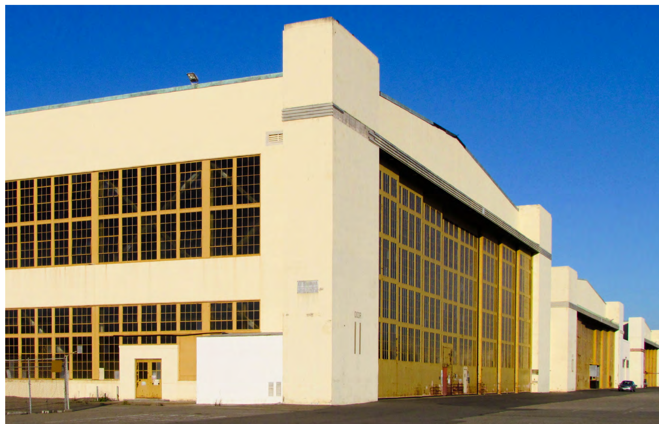
HANGARS WITH STRONG VERTICAL BOUNDING MASSES PUNCTUATE THE MAIN ROAD
