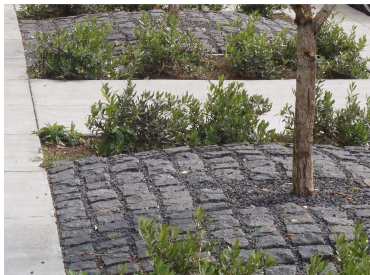
STONE COBBLES AT TREE WELLS
