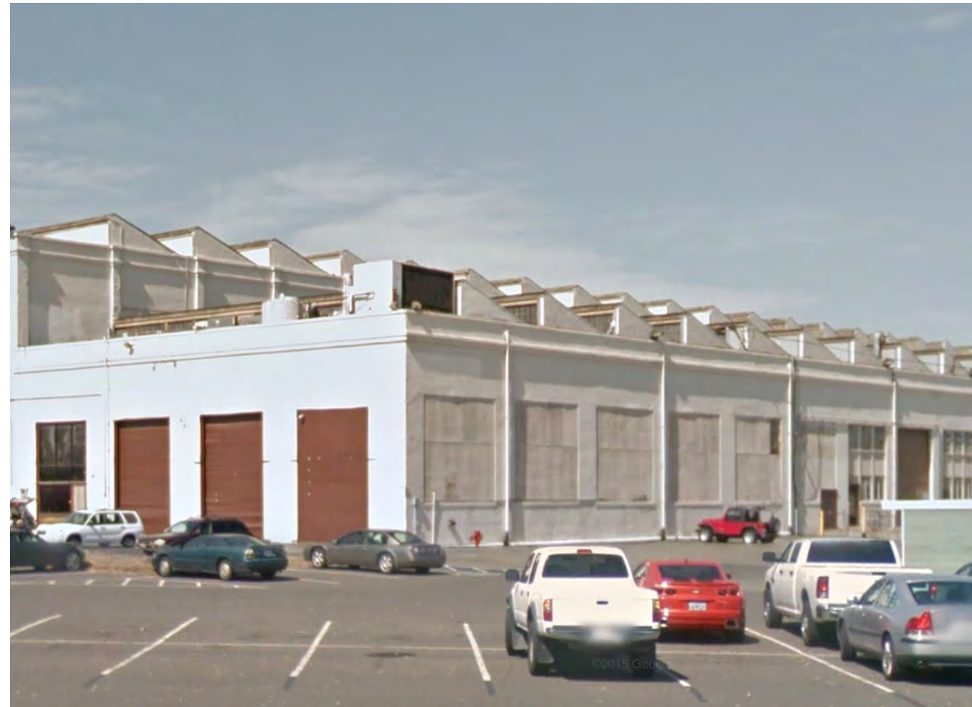
SAWTOOTH ROOFS OCCUR ACROSS THE TOPS OF SURROUNDING HANGARS AND OTHER NEIGHBORING FACILITIES
