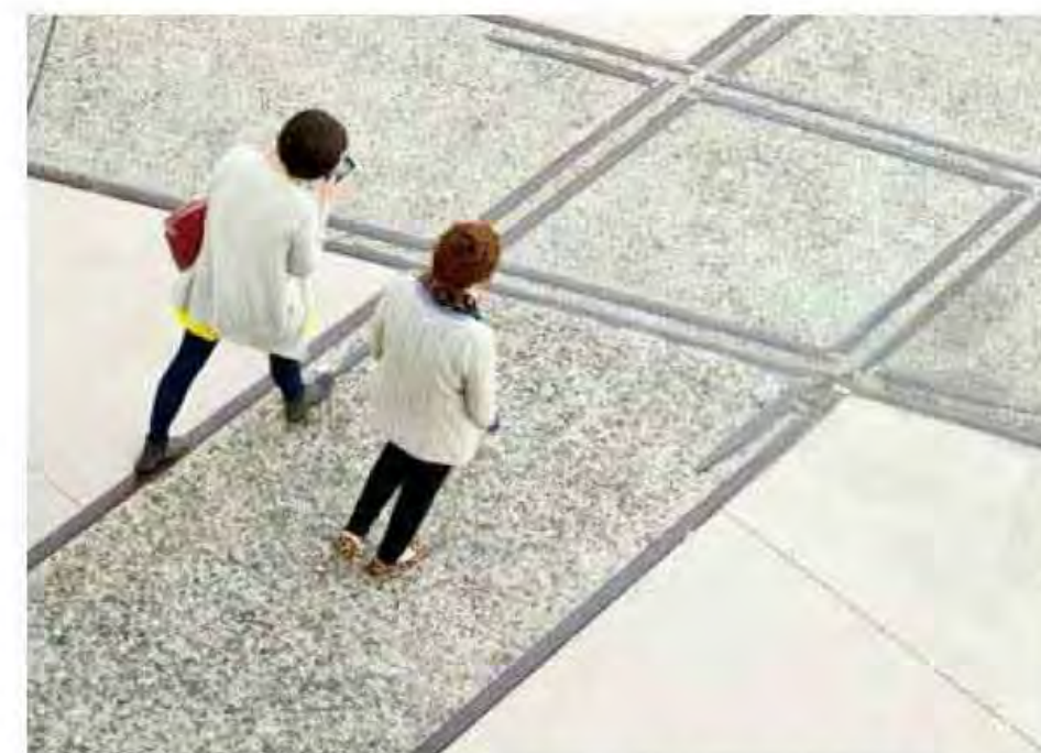
Rail Track in Concrete
