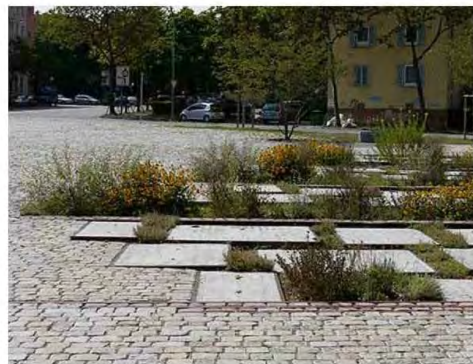
"Eroding" Stormwater Treatment Area
