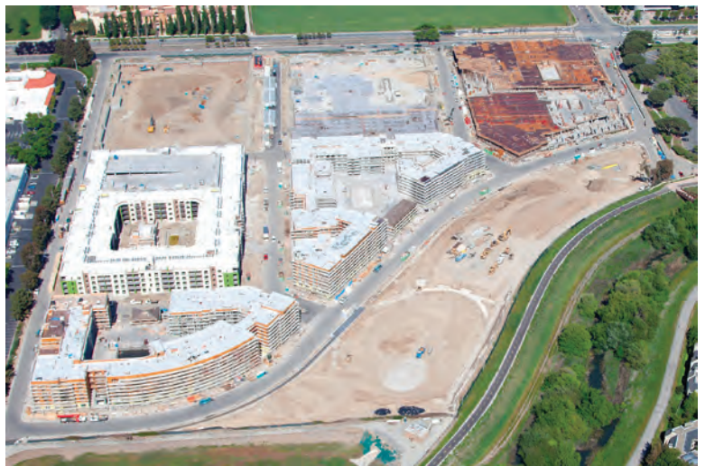
Riverview during construction
