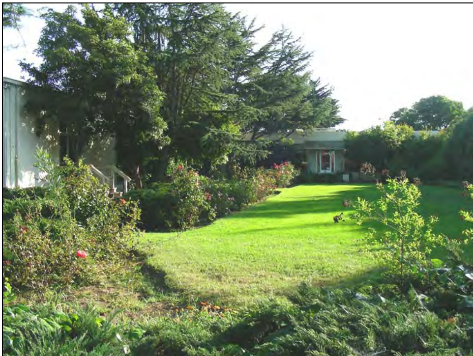
Photograph 9: North side of west wing, camera facing south, November 12, 2009.
