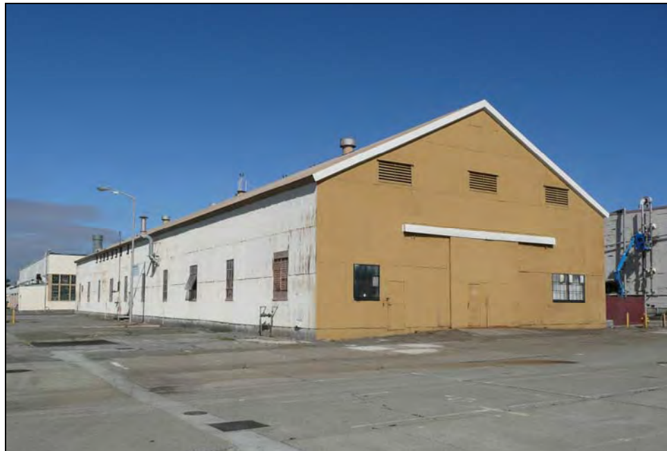
Photograph 2: Camera facing northeast, October 15, 2009.
