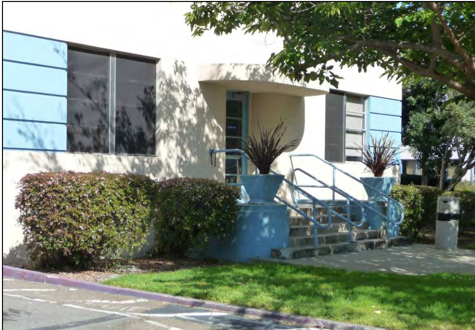
Photograph 4: Building 1, east wing south entrance, camera facing northeast, October 6, 2009.
