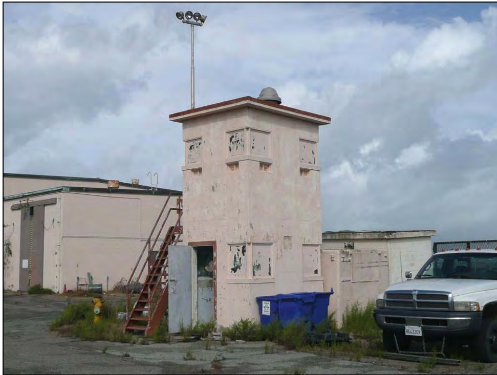
Photograph 6: Building 440, camera facing west, October 14, 2009.
