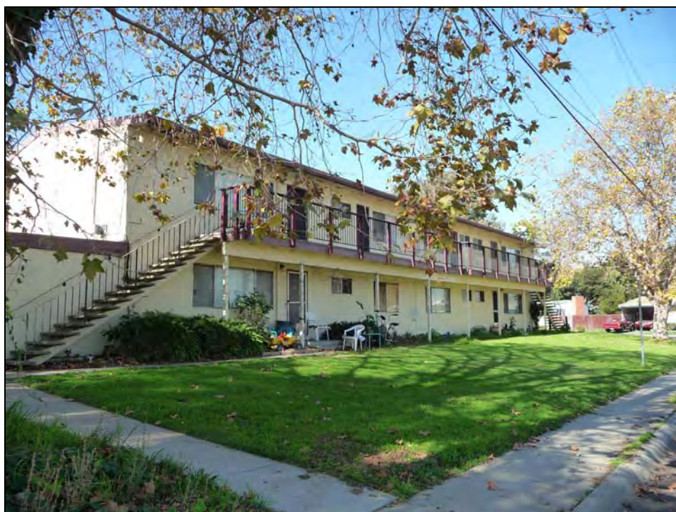
Photograph 10: 2D and 3E plan, Building 738, camera facing southwest, November 3, 2009.
