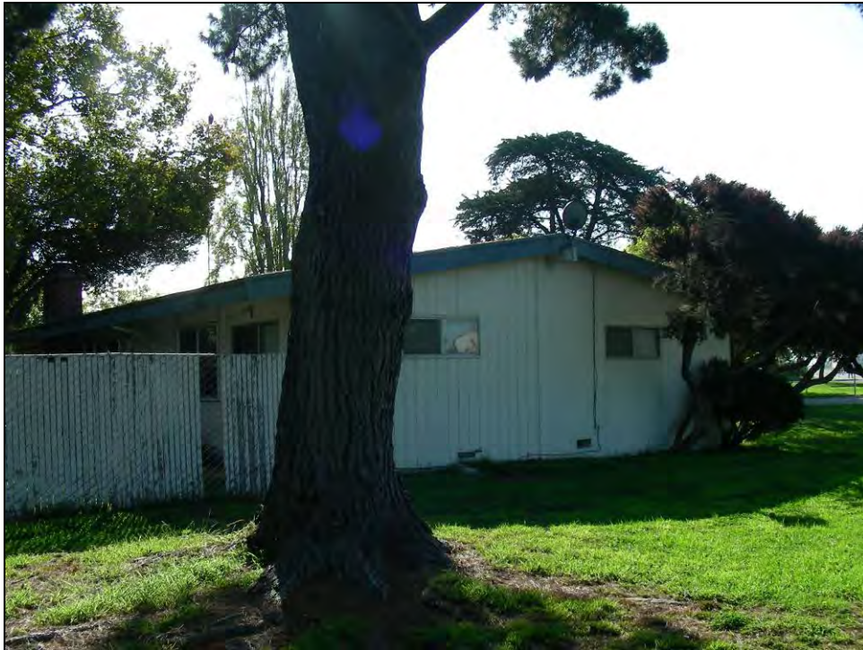
Photograph 8: Alteration to recessed area, FH-775, camera facing southeast, November 12, 2009.
