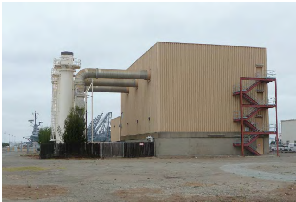
Photograph 57: Pier Utility Boiler Plant (Building 584), October 8, 2009.
