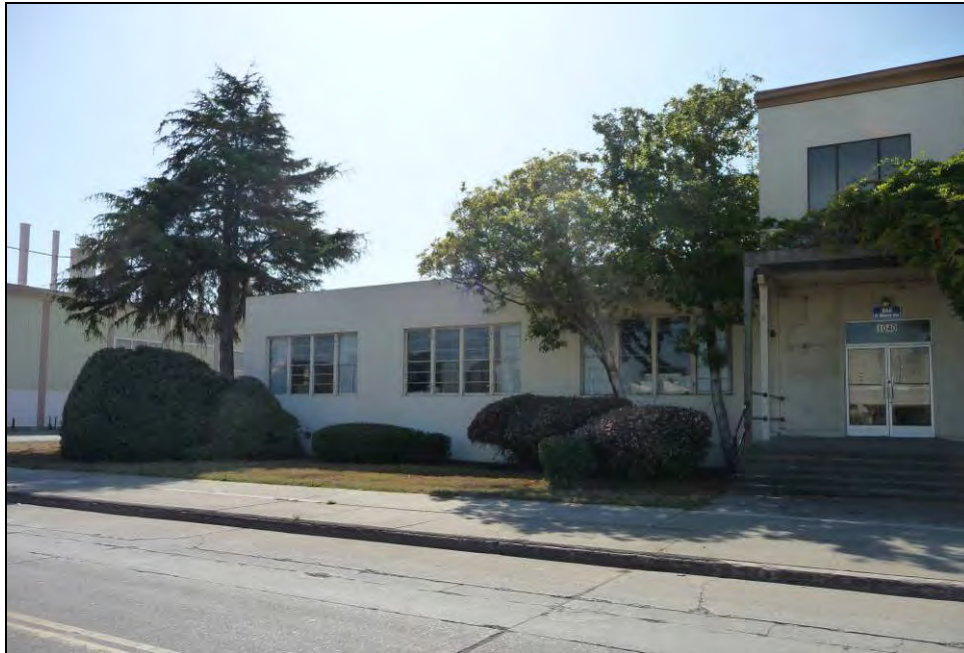
Photograph 6: Northeast side, camera facing northwest, October 6, 2009.
