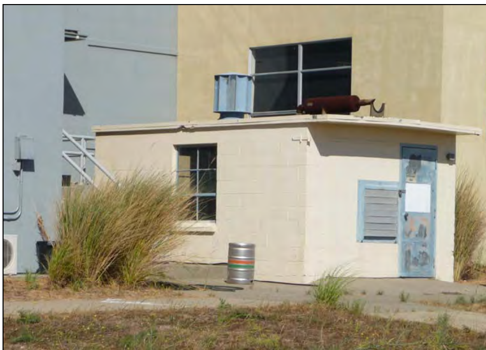
Photograph 2: Building 491, camera facing northeast, September 29, 2009.
