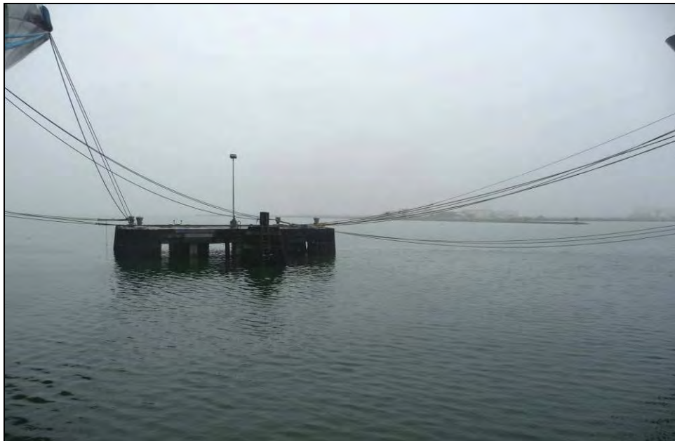
Photograph 8: Building 434 (dolphin), camera facing west, December 16, 2009.
