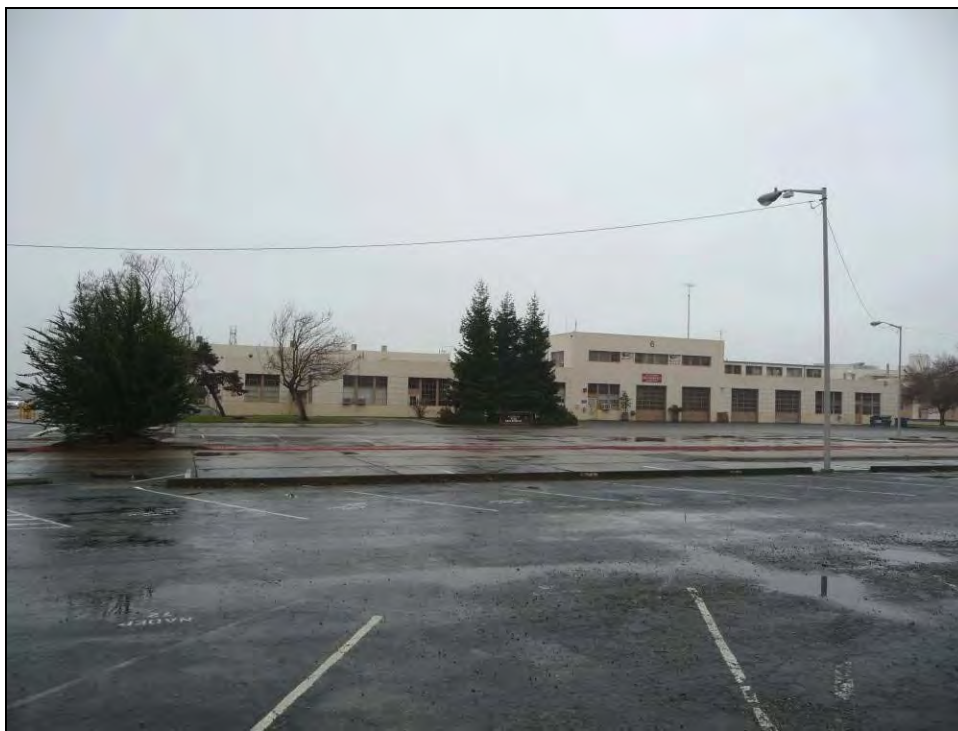
Photograph 1: North wing, camera facing southwest, October 8, 2009.
