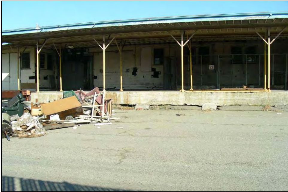
Photograph 8: South side west end of bay, camera facing north, November 12, 2009.
