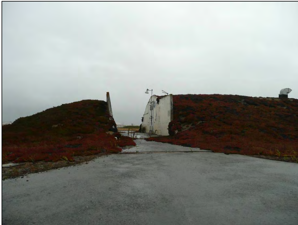
Photograph 5: View through Building 58, camera facing east, October 13, 2009.
