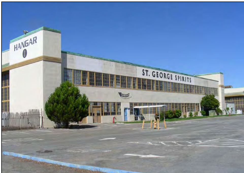
Photograph 4: Hangar 21 east side, camera facing southwest, September 30, 2009.
