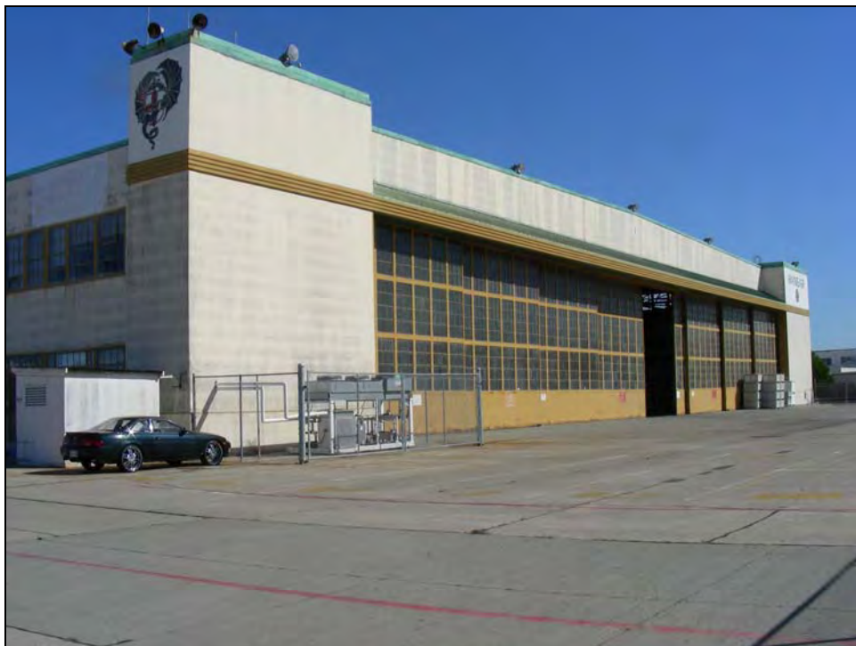
Photograph 2: Hangar 21 south side, camera facing northeast, September 30, 2009.
