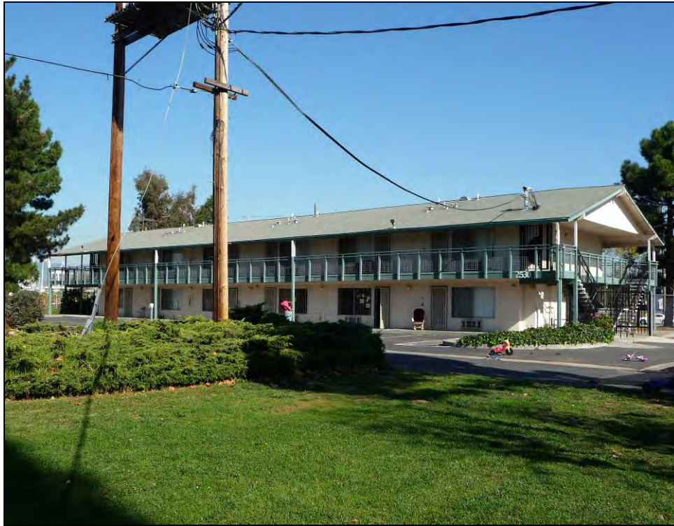
Photograph 3: Building 533, camera facing northeast, November 3, 2009.
