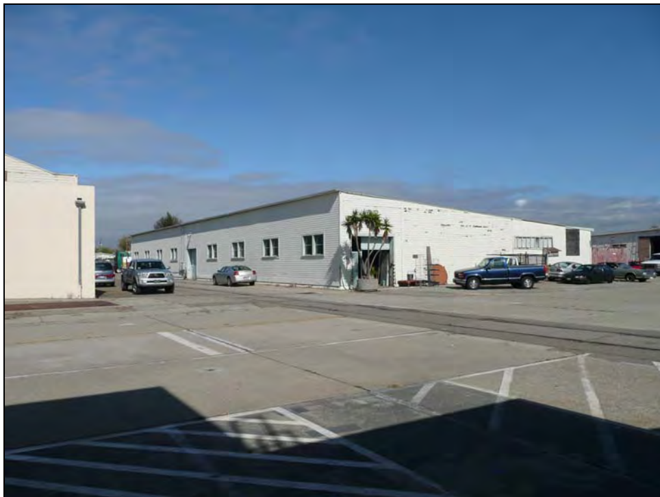
Photograph 2: Southwest corner, camera facing northeast, October 15, 2009.
