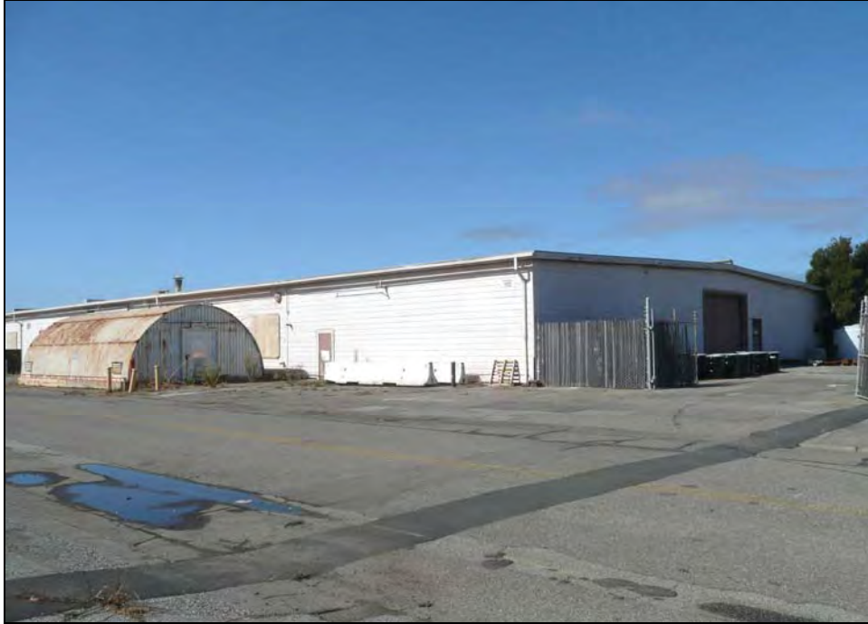
Photograph 1: Camera facing northwest, October 15, 2009.
