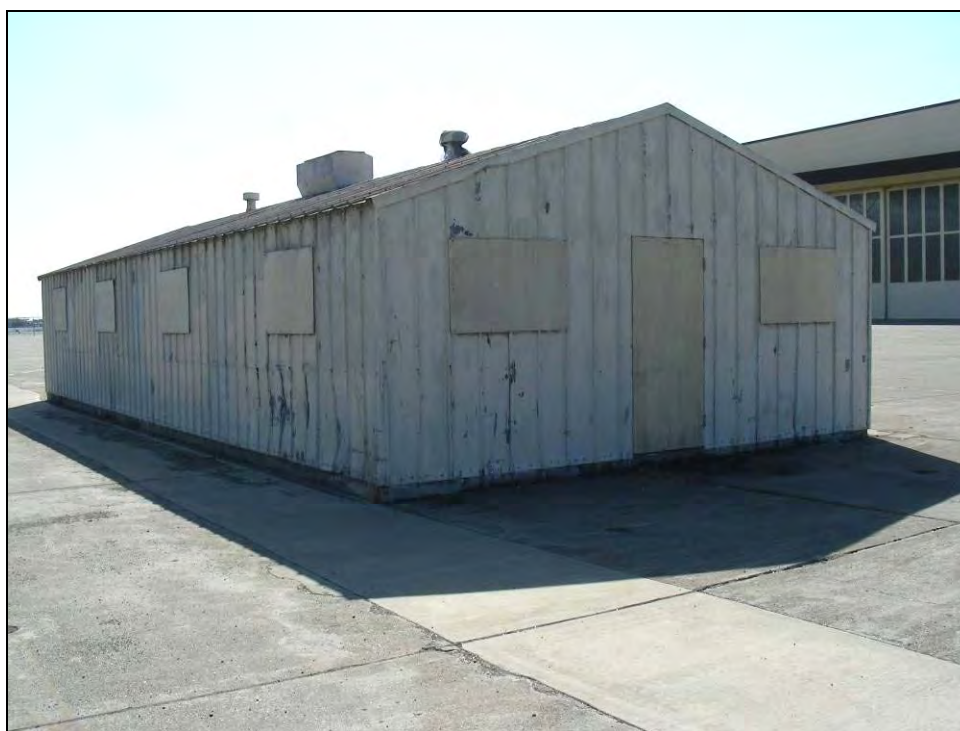
Photograph 2: Camera facing southwest, October 8, 2009.
