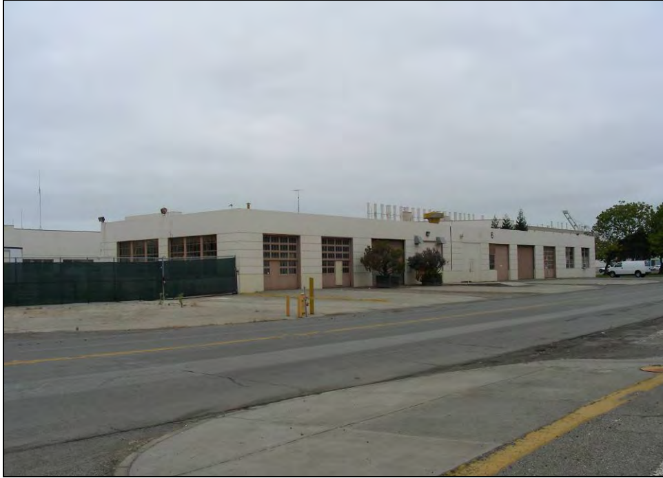
Photograph 8: East wing, camera facing northwest, October 8, 2009.
