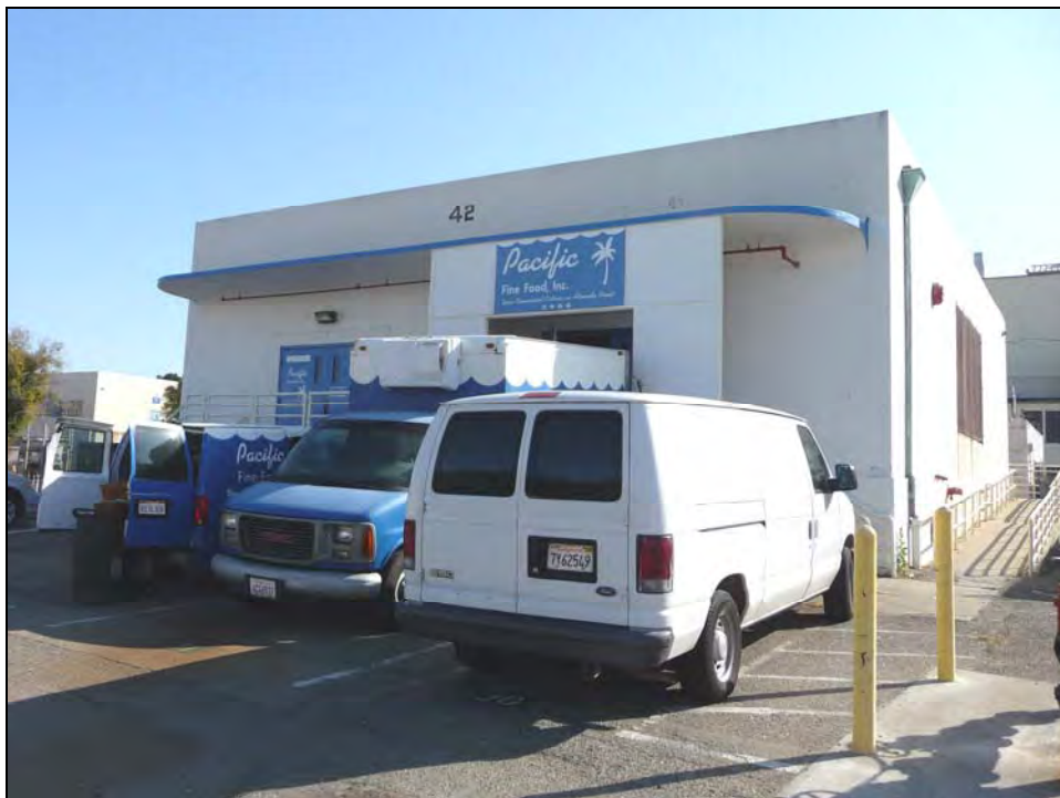
Photograph 2: West side, camera facing northeast, October 6, 2009.
