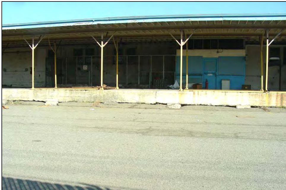
Photograph 7: South side bay, camera facing north, November 12, 2009.
