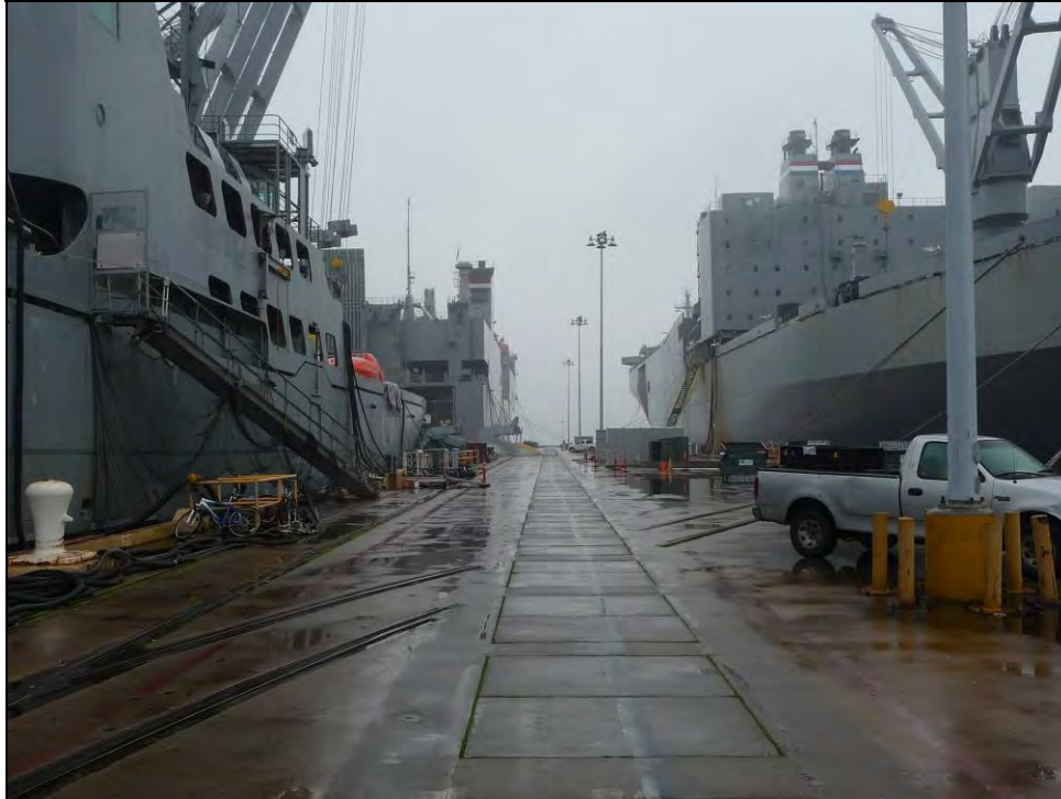
Photograph 2: Railroad tracks at Pier 2, camera facing West, December 16, 2009.
