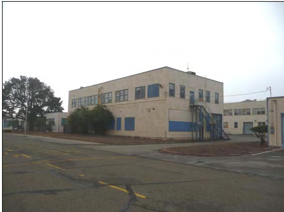
Photograph 2: North end, camera facing southwest, December 16, 2009.
