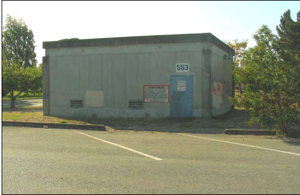
Photograph 2: Typical small substation, Building 553, Electrical Substation No. 6, camera facing southeast, October 9, 2009.
