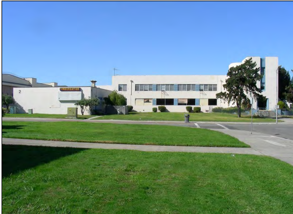
Photograph 9: Wing 20 Building 2, camera facing west, October 7, 2009.
