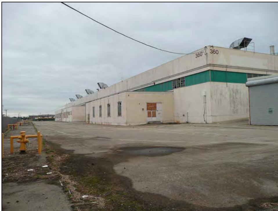
Photograph 4: Showing east side, camera facing southwest, October 15, 2009.
