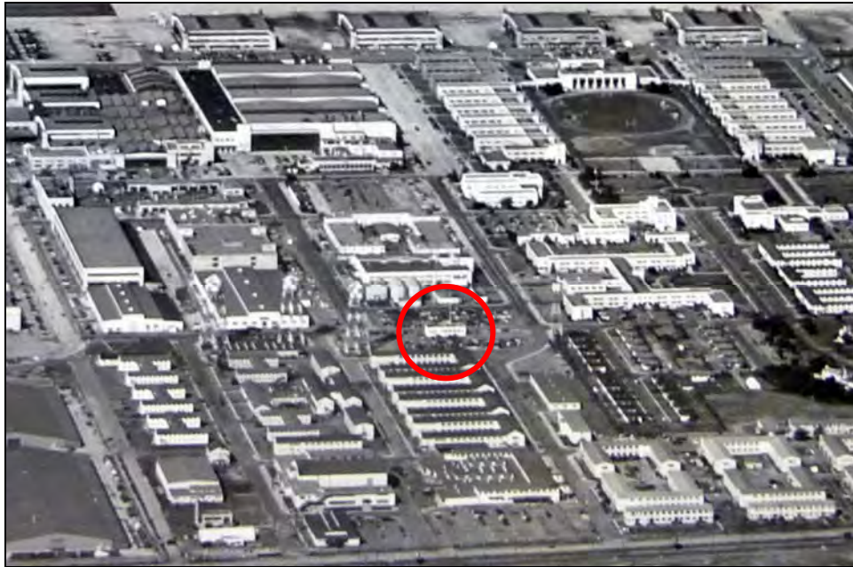
Photograph 7: NAS Alameda, ca. 1952. Building 35 in red circle. 11
