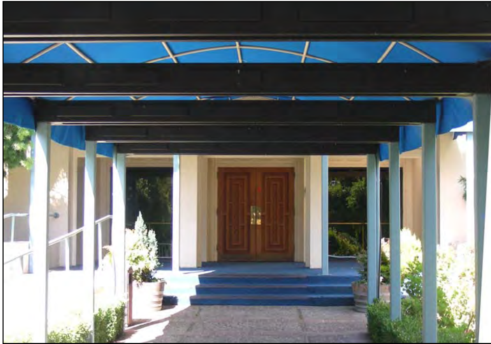
Photograph 2: South entrance detail, camera facing north, September 29, 2009.
