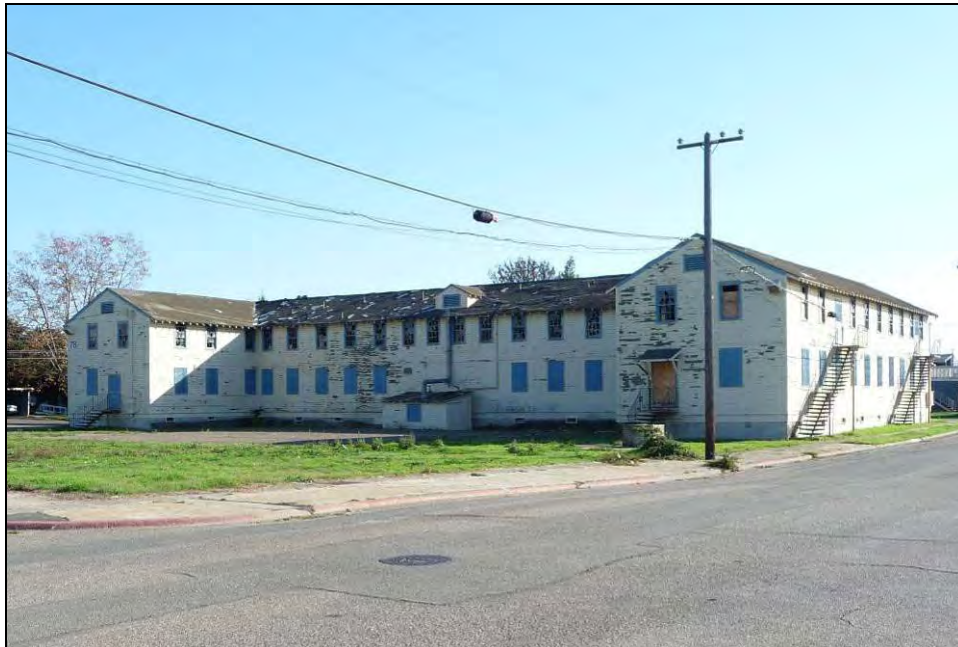
Photograph 48: WAVES Barracks (Building 78), November 4, 2009.
