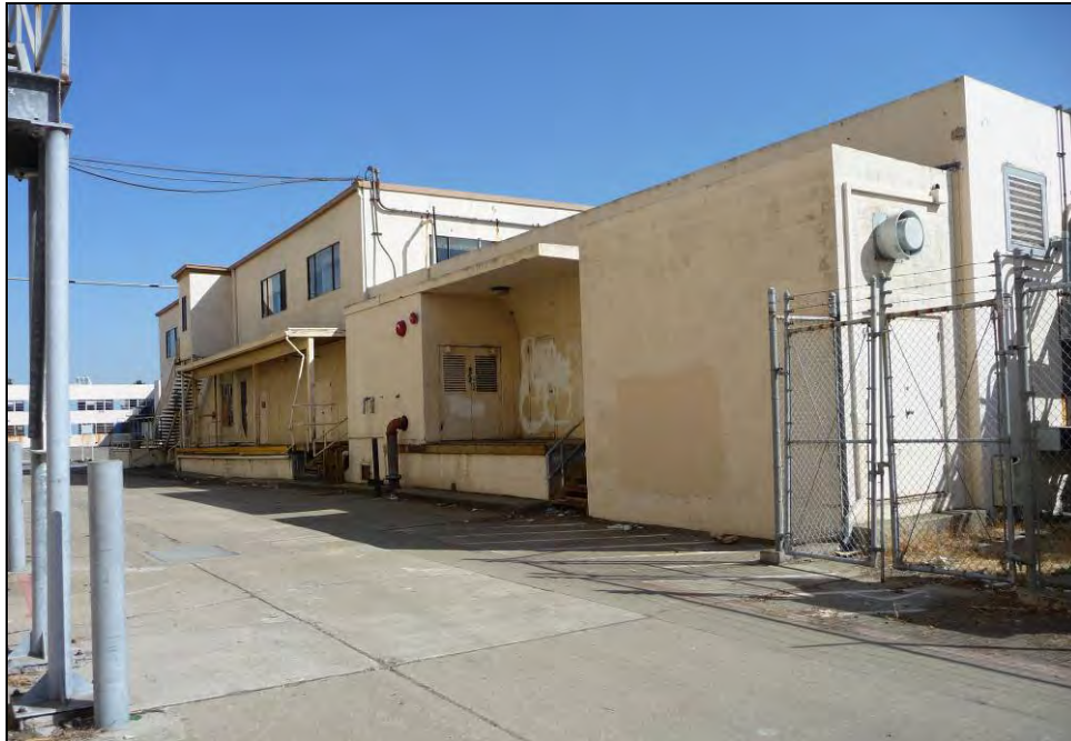
Photograph 4: West side, camera facing northeast, October 6, 2009.
