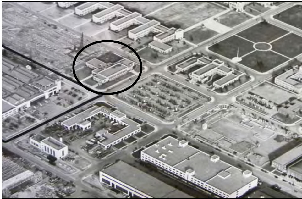
Photograph 9: January 1, 1944 photo showing Building 62 before northwest addition. 2
