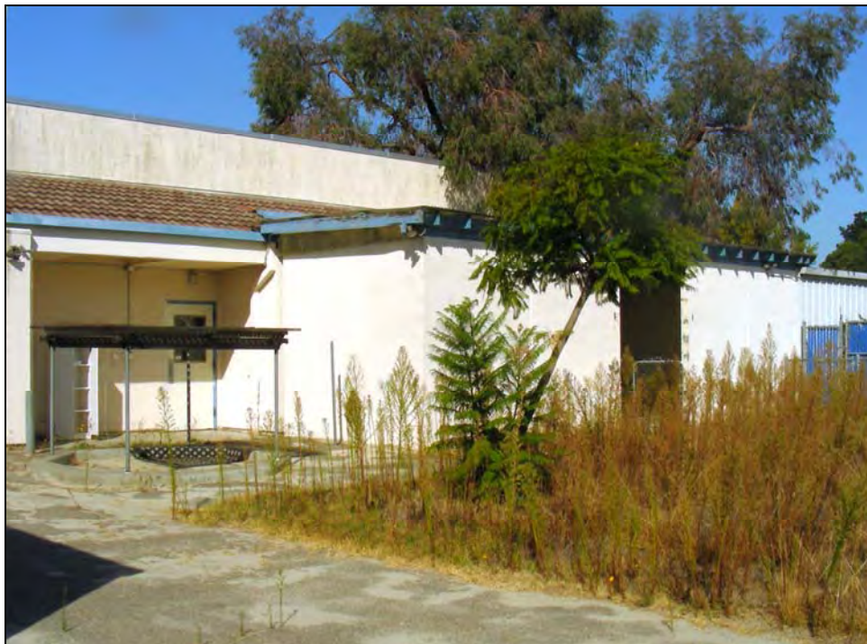
Photograph 3: Building 585 east side, facing northwest, October 6, 2009.
