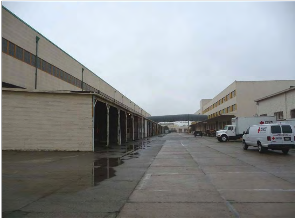
Photograph 5: North side of Building 9 connected to south side of Building 8 with metal skywalk, camera facing west, December 16, 2009.
