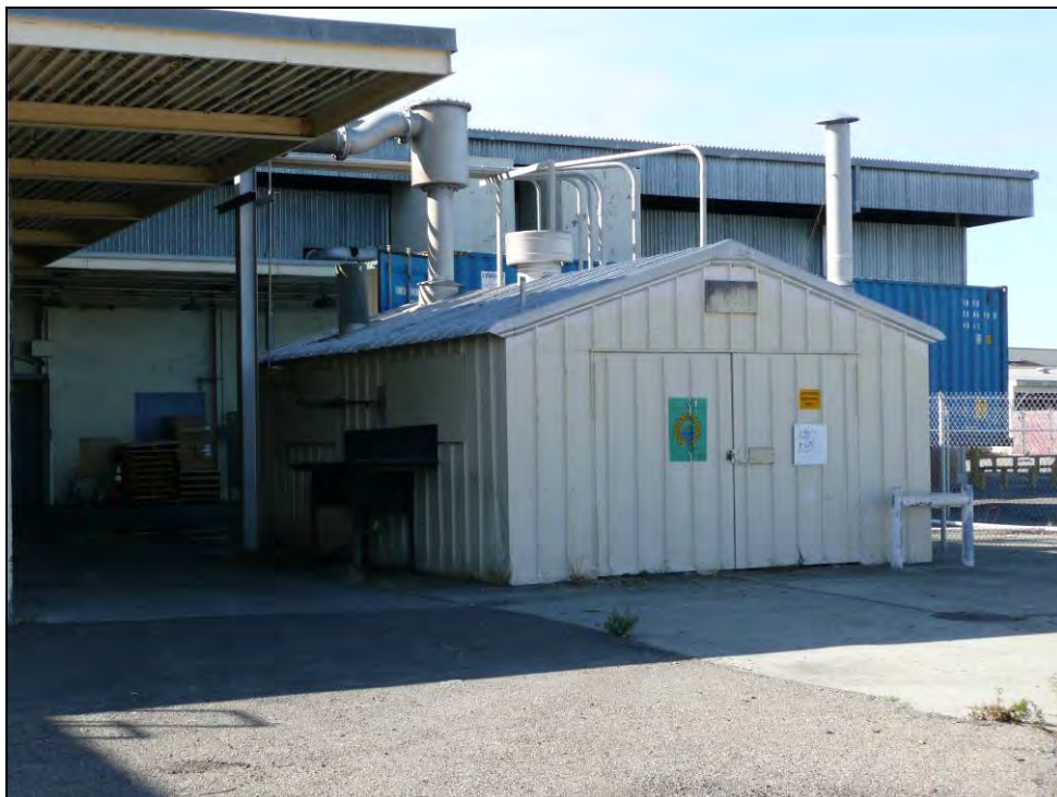
Photograph 3: Building 470, camera facing northwest, October 15, 2009.
