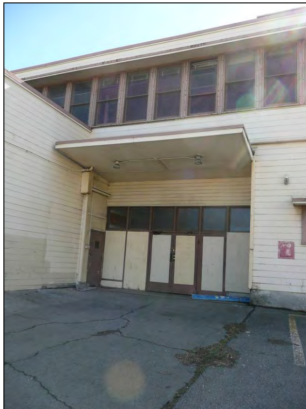
Photograph 3: North entrance detail, camera facing south, October 15, 2009.
