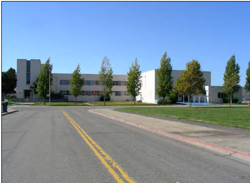
Photograph 10: Wing 20 Building 2, camera facing west, October 7, 2009.
