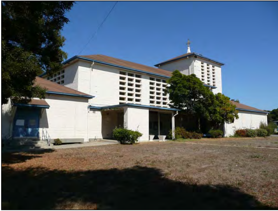
Photograph 2: Camera facing northeast, showing southern entry porch, September 25, 2009.
