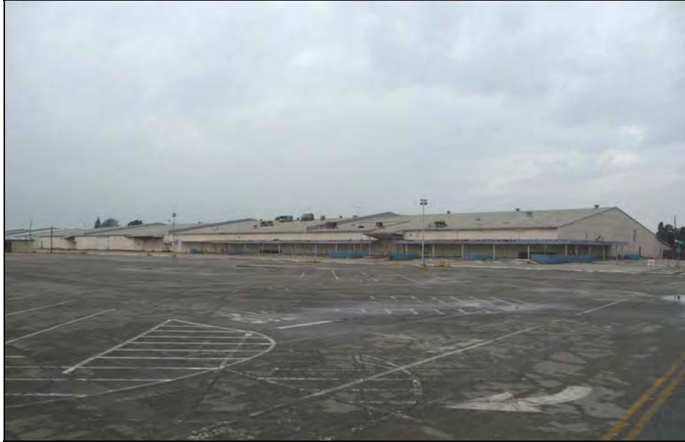
Photograph 2: Camera facing northwest, showing south side, October 15, 2009.
