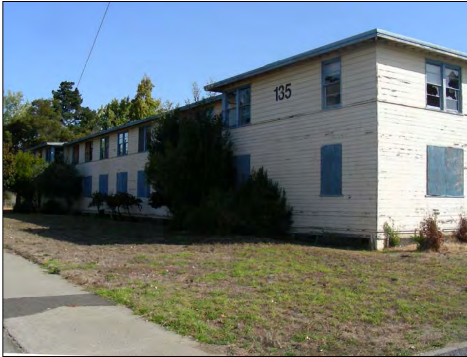
Photograph 5: Building 135, west side of west wing, facing northeast, October 6, 2009.
