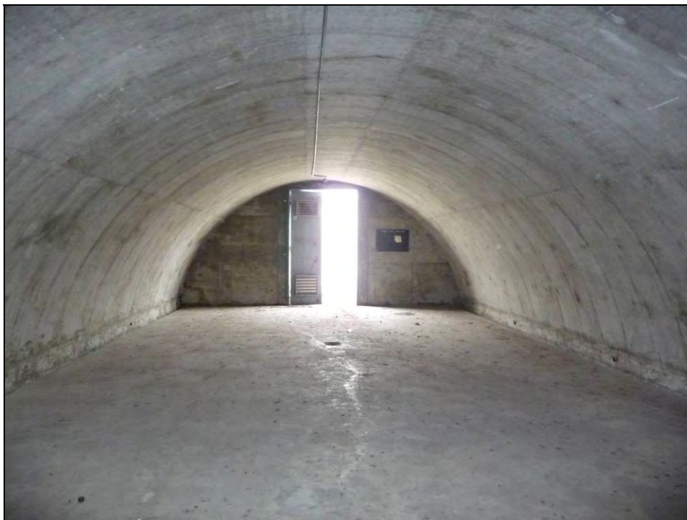
Photograph 6: Interior of Building 56, camera facing north, December 16, 2009.
