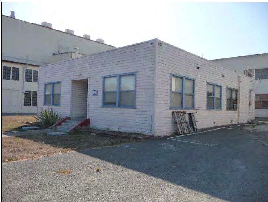
Photograph 3: Camera facing southeast, October 6, 2009.
