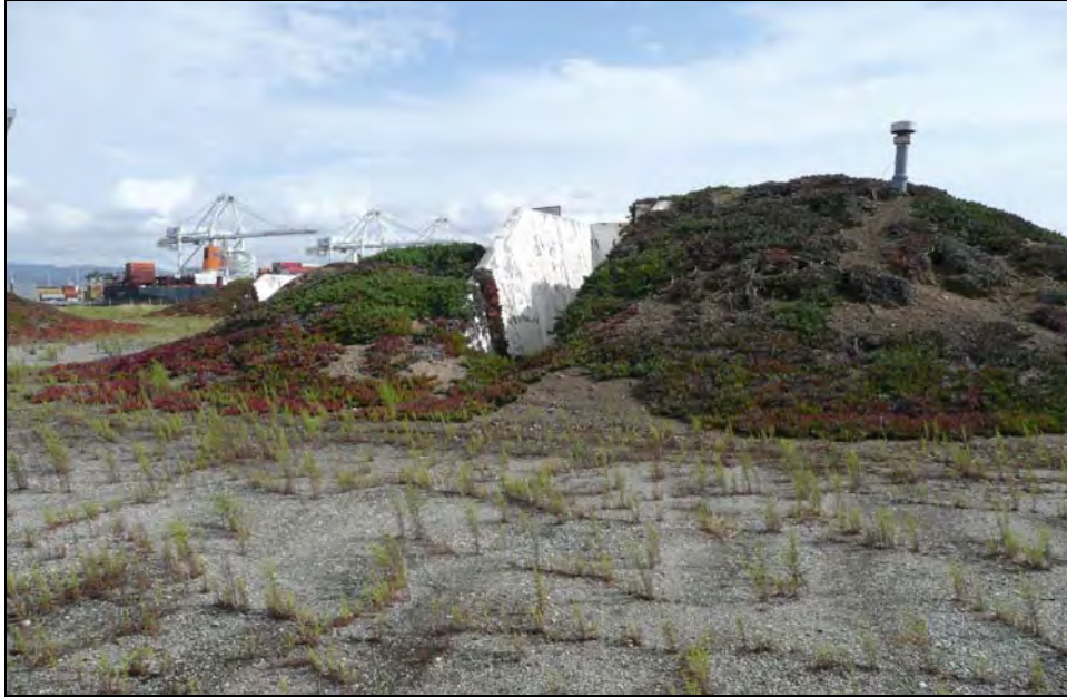
Photograph 2: Building 358, camera facing northeast, October 14, 2009.
