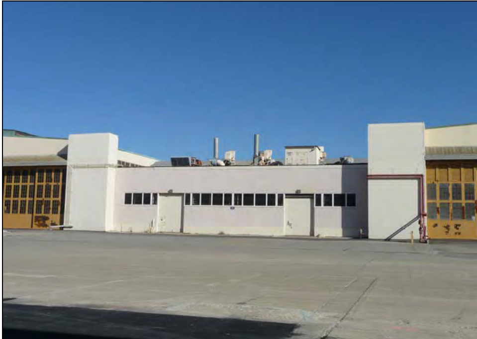
Photograph 11: Area between Door 10 and Entrance Zone 2, rebuilt after removal of 1943 addition, camera facing north, September 29, 2009.
