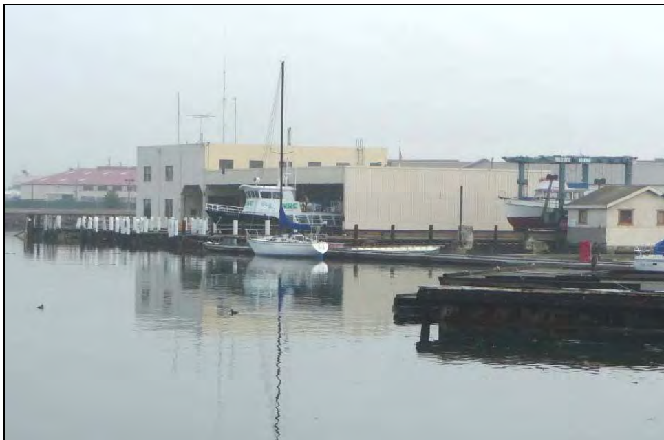
Photograph 4: Camera facing northeast, December 16, 2009.
