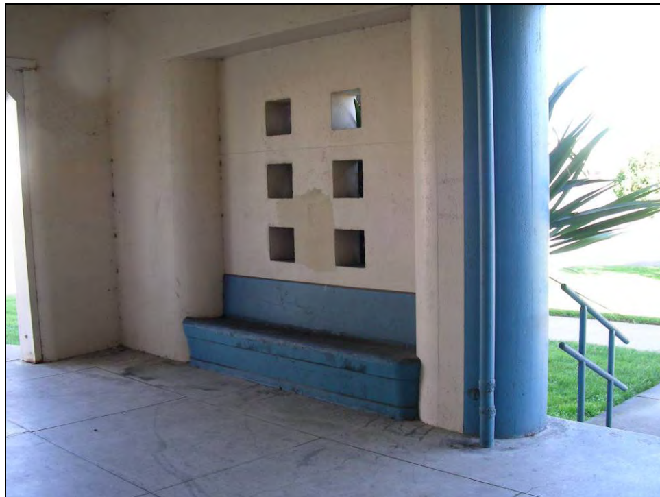
Photograph 4: Built in bench along colonnade, camera facing northwest, October 7, 2009.
