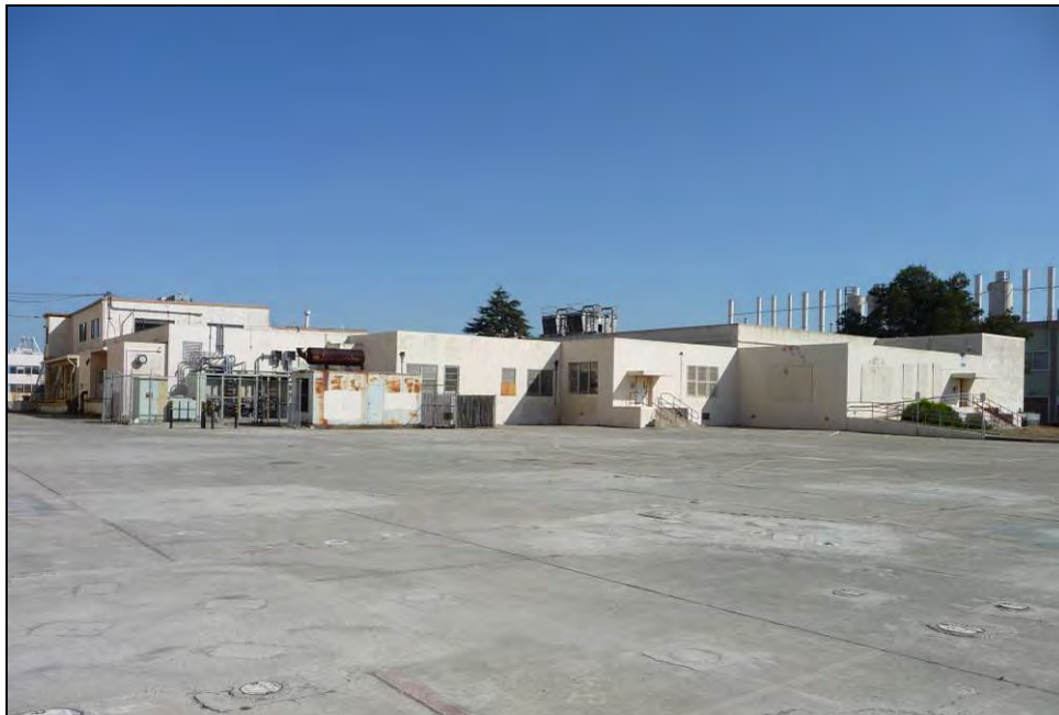
Photograph 3: Southwest corner, camera facing northeast, October 6, 2009.
