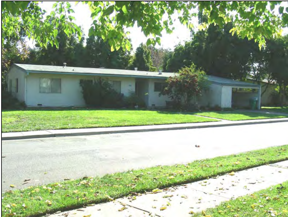
Photograph 2: Typical Plan A, Building FH-736, camera facing south, November 12, 2009.
