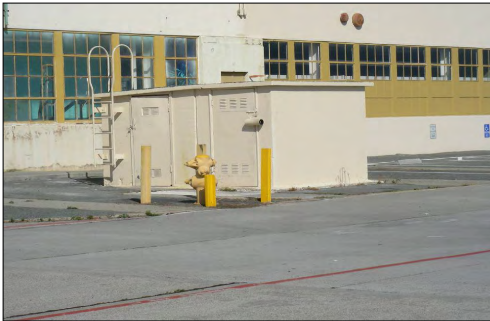
Photograph 2: Building 308, camera facing northeast, October 8, 2009
