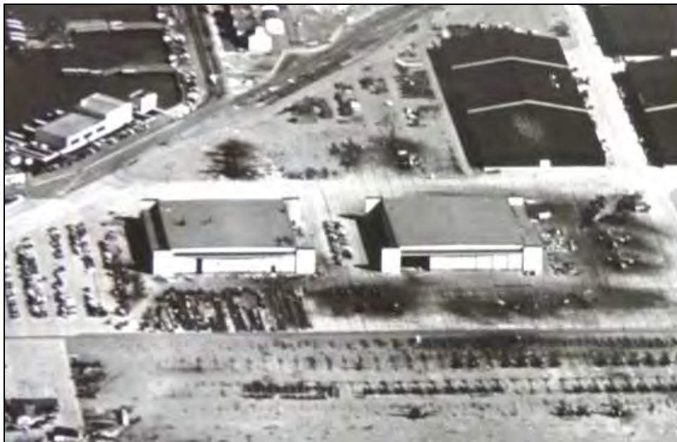
Photograph 5: Circa 1953 aerial photograph of Buildings 166 and 167 – note oil-stained area around Building 166. 7
