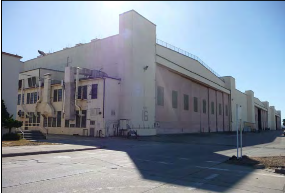
Photograph 3: North side of Building 5 showing three hangar type doors (from left to right Door 16, Door 15 and Door 14), camera facing southwest, September 29, 2009.
