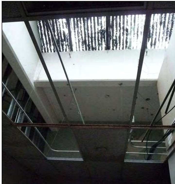
Photograph 8: Exposed light well next to dropped ceiling, interior Building 3, December 11, 2009.
