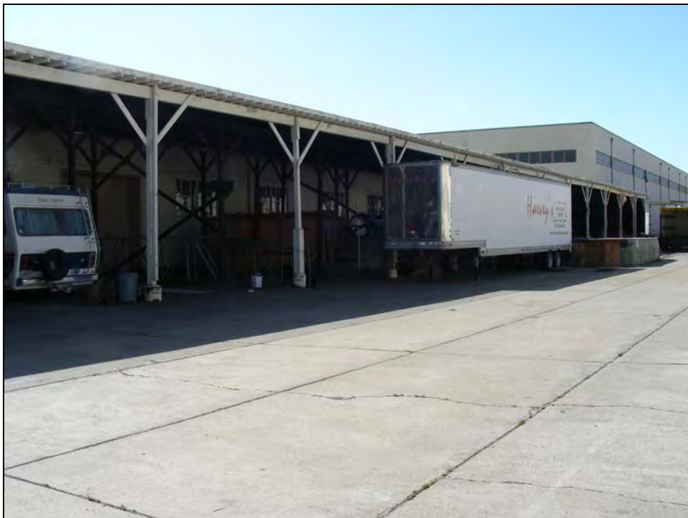
Photograph 4: Detail on north side, camera facing southwest, October 8, 2009.
