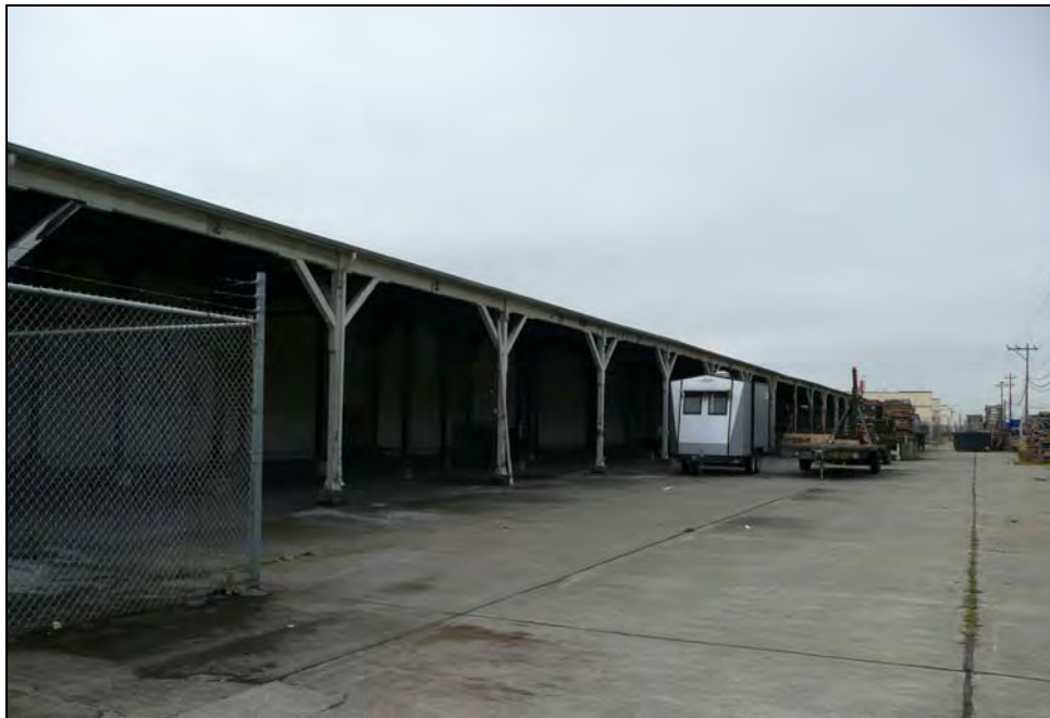
Photograph 2: Showing open bays, camera facing southwest, October 15, 2009.
