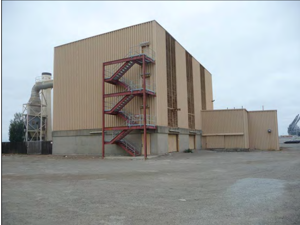
Photograph 2: Building 584, facing southwest, October 8, 2009.
