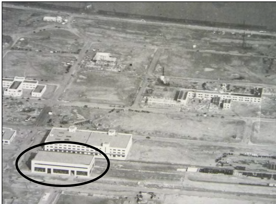
Photograph 6: First phase of Building 9 construction, January 1, 1941. 1
