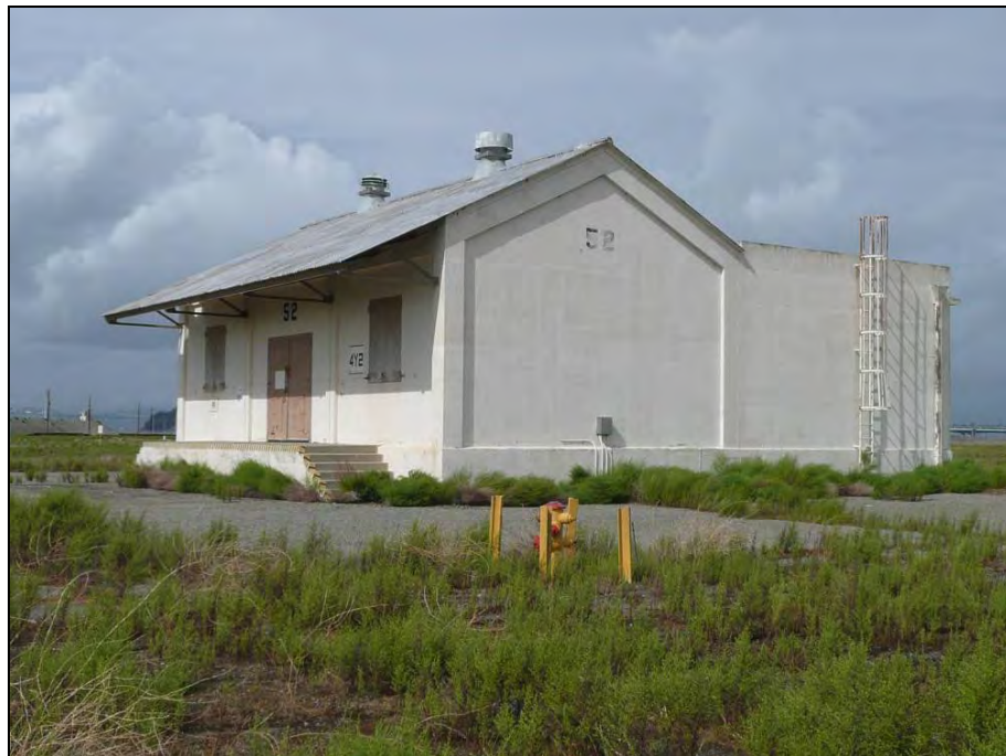
Photograph 3: Building 52, camera facing west, October 13, 2009.
