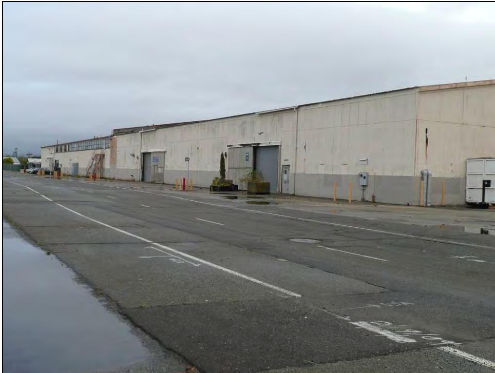
Photograph 4: Building 170, west side, camera facing northeast, October 14, 2009.
