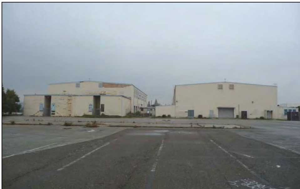
Photograph 1: Building 76 on left, Building 134 on right, camera facing east, December 11, 2009.
