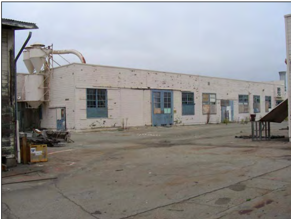
Photograph 9: South extension on North Wing, camera facing northeast, October 8, 2009.
