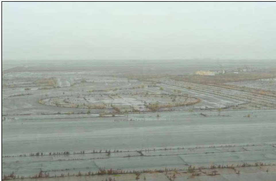
Photograph 21: Compass Rose (Building 489), camera facing west, December 16, 2009.
