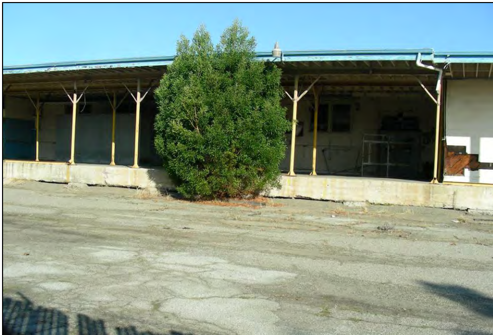
Photograph 5: South side bay, camera facing north, November 12, 2009.
