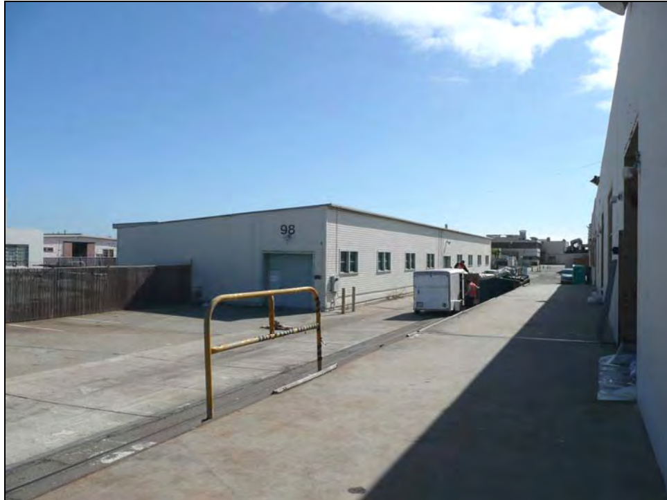
Photograph 1: Camera facing southeast, October 15, 2009.
