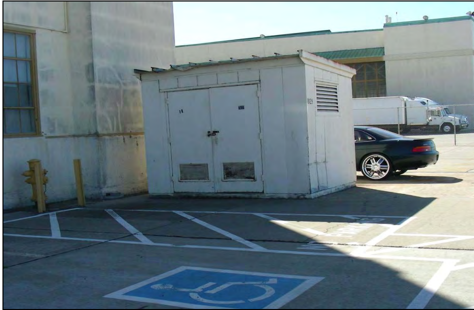
Photograph 3: Building 315, camera facing southeast, September 30, 2009.
