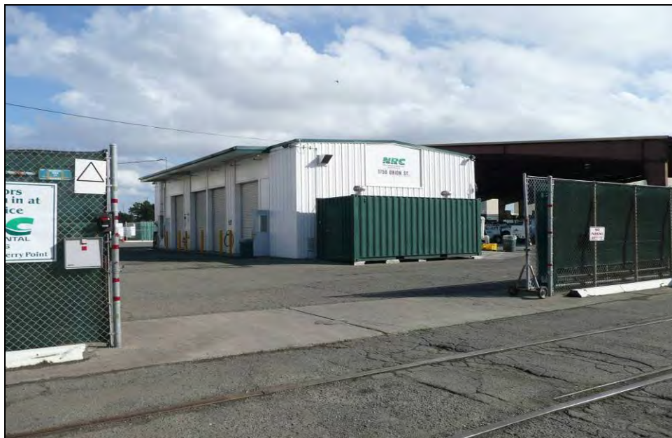
Photograph 3: Building 616, camera facing southeast, October 14, 2009.
