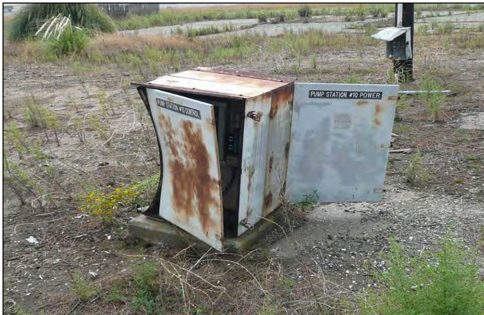
Photograph 7: Building 468, facing east, October 13, 2009.
