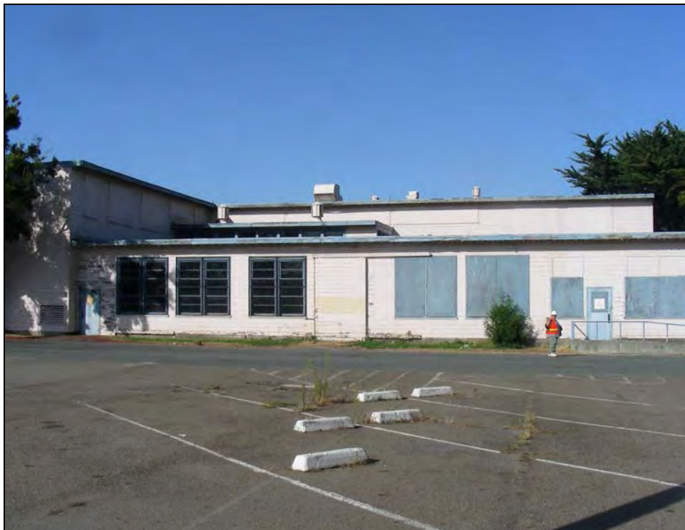
Photograph 2: Building 137, east side with clerestory, camera facing west, October 6, 2009.
