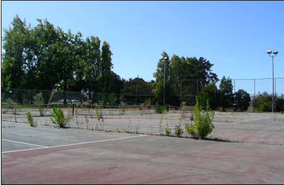
Photograph 2: Building 423, Tennis Courts, facing northwest, September 29, 2009.
