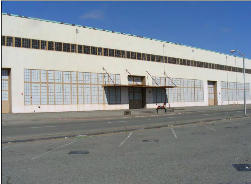
Photograph 3: Suspended roof on south side, camera facing northeast, October 8, 2009.
