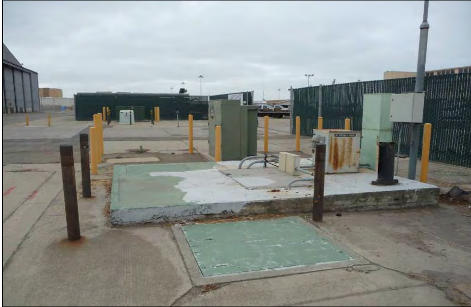
Photograph 2: Building 287, camera facing south, October 8, 2009.
