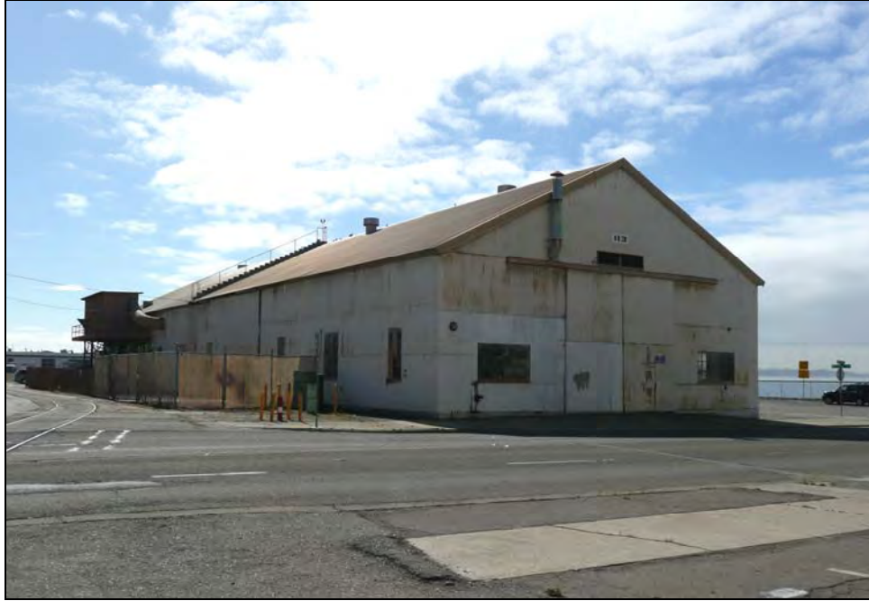
Photograph 1: Camera facing southwest, October 15, 2009.
