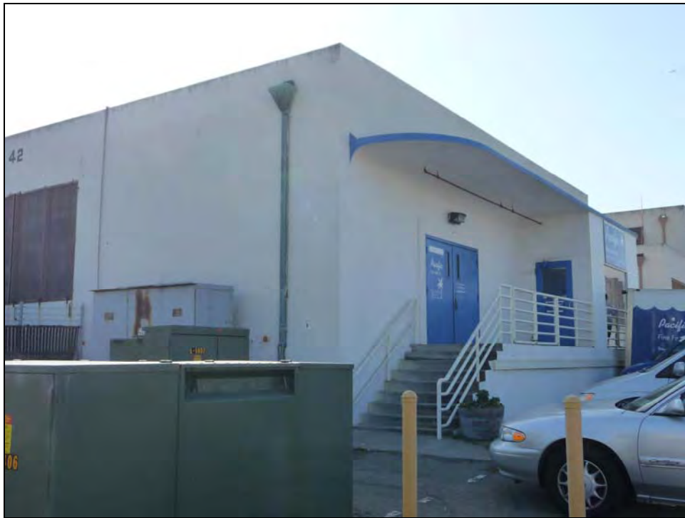
Photograph 3: Northwest corner, camera facing southeast, October 6, 2009.
