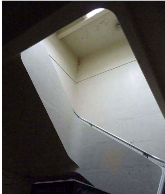
Photograph 11: Curved stairwell with metal handrail, interior Building 3, camera facing southwest, December 11, 2009.
