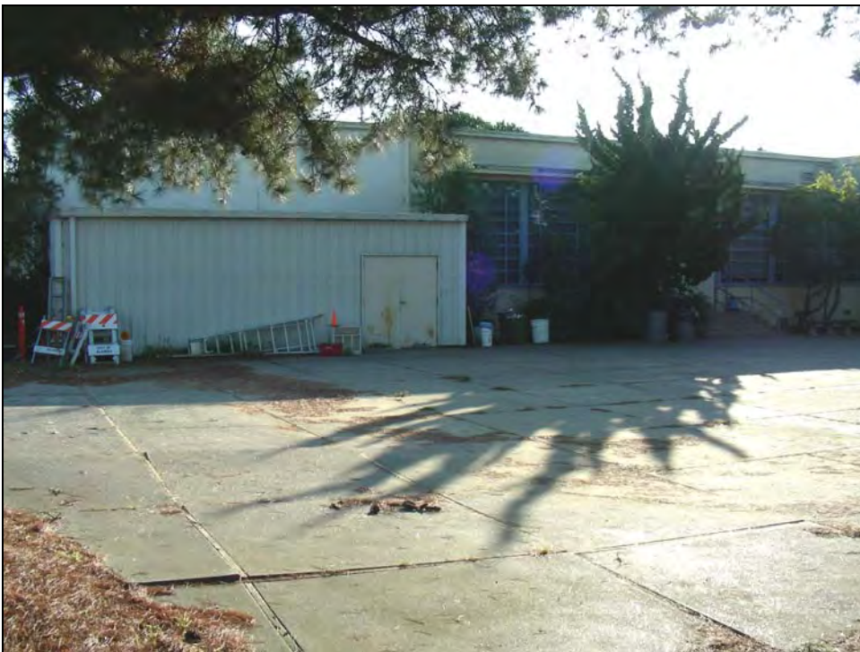
Photograph 5: North side of 'L' shaped wing, camera facing south, November 12, 2009.
