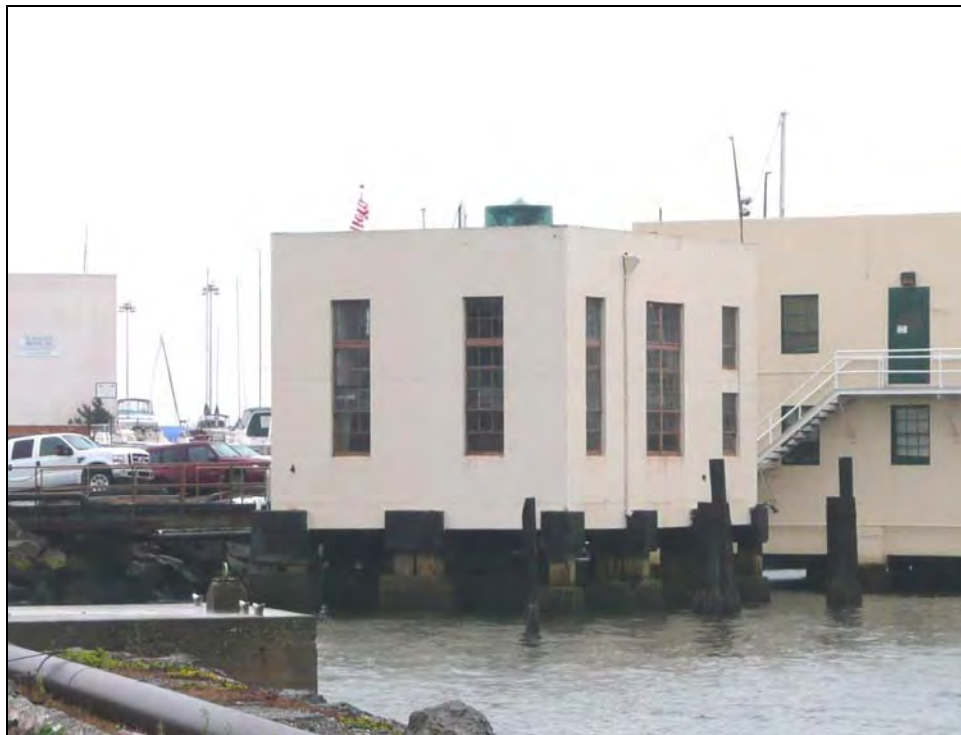
Photograph 2: Camera facing southwest, October 13, 2009
