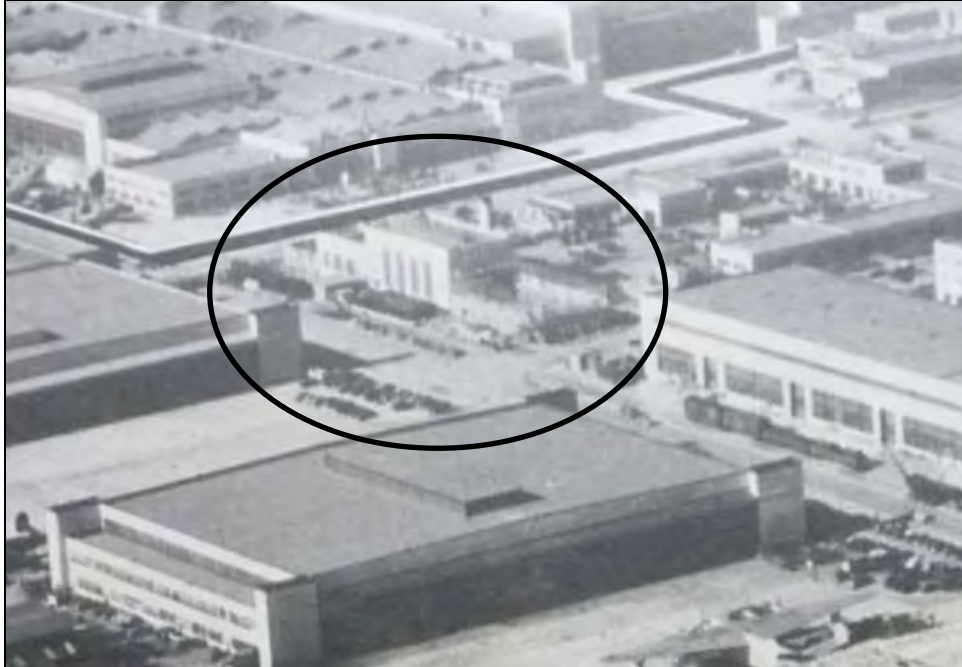
Photograph 5: East and west additions to Building 10 under construction, January 1, 1945, camera facing northwest.
