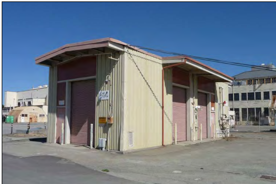
Photograph 59: Hazardous Material Storage (Building 614), October 1, 2009.
