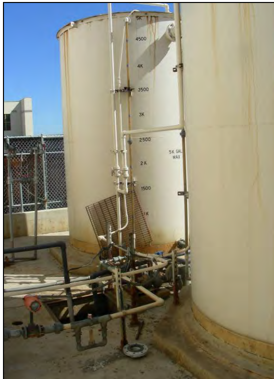
Photograph 3: Tank area detail, camera facing northeast, September 30, 2009.
