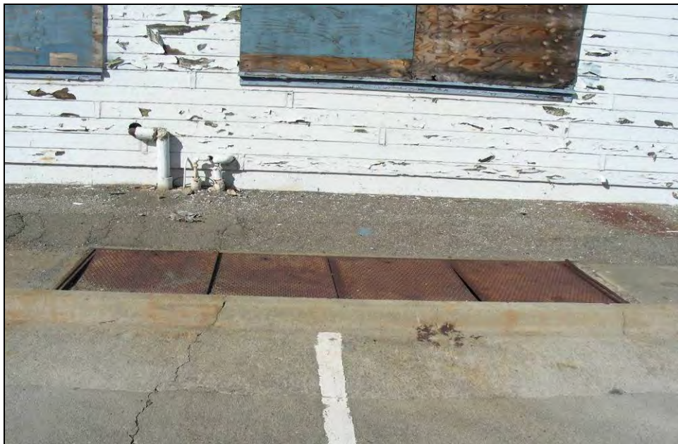
Photograph 9: Building 469 section 2 northwest of section 1, facing north, October 7, 2009.
