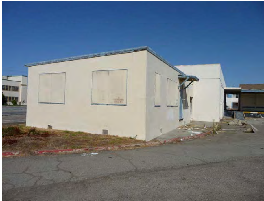
Photograph 2: Camera facing southwest, October 6, 2009.
