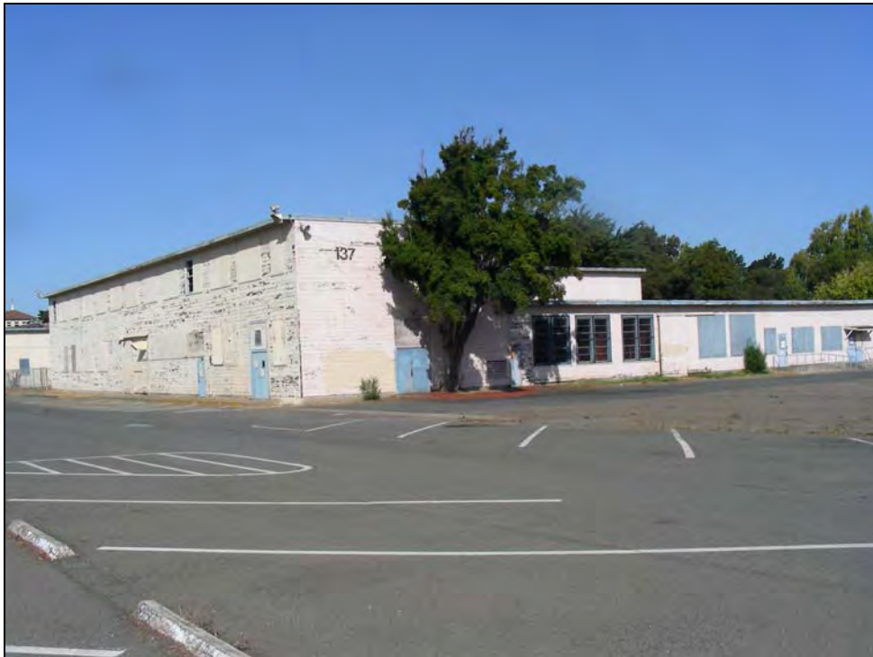
Photograph 1: Building 137, facing northwest, October 6, 2009.
