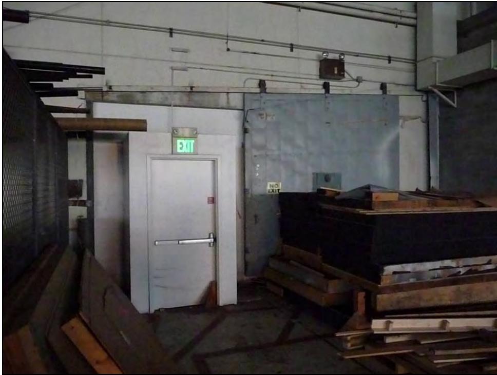
Photograph 9: Interior of Building 12, showing access to Building 400, camera facing west, December 11, 2009.
