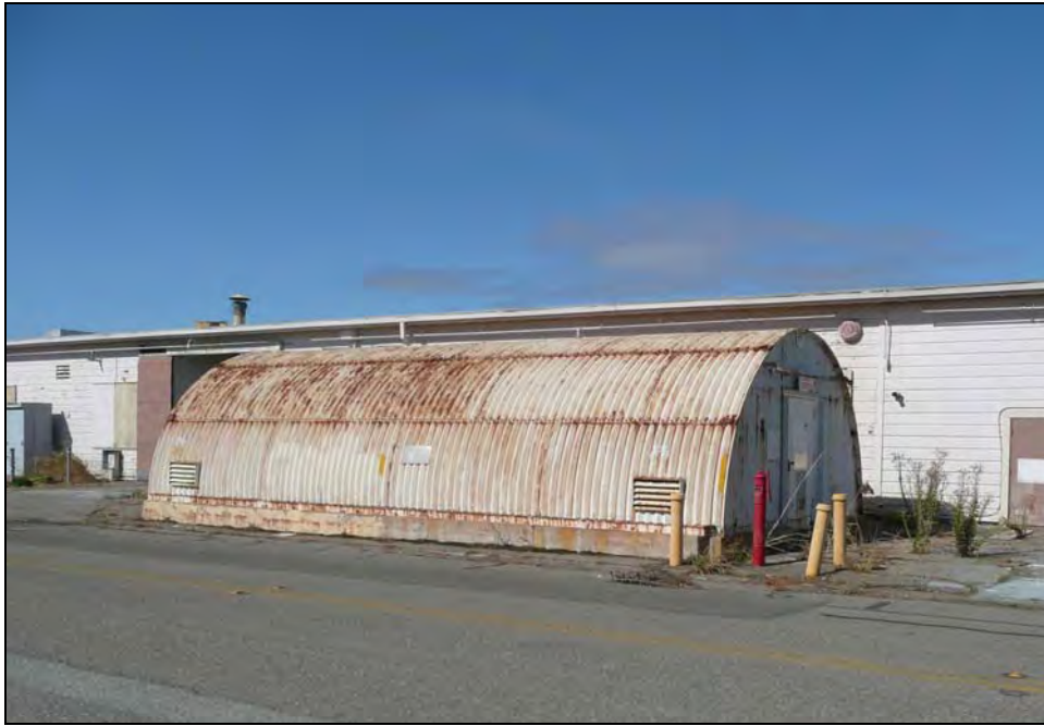
Photograph 6: Building 337, camera facing northwest, October 15, 2009.
