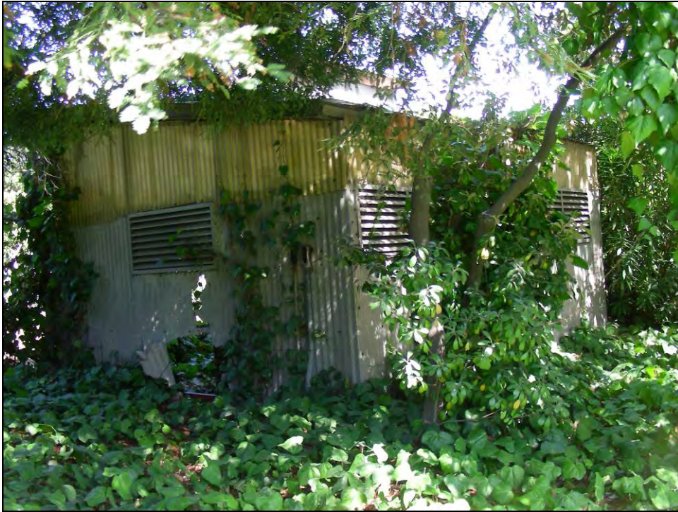
Photograph 2: Building 419, camera facing northeast, September 29, 2009.
