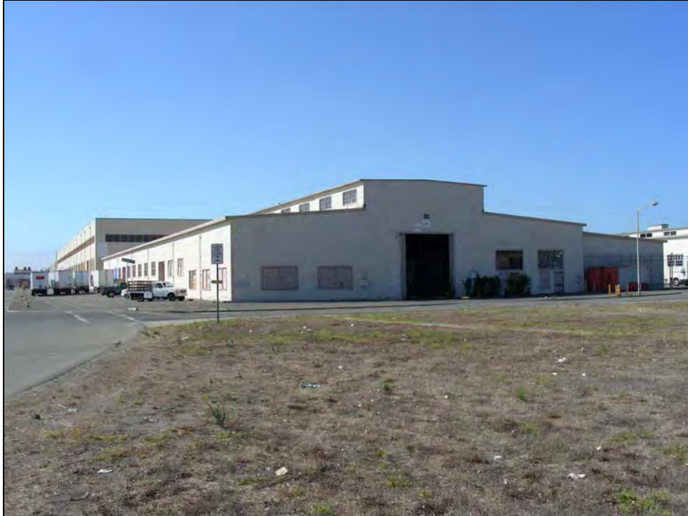
Photograph 1: East façade, camera facing northwest, October 8, 2009.
