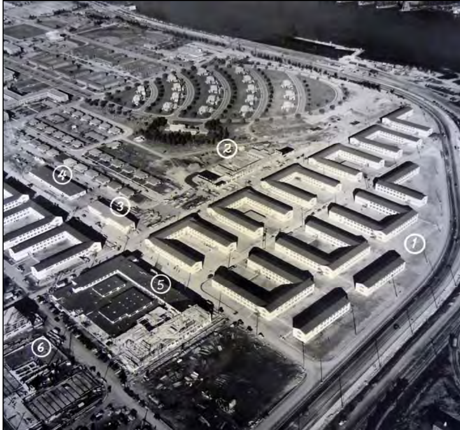
Photograph 25: Construction of temporary style barrack on east end of NAS Alameda, 1944. Numbers indicated specific projects on original photograph. 105
