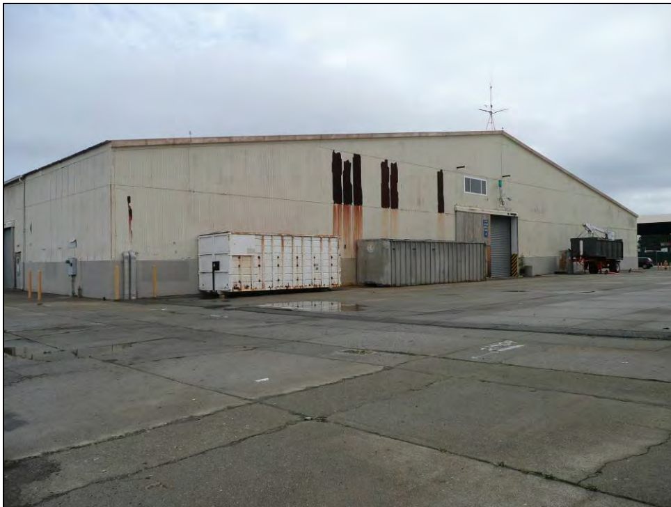
Photograph 3: Building 170, south side, camera facing northeast, October 14, 2009.
