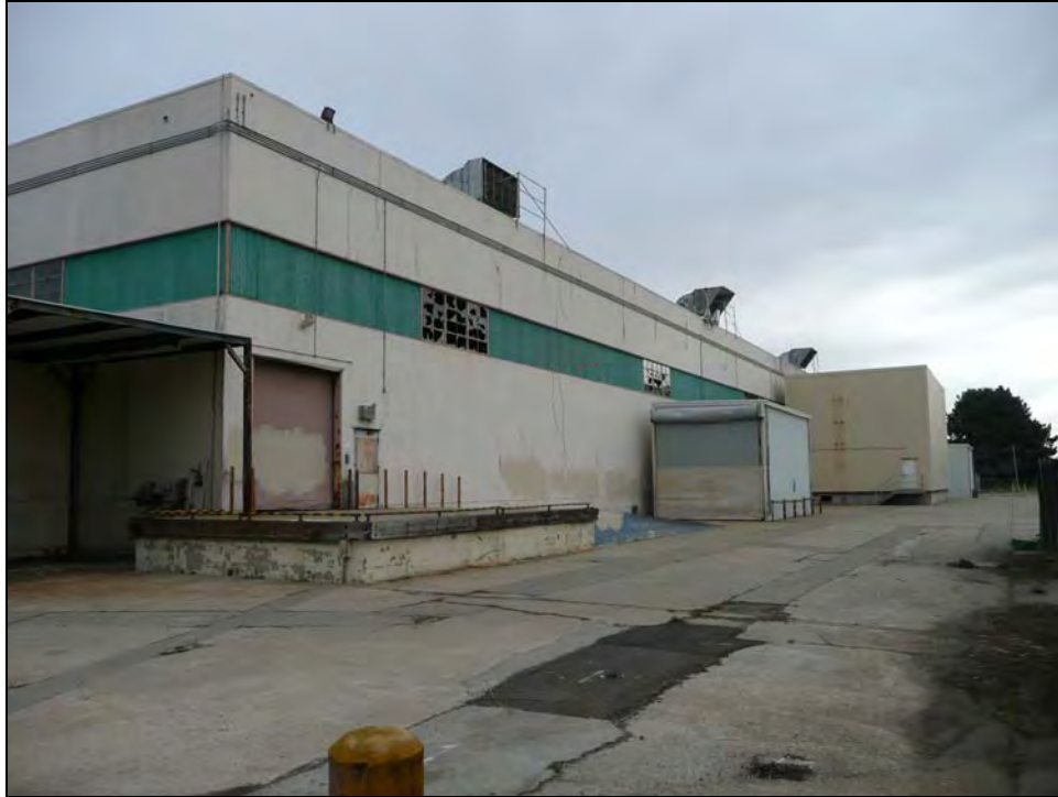
Photograph 2: South side, camera facing north, December 16, 2009.
