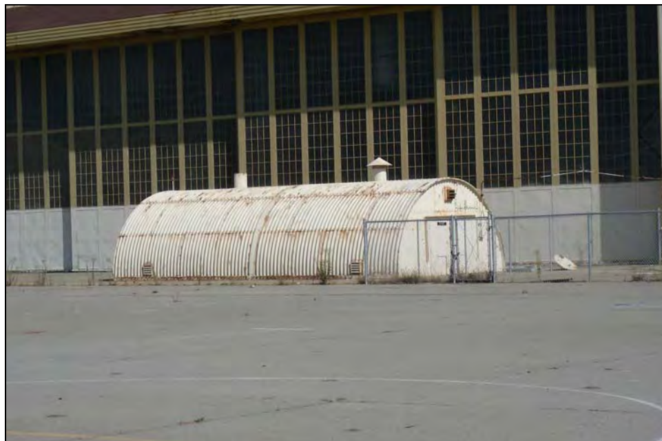
Photograph 5: Building 273, camera facing northeast, October 8, 2009
