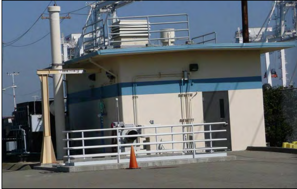
Photograph 6: Eastern component of Building 562, camera facing north, September 25, 2009.
