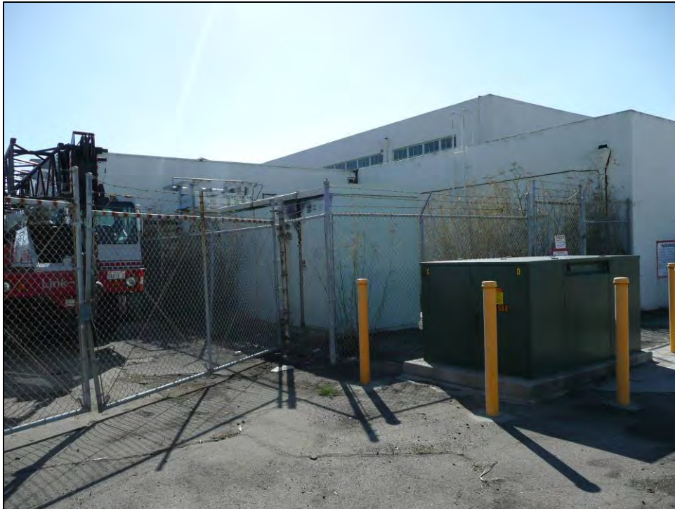
Photograph 2: Building 412, camera facing southwest, October 15, 2009.
