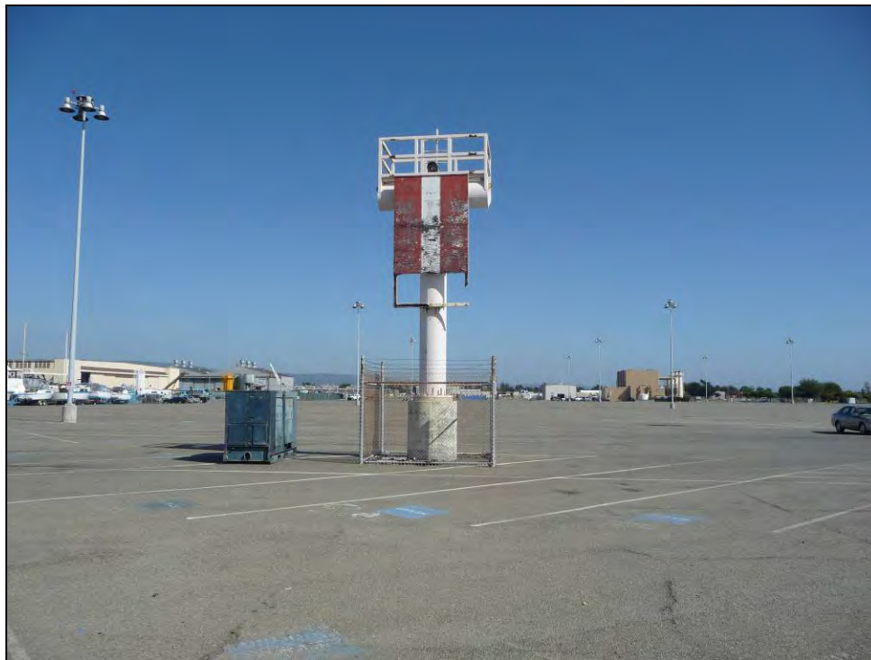
Photograph 2: Building 302W, camera facing east, October 8, 2009.
