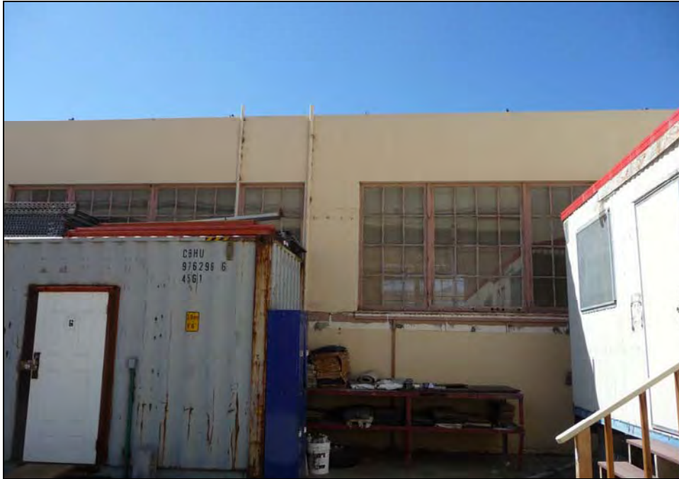
Photograph 3: North end of east side, camera facing west, October 1, 2009.
