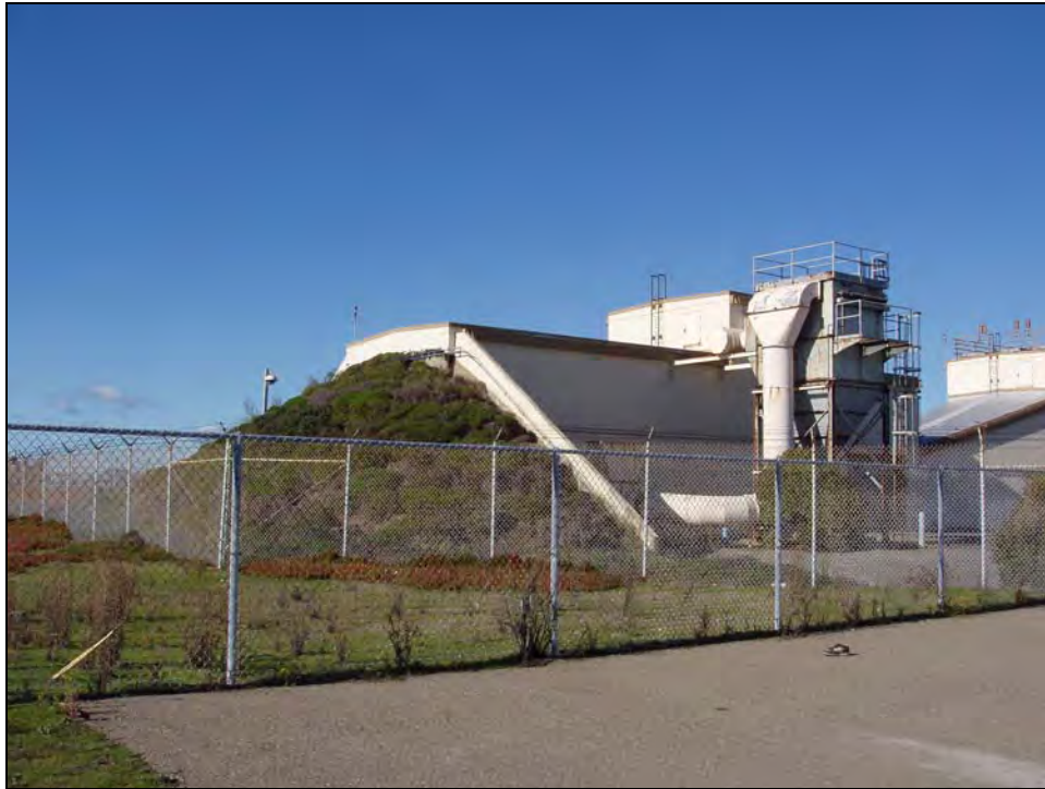
Photograph 8: Earth mound at south end of Building, photo from PGA, camera facing northwest, December 22, 2009.
