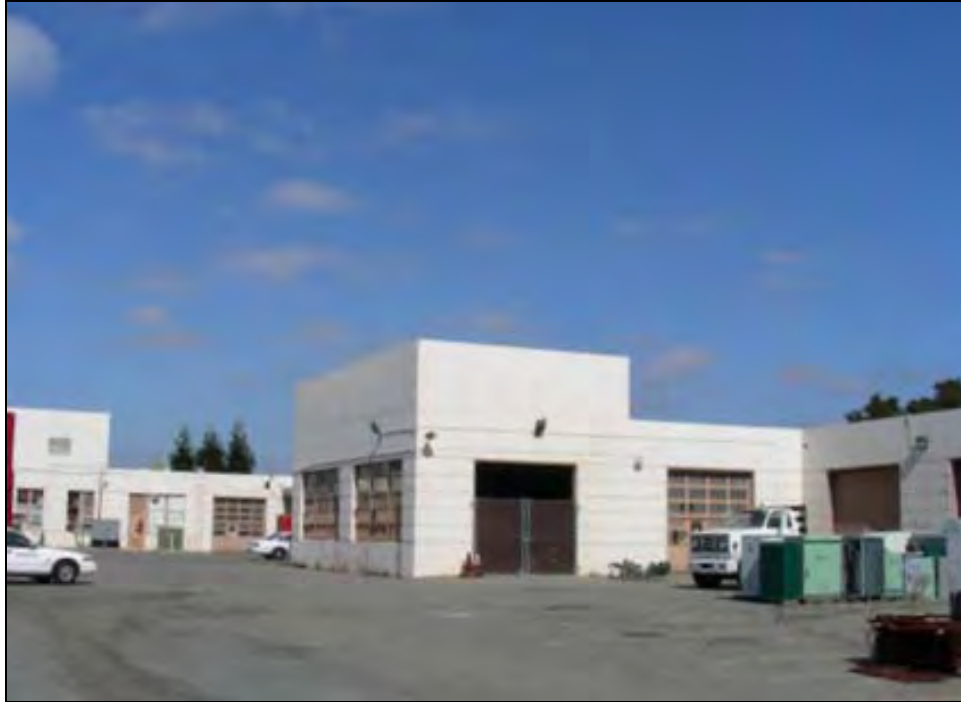
Photograph 6: Southeast side, camera facing northeast, October 8, 2009.
