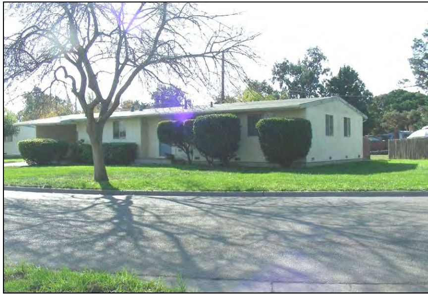
Photograph 35: Single family officers' housing, Building 770, November 4, 2009.
