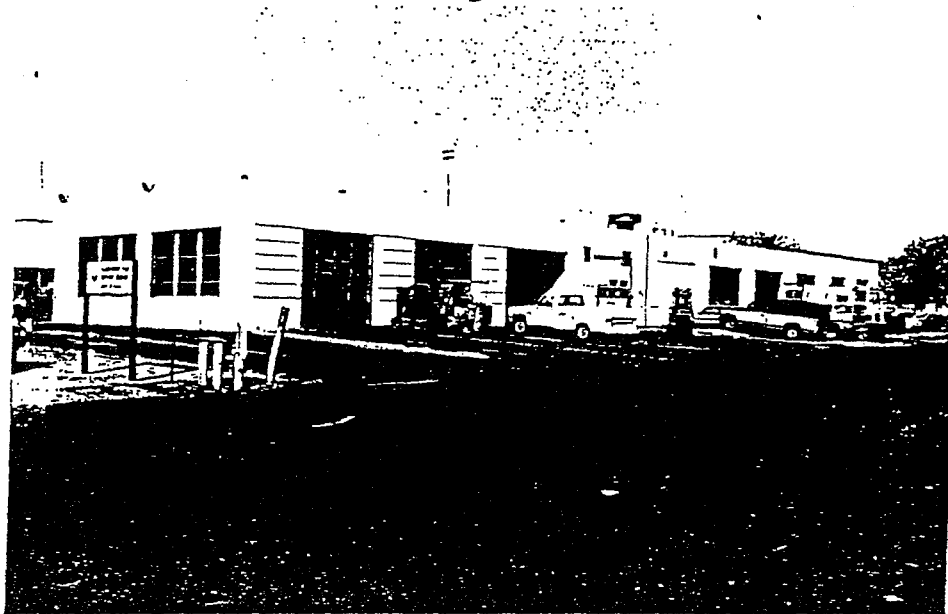
NAS ALAMEDA Building 6
