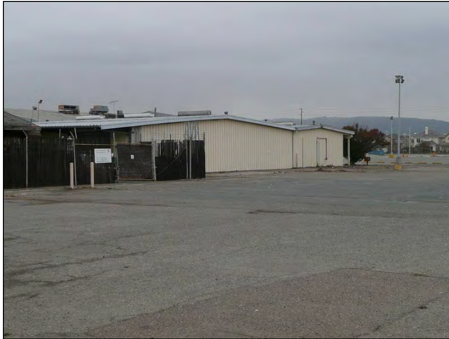
Photograph 3: Camera facing northeast, October 15, 2009.
