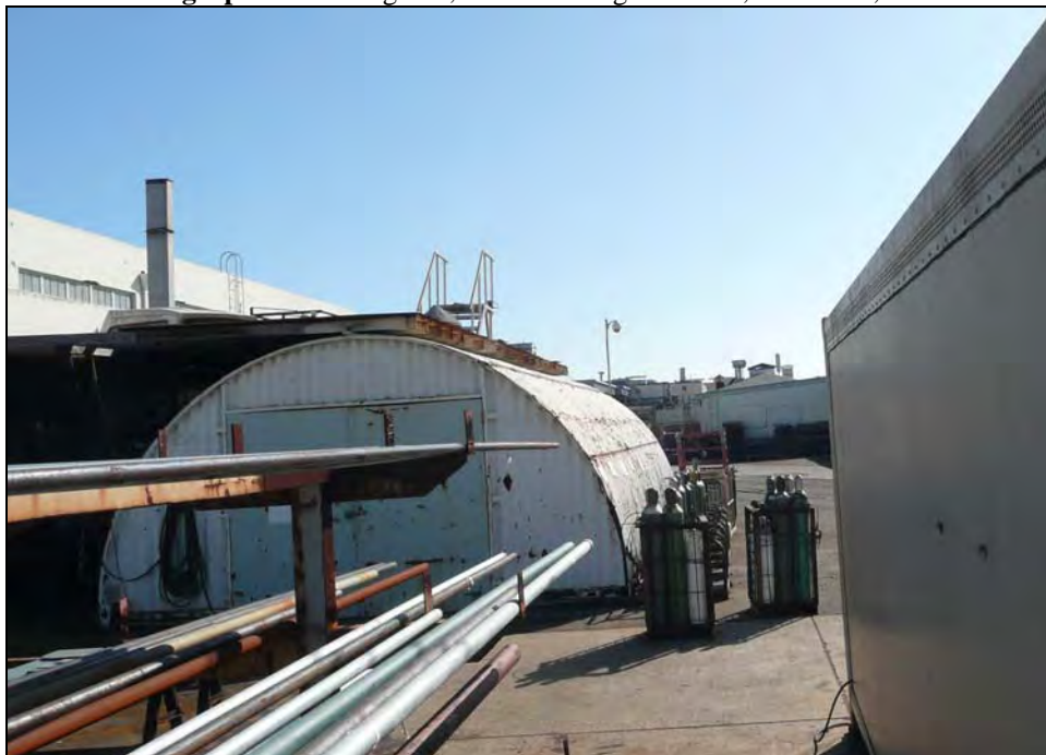
Photograph 3: Building 263, camera facing south, October 15, 2009.
