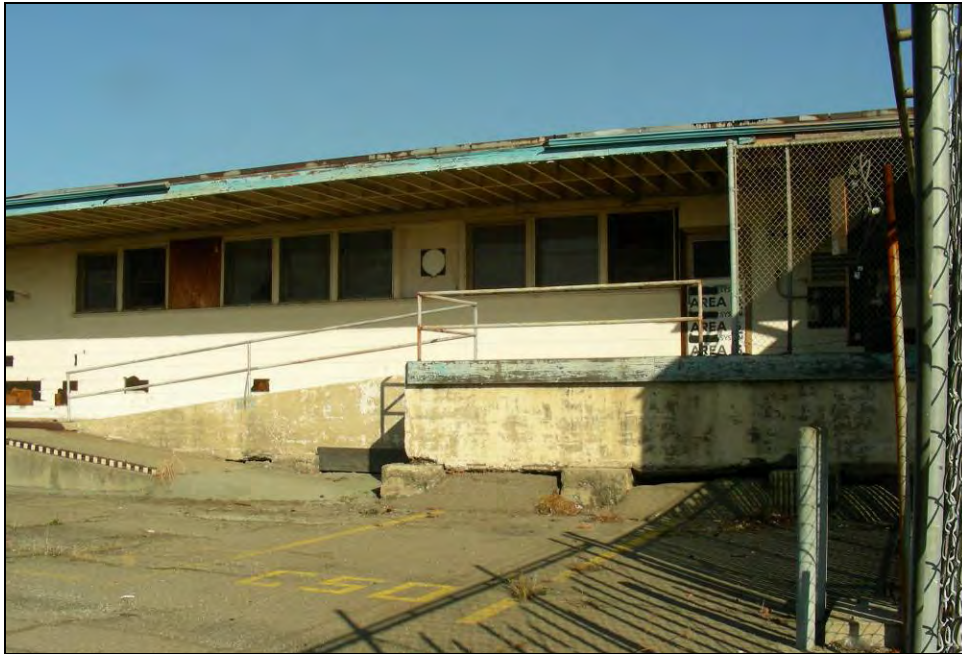
Photograph 4: East end of south side bay, camera facing north, November 12, 2009.
