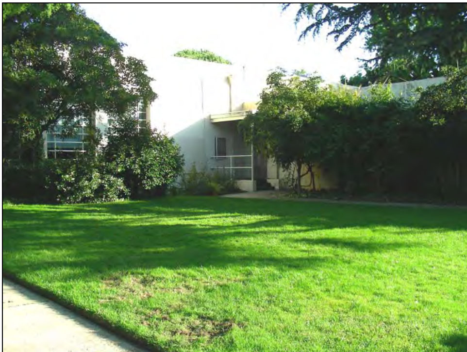
Photograph 11: Southeast corner of inner courtyard area, camera facing southeast, November 12, 2009.
