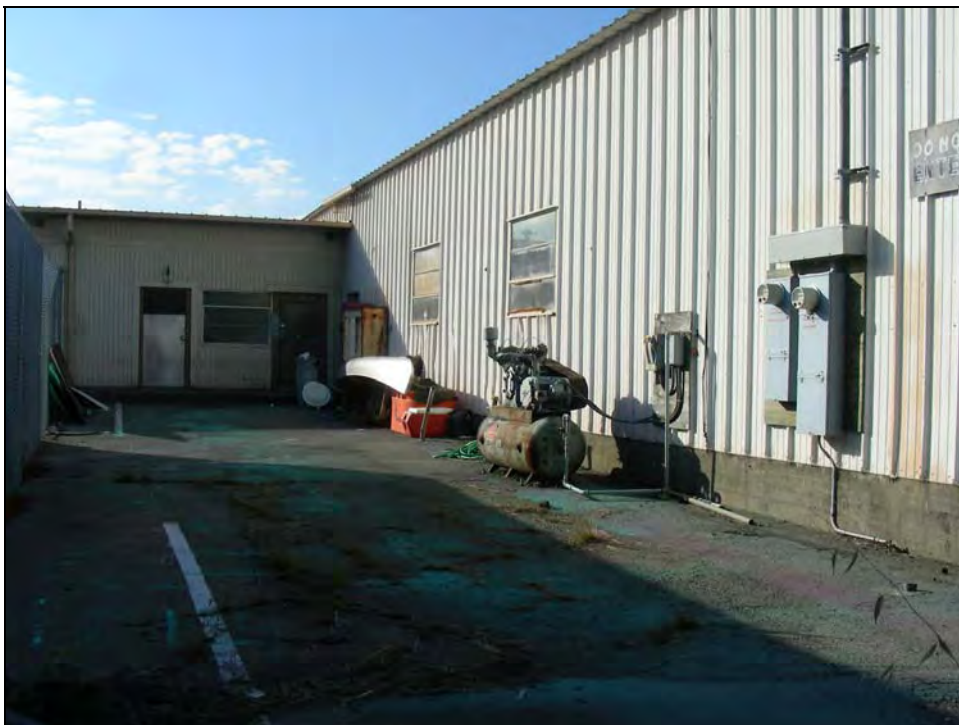
Photograph 3: Northeast corner of north-south wing, camera facing south, November 12, 2009.
