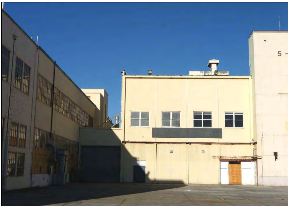
Photograph 6: Detail view east end of the Mezzanine, former main entrance was at the lower right, camera facing west, October 1, 2009.
