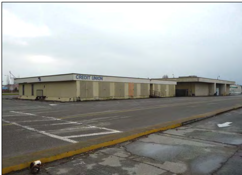
Photograph 2: Building 527, camera facing southeast, December 11, 2009.
