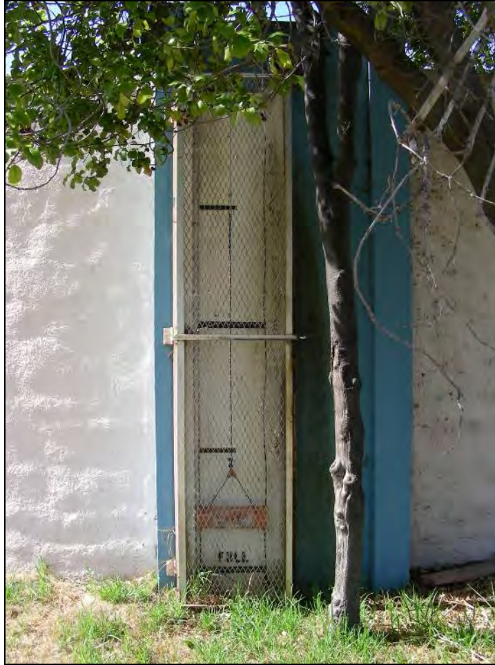
Photograph 2: Building 95, detail of gauge, camera facing west, September 29, 2009.
