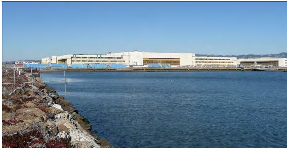
Photograph 52: Maintenance Hangars and Avionics Building (Building 11, 12, and 400), October 1, 2009.
