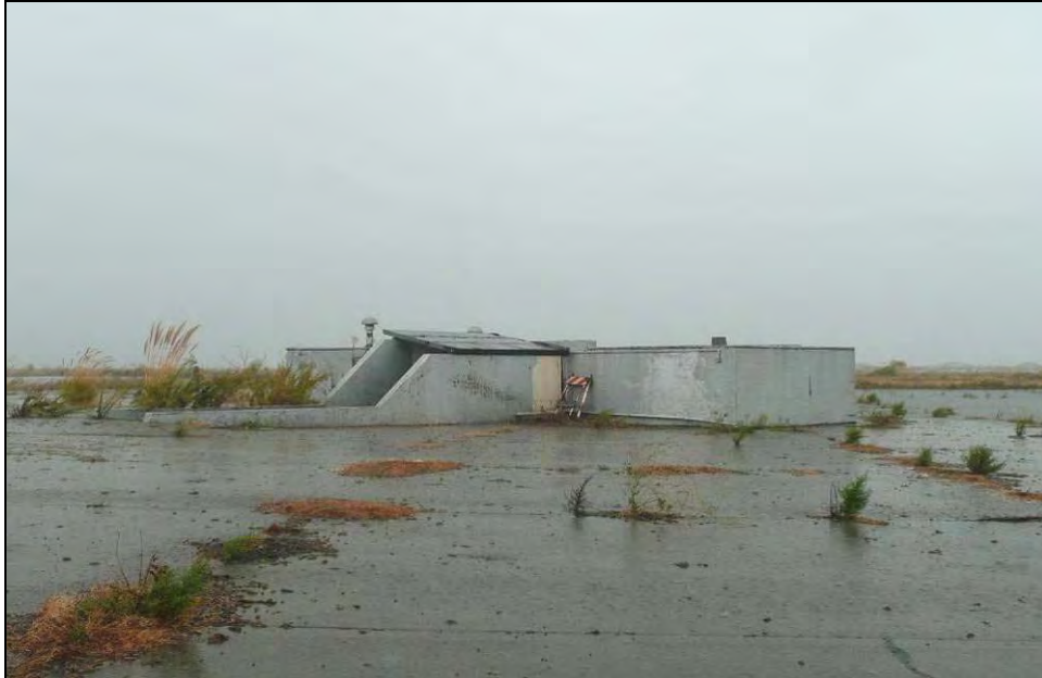
Photograph 28: Transformer Vault (Building 100), camera facing east, October 13, 2009
