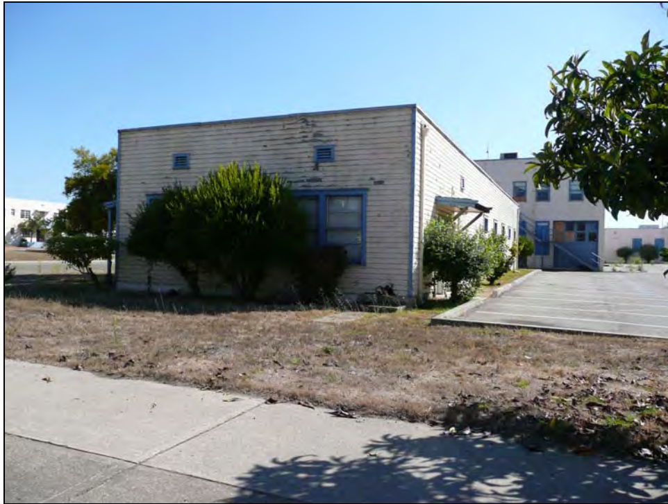
Photograph 3: North side, camera facing southeast, September 25, 2009.
