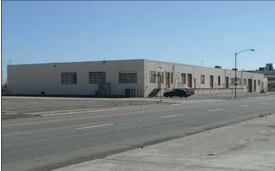
Photograph 1: Camera facing southeast, showing south end of building, October 15, 2009.
