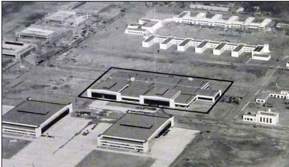
Photograph 15: Building 5 original construction before construction of the Southwest Extension began, January 1, 1941. (Black outline is on original photograph.) 13
