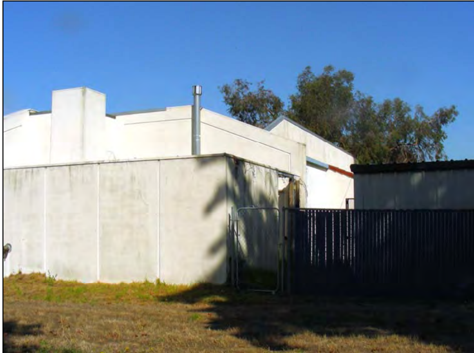
Photograph 2: Building 585 southeast corner, facing north, October 6, 2009.
