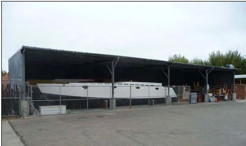
Photograph 5: Building 608 B, camera facing southwest, October 8, 2009.
