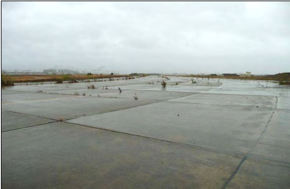
Photograph 15: Taxiway B / Taxiway 50 (Building 201256), camera facing southwest, October 13, 2009.
