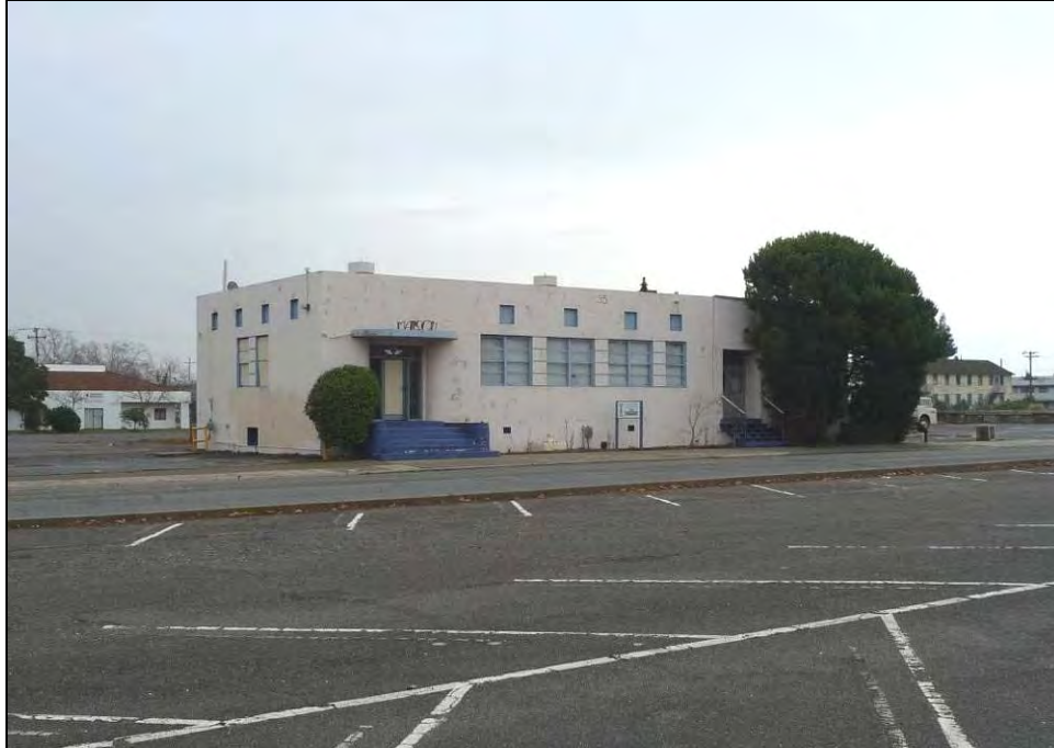
Photograph 1: Camera facing southeast, December 16, 2009.
