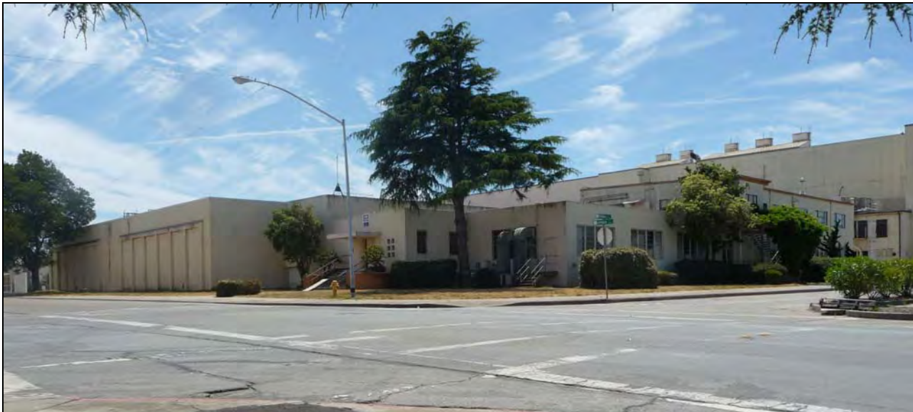
Photograph 1: Northeast corner, camera facing southwest, June 9, 2010.
