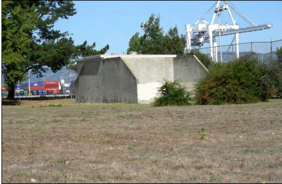
Photograph 4: Building 382, Squash Courts, facing northeast, September 29, 2009.
