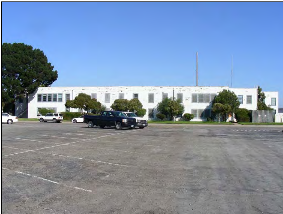
Photograph 5: West Wing, camera facing east, October 7, 2009.
