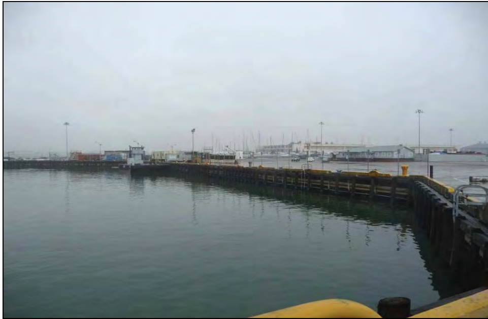
Photograph 13: Wharf 2, camera facing north, December 16, 2009.
