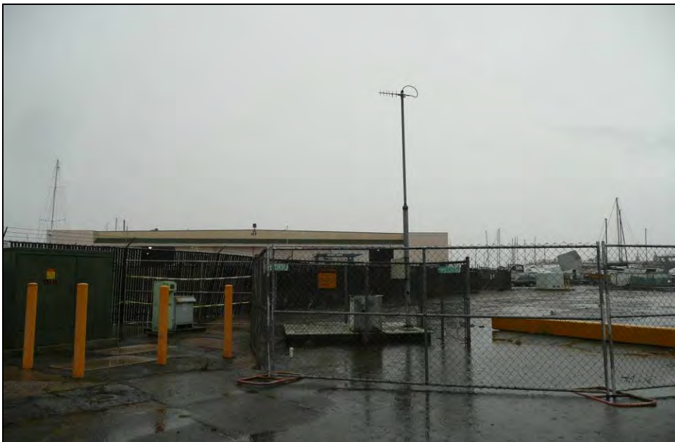
Photograph 3: Building 449, camera facing southeast, October 13, 2009.
