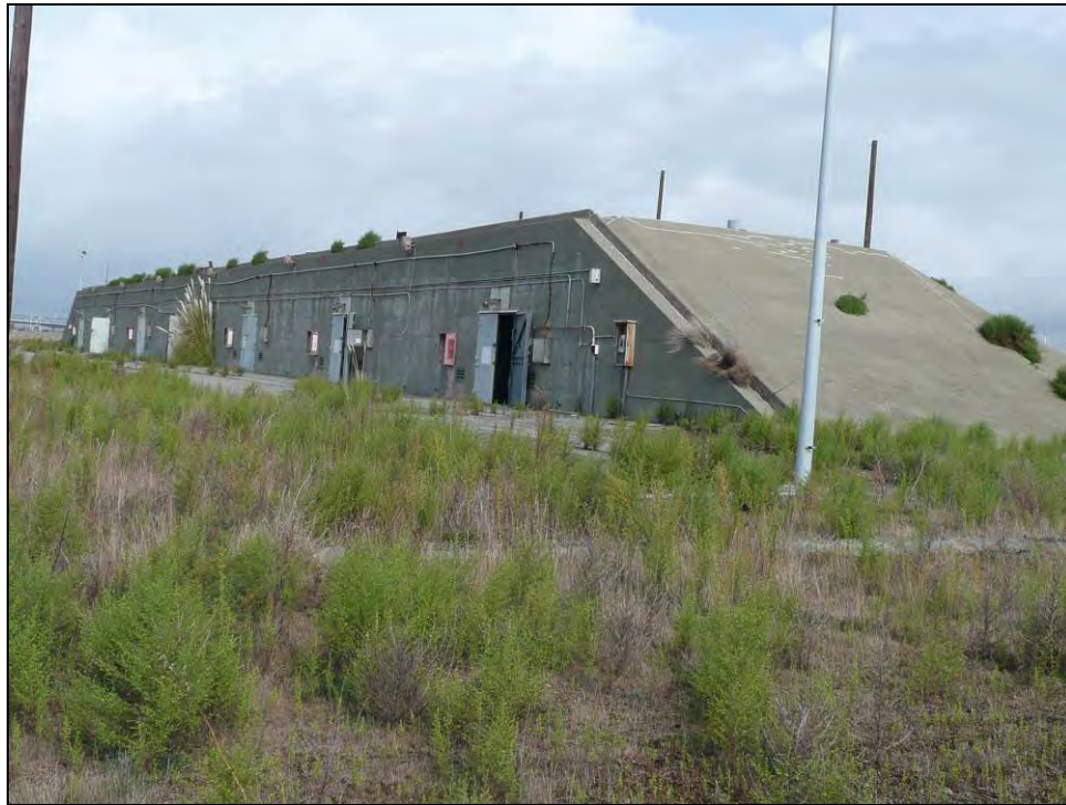
Photograph 8: Building 497, camera facing northeast, October 14, 2009.
