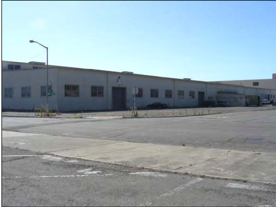
Photograph 3: North side, camera facing southwest, October 8, 2009.
