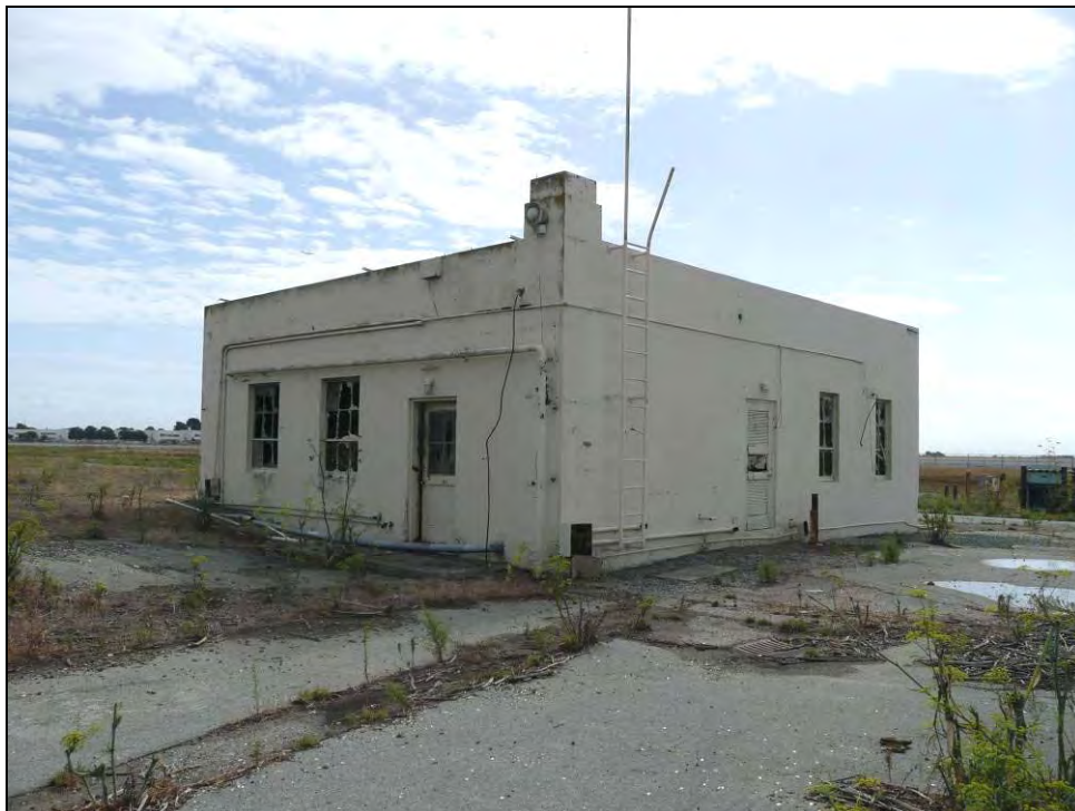
Photograph 2: Camera facing southeast, October 14, 2009.
