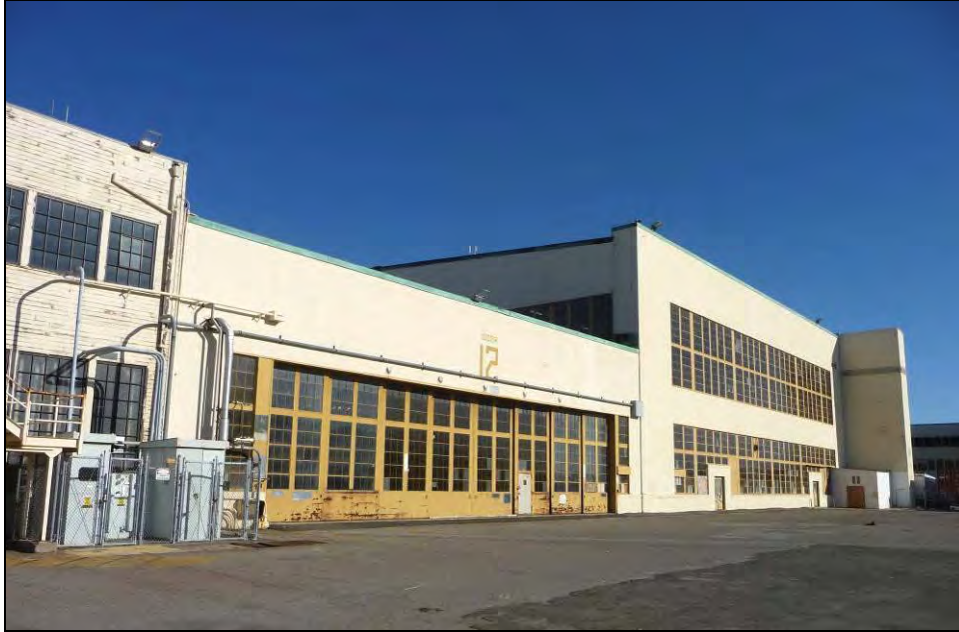
Photograph 9: Door 12 and west side of Door 11, camera facing southeast, September 29, 2009.
