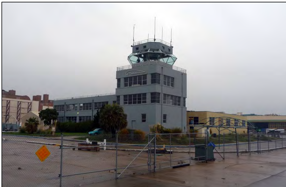
Photograph 2: Building 19, camera facing northeast, December 16, 2009.
