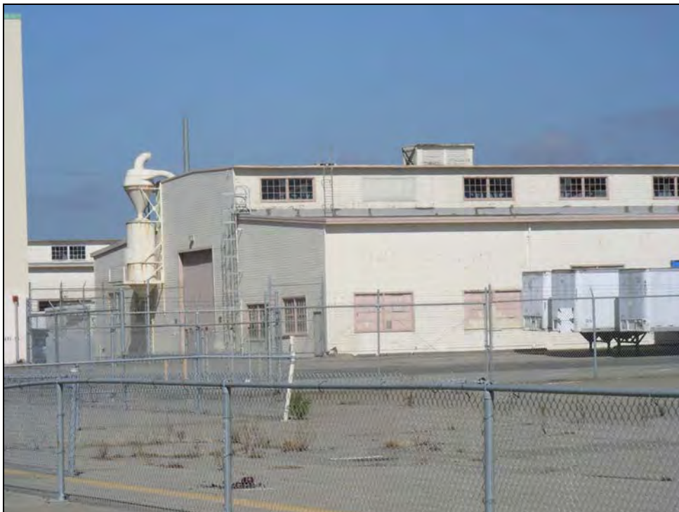
Photograph 2: Southwest corner, camera facing northeast, October 8, 2009.
