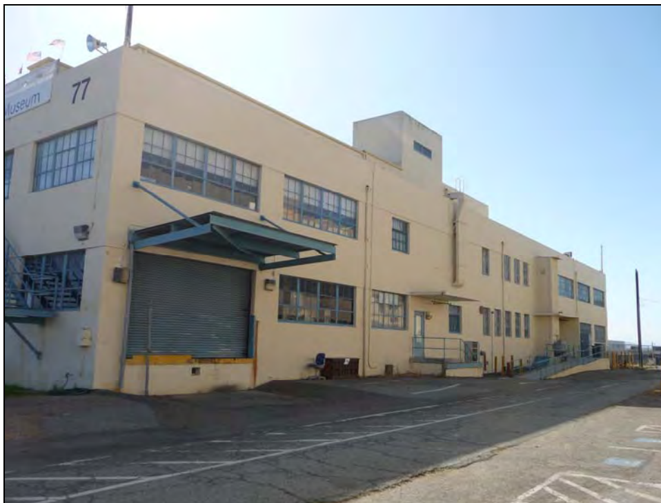
Photograph 5: North wall, camera facing southwest, October 8, 2009.
