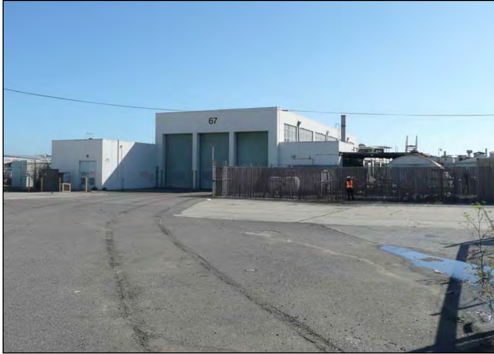
Photograph 3: Camera facing southeast, October 15, 2009.
