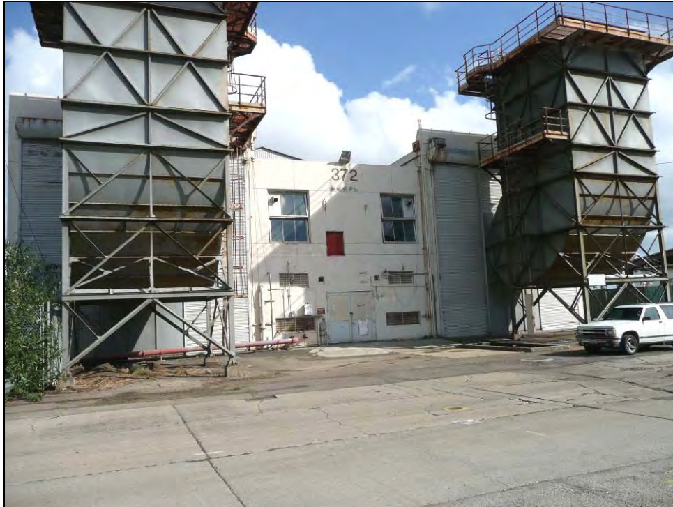
Photograph 3: West side, camera facing southeast, October 14, 2009.
