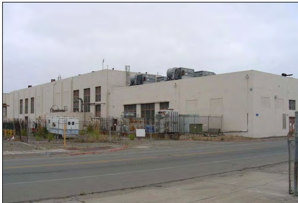
Photograph 2: Building 34 at northwest corner camera facing southeast, October 8, 2009.
