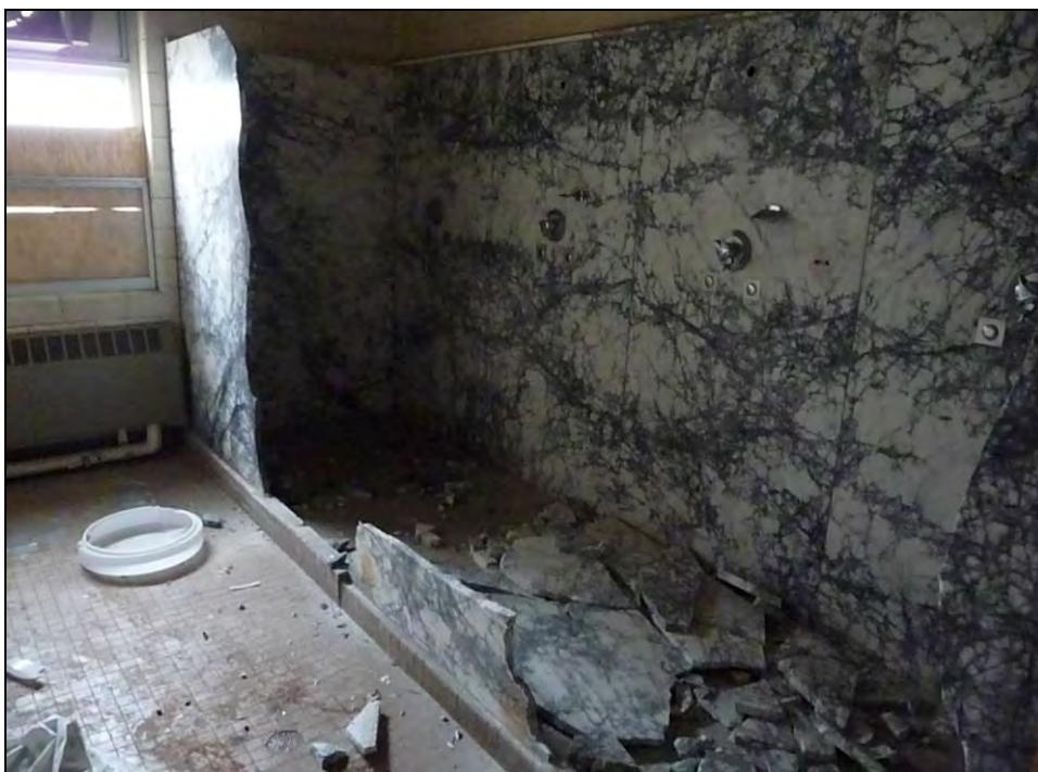
Photograph 15: Showing partially demolished marble shower stalls, Building 2, camera facing east, December 11, 2009.
