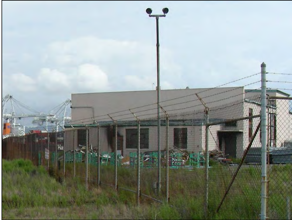
Photograph 2: Building 420, camera facing northeast, October 14, 2009.
