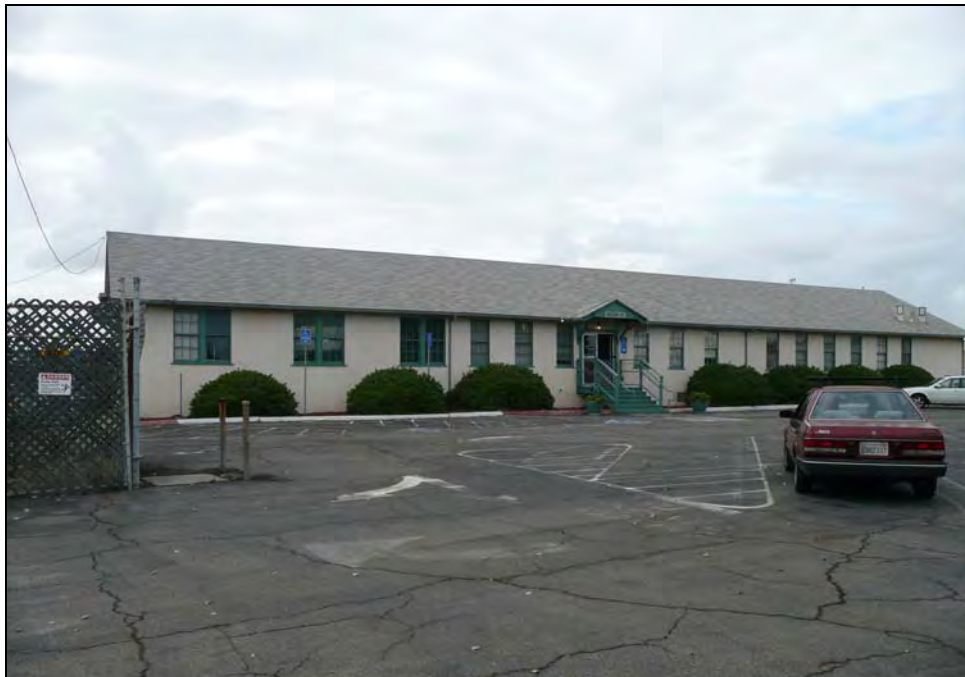
Photograph 2: Main entrance on east façade, camera facing northwest, October 14, 2009.
