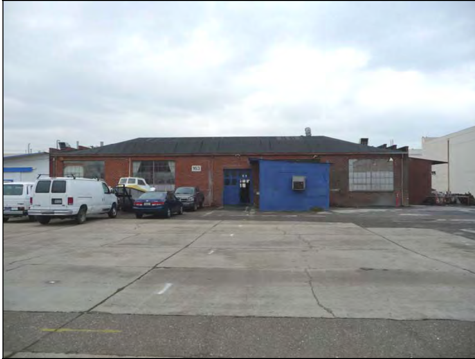
Photograph 3: West side, camera facing east, October 14, 2009.
