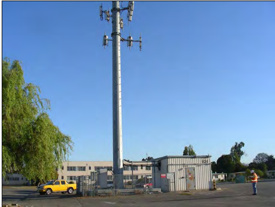
Photograph 2: Camera facing northeast, October 7, 2009.
