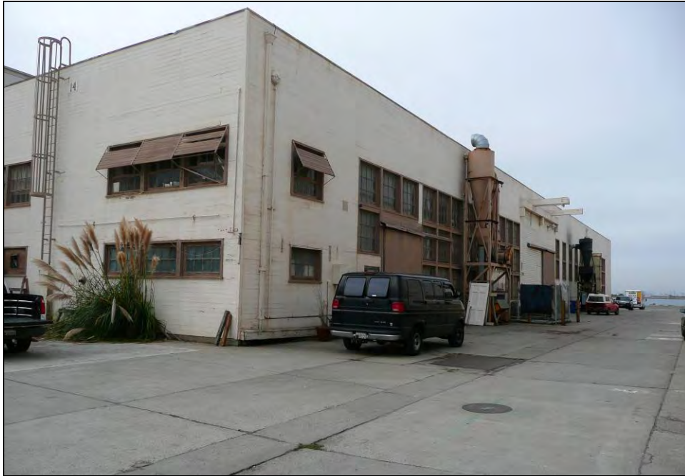
Photograph 2: Preservation shop section along north side, camera facing southwest, October 15, 2009.
