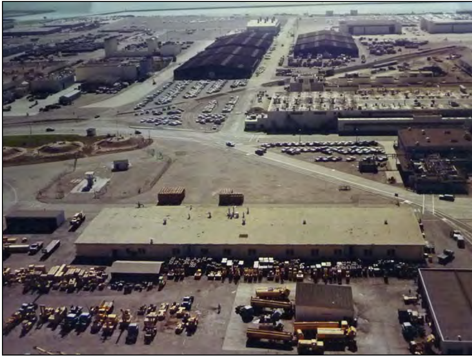
Photograph 3: 1960s Oblique aerial photograph of Building 112 facing south. 1
