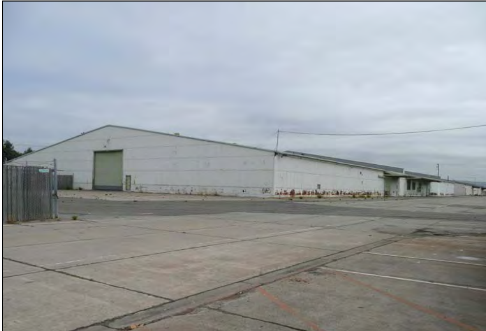
Photograph 1: Camera facing northeast, October 15, 2009.
