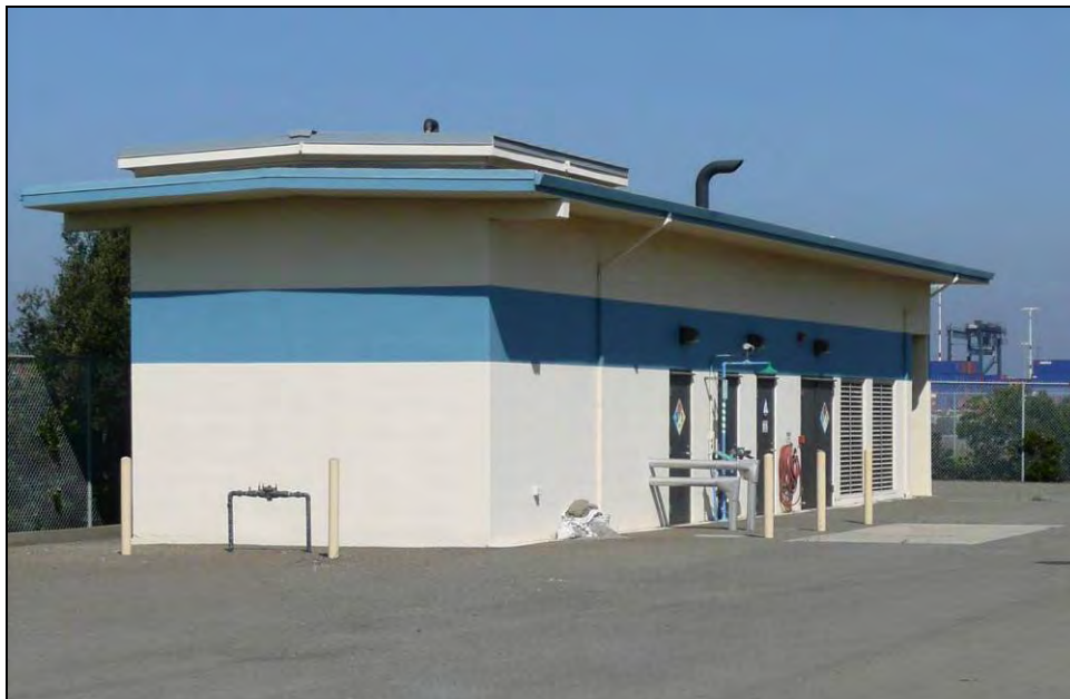
Photograph 5: Western component of Building 562, camera facing north, September 25, 2009.
