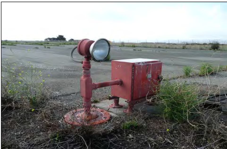
Photograph 5: Elevated high intensity runway light / beacon, northwest end of Runway 13-31, camera facing southwest, October 13, 2009.
