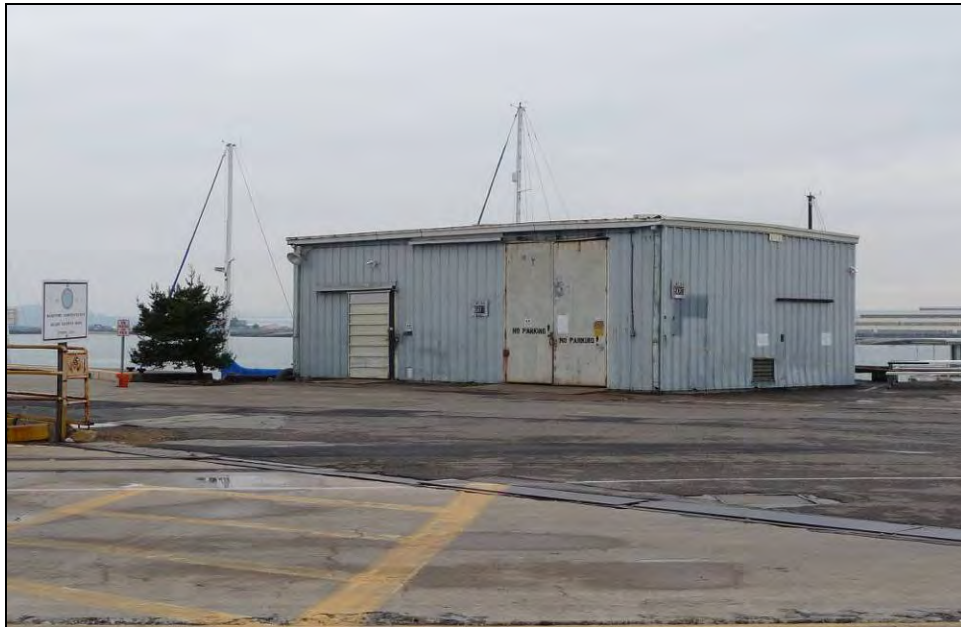
Photograph 4: Building 601 at east end of Pier 1, camera facing northwest, December 11, 2009.
