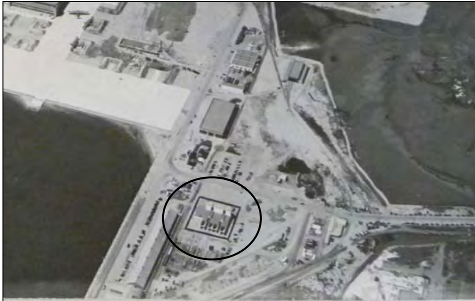
Photograph 4: Building 14 aerial view, first phase of construction, June 1942.
