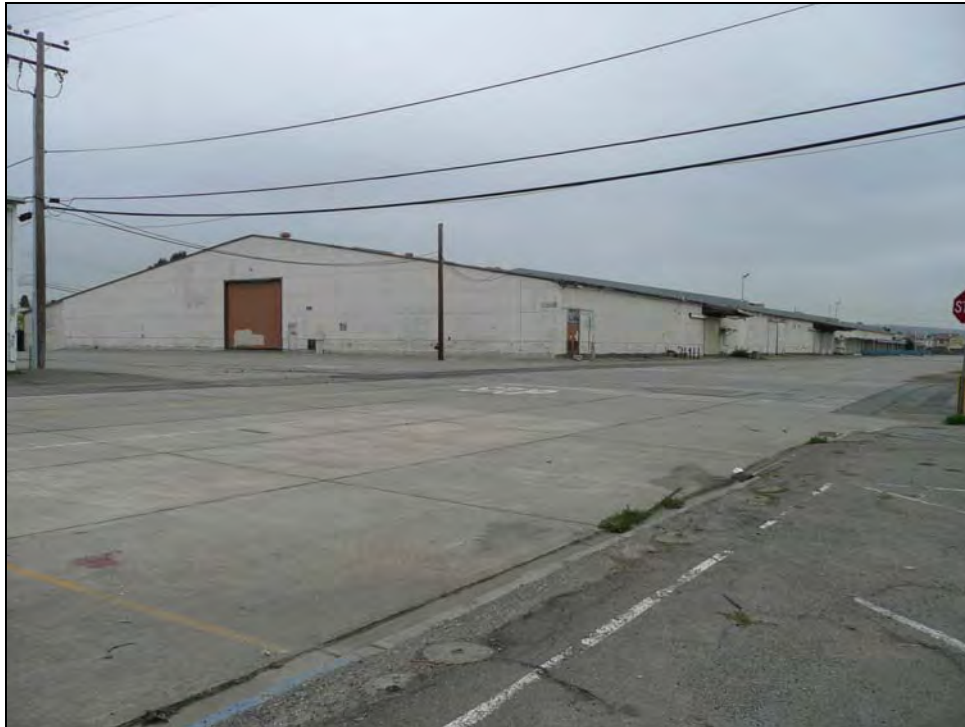
Photograph 1: Camera facing northwest, showing west side, October 15, 2009.
