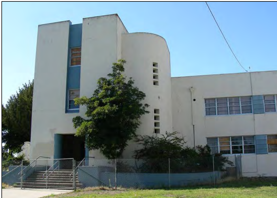
Photograph 7: Tower on southeast corner of Wing 20 Building 4, camera facing southwest, October 7, 2009.
