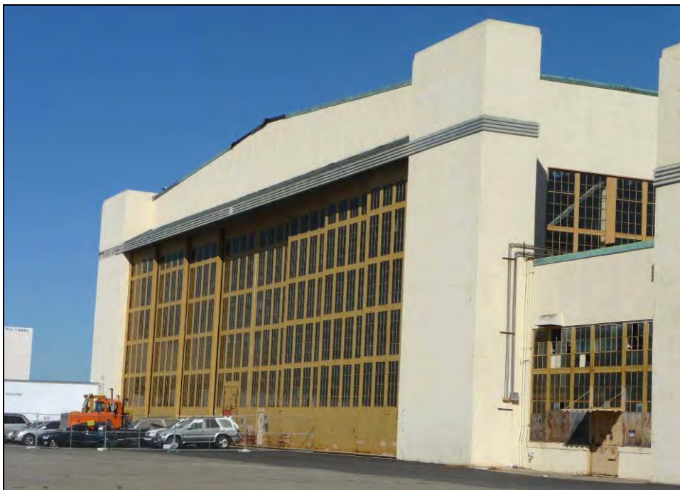
Photograph 8: Door 11 and adjoining shop area at southwest corner of Building 5, camera facing northwest, October 1, 2009.
