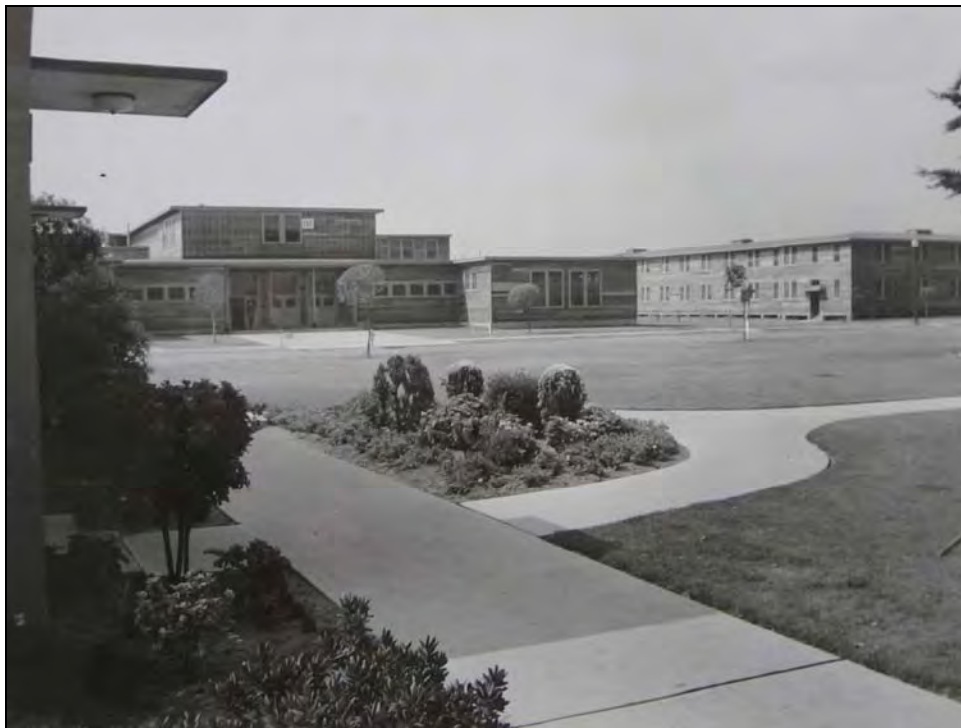
Photograph 6: May 1945 photo of main entrance on north side of Building 137. 1
