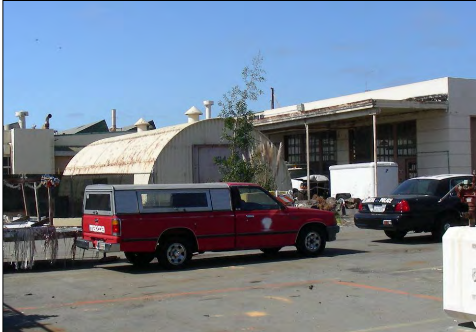
Photograph 2: Building 194, camera facing northeast, October 8, 2009.
