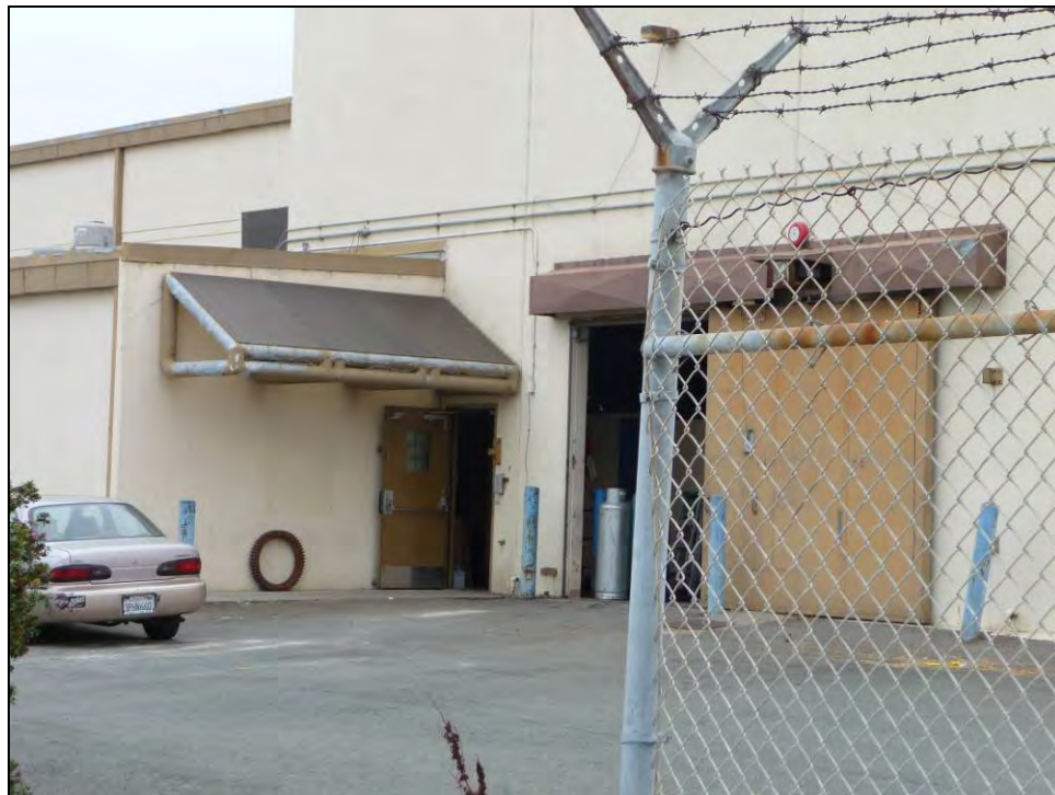
Photograph 3: Door detail north side, camera facing southwest, October 8, 2009.
