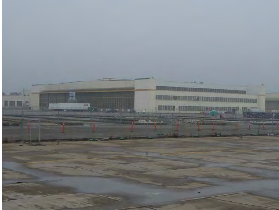
Photograph 1: Building 39, camera facing northeast, December 16, 2009.
