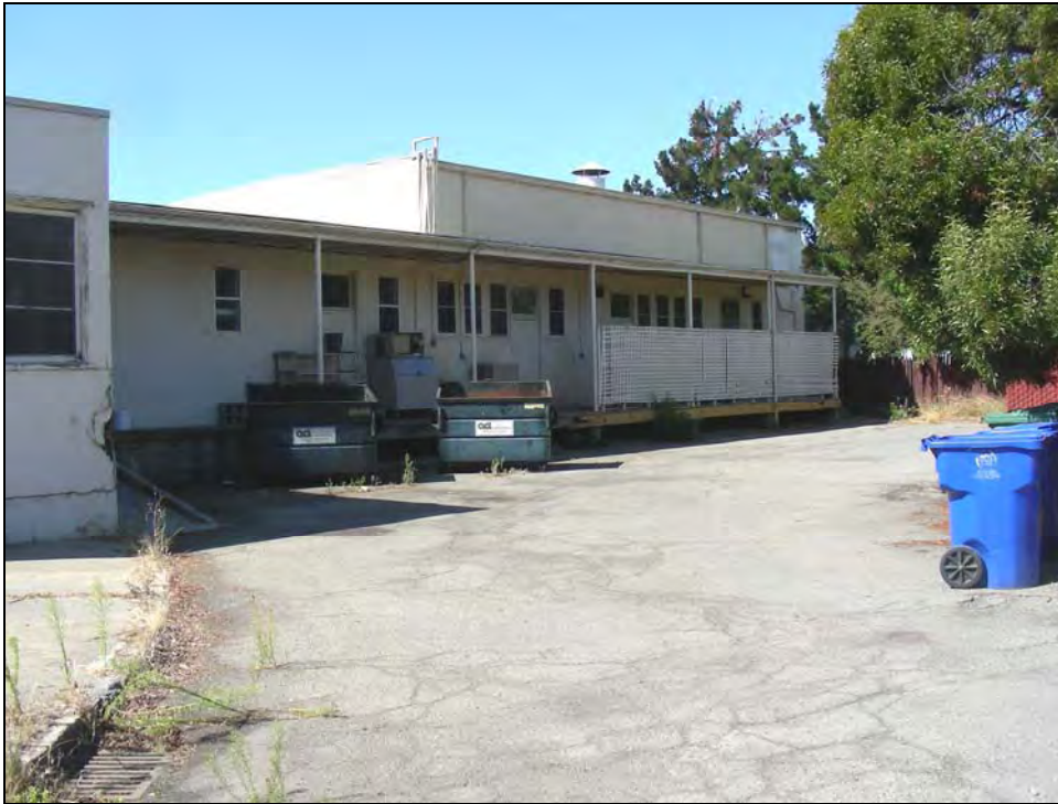
Photograph 4: East side, camera facing northwest, September 29, 2009.
