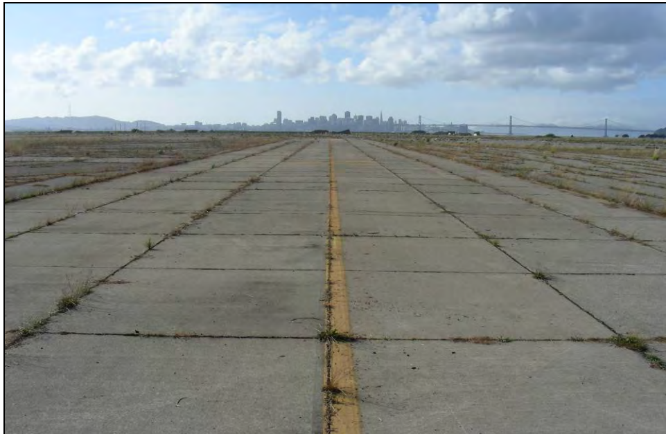
Photograph 17: Taxiway F, camera facing west, October 14, 2009.
