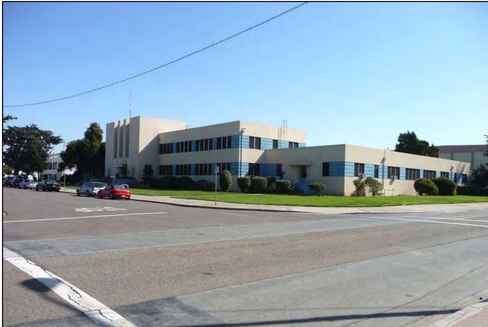
Photograph 1: Building 1, camera facing southeast, October 6, 2009.
