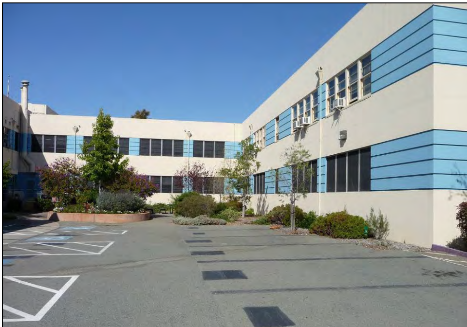
Photograph 5: Building 1, Courtyard – north building and east wing, camera facing northeast, October 6, 2009.
