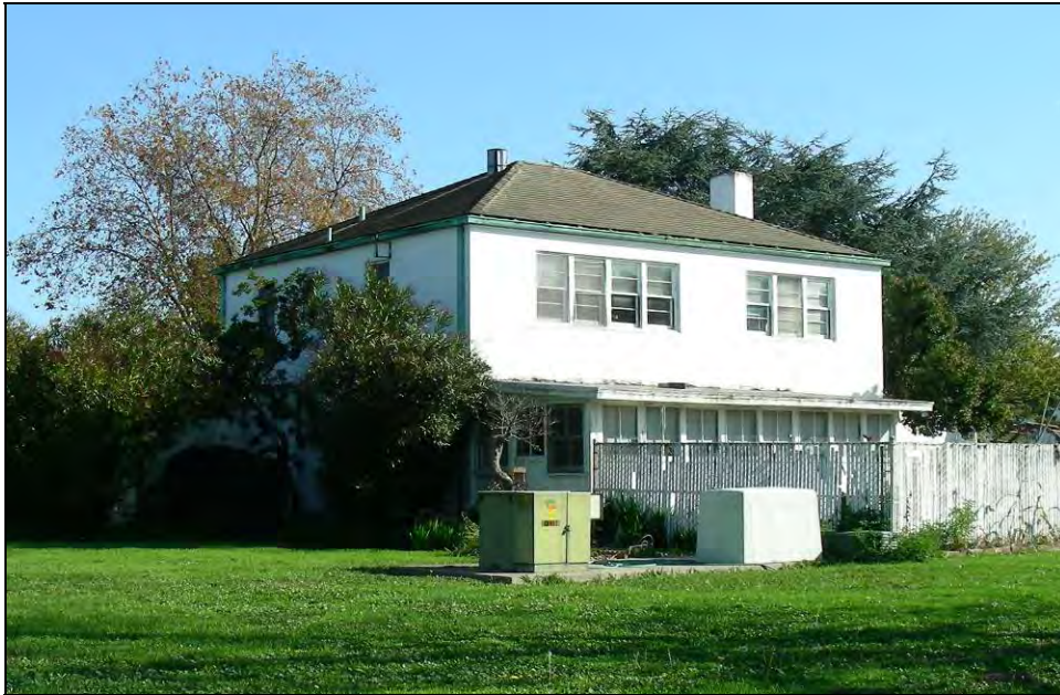
Photograph 3: Typical rear sun porch, building FH-N, camera facing northeast, November 12, 2009.
