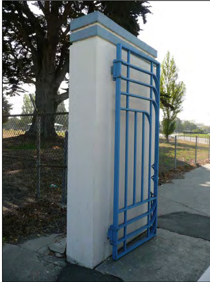
Photograph 2: Main Gate pedestrian gate posts and gate, camera facing southeast, September 25, 2009.
