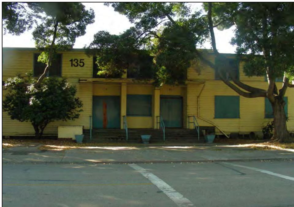
Photograph 2: Building 135, main entrance on north side of building, facing south, October 6, 2009.
