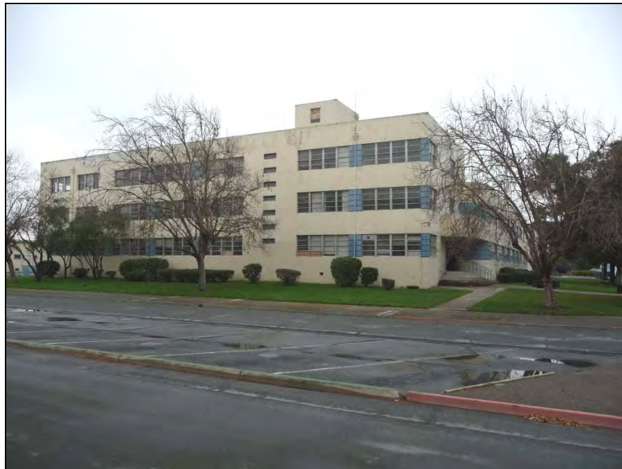
Photograph 2: North wall, camera facing southeast, December 16, 2009.
