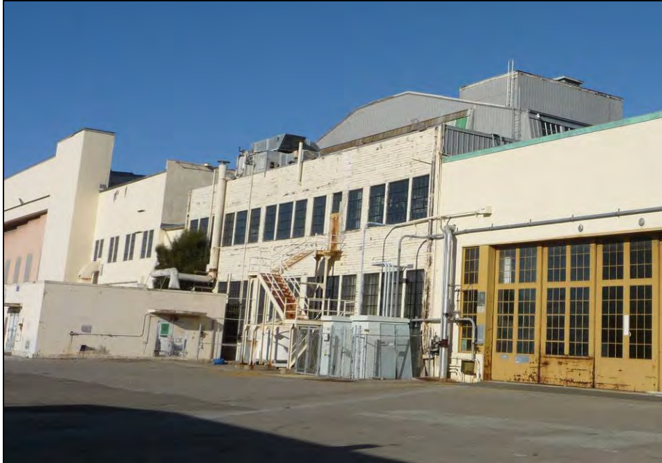
Photograph 7: Northwest extension center, Building 347 to the left, camera facing northeast, September 29, 2009.
