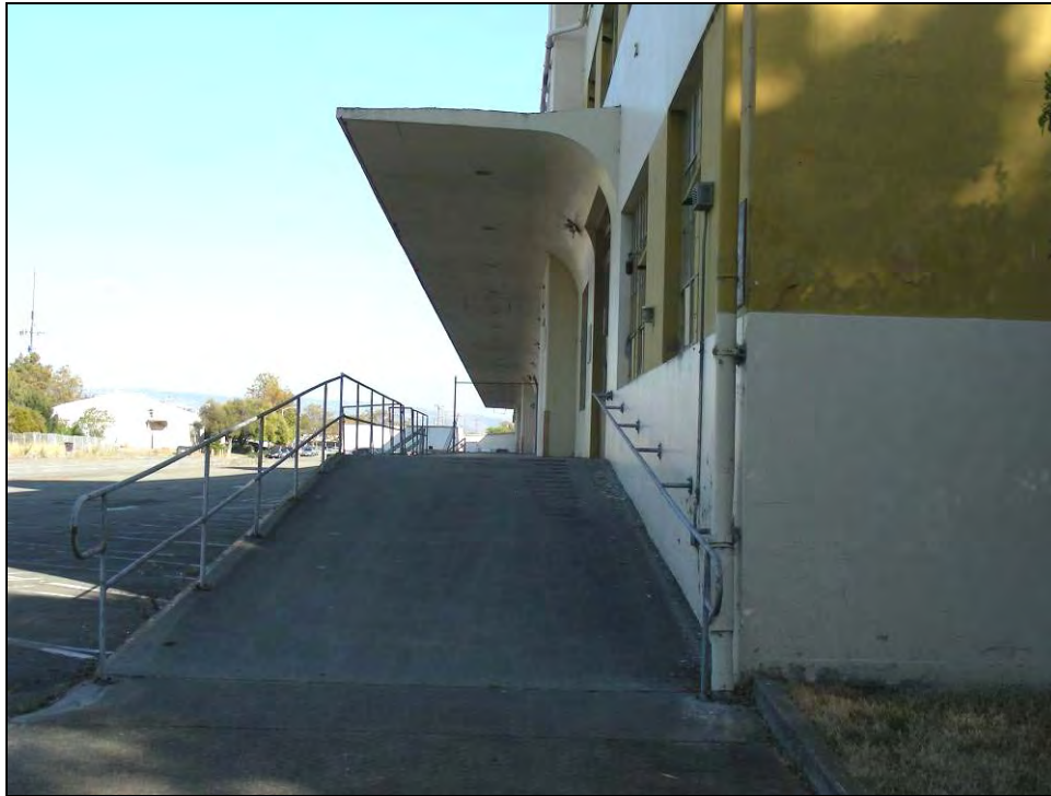
Photograph 3: Curved cantilevered concrete roof along north side, camera facing east, October 7, 2009.
