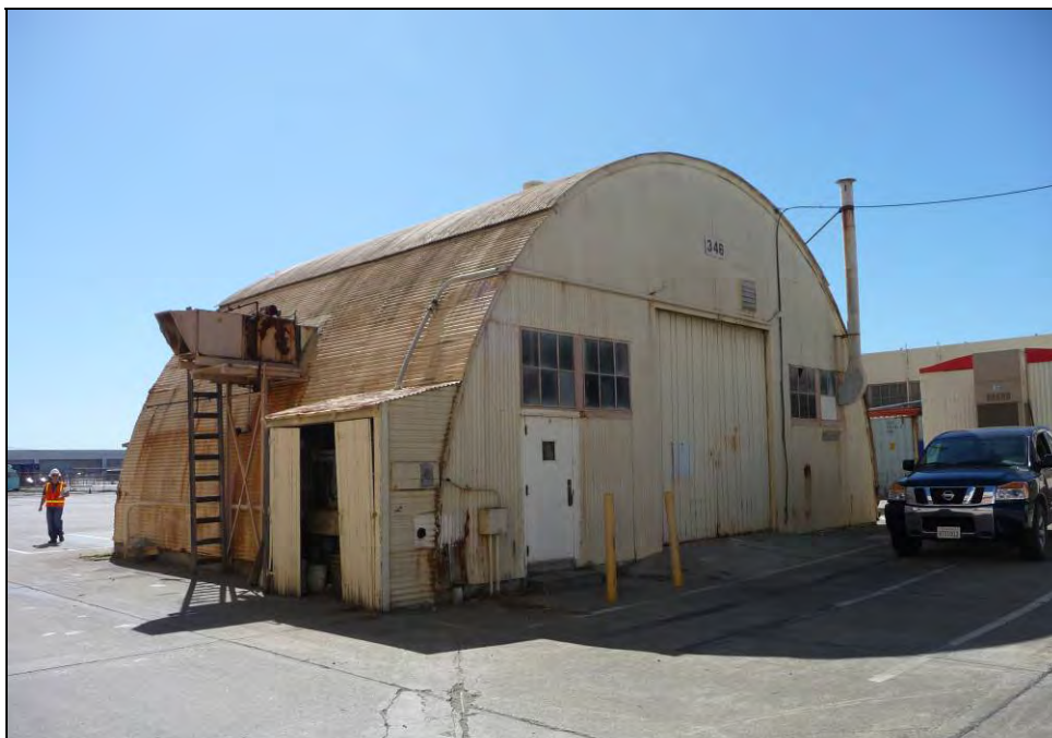
Photograph 2: North side, camera facing southwest, October 1, 2009.
