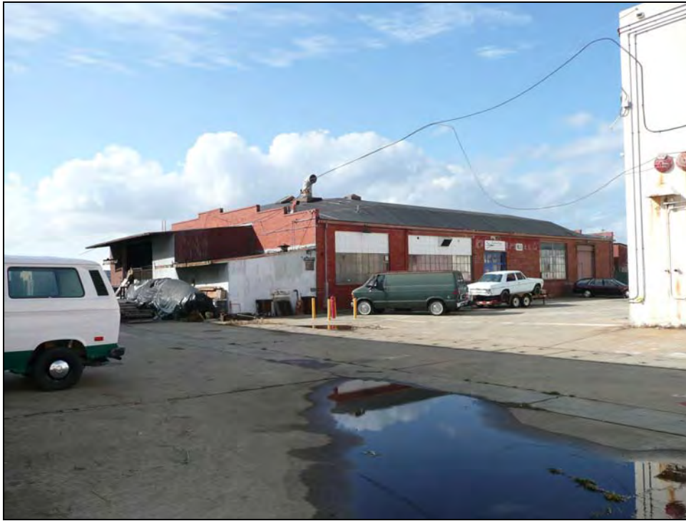
Photograph 5: Camera facing northwest, October 14, 2009.
