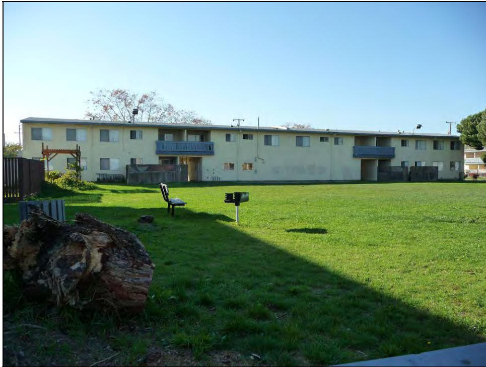
Photograph 13: Four G and two J units, Building FH-808, camera facing west, November 3, 2009.
