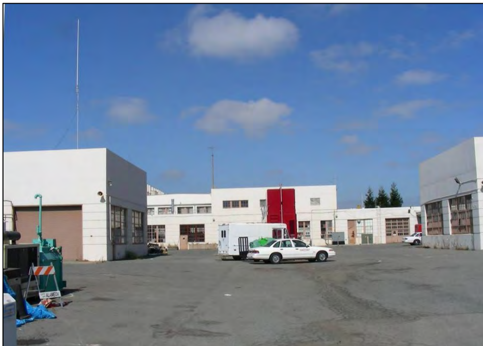
Photograph 7: South side courtyard, camera facing north, October 8, 2009.
