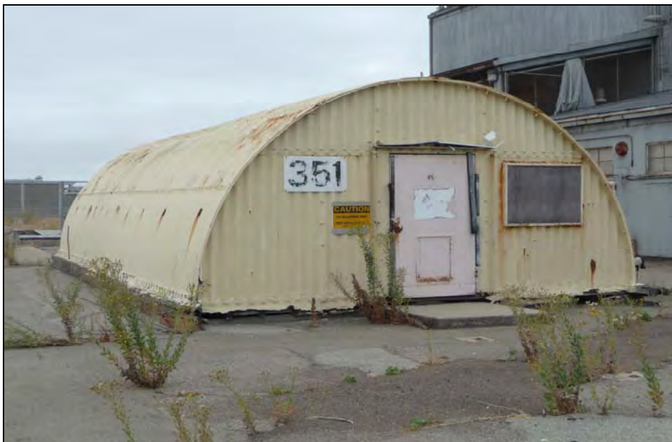
Photograph 4: Building 351, camera facing southeast, October 8, 2009.
