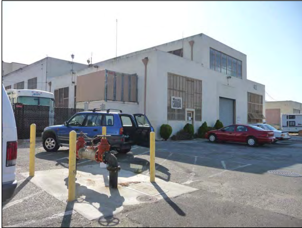
Photograph 1: Camera facing southeast, October 6, 2009.
