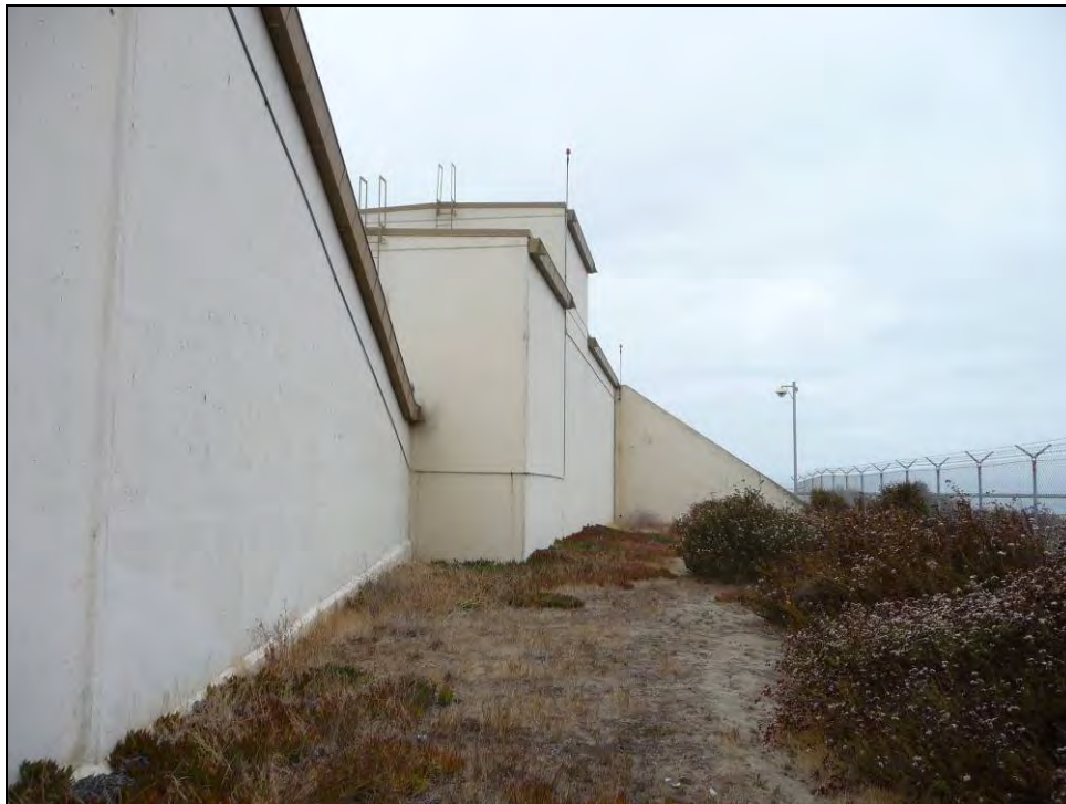
Photograph 9: South end of west side, camera facing south, October 8, 2009.
