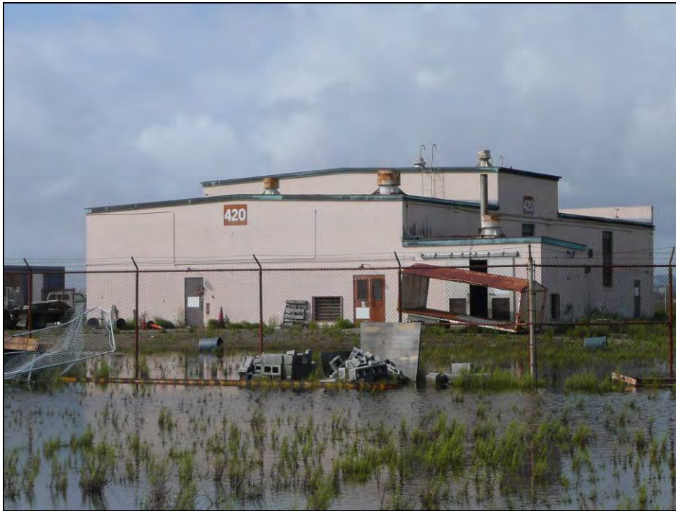
Photograph 4: Building 420 East side, camera facing west, October 14, 2009.
