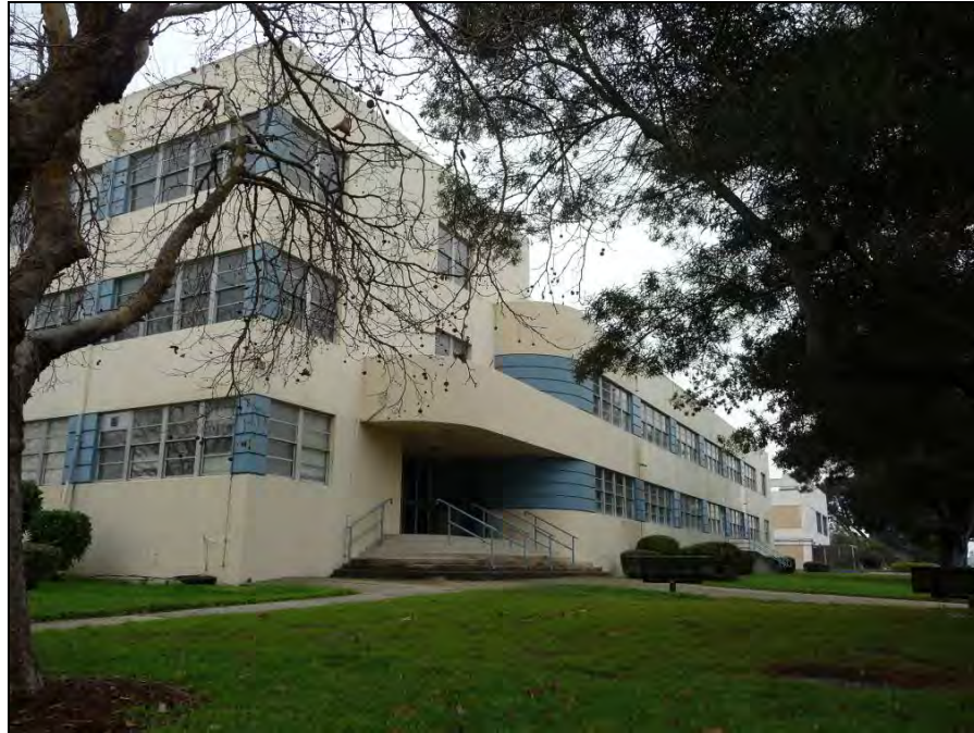
Photograph 1: Main entrance at northwest corner, camera facing south, December 16, 2009.
