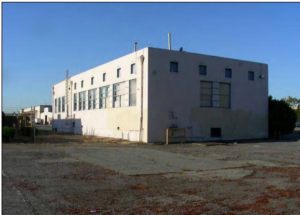
Photograph 2: Camera facing southwest, October 7, 2009.
