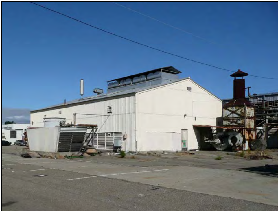
Photograph 2: Camera facing northeast, October 15, 2009.
