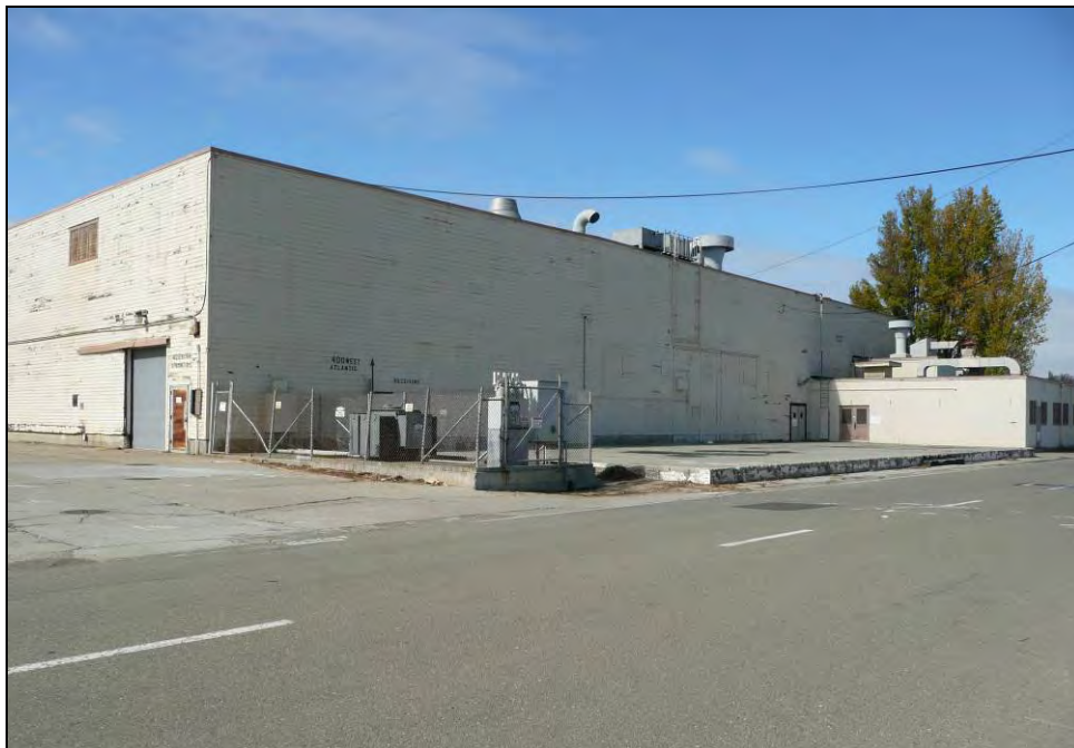
Photograph 7: Northeast addition and east wall, camera facing northwest, October 15, 2009.
