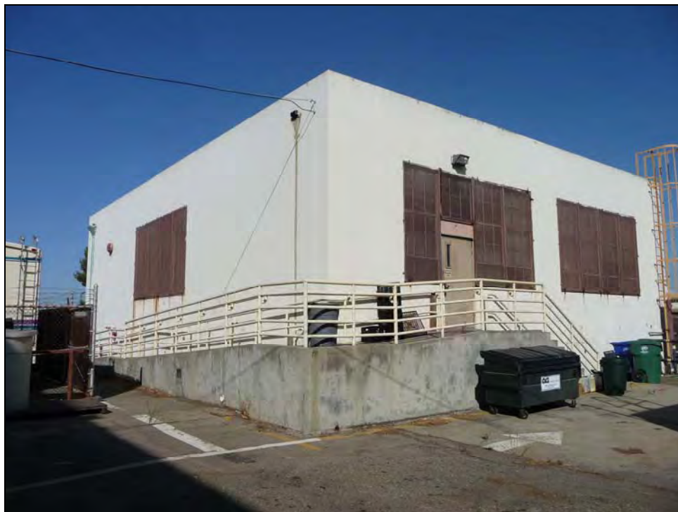
Photograph 4: Southeast corner, camera facing northwest, October 6, 2009.
