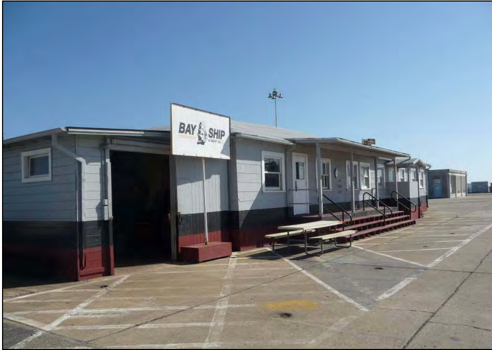
Photograph 2: Building 292, camera facing southeast, October 8, 2009.
