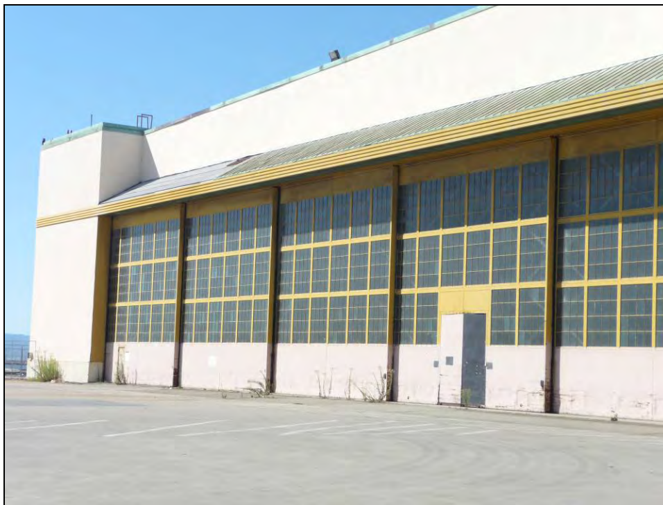
Photograph 4: Building 12 showing hangar doors, camera facing southwest, October 1, 2009.
