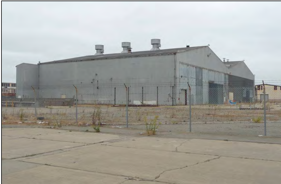
Photograph 2: Building 410, southeast corner, camera facing northwest, October 8, 2009.
