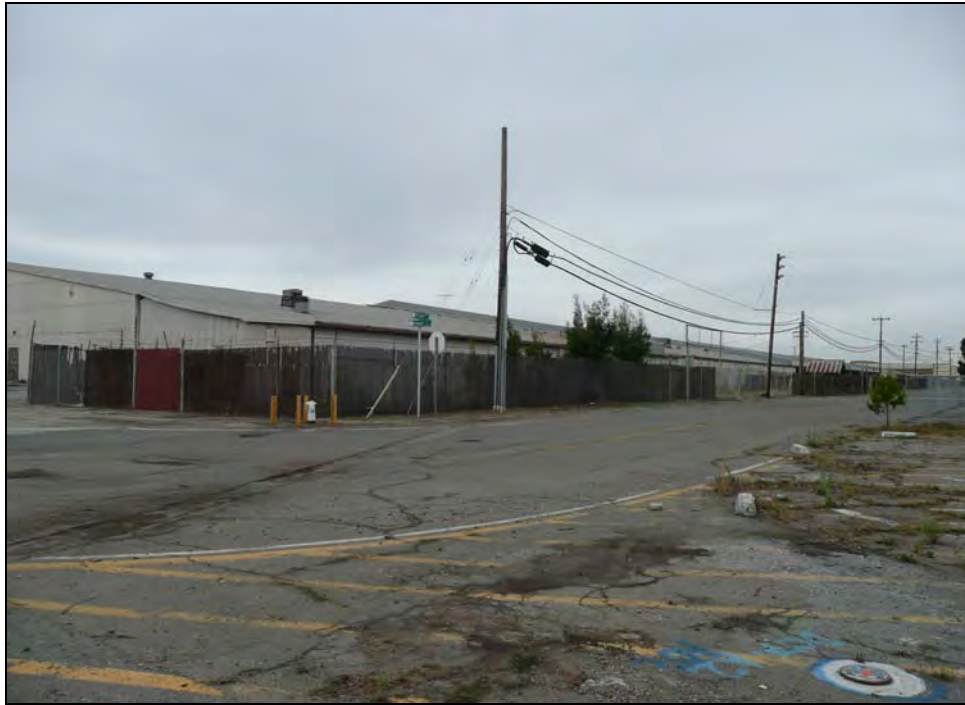
Photograph 4: Camera facing southwest, showing north side, October 15, 2009.
