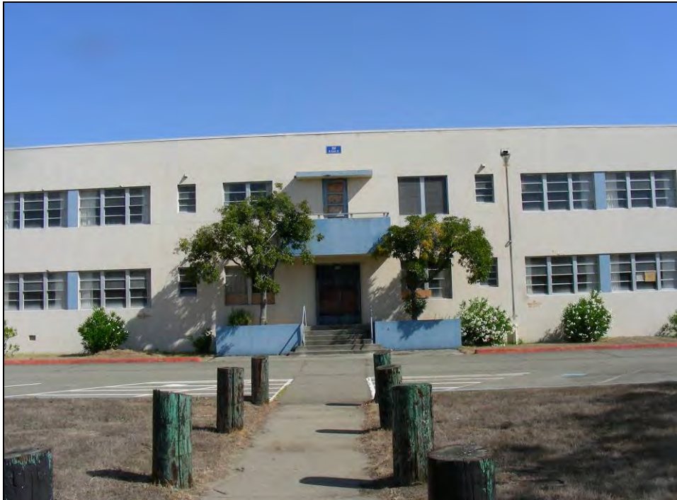
Photograph 5: Entrance at base of U, camera facing east, October 6, 2009.
