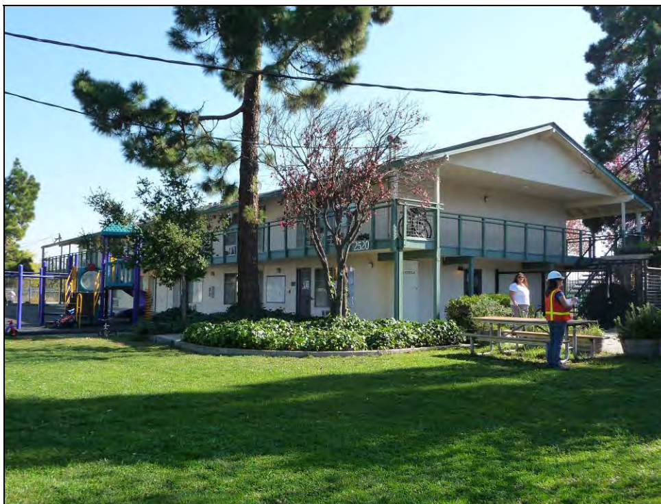
Photograph 2: Building 532, camera facing southeast, November 3, 2009.
