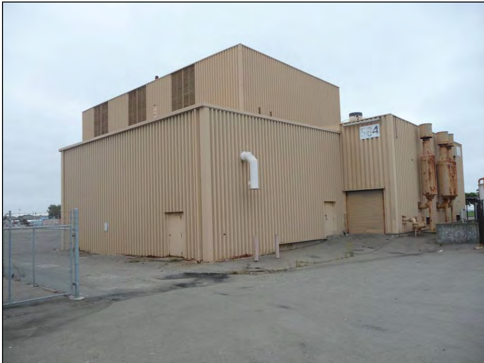
Photograph 3: Building 584, facing southeast, October 8, 2009.
