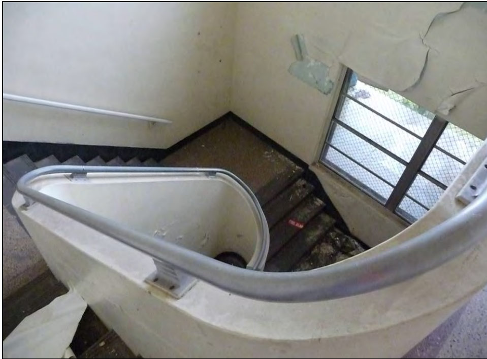
Photograph 13: Curved staircase with metal railing, Building 2, camera facing north, December 11, 2009.
