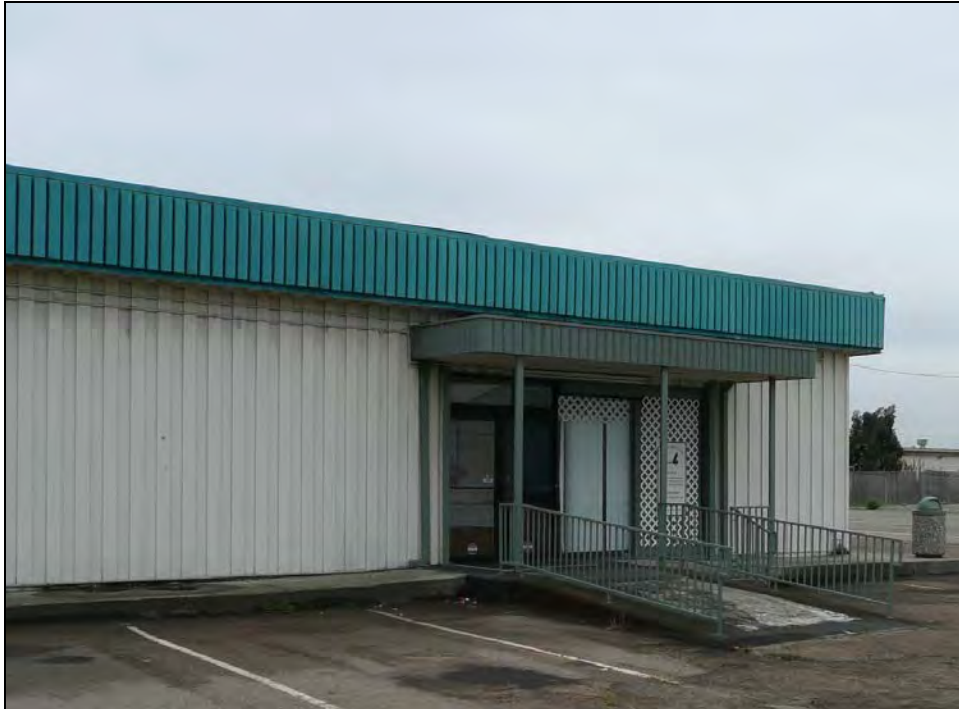
Photograph 2: Main entry detail, camera facing southwest, October 15, 2009.
