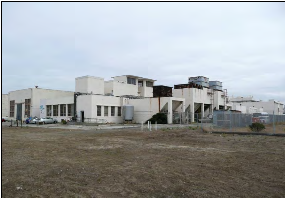
Photograph 1: Western shop and test cells 1-4, camera facing northeast, October 15, 2009. Cells 11 and 12 visible at far right.
