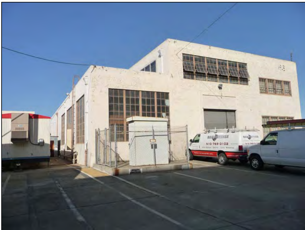
Photograph 4: Southeast corner, camera facing northwest, October 6, 2009.
