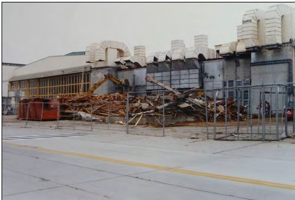
Photograph 20: Demolition of former cleaning shop, ca. 1994, on south side Building 5. 34
