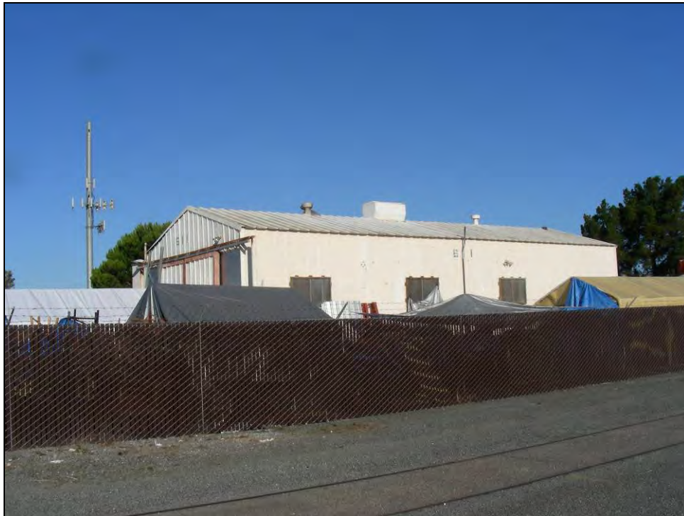
Photograph 2: Camera facing northwest, October 7, 2009.
