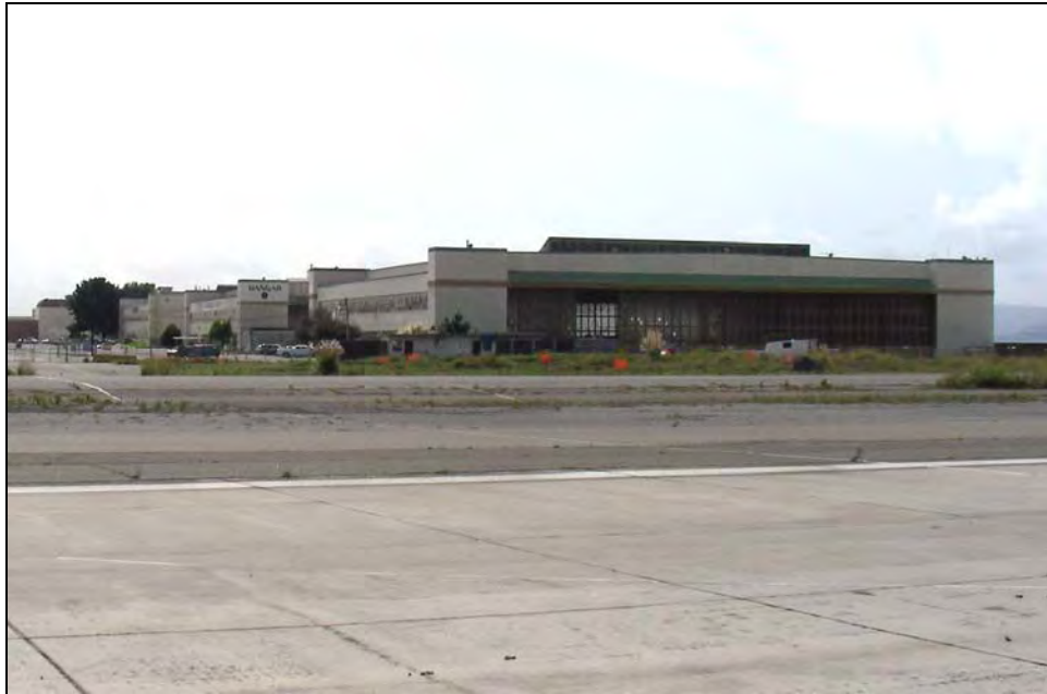
Photograph 1: Hangar 20 in foreground with Hangars 21-23 in background, camera facing south, December 16, 2009.
