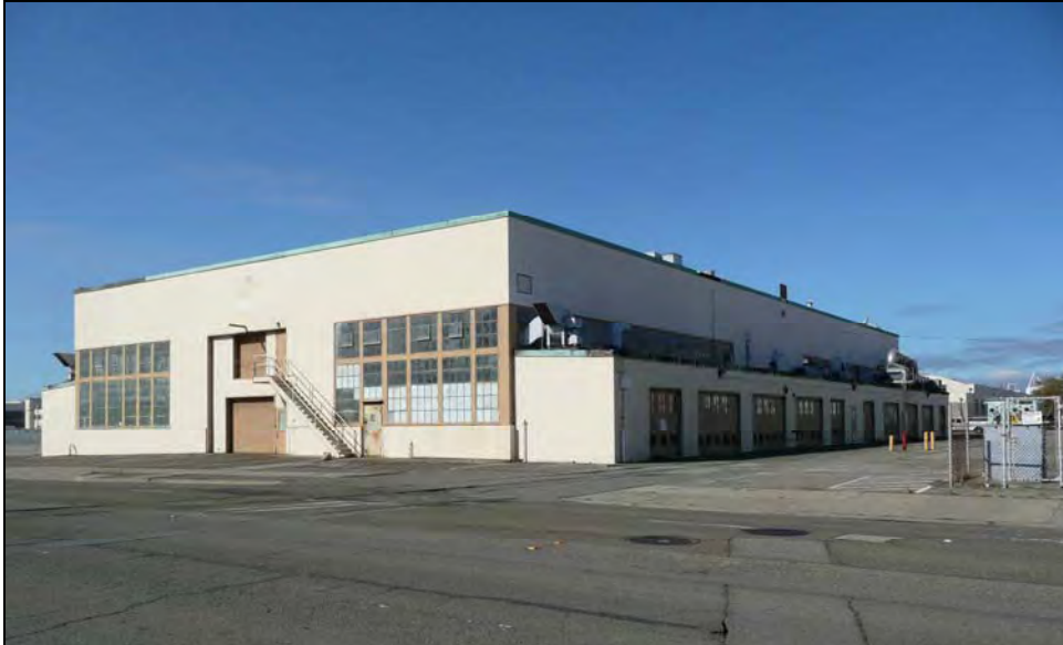
Photograph 2: Building 66, camera facing northwest, October 15, 2009.
