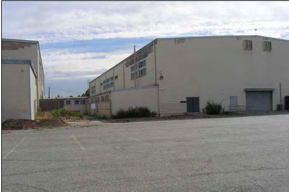
Photograph 4: Building 134 northwest corner, Camera facing southeast, September 29, 2009.
