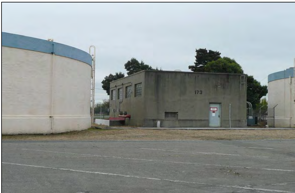
Photograph 4: Tank ladder details, camera facing southwest, October 15, 2009.
