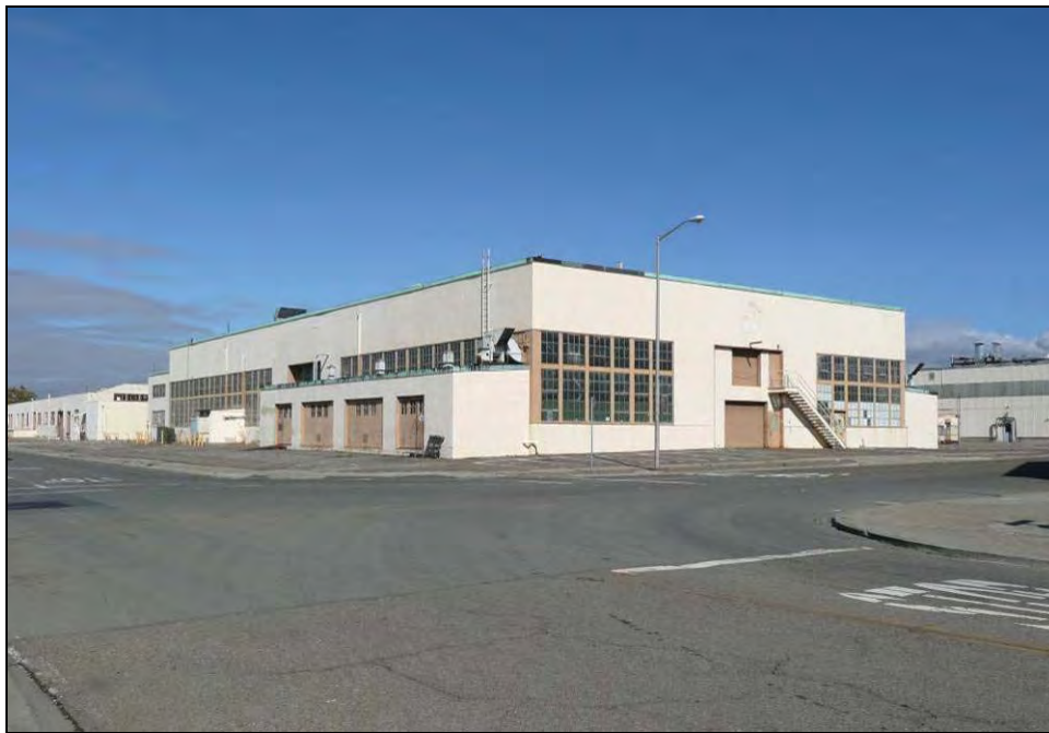
Photograph 42: Engine Accessory Test Shop (Building 66), October 15, 2009.
