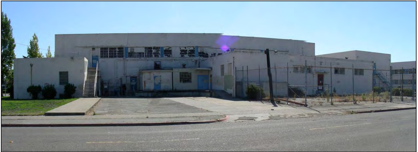
Photograph 11: North side Wing 20 Building 4, camera facing south, October 7, 2009.
