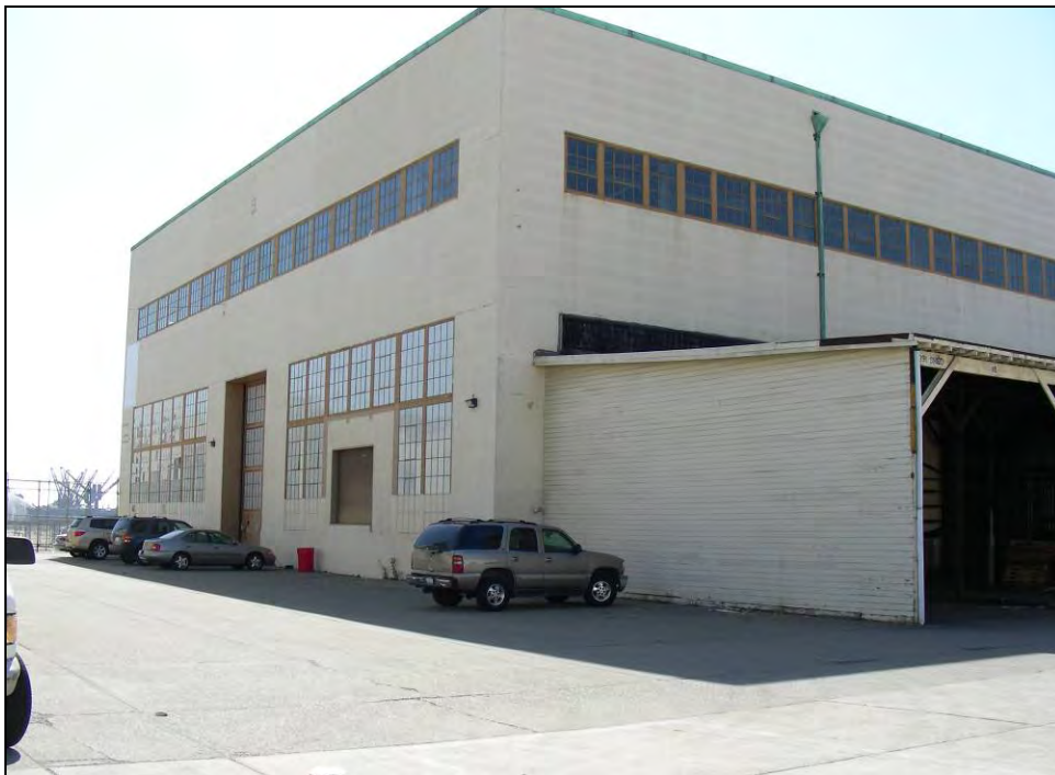
Photograph 4: Northeast corner, camera facing southwest, October 8, 2009.
