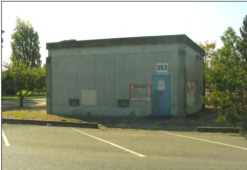
Photograph 56: Electrical Substation No. 6 (Building 553), October 9, 2009.
