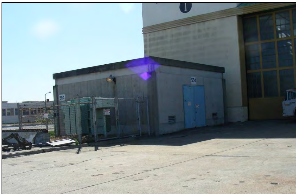
Photograph 3: Building 554, camera facing east, September 30, 2009.
