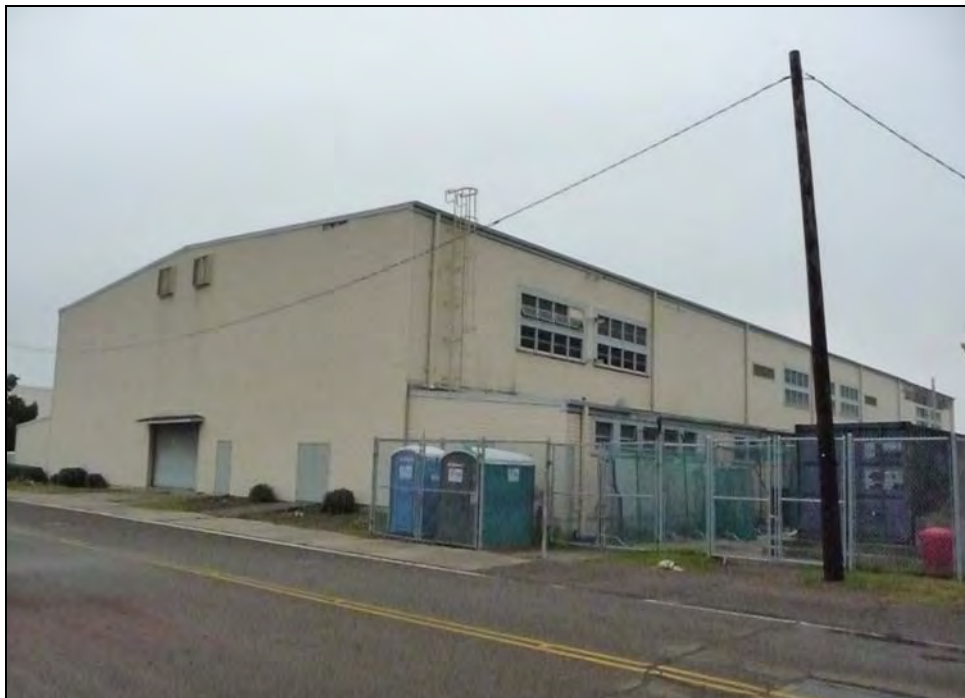
Photograph 6: Building 134 northeast corner, camera facing southwest, December 16, 2009.
