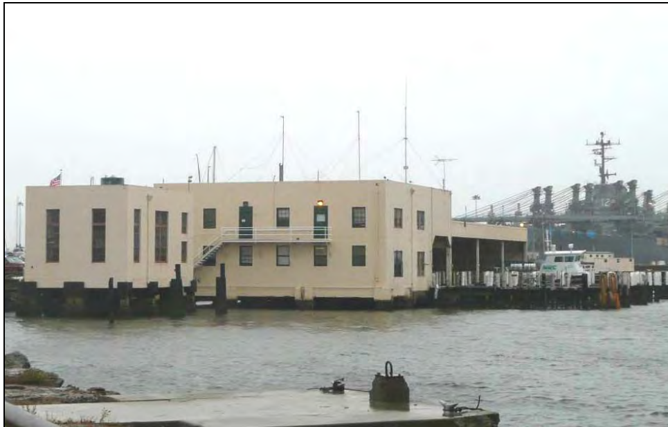
Photograph 3: Camera facing southwest (Building 64 on left), October 13, 2009.
