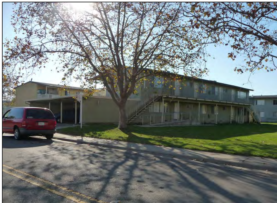
Photograph 14: Building 812, four H units, camera facing southwest, November 3, 2009.
