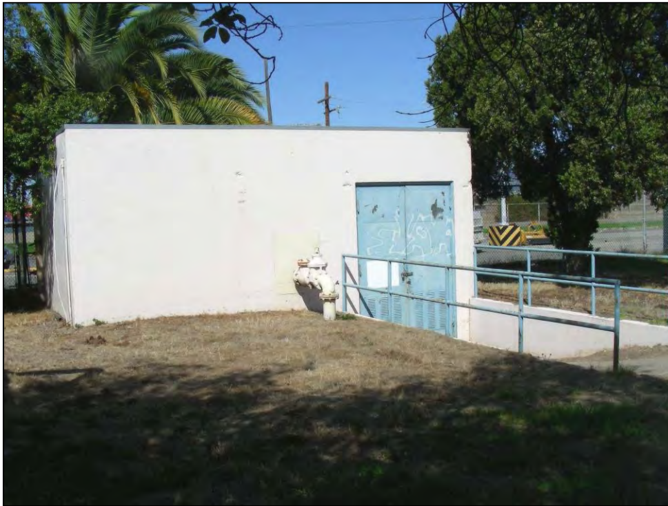
Photograph 5: Building 176, camera facing north, September 29, 2009.
