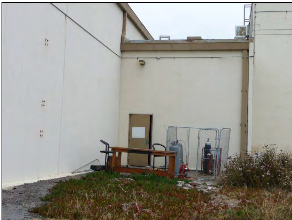
Photograph 11: Detail of north end of west side, camera facing east, October 8, 2009.
