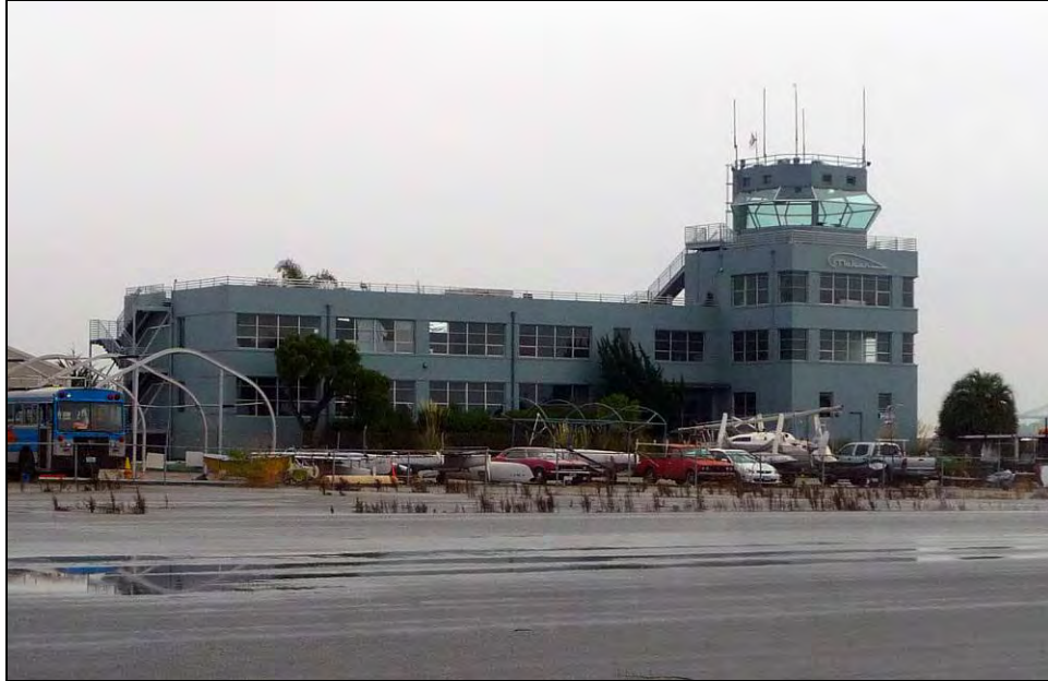
Photograph 1: Building 19, camera facing southeast, December 16, 2009.
