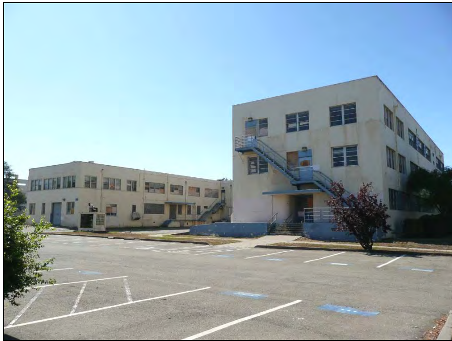
Photograph 3: Camera facing southwest, September 25, 2009.
