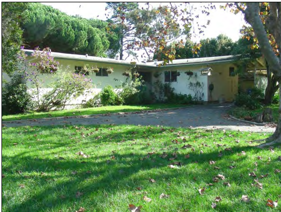
Photograph 3: Typical Plan C, FH-749, camera facing east, November 12, 2009.
