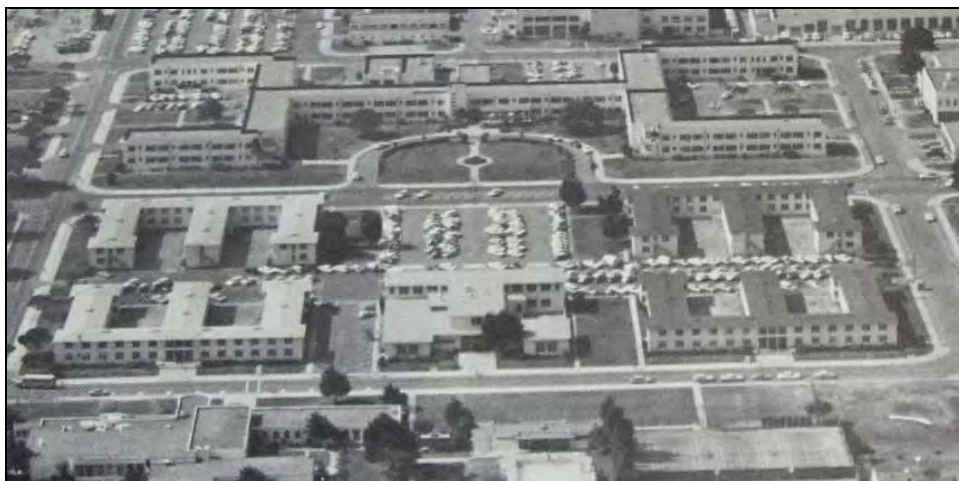
Photograph 39: Building 137 shown below the BOQ landscaped drive, circa 1965. 178
