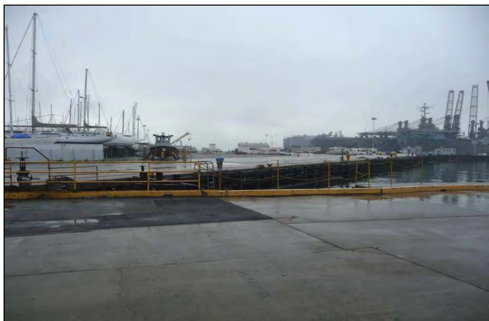
Photograph 12: Pier 1 in foreground with Wharf 1 in background, camera facing southwest, December 16, 2009.
