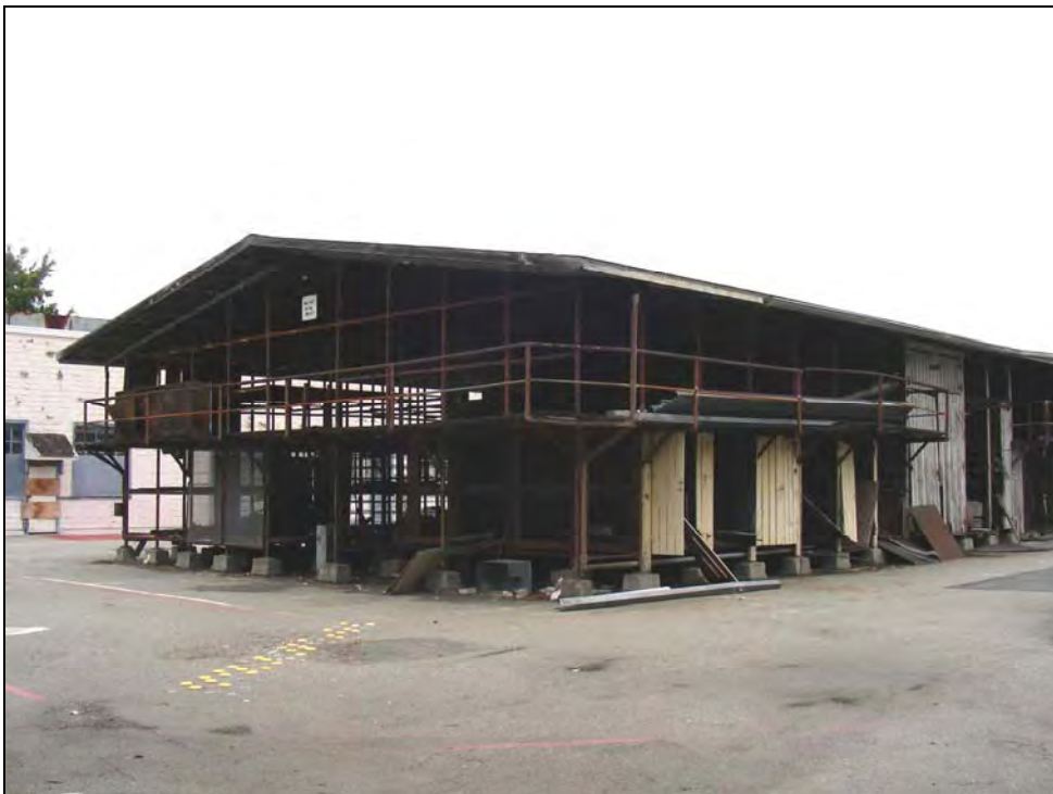
Photograph 3: Southwest corner, camera facing northeast, October 8, 2009.
