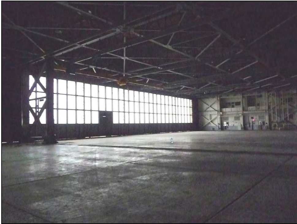
Photograph 7: Interior of Building 12, camera facing southeast, December 11, 2009.
