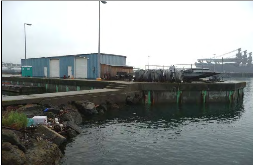
Photograph 3: Building 617A located at west end of pier, camera facing east, December 16, 2009.
