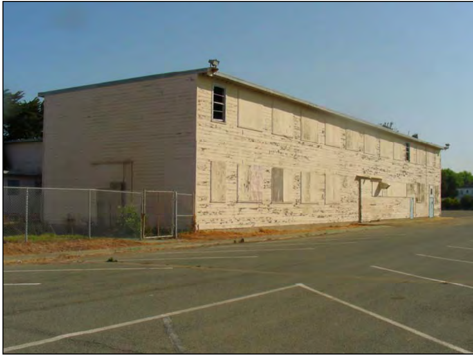
Photograph 5: Building 137, south side, camera facing northeast, October 6, 2009.
