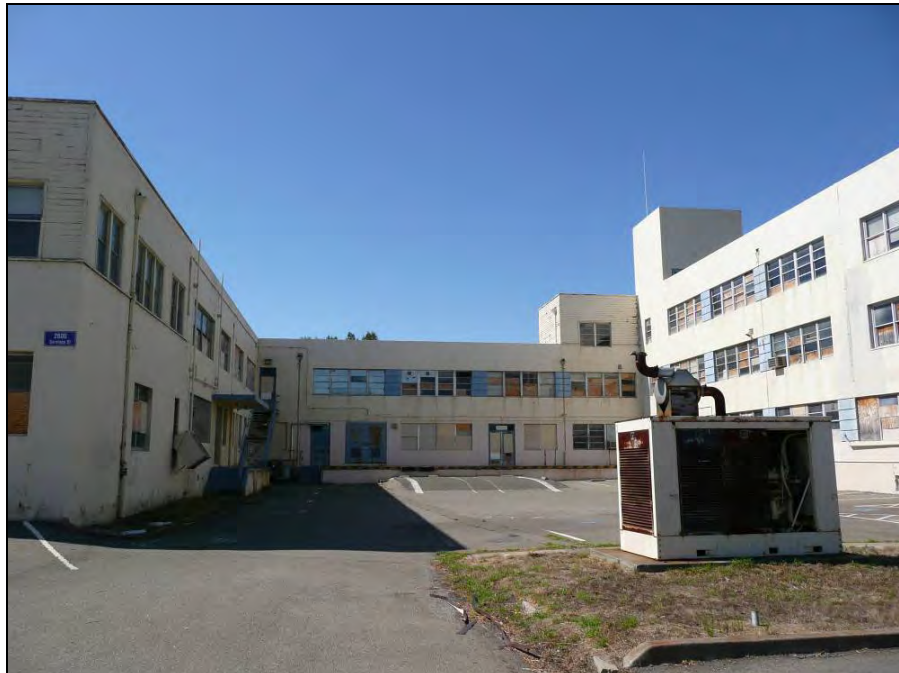
Photograph 4: Camera facing west, September 25, 2009.
