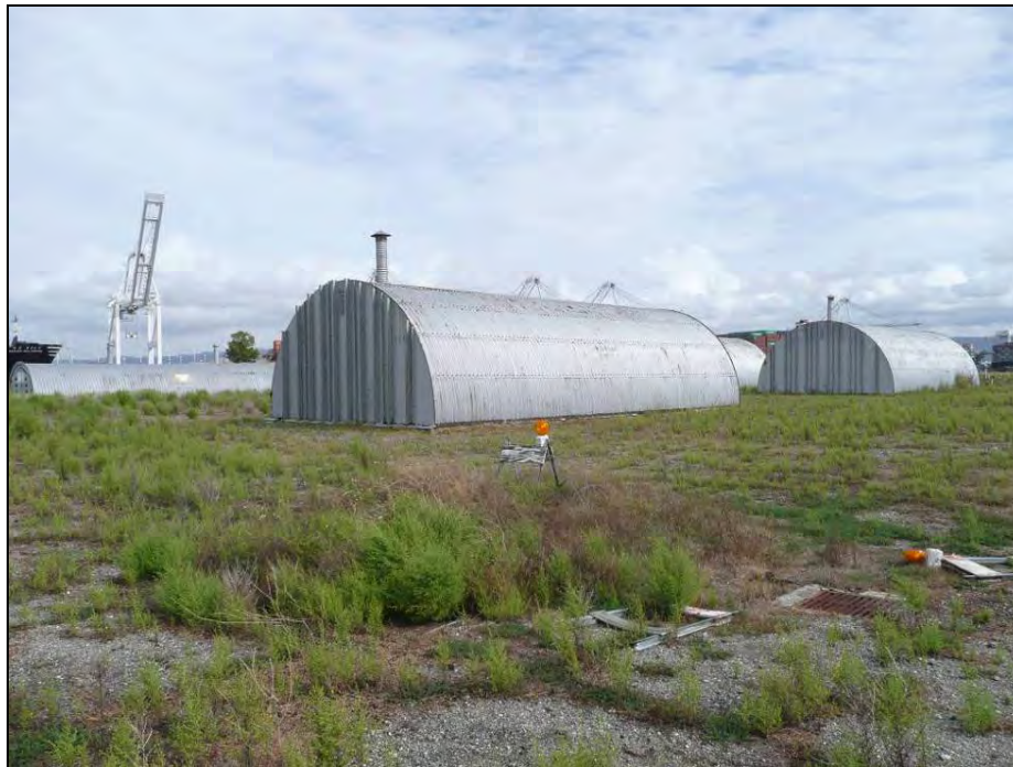
Photograph 2: Building 121 in foreground, camera facing north, October 14, 2009.
