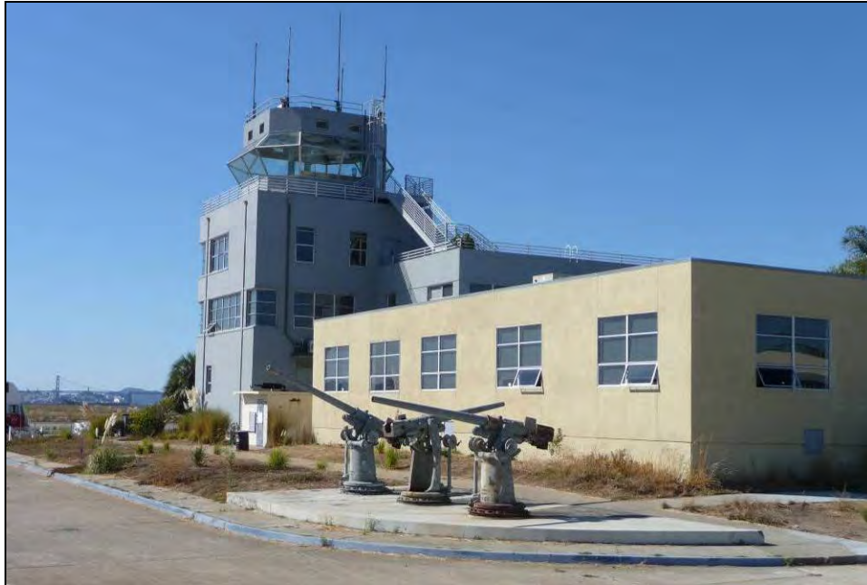
Photograph 3: Building 19, southern portion of east-west wing in foreground, tower in background, camera facing northwest, September 30, 2009.
