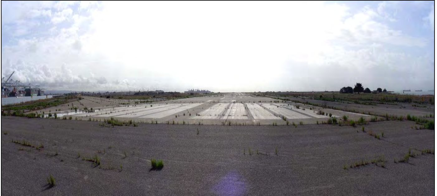
Photograph 16: Panoramic view of Runway 13 (center) and Taxiway C (left), camera facing southeast, October 14, 2009.
