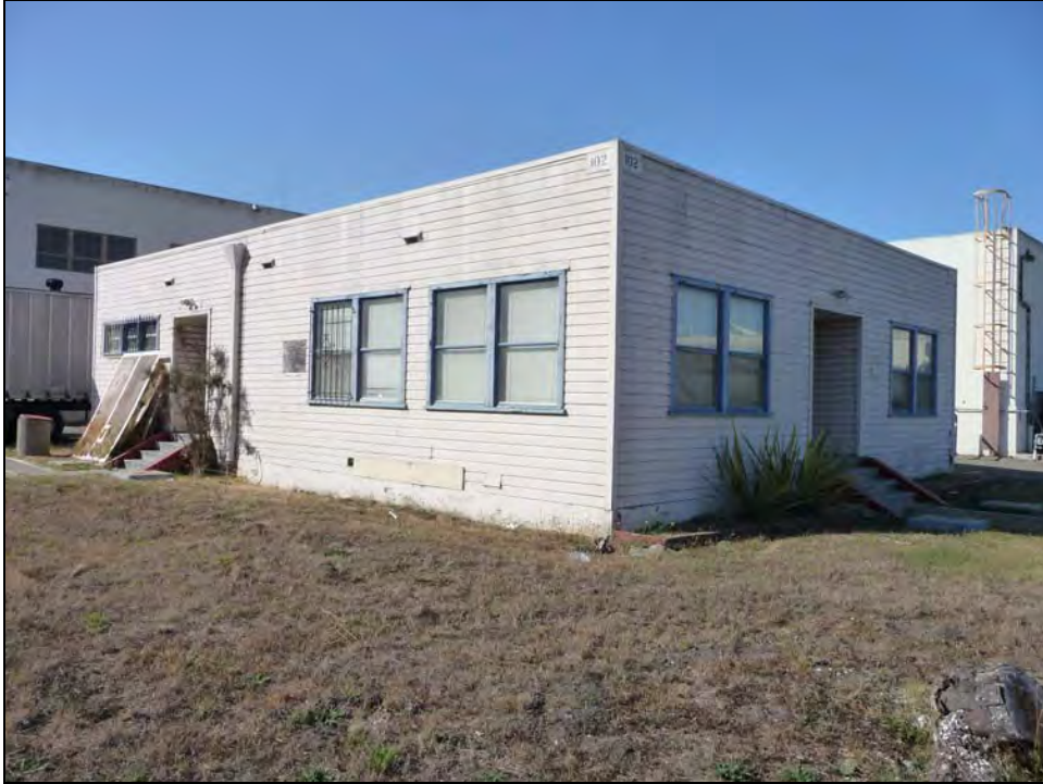
Photograph 1: Camera facing southwest, October 6, 2009.
