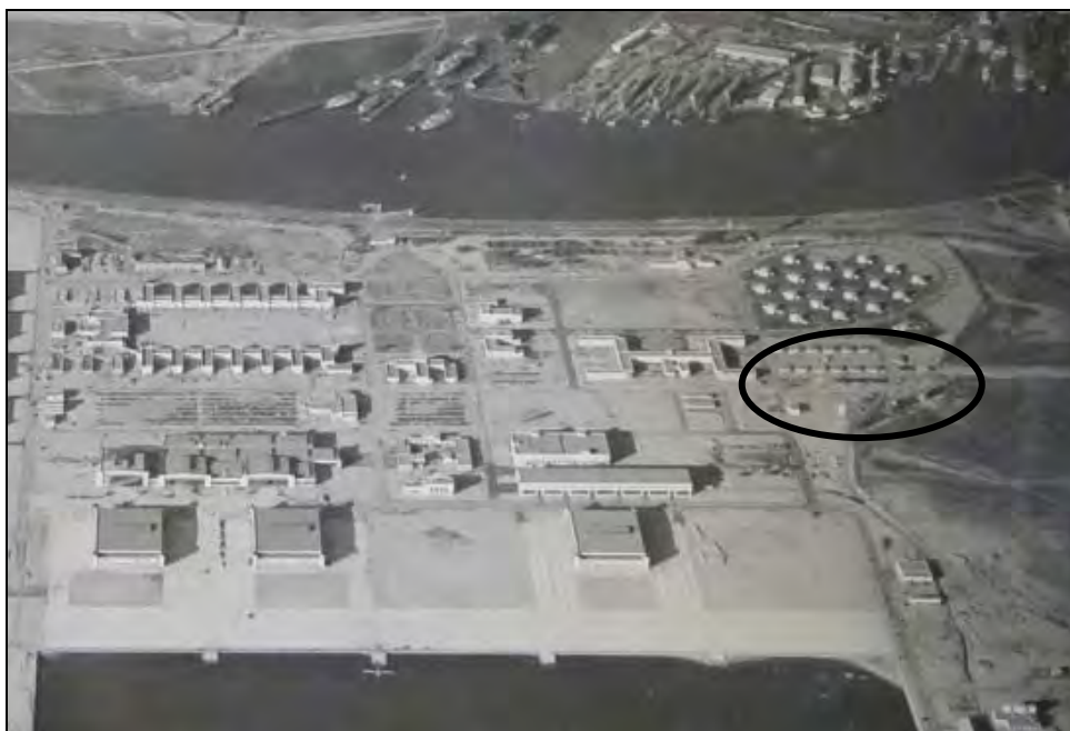
Photograph 6: 1941 photo of the first phase of CPO housing construction, east side not yet filled. 1
