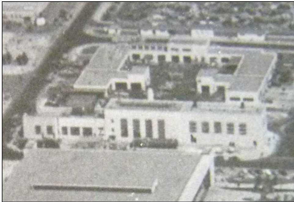
Photograph 6: Completed additions on west and east ends, September 1, 1945, camera facing north. 10
