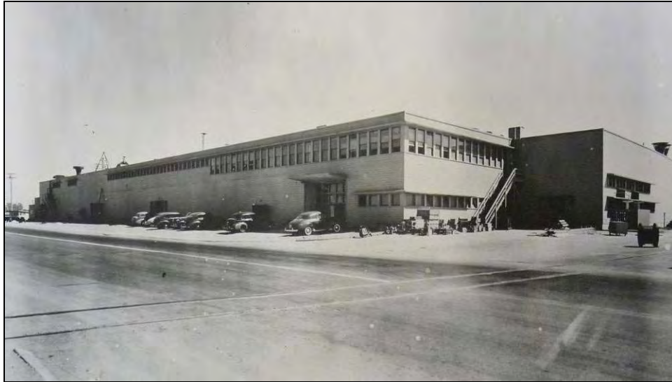
Photograph 29: Building 162, Engine Overhaul Building, was constructed as shown in 1945. Following World War II the interior was reconfigured for assembly line overhaul of both jet and reciprocating piston engines. 122
