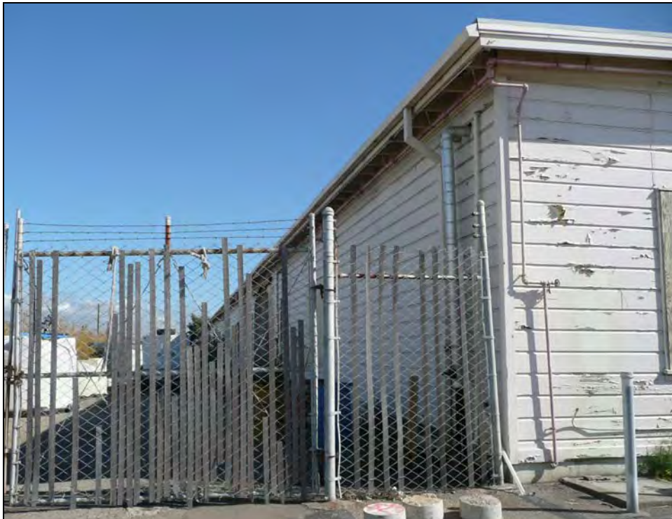
Photograph 2: Camera facing southeast, October 15, 2009.
