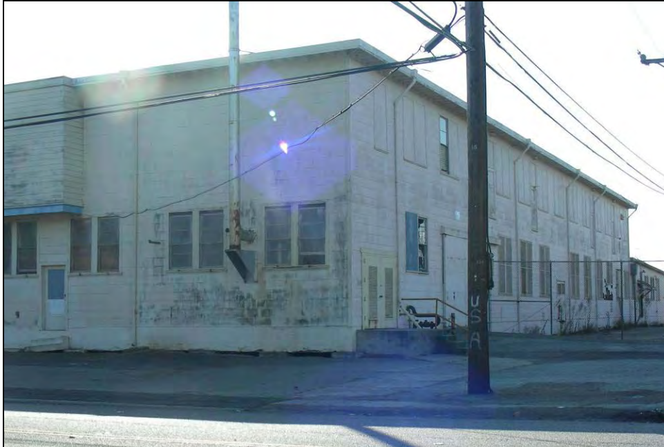
Photograph 11: Northwest corner south wall detail, camera facing southeast, November 12, 2009.
