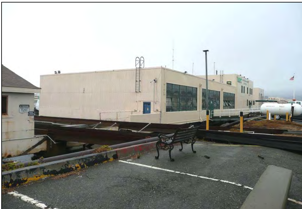
Photograph 2: Camera facing northwest, October 13, 2009.
