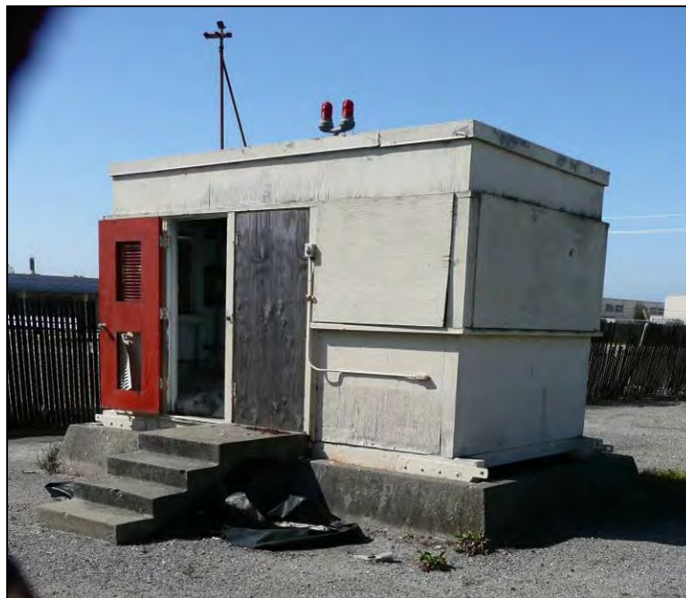
Photograph 11: Building 514, camera facing southwest, September 25, 2009.
