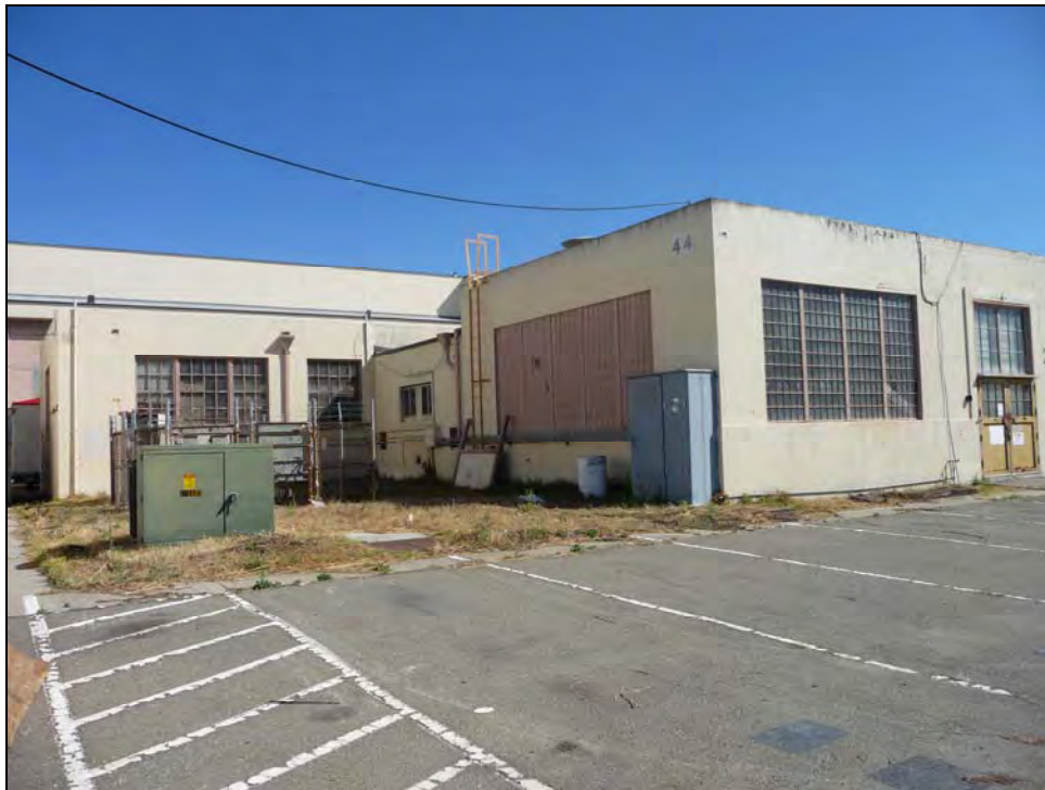
Photograph 4: Camera facing southeast, October 1, 2009.
