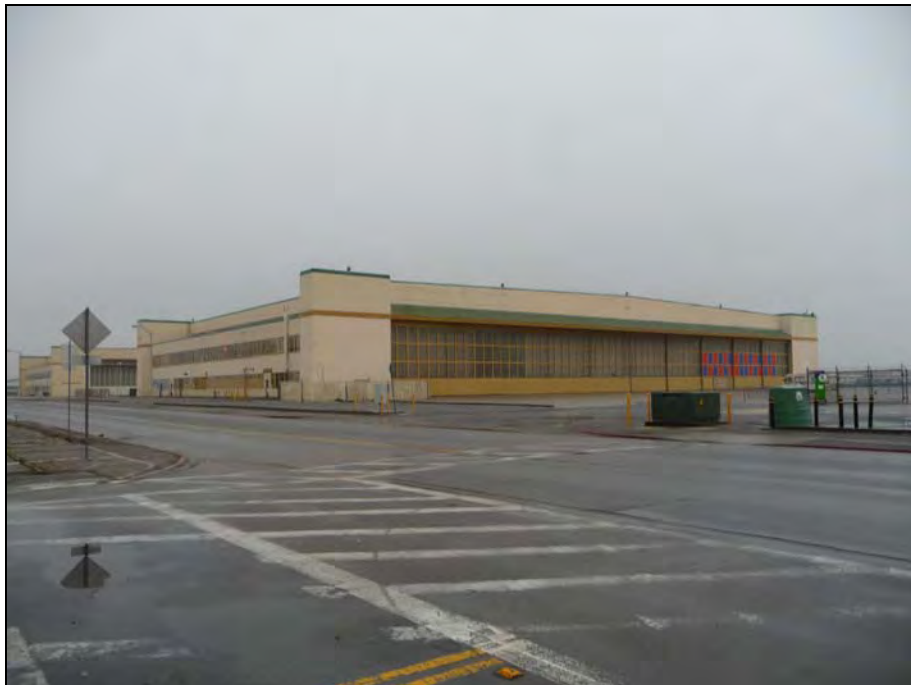
Photograph 2: Building 40, camera facing southeast, October 14, 2009.
