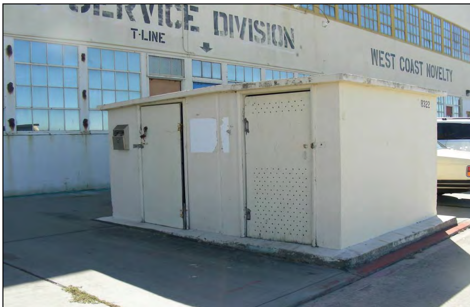
Photograph 6: Building 322, camera facing northeast, September 30, 2009.
