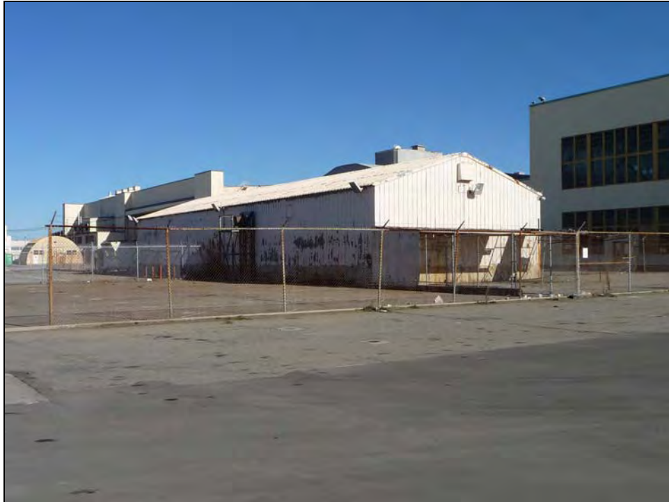
Photograph 2: Camera facing northeast, October 1, 2009.
