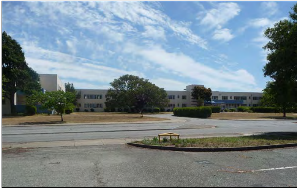
Photograph 3: North side of Building 17 with main entrance, June 9, 2010.
