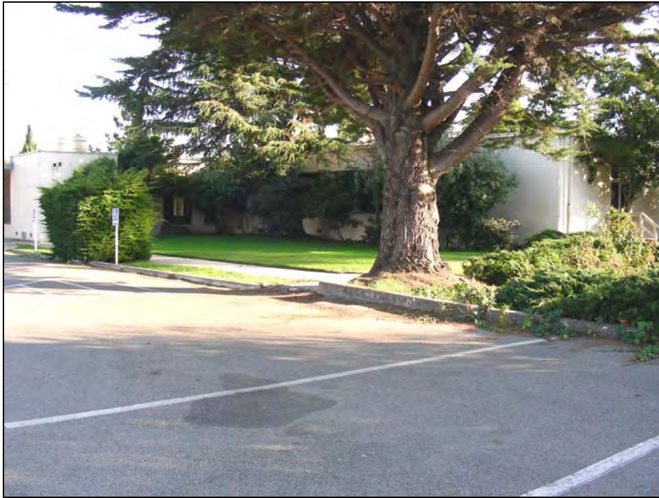
Photograph 8: Northwest corner of east-west wing on west side of building, camera facing southeast, November 12, 2009.
