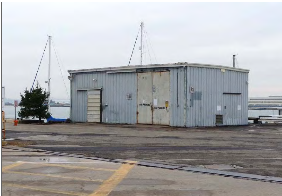
Photograph 61: Oil Water Separator (Building 601), December 11, 2009.
