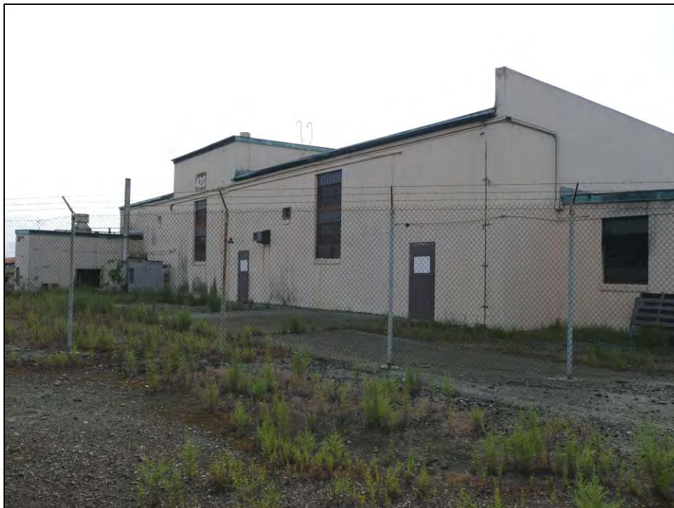
Photograph 3: Building 420 north side, camera facing southeast, October 14, 2009.
