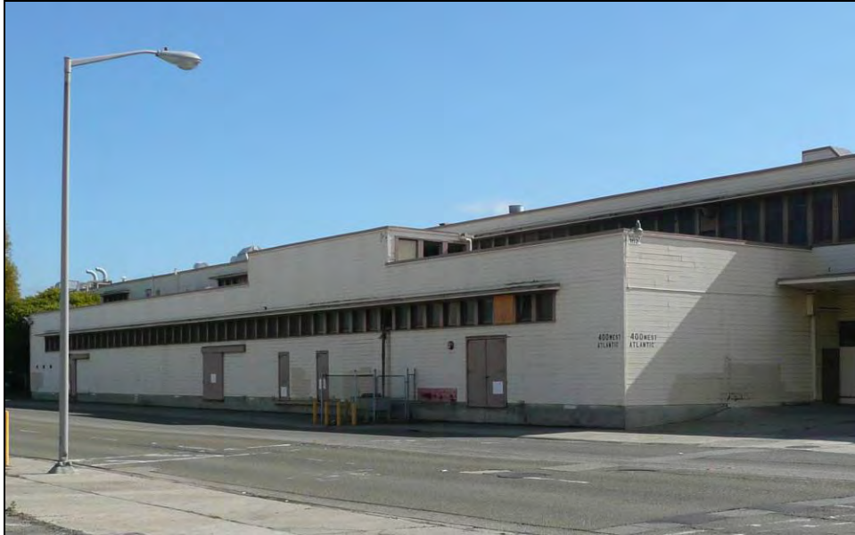
Photograph 4: North side addition, camera facing southeast, October 15, 2009.
