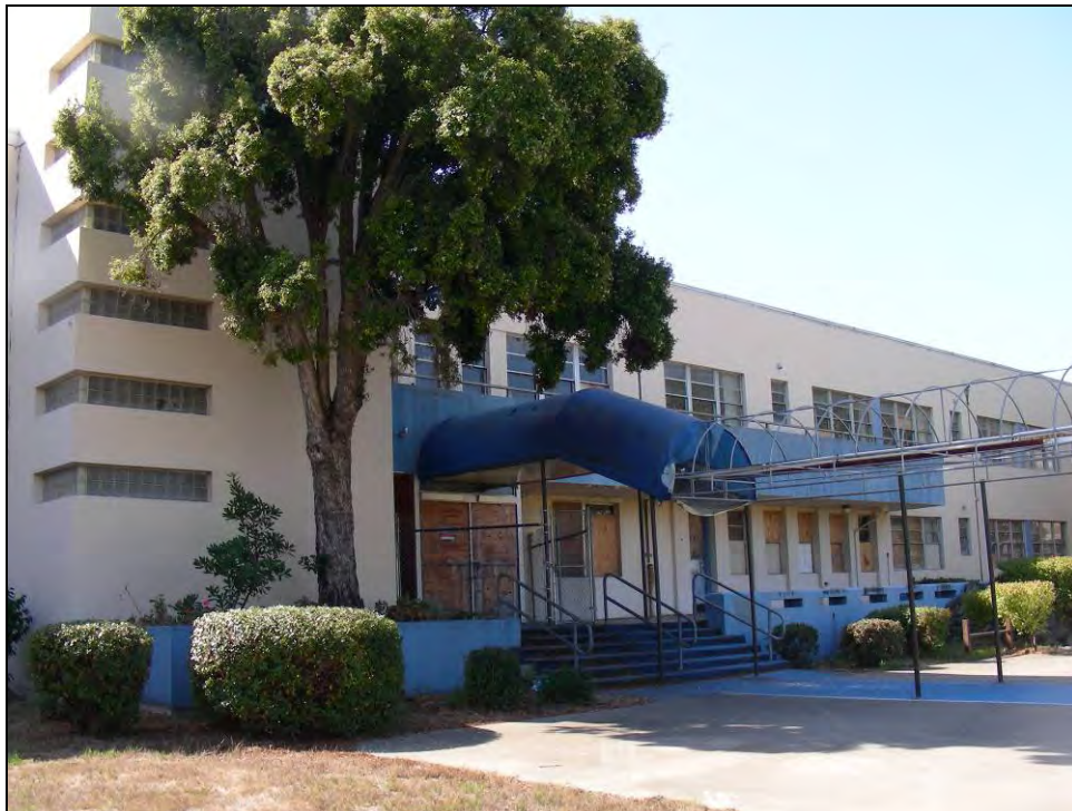
Photograph 4: Detail of main entrance, camera facing southwest, October 6, 2009.
