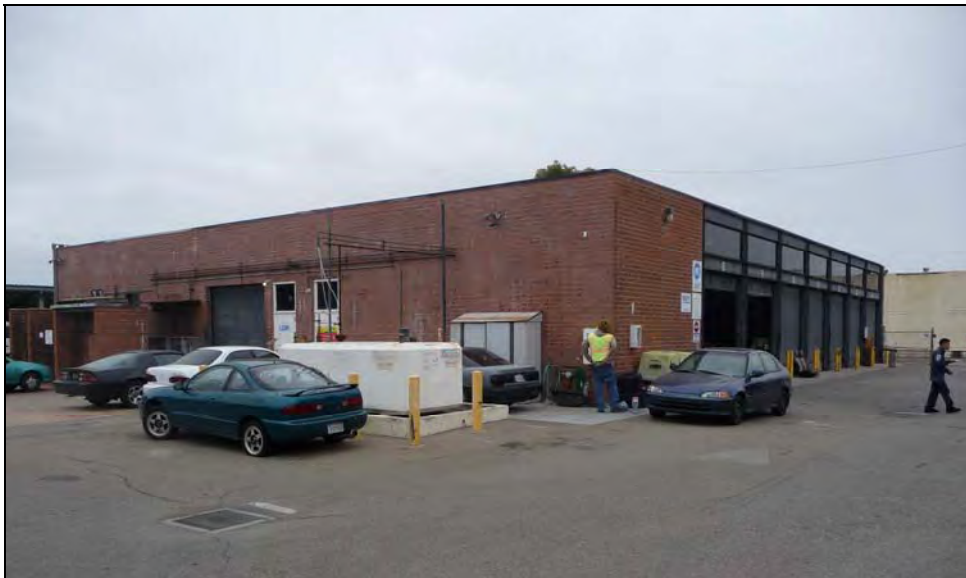
Photograph 3: Building 608, camera facing northwest, October 8, 2009.
