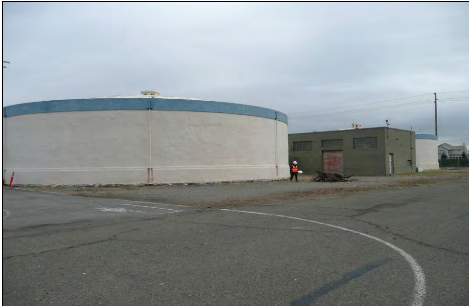
Photograph 3: Building 174A in foreground, October 15, 2009.
