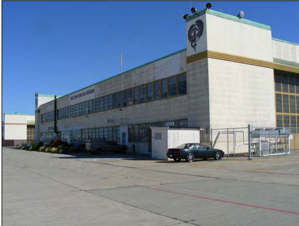
Photograph 3: Hangar 21 west side, camera facing northeast, September 30, 2009.
