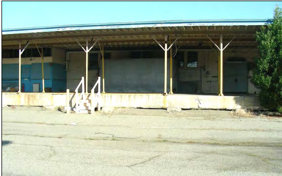
Photograph 6: South side center bay, camera facing north, November 12, 2009.
