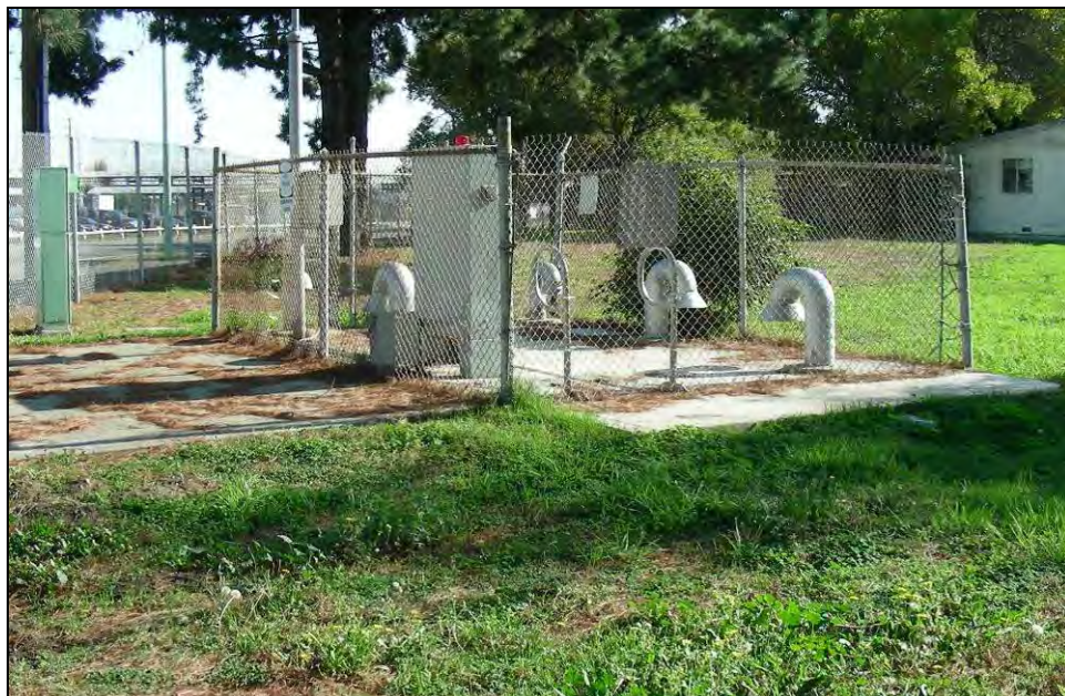
Photograph 11: Building 493, camera facing east, November 12, 2009.
