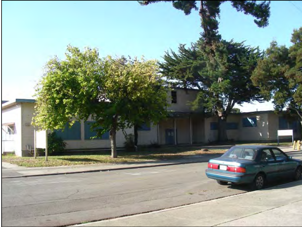
Photograph 3: Building 137, Main entrance, camera facing southwest, October 6, 2009.
