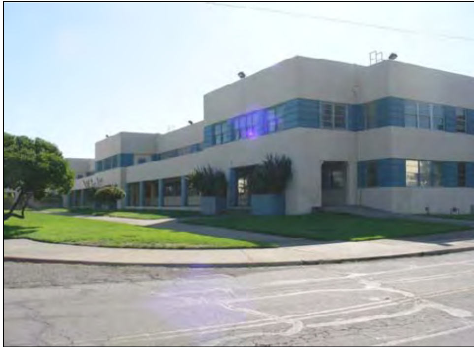
Photograph 3: Courtyard side of Wings 8, 9 and 10, Building 2 illustrating typical elevation. Camera facing Southeast, October 7, 2009.
