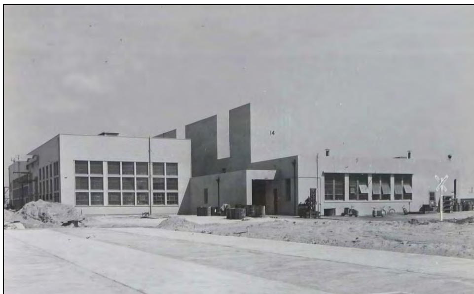
Photograph 28: Building 14, Engine Test Facility, photo dated 1945. 120 The engine test cells were built in stages during World War II and altered starting in 1947 to accommodate jet engines.
