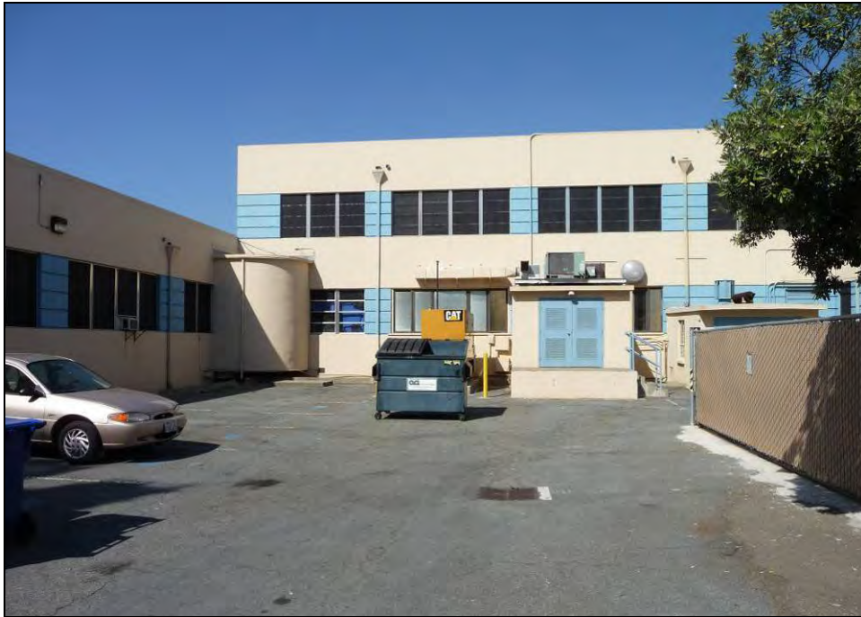
Photograph 8: Building 1, Courtyard - west wing and north building, camera facing north, October 6, 2009.
