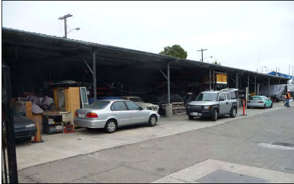
Photograph 6: Building 608 C, camera facing southeast, October 8, 2009.
