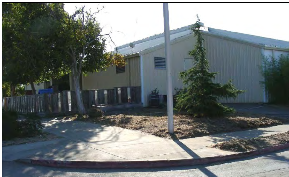
Photograph 2: Camera facing southeast, October 7, 2009.
