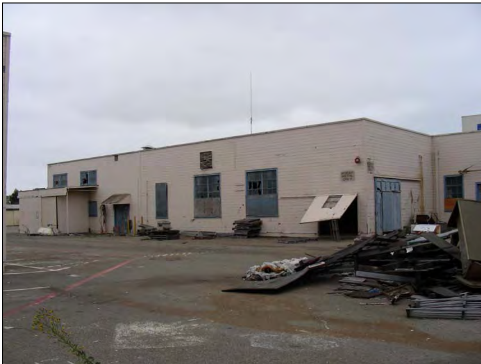
Photograph 3: North side of South Wing, camera facing southeast, October 8, 2009.
