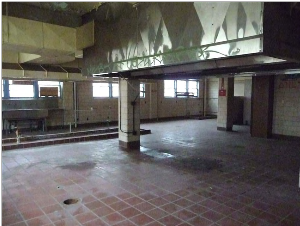
Photograph 10: Kitchen area in Building 17, camera facing southeast, December 11, 2009.
