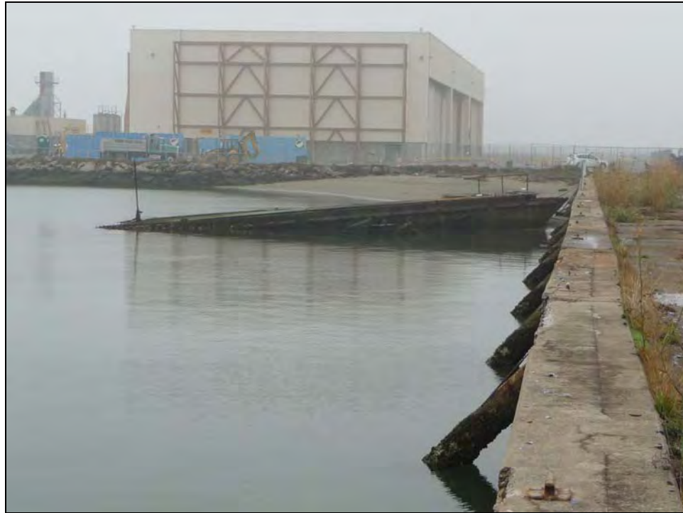
Photograph 7: Barge tied in northwest corner of Seaplane Lagoon and close-up view of Bulkhead, camera facing west, December 16, 2009.
