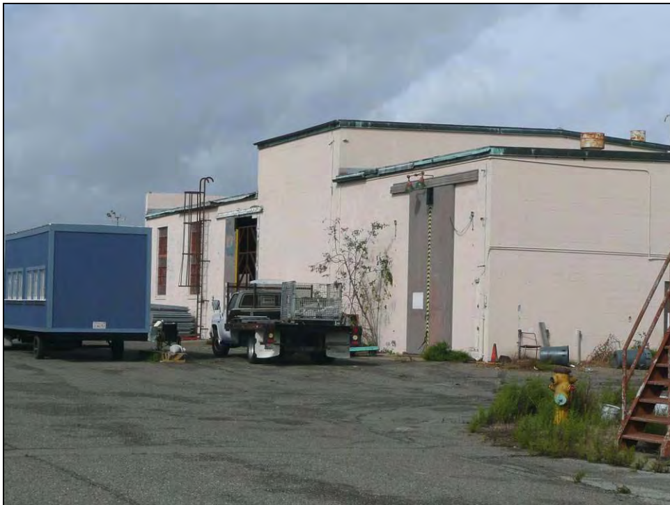
Photograph 5: Building 420 South side, camera facing west, October 14, 2009.
