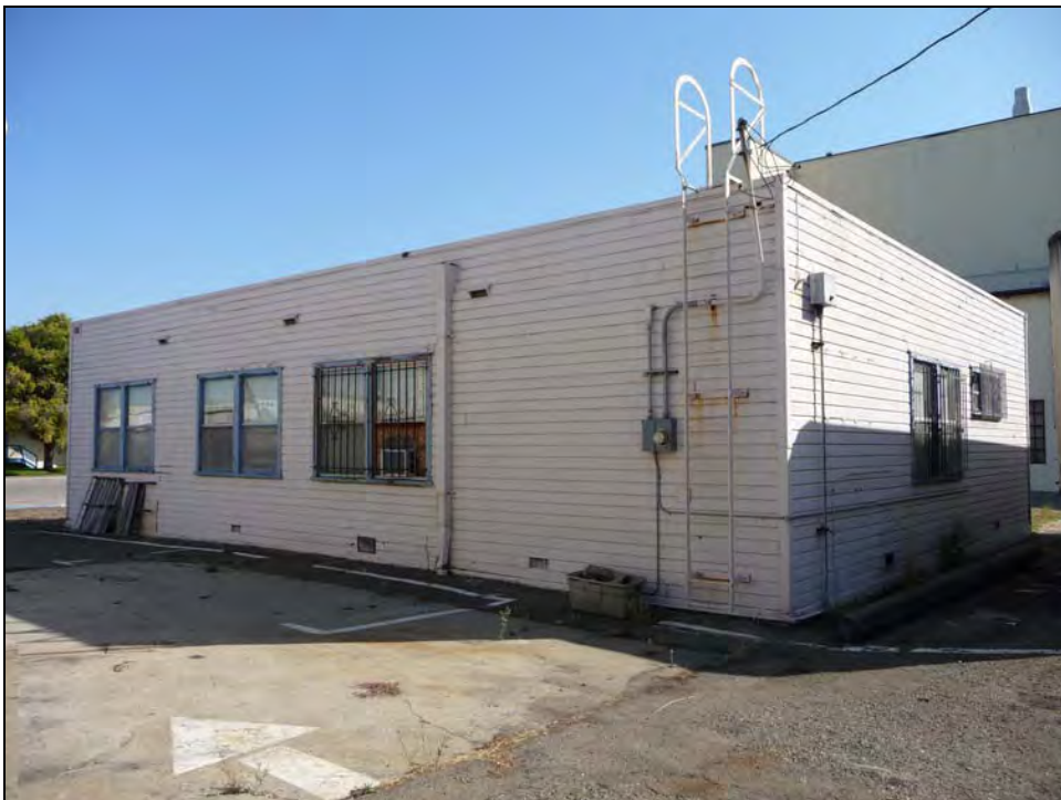
Photograph 2: Camera facing northeast, October 6, 2009.
