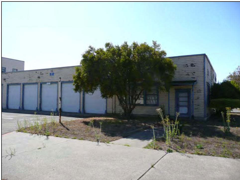
Photograph 2: East entrance detail, camera facing southwest, September 25, 2009.
