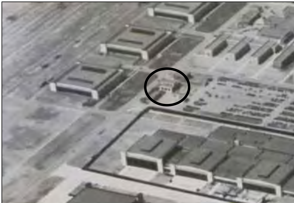
Photograph 6: First phase of Building 43 construction before addition to clerestory, June 1, 1942. 1
