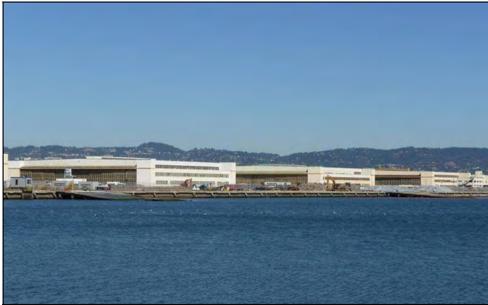
Photograph 53: Seaplane Hangars (Buildings 39, 40 and 41) with Seaplane Lagoon, October 1, 2009.
