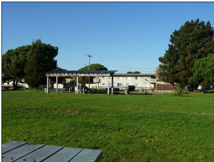
Photograph 2: Building FH-2127, camera facing northwest, November 3, 2009.
