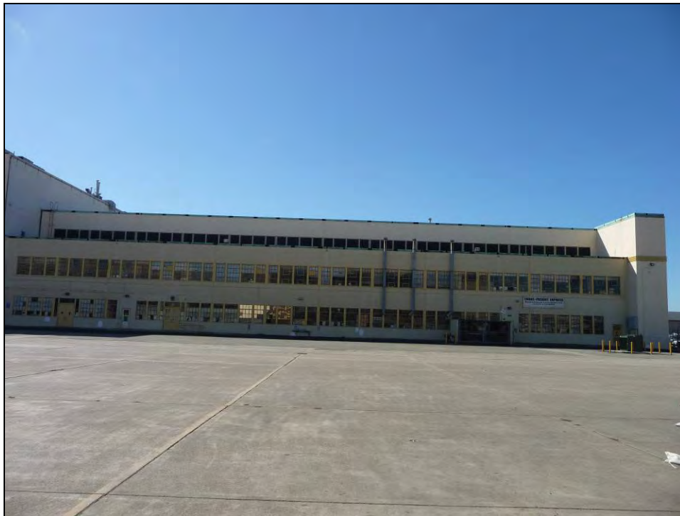
Photograph 3: Building 11, camera facing south, October 1, 2009.
