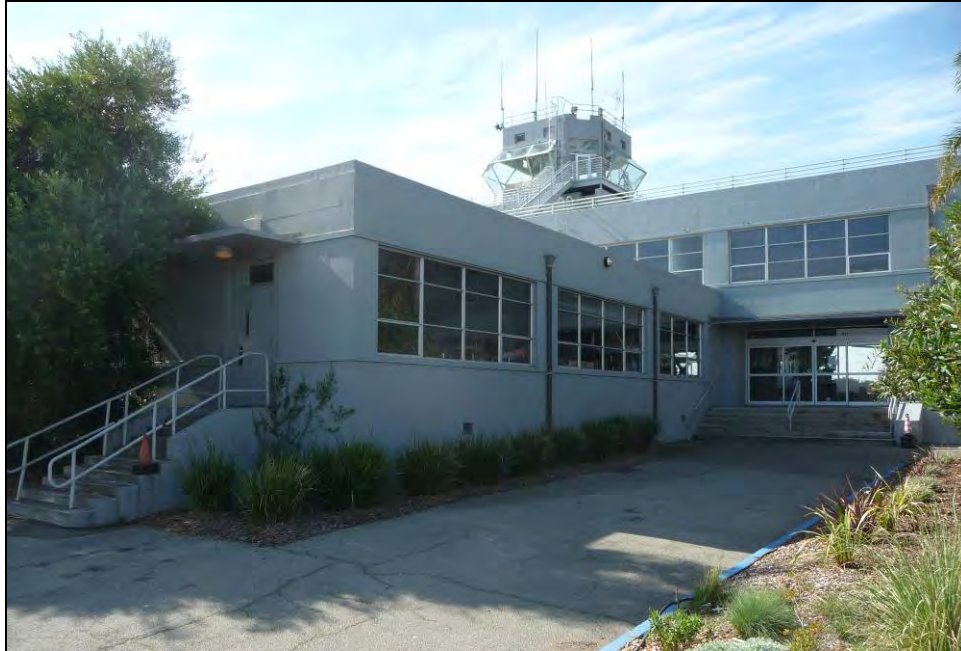
Photograph 5: Building 19, east-west wing and east entrance, camera facing southwest, November 3, 2010.
