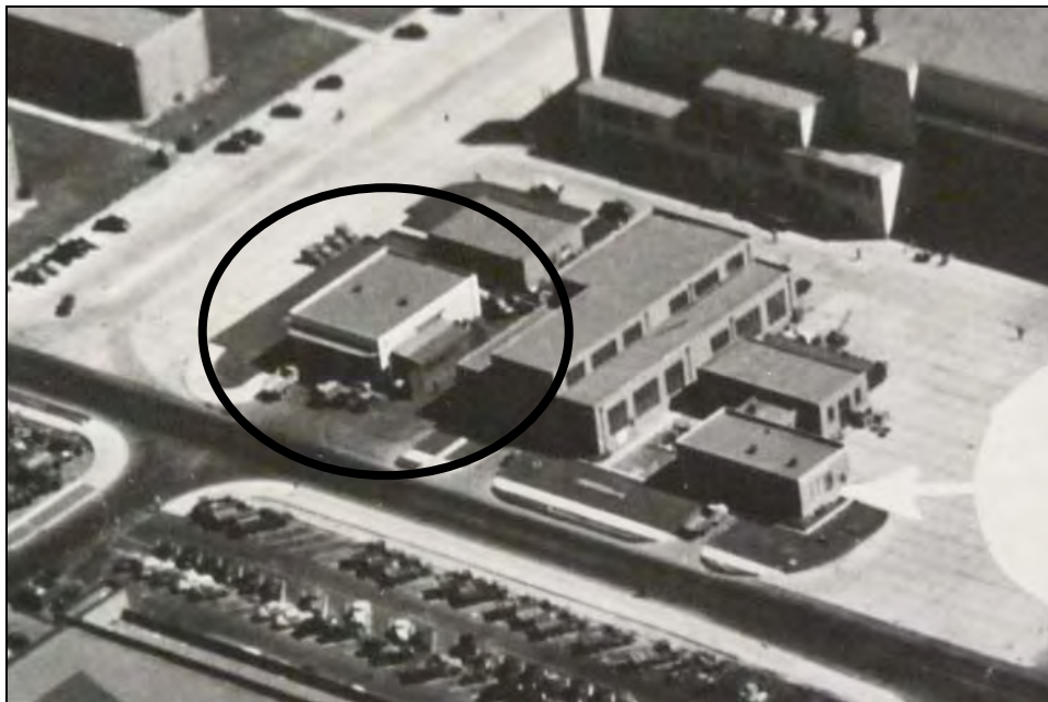
Photograph 6: September 1, 1945 photo, note shed roof on south side no longer present. 1
