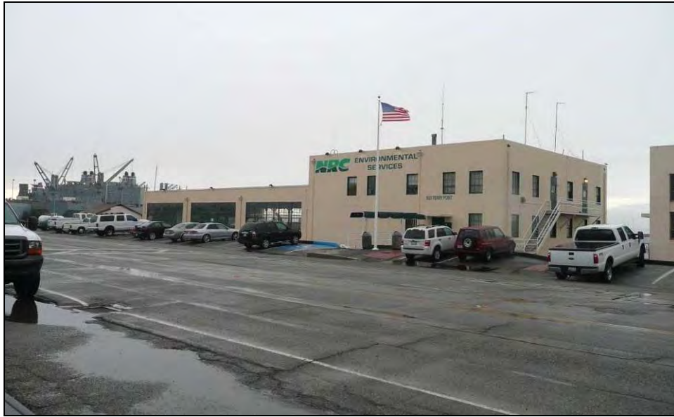
Photograph 50: Boathouse (Building 16), October 13, 2009.
