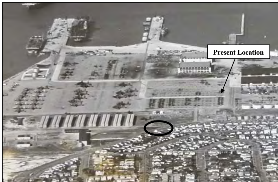
Photograph 5: Circa 1953 aerial photograph with original location of Building 351 circled, camera facing west. 7
