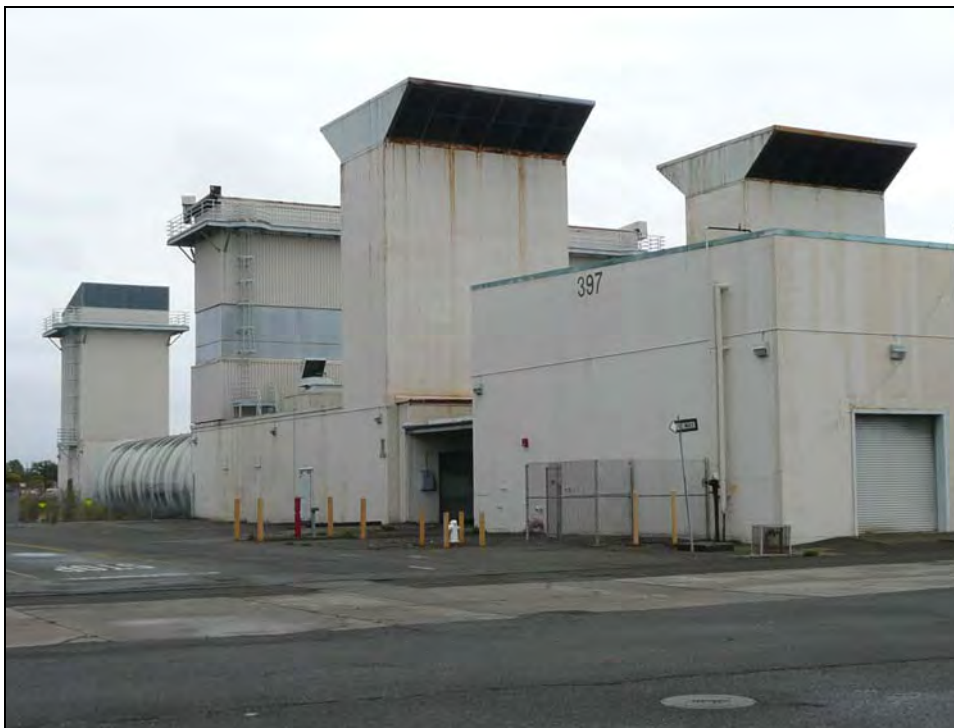
Photograph 2: North side, camera facing southeast, October 14, 2009.
