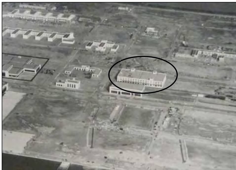
Photograph 4: 1941 photo of Building 8 first phase of construction, camera facing north. 1
