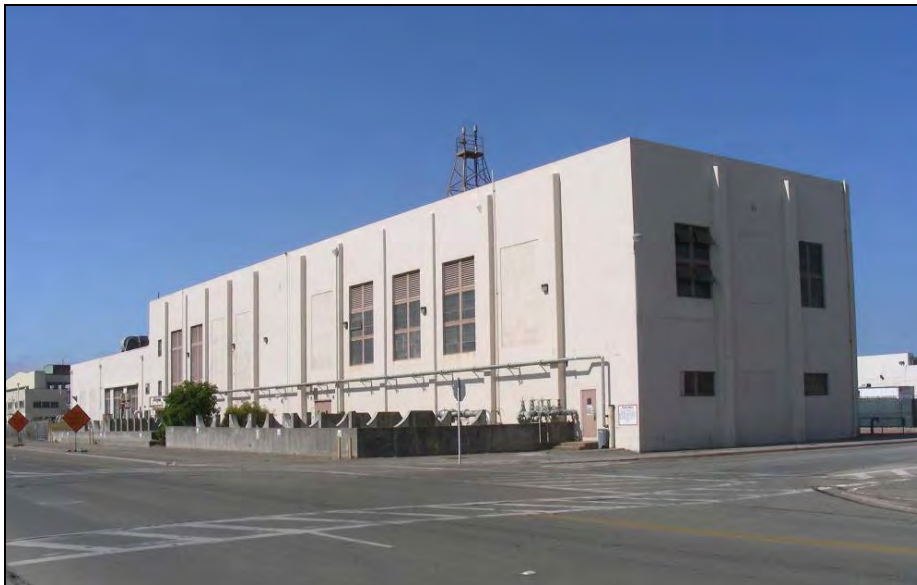
Photograph 46: Power Plant (Building 10), October 3, 2009.
