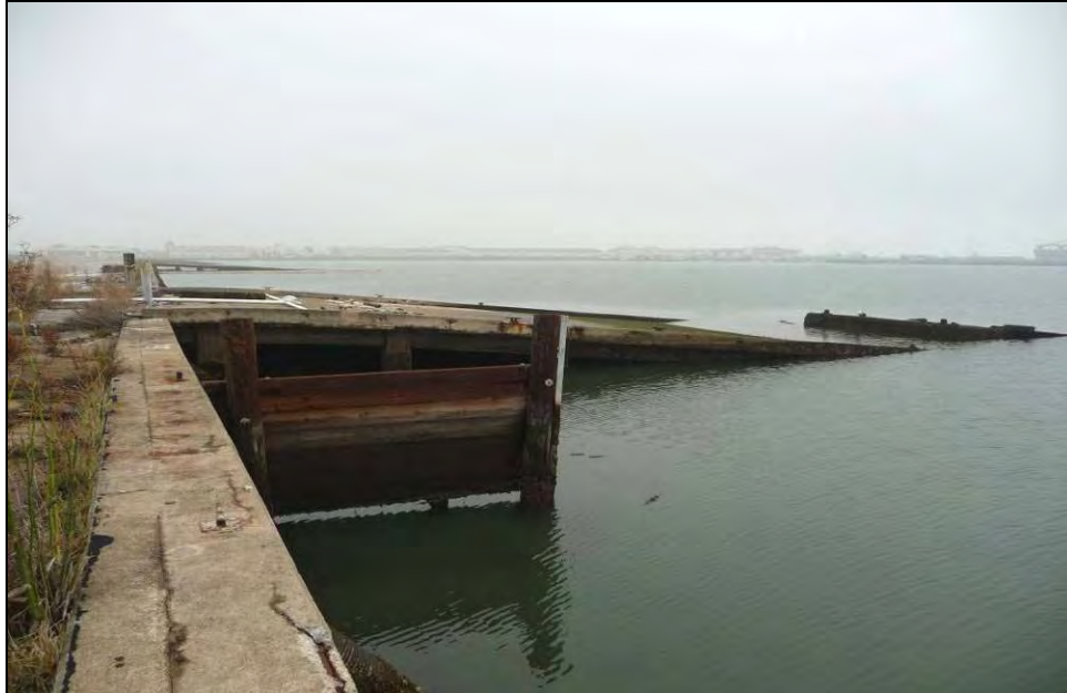
Photograph 8: Ramp 1, camera facing east, December 16, 2009.
