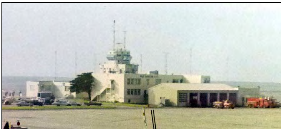
Photograph 9: Building 19 during 1960s, camera facing southwest. 12
