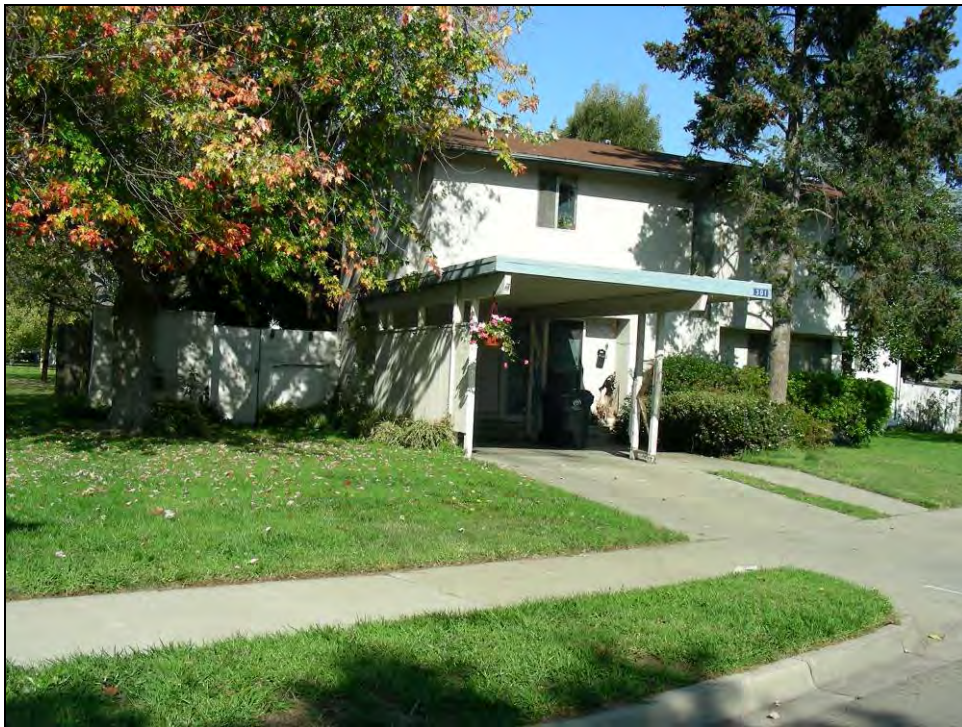
Photograph 9: Building FH-777, camera facing northeast, November 12, 2009.
