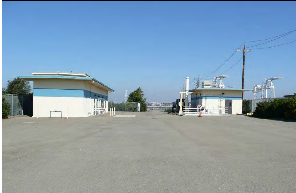
Photograph 4: Building 562, camera facing north, September 25, 2009.
