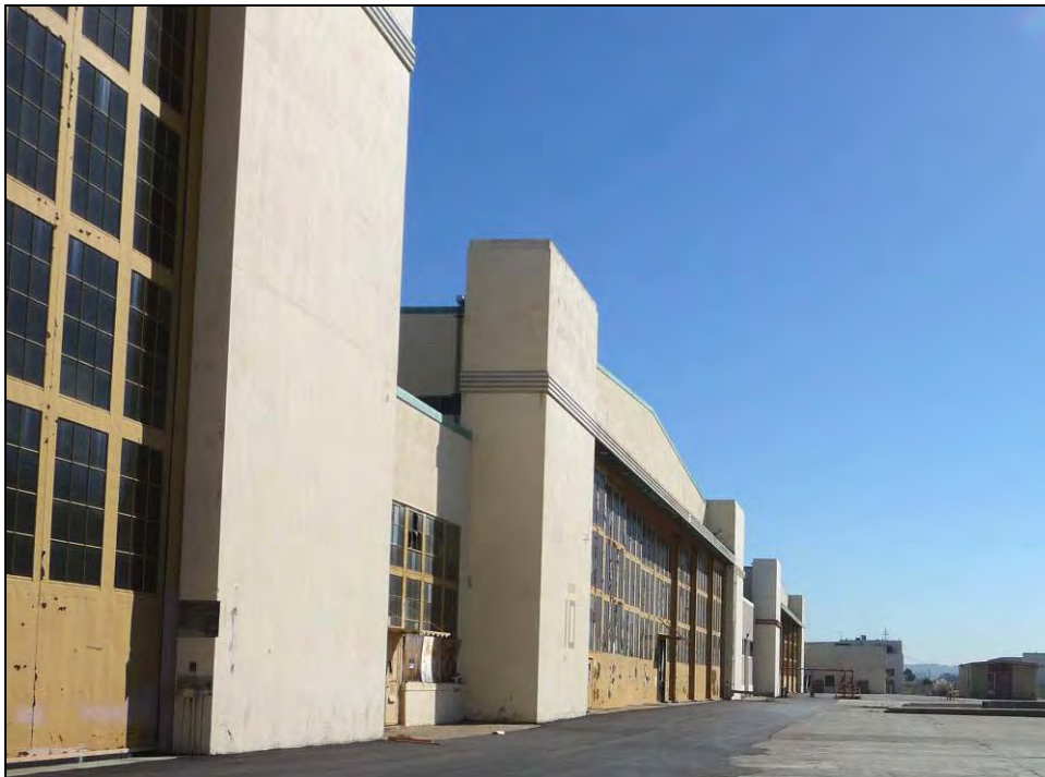
Photograph 10: South side of Building 5 (Door 10), camera facing northeast, October 1, 2009.
