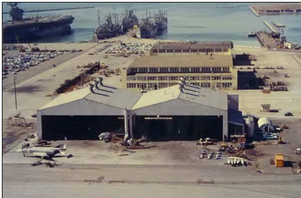
Photograph 6: Circa 1960s oblique aerial photograph of Building 410, camera facing west. 8
