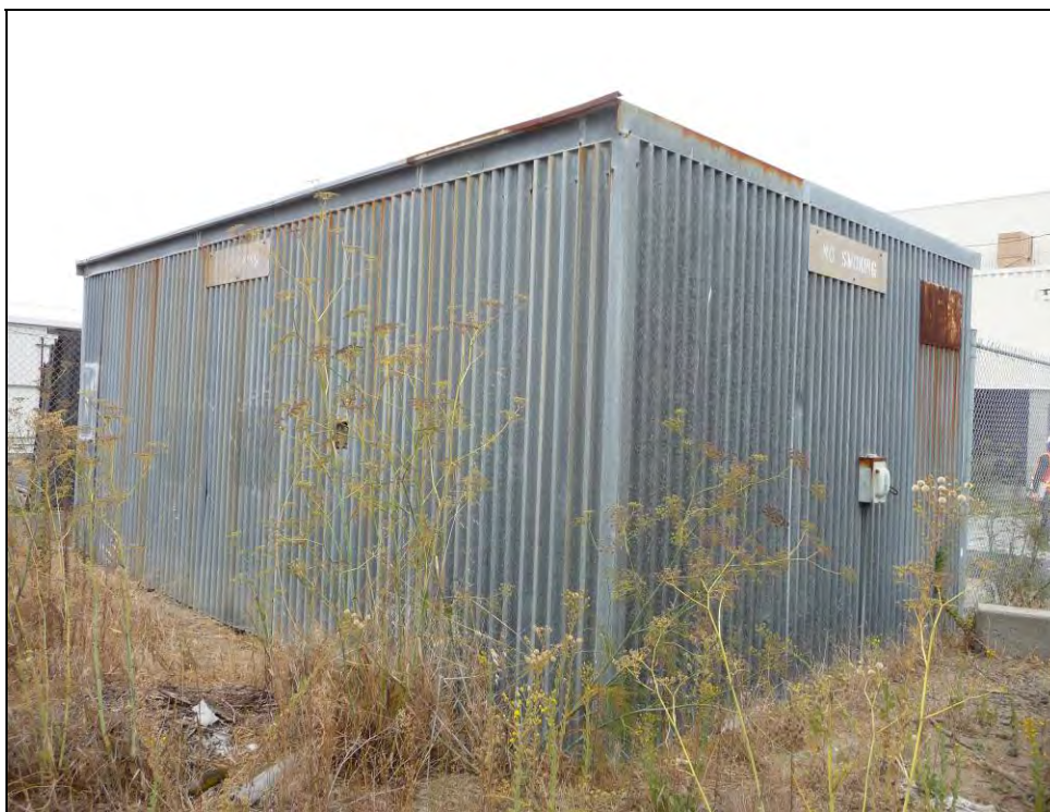
Photograph 2: Camera facing northwest, October 8, 2009.
