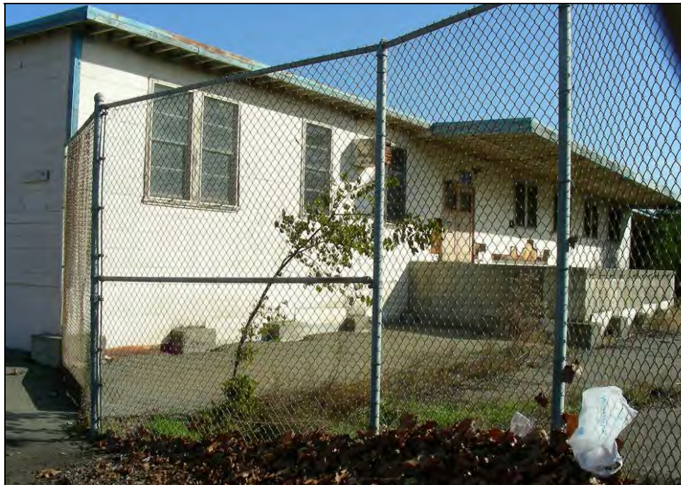
Photograph 9: West end of south side, camera facing northeast, November 12, 2009.
