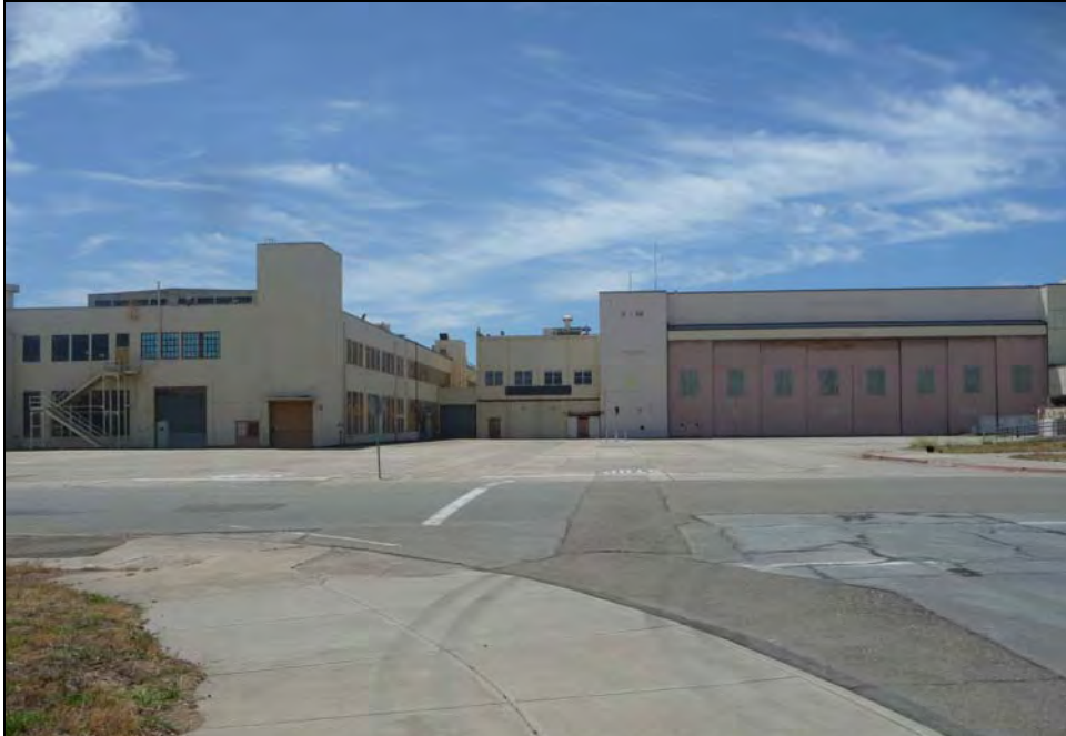
Photograph 5: East side of Building 5, left to right- Northeast Extension, Mezzanine, Door 5A camera facing west, June 9, 2010.
