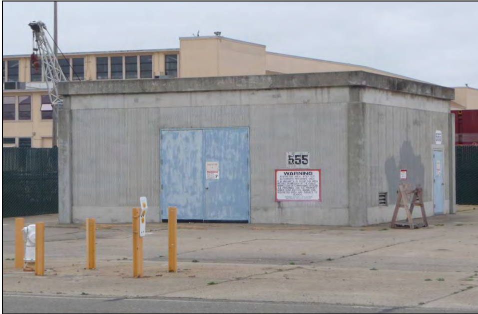
Photograph 4: Building 555, camera facing northwest, October 9, 2009.
