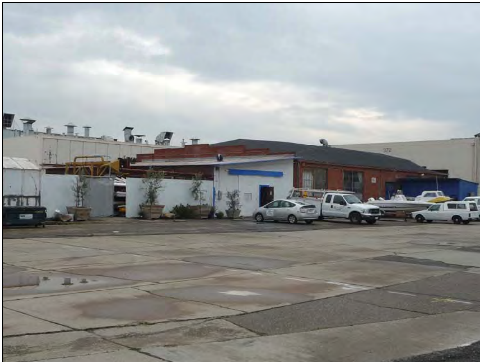
Photograph 2: Camera facing southeast, December 16, 2009.
