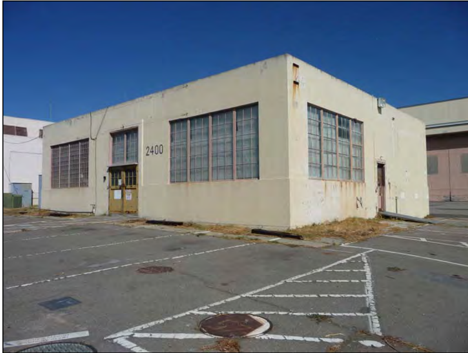
Photograph 1: Camera facing northeast, October 1, 2009.
