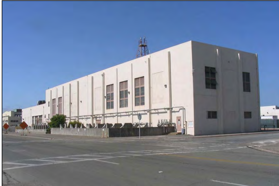
Photograph 1: Building 10, camera facing northwest, October 8, 2009.
