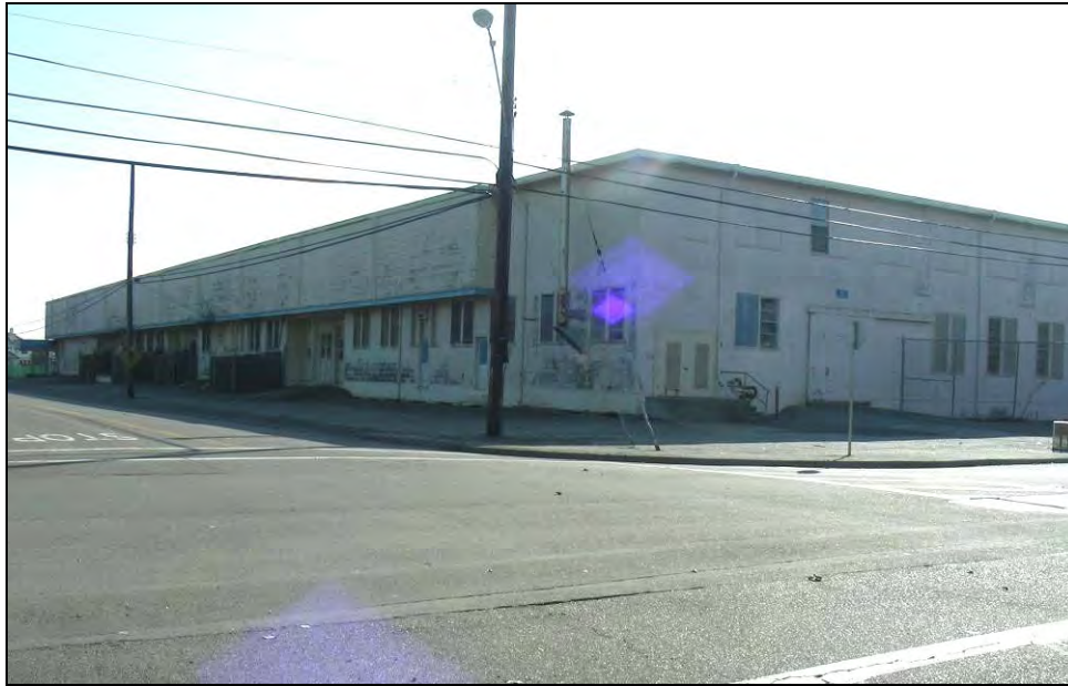
Photograph 12: Northwest corner, camera facing northeast, November 12, 2009.
