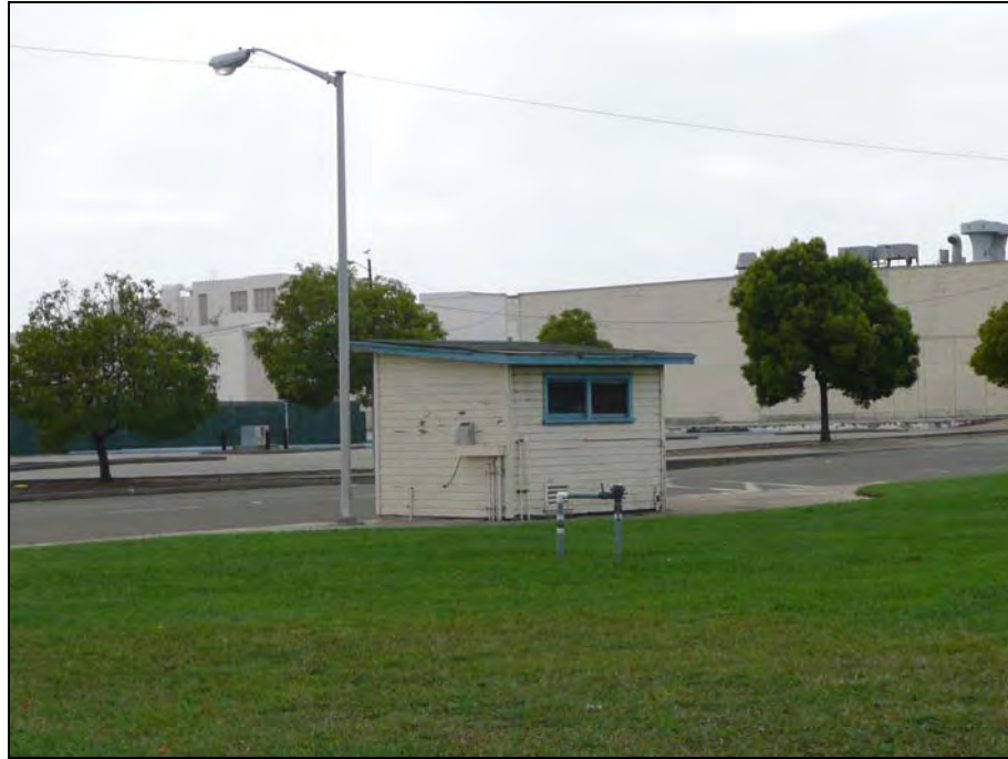
Photograph 2: Camera facing southwest, October 14, 2009.
