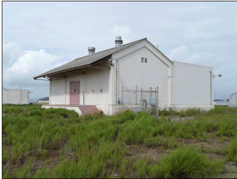
Photograph 2: Building 26, camera facing west, October 13, 2009.
