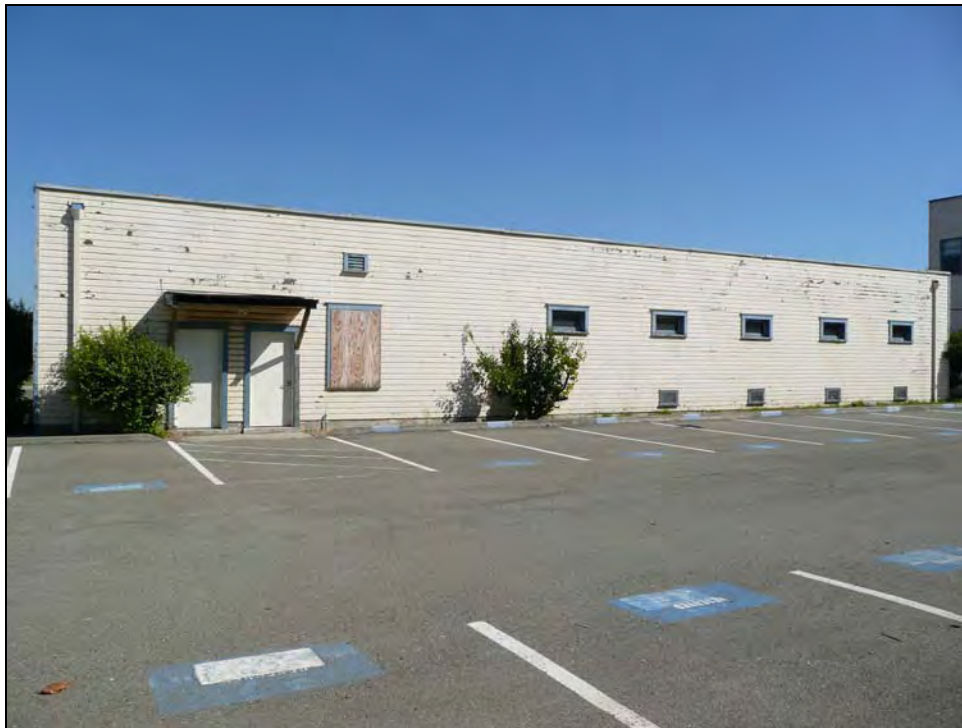
Photograph 4: West side, camera facing southeast, September 25, 2009.
