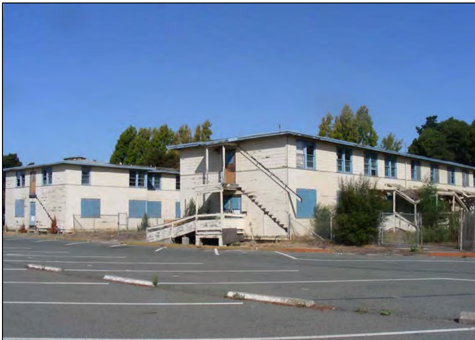
Photograph 4: Building 135, west wing (left) and central wing (right), facing northwest, October 6, 2009.
