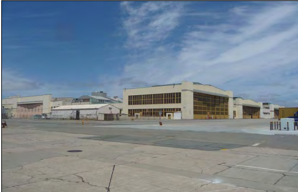
Photograph 1: Southwest corner of Building 5, camera facing northeast, June 9, 2010. Left foreground includes Building 405.
