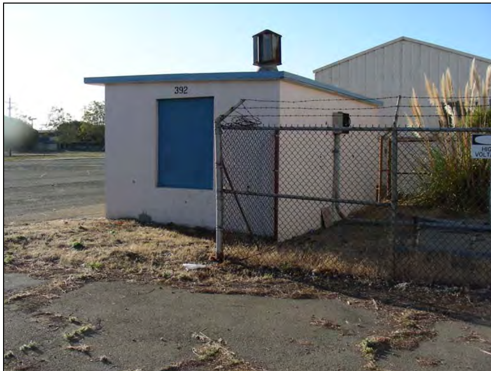
Photograph 2: Camera facing southeast, October 7, 2009.
