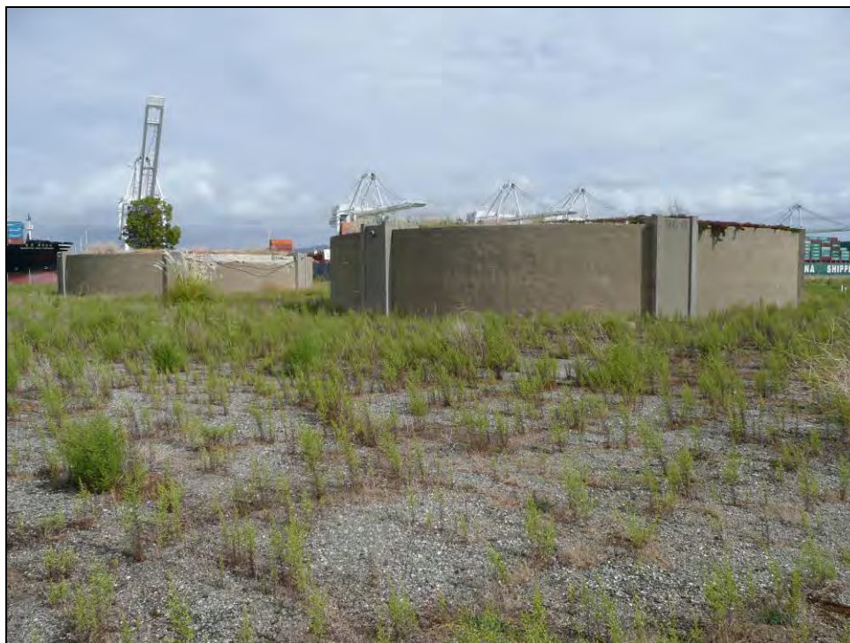
Photograph 4: Building 96A in background and 96B in foreground, camera facing north, October 14, 2009.
