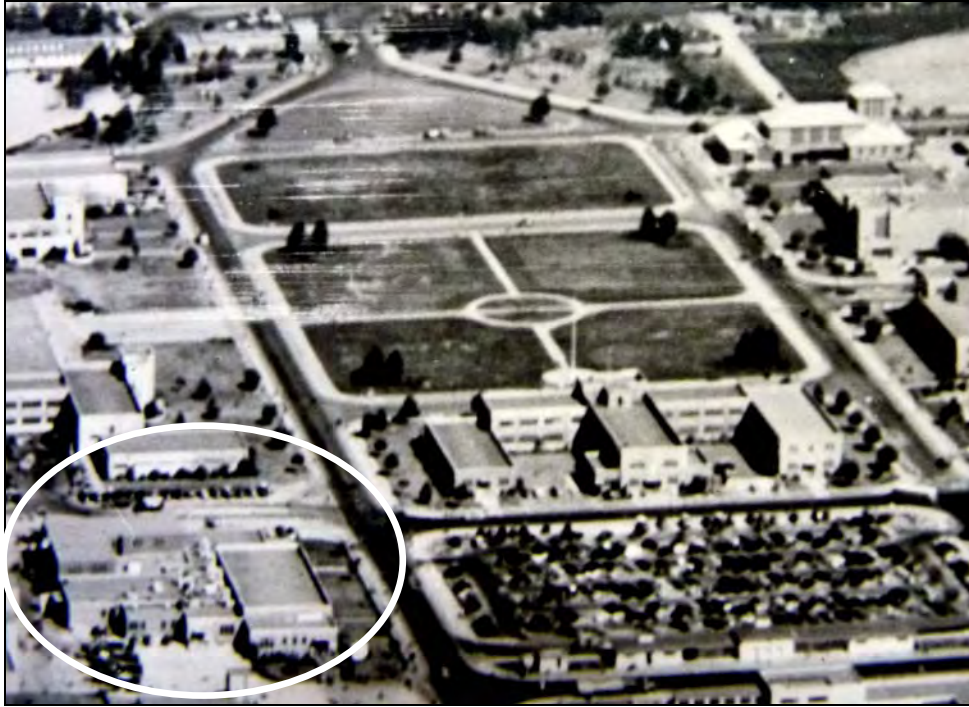
Photograph 10: Lower left corner, Building 62 after addition on northwest corner, September 1, 1945. 3
