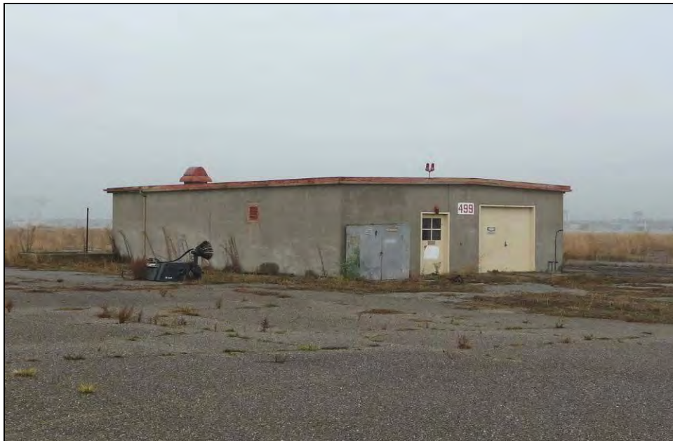
Photograph 27: Field Lighting Vault (Building 499), camera facing north, December 16, 2009.
