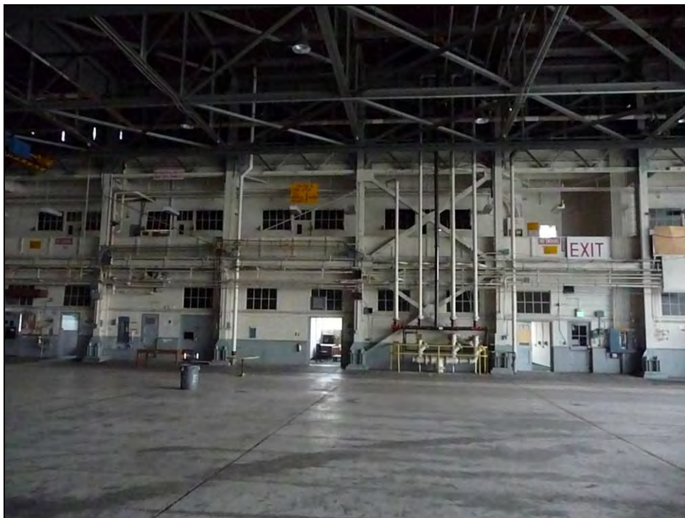
Photograph 8: Interior of Building 12, camera facing north, December 11, 2009.
