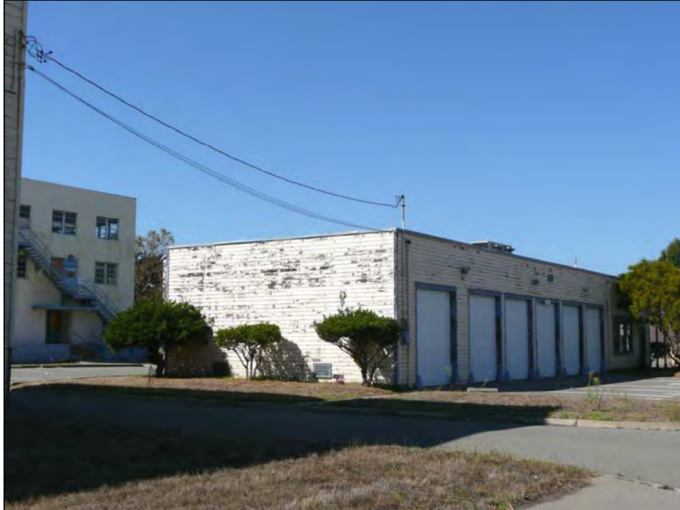
Photograph 1: Southeast corner, camera facing northwest, September 25, 2009.
