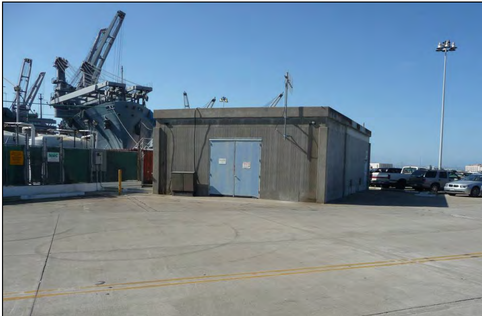
Photograph 5: Building 558, camera facing northwest, September 30, 2009.
