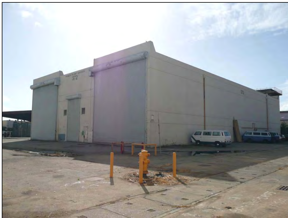
Photograph 2: Northeast corner, camera facing southwest, October 14, 2009.
