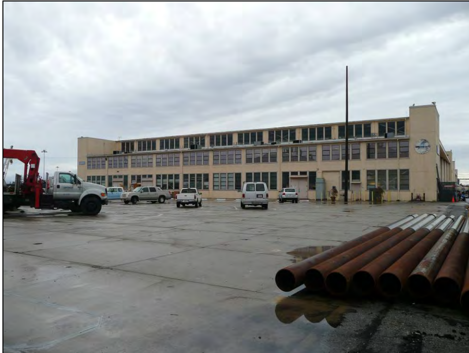
Photograph 2: Building 166, camera facing west, October 13, 2009.
