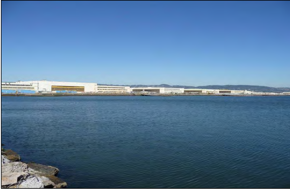
Photograph 4: Seaplane Lagoon, northern edge, Seaplane Hangars in background, Ramps 1, 2, and 3 at water level, camera facing northeast, October 1, 2009.
