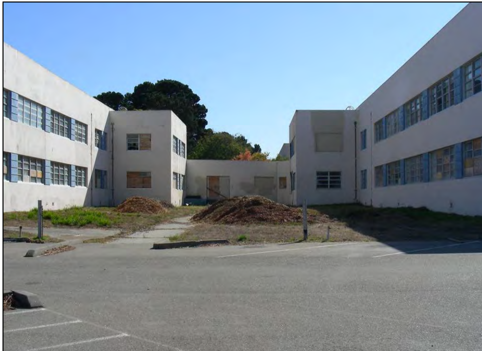
Photograph 6: Gap between Wings 13 and 14, Building 4, camera facing south, October 7, 2009.
