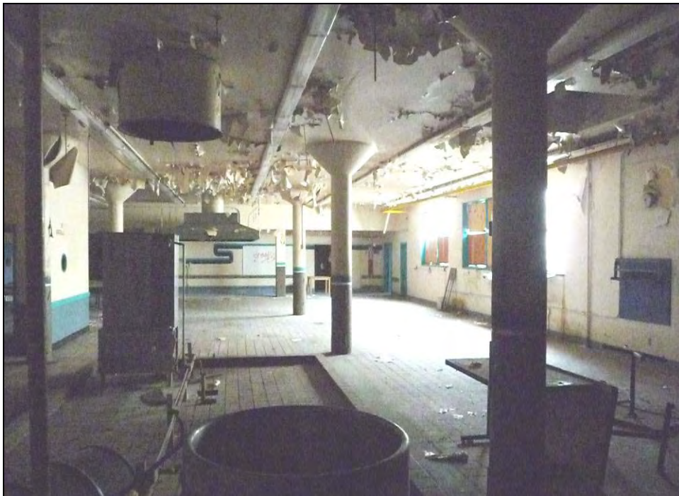
Photograph 10: Building 3 kitchen, camera facing south, December 11, 2009.
