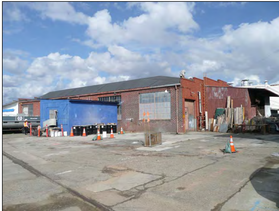
Photograph 4: Additions on south and west walls, camera facing northeast, October 14, 2009.
