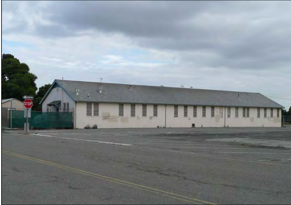
Photograph 1: Camera facing southeast, October 14, 2009.
