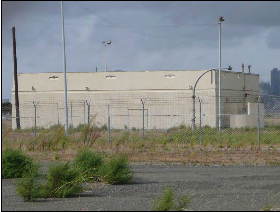
Photograph 12: East and north sides, camera facing southwest, October 14, 2009.
