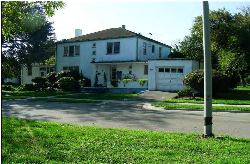
Photograph 2: Typical ‘long porch’ plan (Senior Officer’s) building FH-F, camera facing southwest, November 12, 2009.
