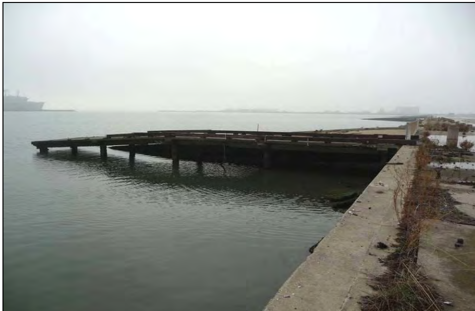
Photograph 13: Remains of Dock 4 adjoining Ramp 4, camera facing southwest, December 16, 2009.
