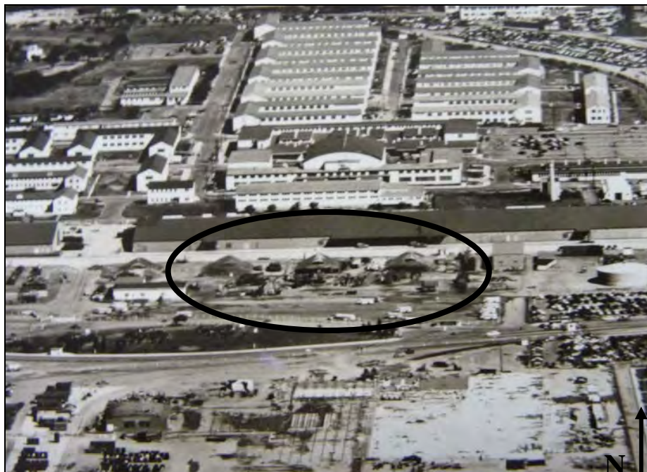
Photograph 3: Circa 1953 photo of Buildings 120-122 from left to right south of Building 118. 4
