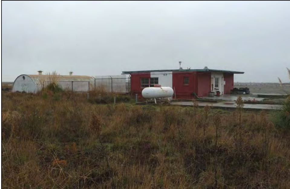
Photograph 26: Liquid Oxygen Facility (Building 407) (center), camera facing south, December 16, 2009.
