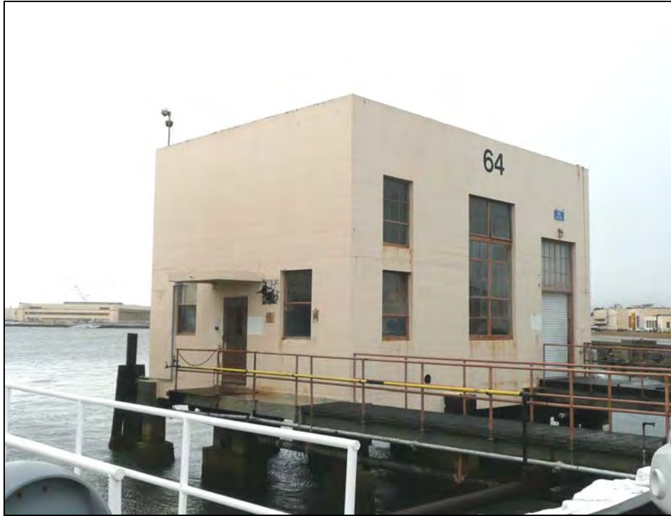
Photograph 1: Camera facing northwest, October 13, 2009.
