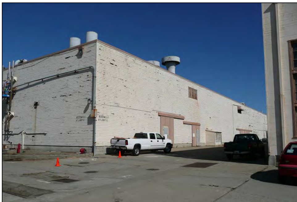
Photograph 10: South wall at southwest corner, camera facing northeast, October 15, 2009.
