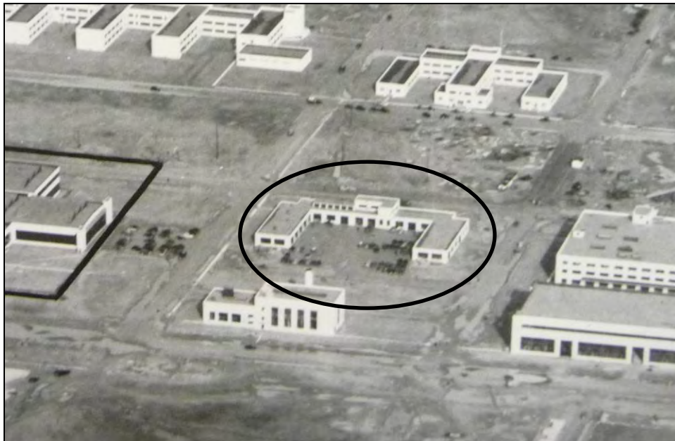
Photograph 9: Oblique aerial view of Building 6-Building 7, January 1, 1941.
