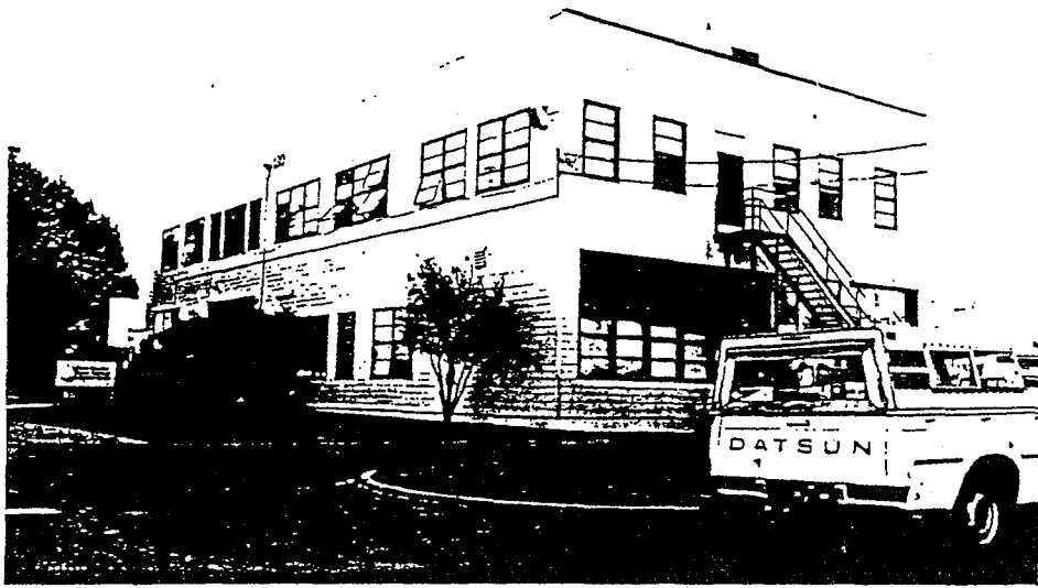
NAS ALAMEDA Building 130
