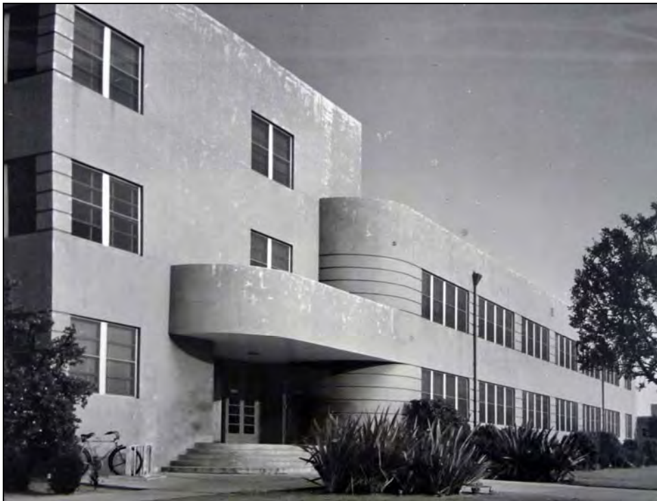
Photograph 12: Building 16, photo dated 1945. 57
