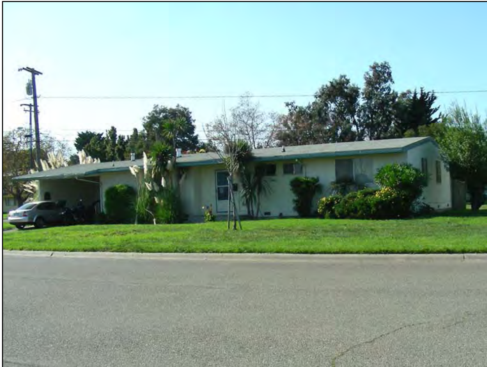
Photograph 4: Typical Plan M view, FH-768, camera facing west, November 12, 2009.
