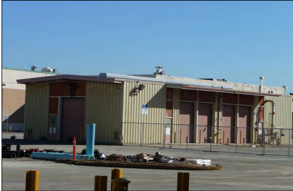
Photograph 2: Building 615, camera facing southwest, October 1, 2009.
