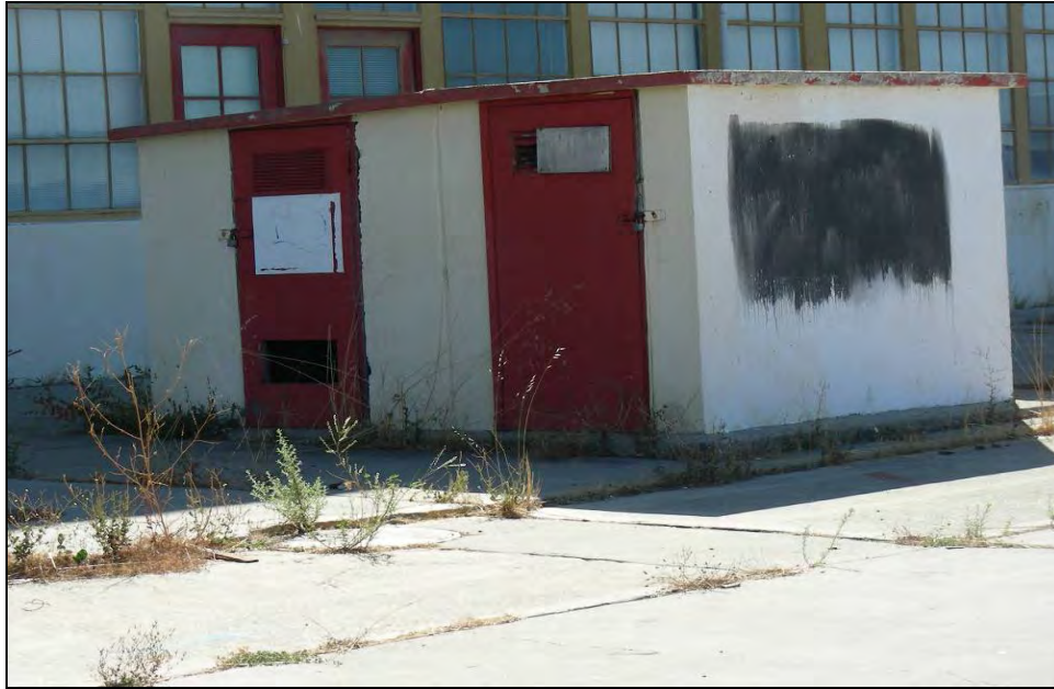
Photograph 5: Building 321, camera facing southeast, September 30, 2009.
