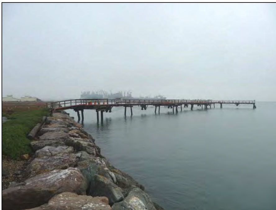
Photograph 2: Building 512 with lighting, camera facing east, December 16, 2009.
