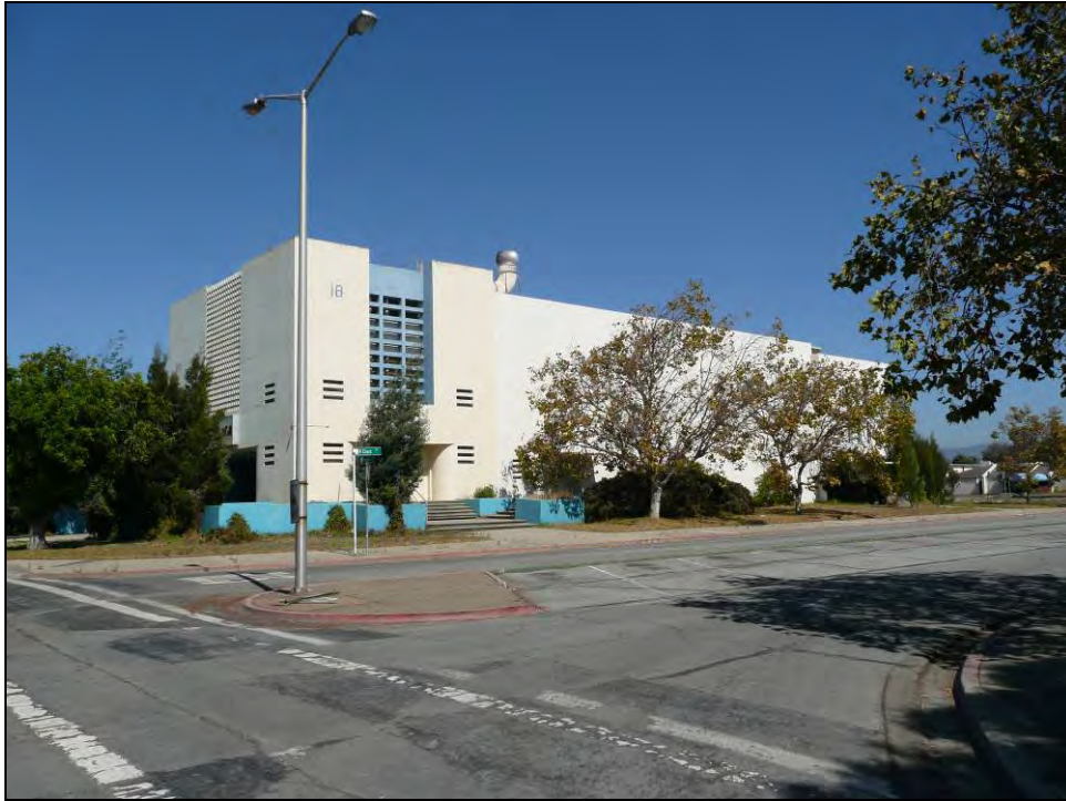
Photograph 1: Building No. 18, camera facing northeast, September 25, 2009.
