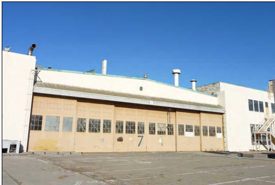
Photograph 12: Door 7 on east side of Building 5, camera facing northwest, October 1, 2009.
