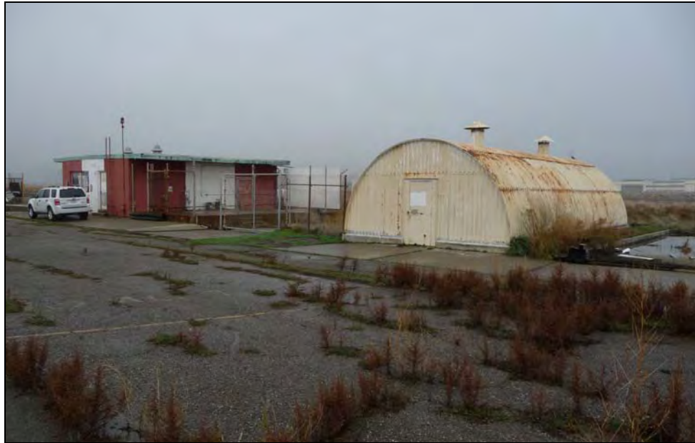
Photograph 4: Building 272, camera facing northeast, October 8, 2009.
