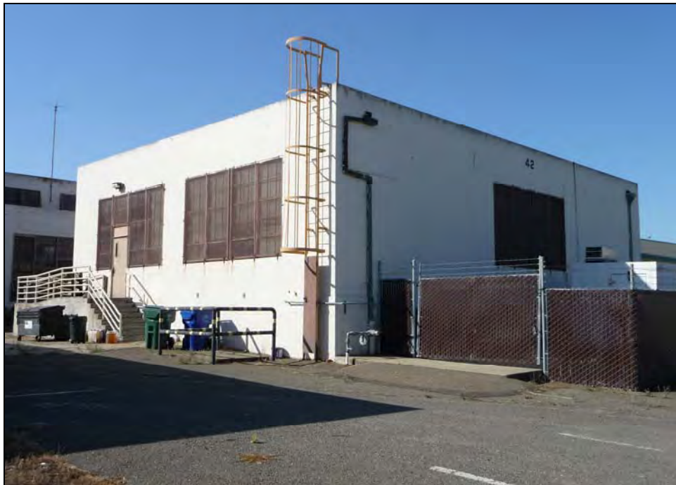
Photograph 5: Northwest corner, camera facing southwest, October 6, 2009.
