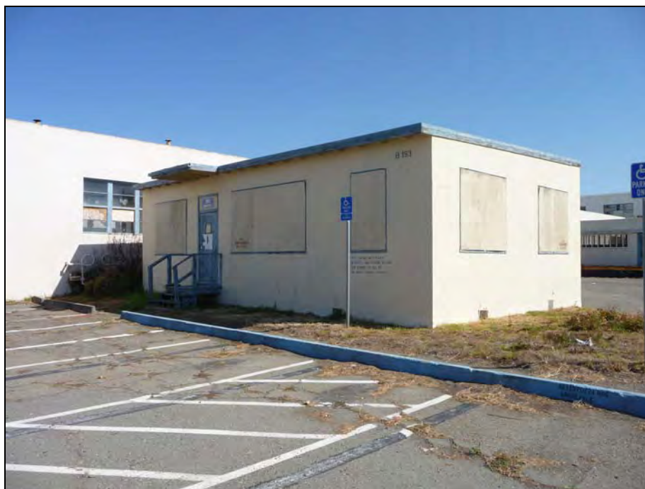
Photograph 1: Camera facing northeast, October 6, 2009.
