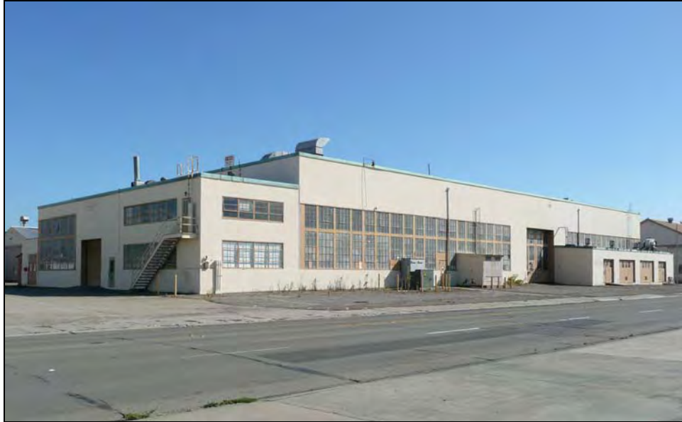
Photograph 1: Building 66, camera facing southeast, October 15, 2009.
