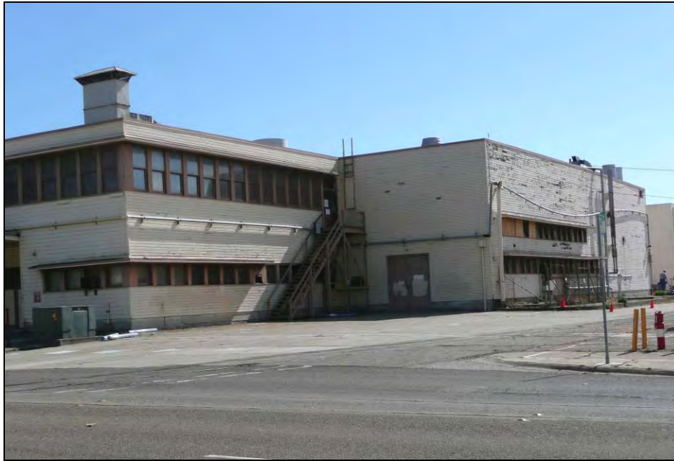
Photograph 2: Bump out on west side, camera facing southeast, October 15, 2009.
