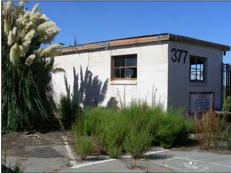
Photograph 12: Building 377, camera facing northwest, September 30, 2009.
