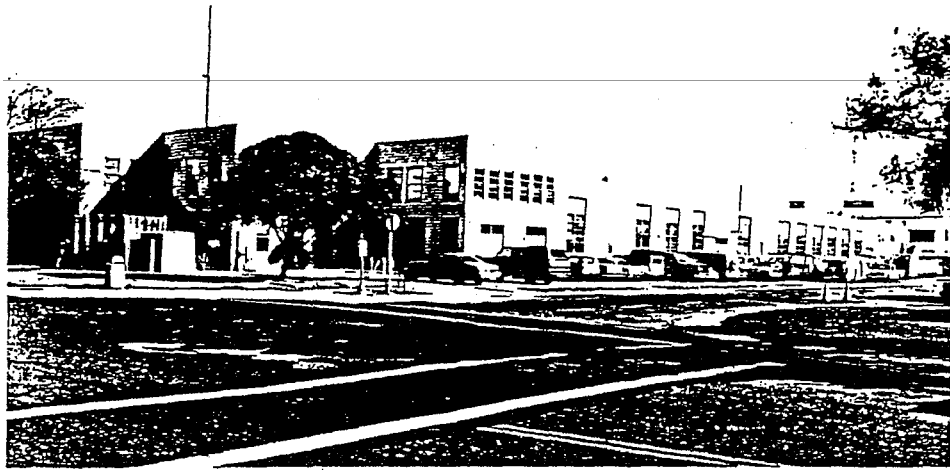
NAS PALM BEACH Building 114
