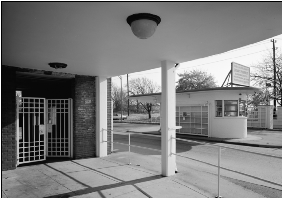
Photograph 19: Buildings 10 and 850, NAS Quonset Point, RI, 1979. 68
