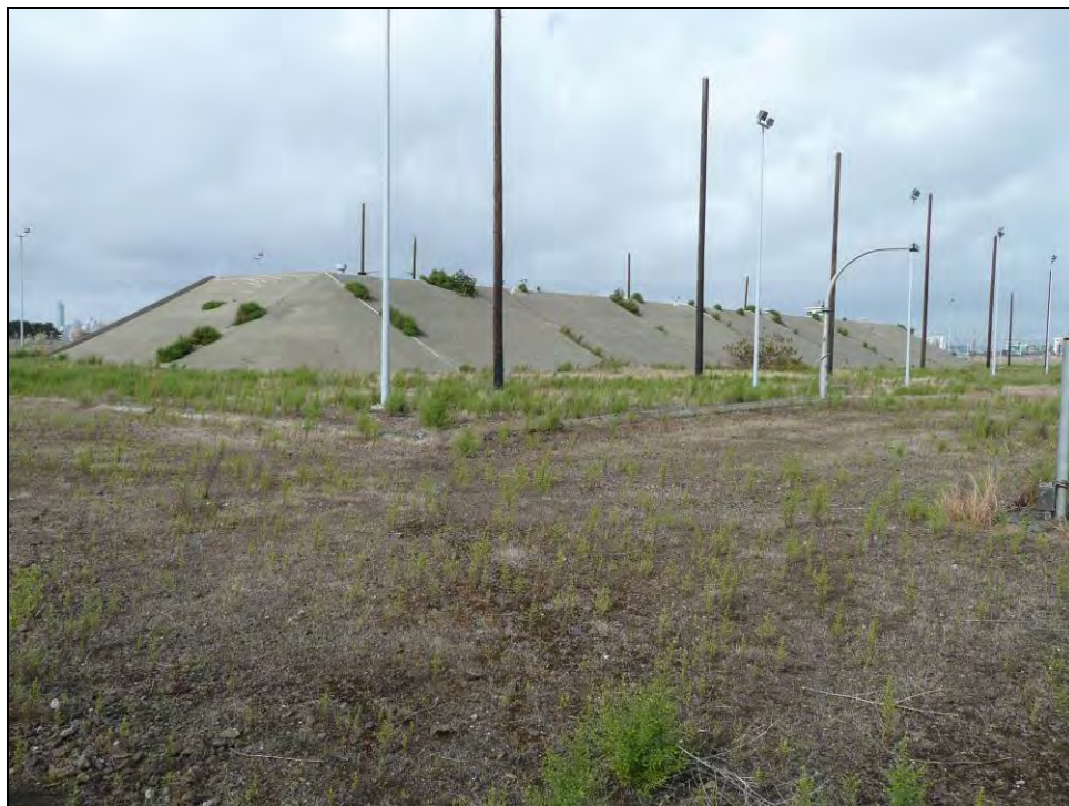
Photograph 9: Building 497, camera facing northwest, October 14, 2009.
