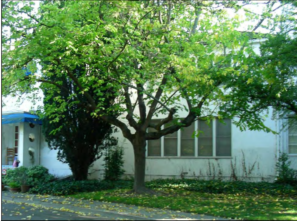
Photograph 3: Main house west section, camera facing south, November 12, 2009.
