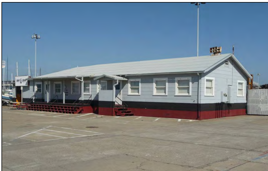
Photograph 47: Public Works Riggers (Building 292), October 8, 2009.
