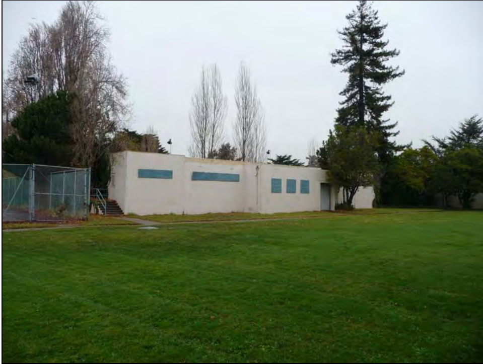
Photograph 1: Building 75, camera facing northeast, December 11, 2009.
