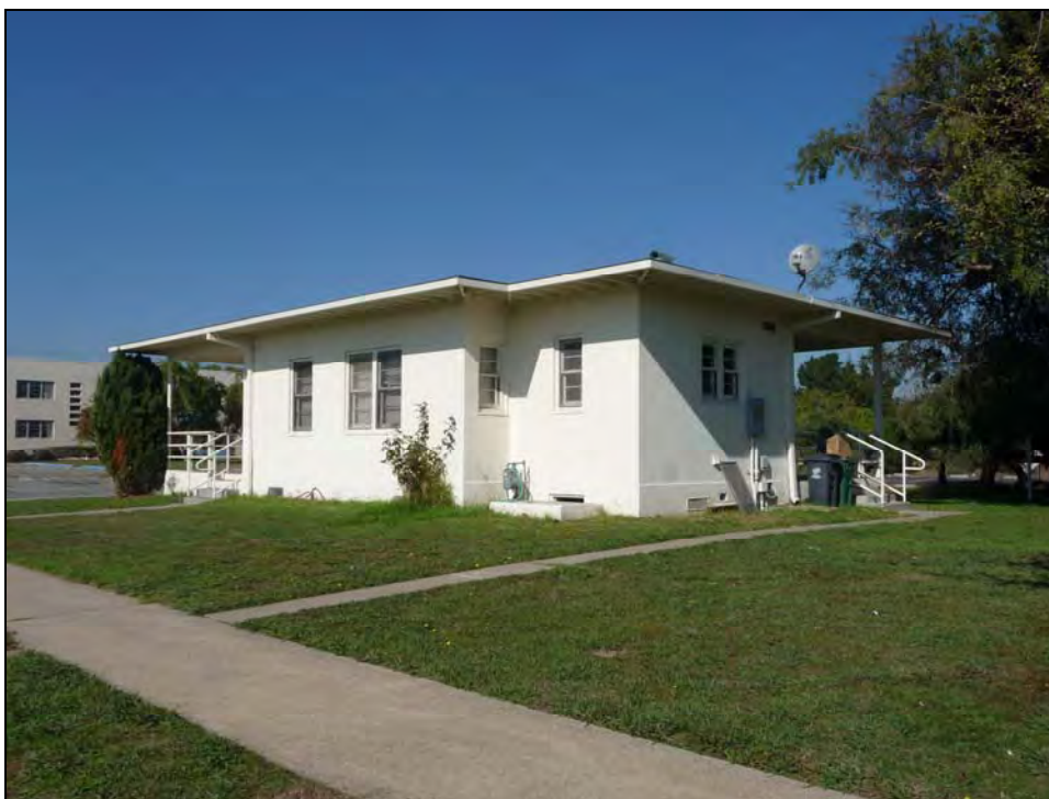
Photograph 1: CPO-1, 101 Corpus Christie Road, camera facing northeast.
