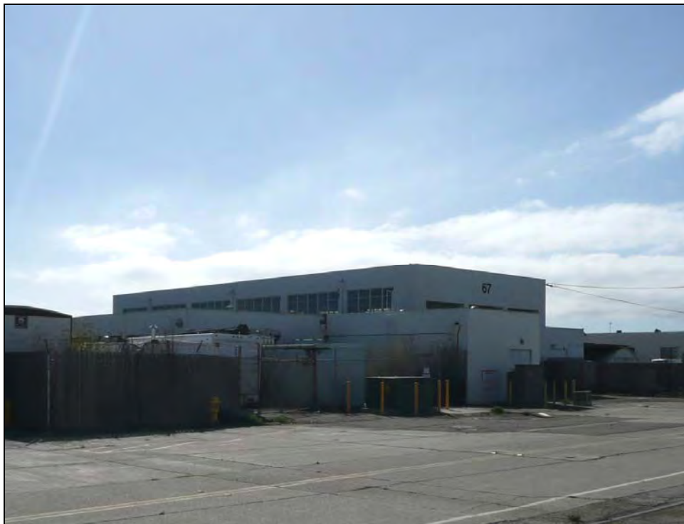
Photograph 4: Camera facing southwest, October 15, 2009.
