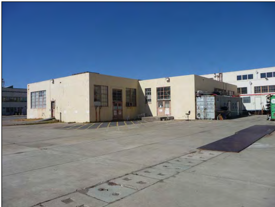
Photograph 2: Camera facing northwest, October 1, 2009.
