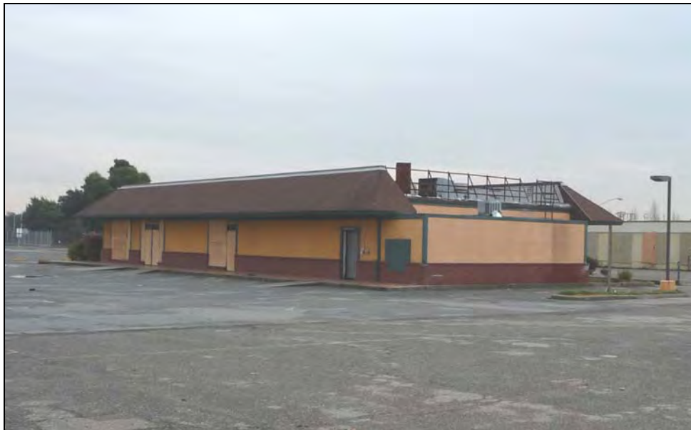
Photograph 2: Camera facing southeast, December 16, 2009.
