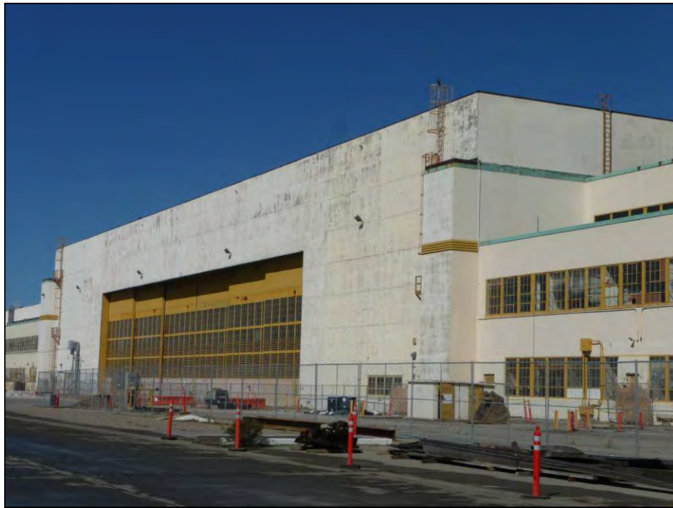
Photograph 5: Building 400, camera facing northwest, October 1, 2009.
