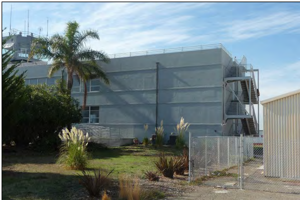
Photograph 6: Building 19, north end of east side, camera facing west, November 3, 2010.
