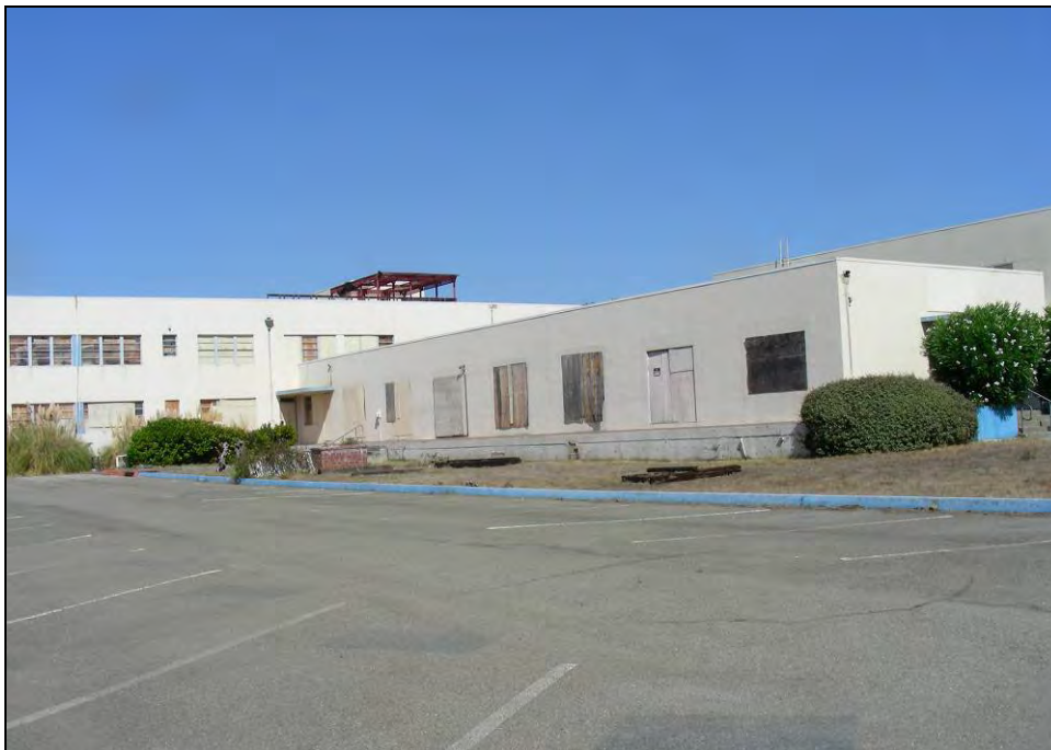
Photograph 6: One story portion of south facing block, camera facing northeast, October 6, 2009.
