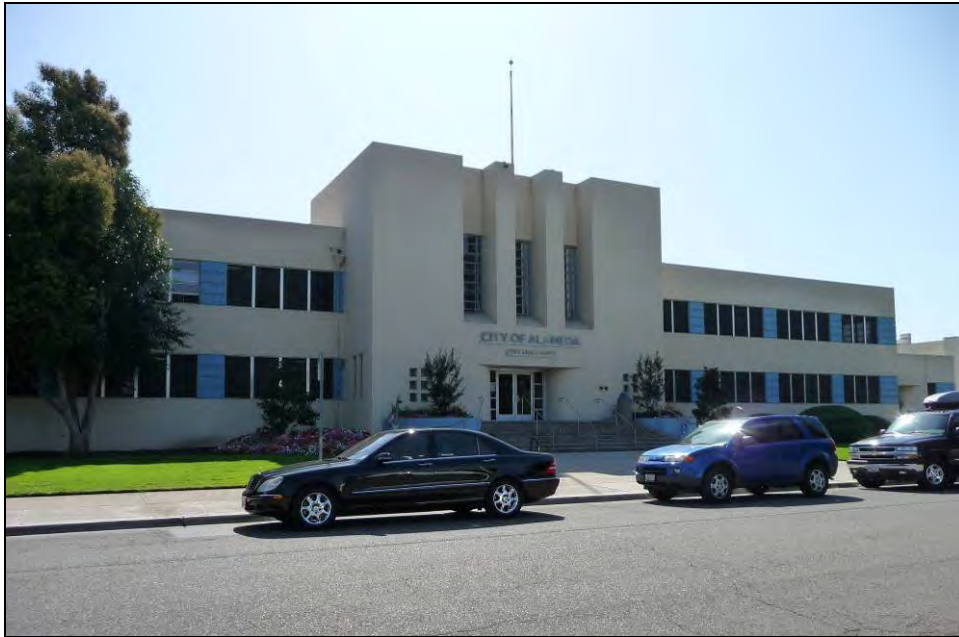
Photograph 2: Building 1, main entrance tower, camera facing southwest, October 6, 2009.
