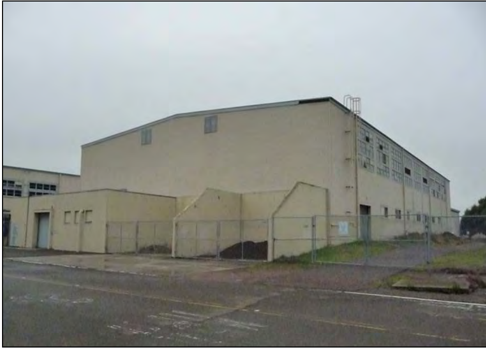
Photograph 2: Building 76 northeast corner, facing southwest, December 11, 2009.
