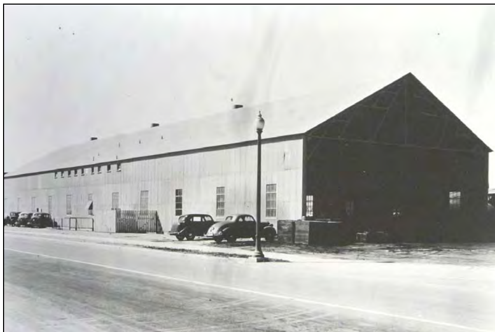
Photograph 3: Circa 1943 west side view of Building 113. 5
