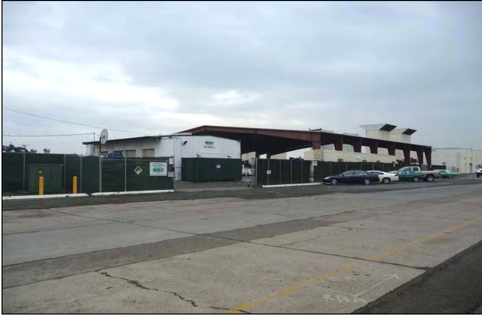
Photograph 4: Building D-13, camera facing southeast, December 16, 2009.
