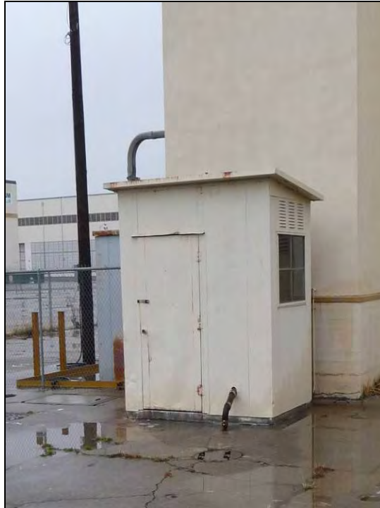
Photograph 12: Building 501, camera facing northwest, December 16, 2009.
