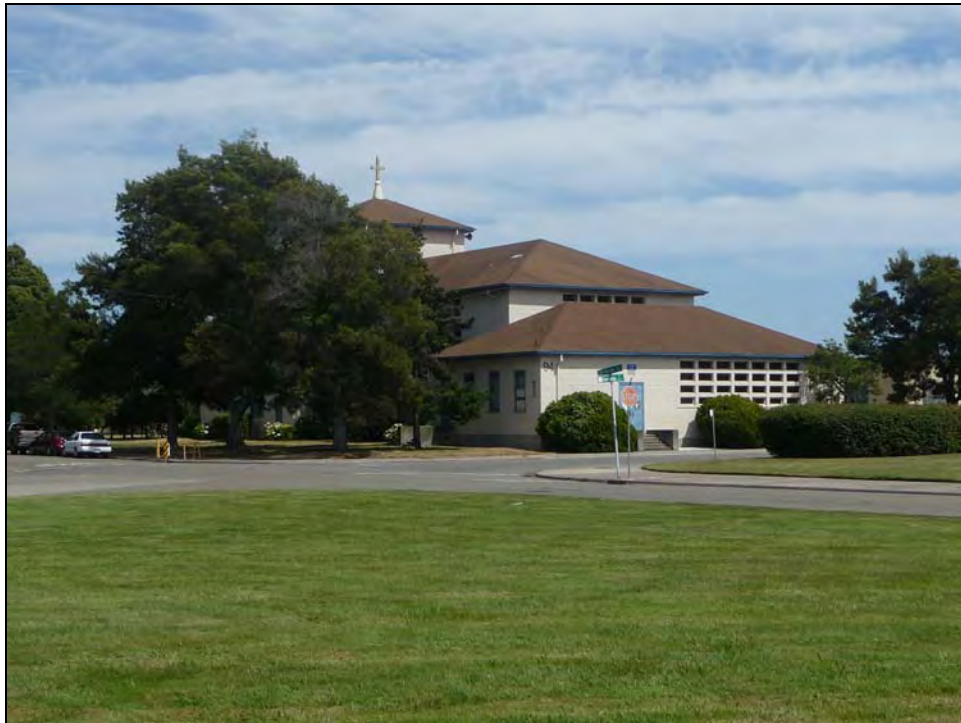
Photograph 3: Camera facing southeast, June 9, 2010.
