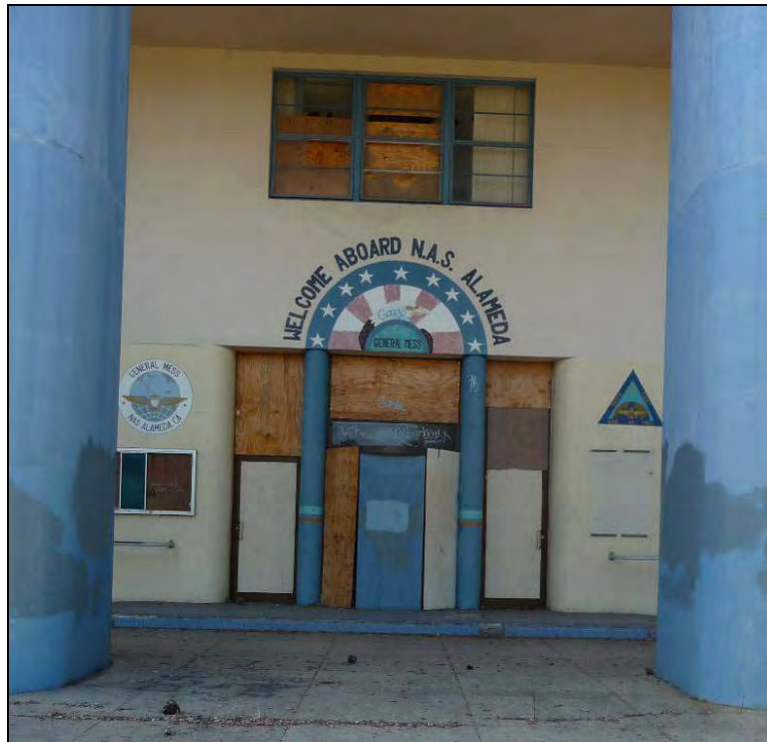
Photograph 2: Detail of Mess Hall entrance, camera facing west, October 6, 2009.
