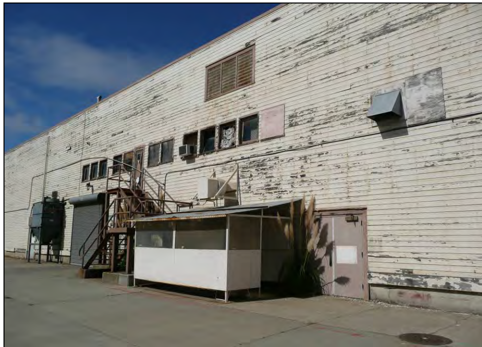
Photograph 9: South wall detail, camera facing northwest, October 15, 2009.
