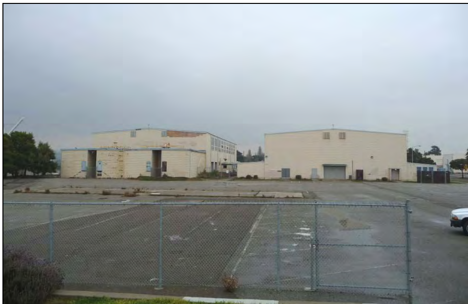
Photograph 44: Enlisted Men's Pool (Building 76) and Gymnasium (Building 134), December 16, 2009.
