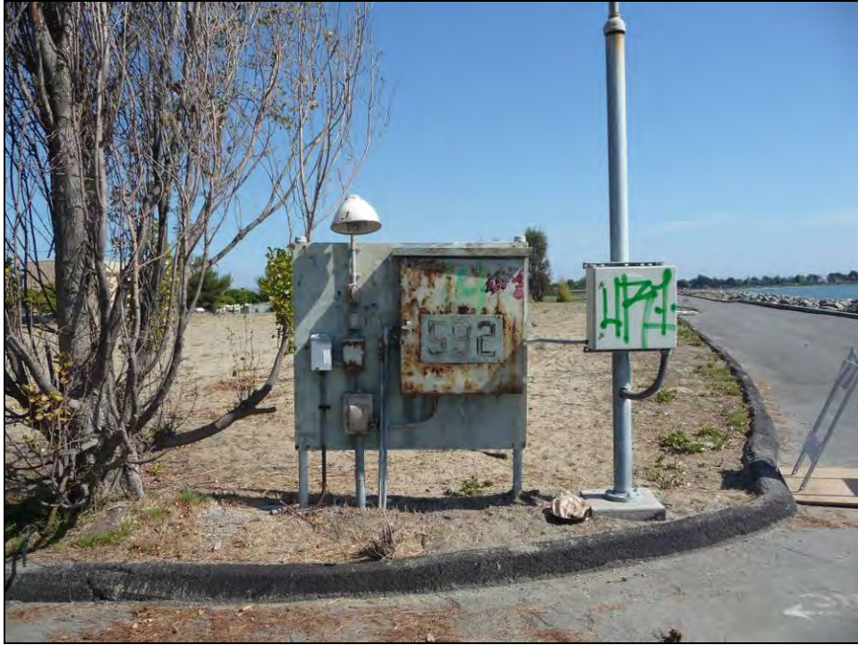
Photograph 14: Building 592, camera facing east, October 8, 2009.
