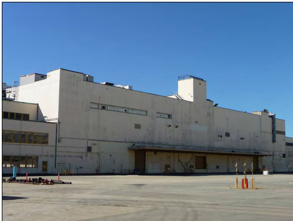
Photograph 6: Building 400, camera facing southwest, October 1, 2009.
