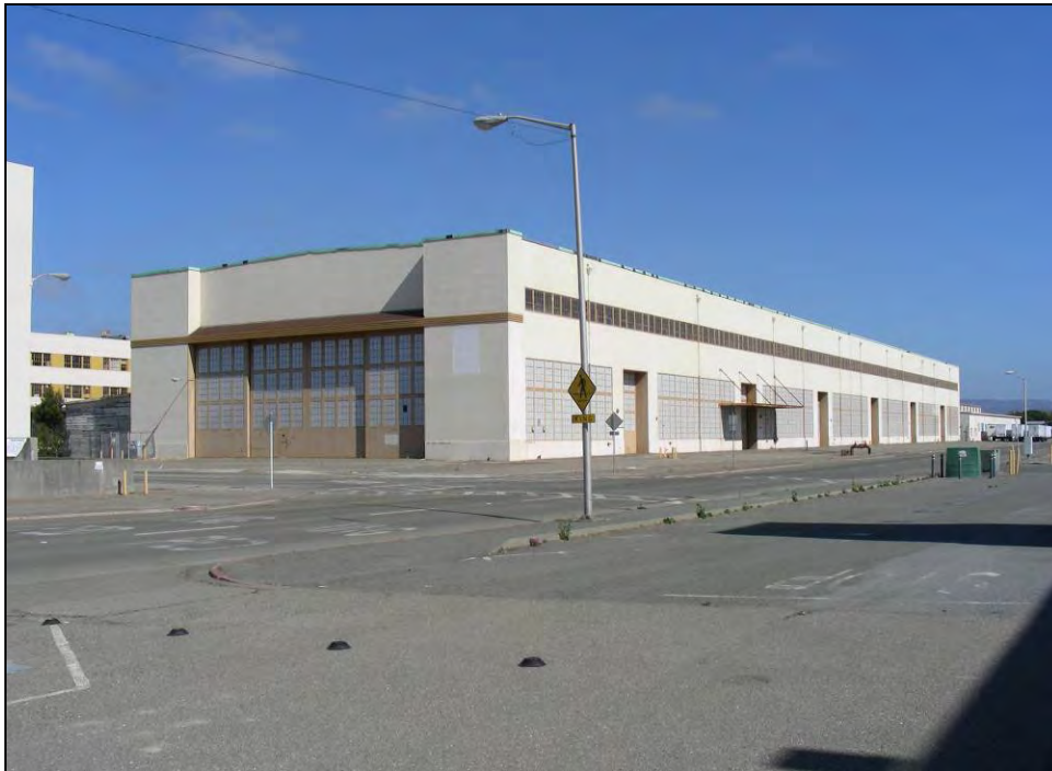
Photograph 2: West and south sides, camera facing northeast, October 8, 2009.
