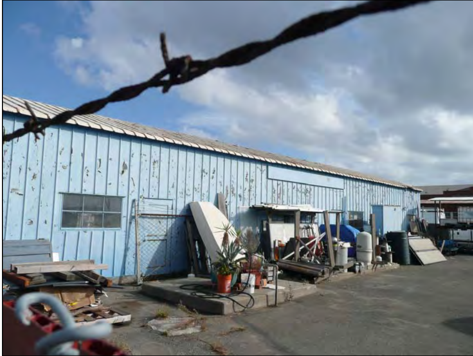
Photograph 2: Camera facing southeast, October 14, 2009.
