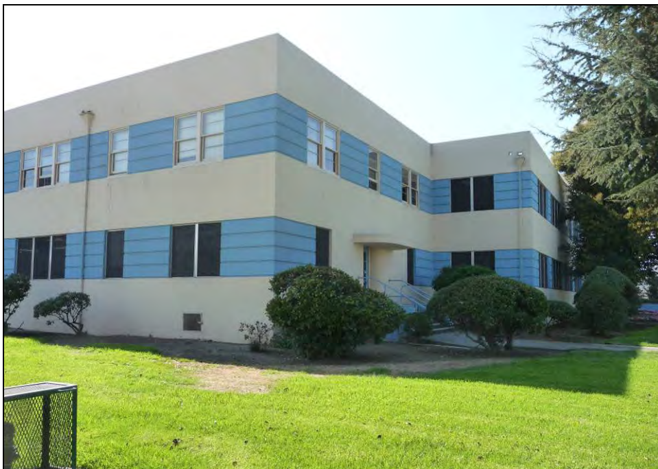
Photograph 3: Building 1, main façade and east wing, camera facing southwest, October 6, 2009.
