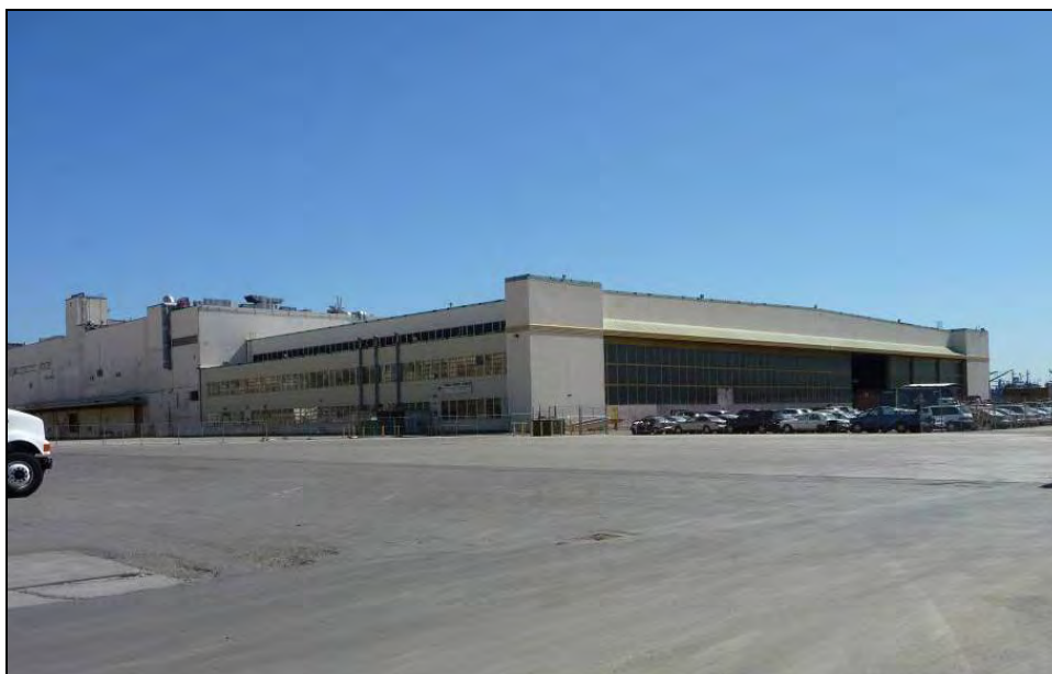
Photograph 2: Building 11, camera facing southeast, October 11, 2009.
