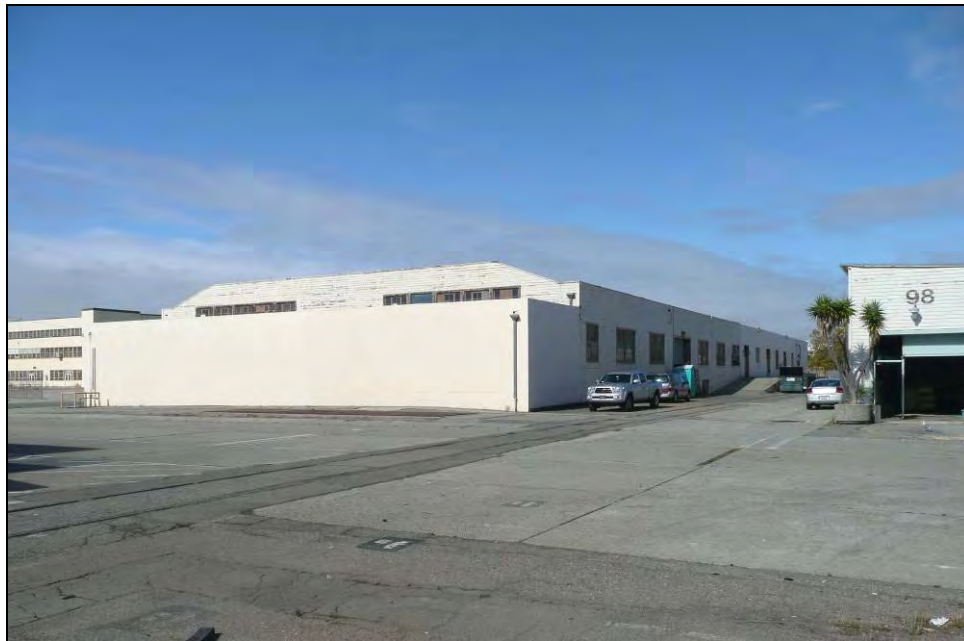
Photograph 2: Camera facing northwest, showing south end of building, October 15, 2009.
