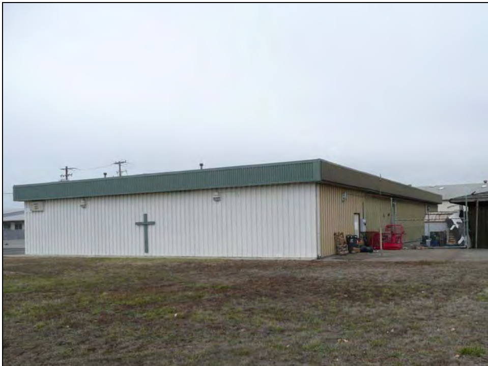
Photograph 3: Camera facing northwest, October 15, 2009.
