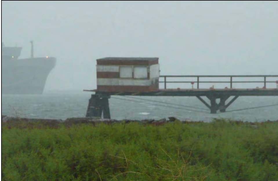
Photograph 10: Building 513, camera facing southeast, October 13, 2009.
