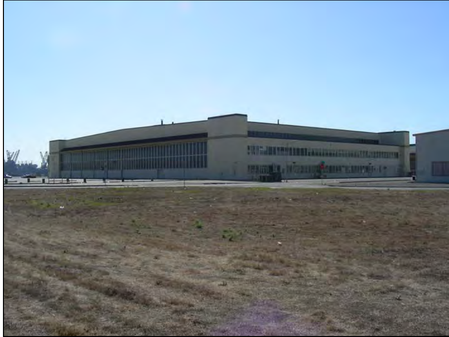
Photograph 3: Building 41, camera facing southwest, October 8, 2009.
