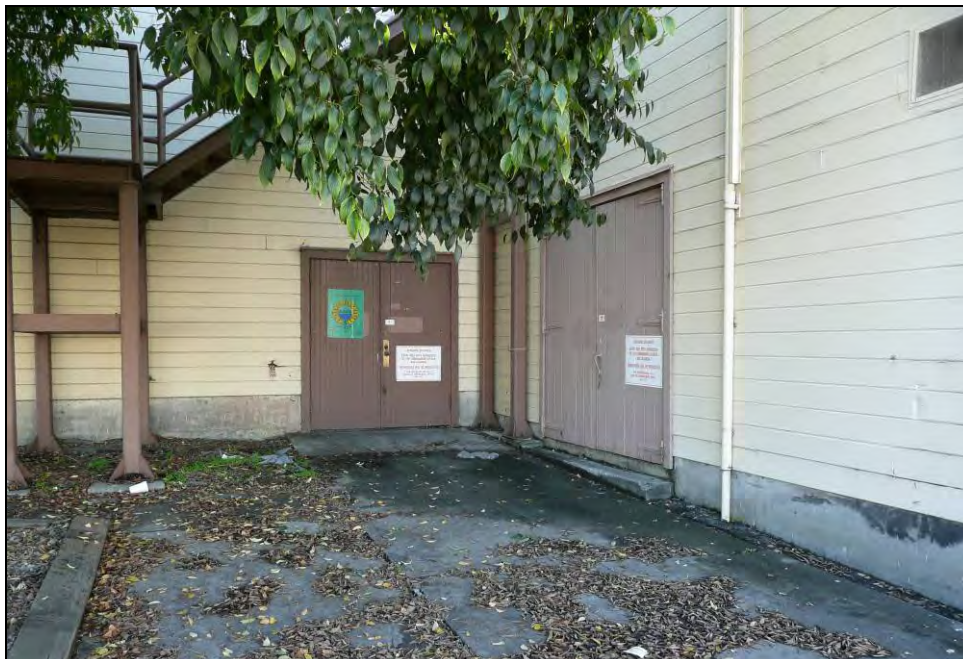
Photograph 5: Addition and north wall detail, camera facing south, October 15, 2009.
