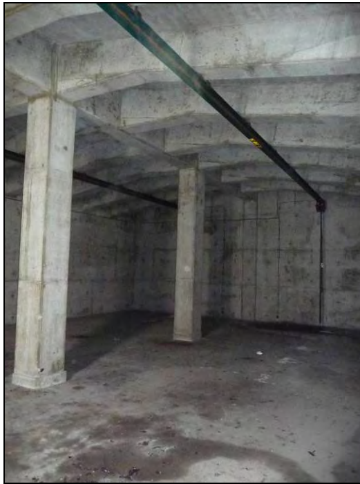
Photograph 3: Interior of Building 51, camera facing east, December 16, 2009.
