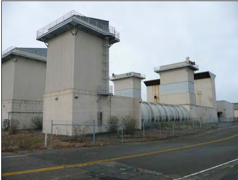
Photograph 3: North side, camera facing southwest, October 14, 2009.
