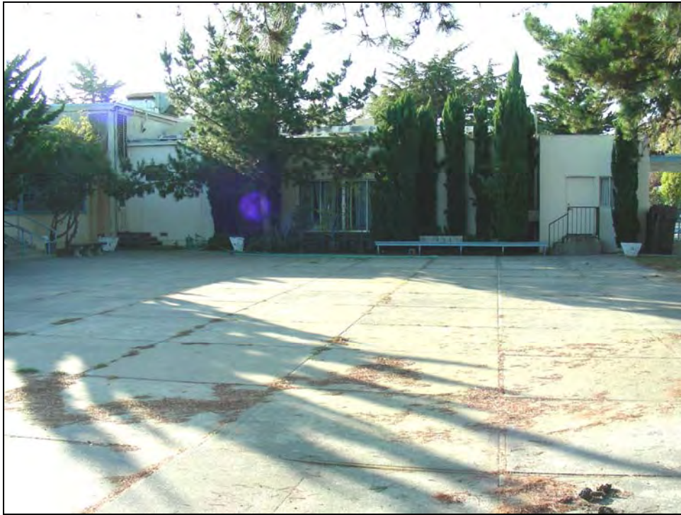
Photograph 6: West side of 'L' shaped north-south wing, camera facing northwest, November 12, 2009.
