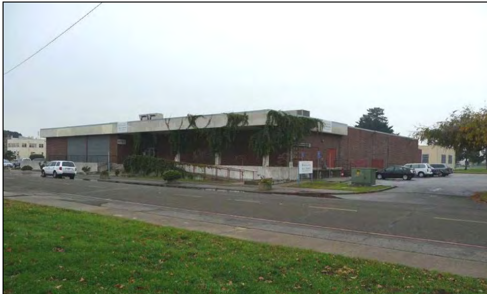
Photograph 54: Bowling Lanes (Building 525), December 11, 2009.
