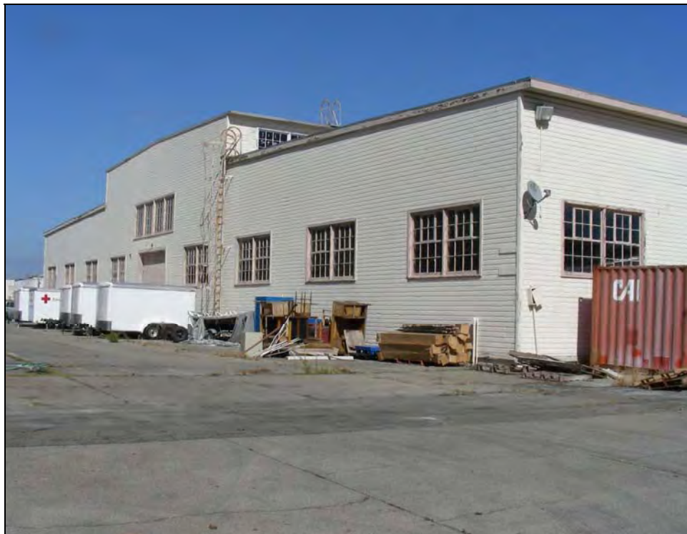
Photograph 4: West side, camera facing northeast, October 8, 2009.
