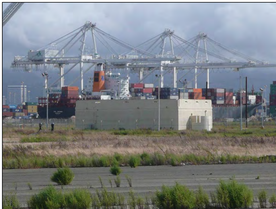
Photograph 11: Building 594, camera facing northeast, October 14, 2009.
