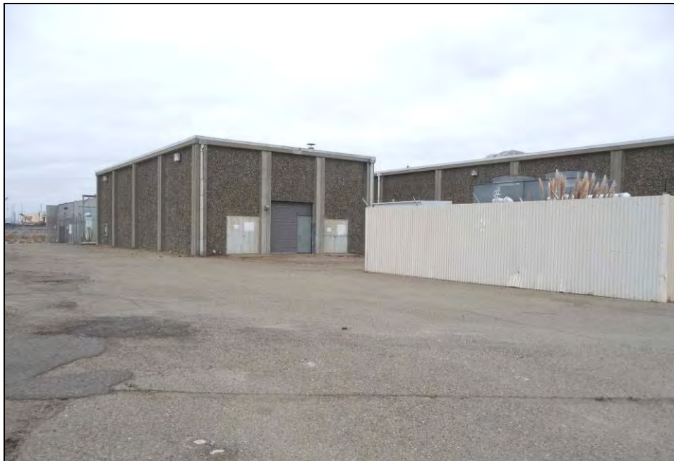
Photograph 3: Building 529, facing northwest, October 8, 2009.
