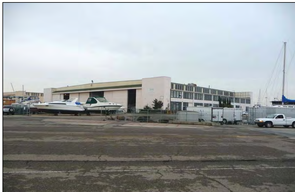
Photograph 3: Building 167, camera facing southeast, October 13, 2009.
