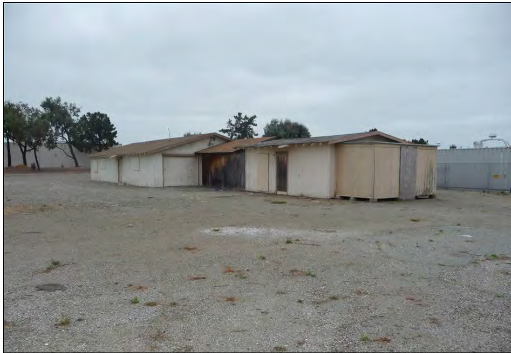
Photograph 2: Camera facing southwest, October 8, 2009.
