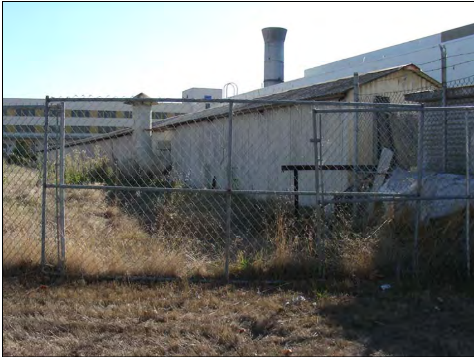
Photograph 3: Camera facing southwest, October 14, 2009.
