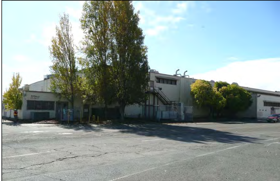
Photograph 6: Northeast corner, camera facing southwest, October 15, 2009.
