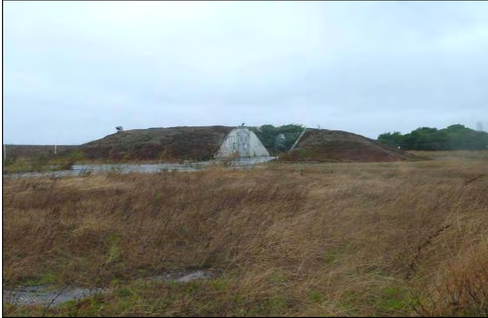
Photograph 2: Building 353, camera facing southwest, October 13, 2009.
