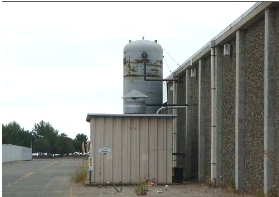
Photograph 5: Building 600 and equipment attached to Building 530, camera facing south, October 8, 2009.
