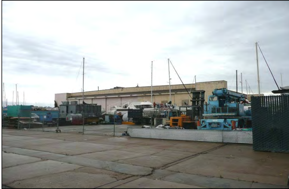
Photograph 4: Building 167, south side, camera facing northwest, October 13, 2009.
