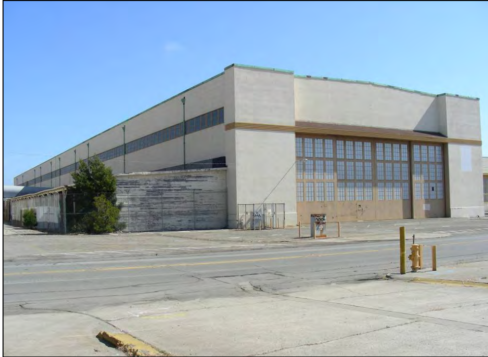
Photograph 1: North and west sides, showing hangar type doors and shed roof addition, camera facing southeast, October 8, 2009.
