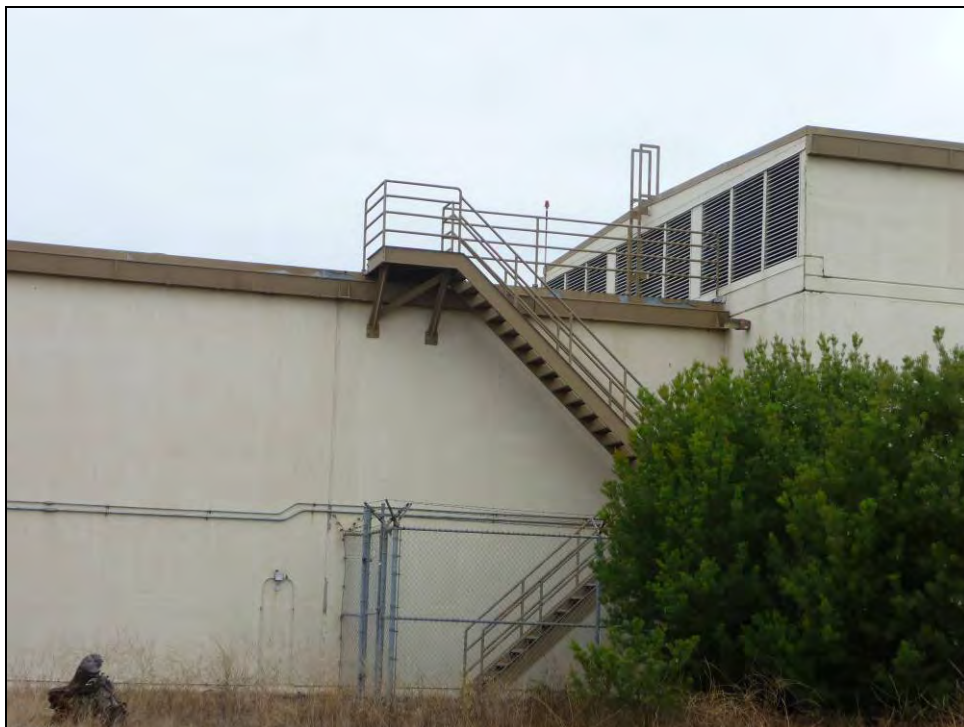
Photograph 5: East side middle section, camera facing northwest, October 8, 2009.
