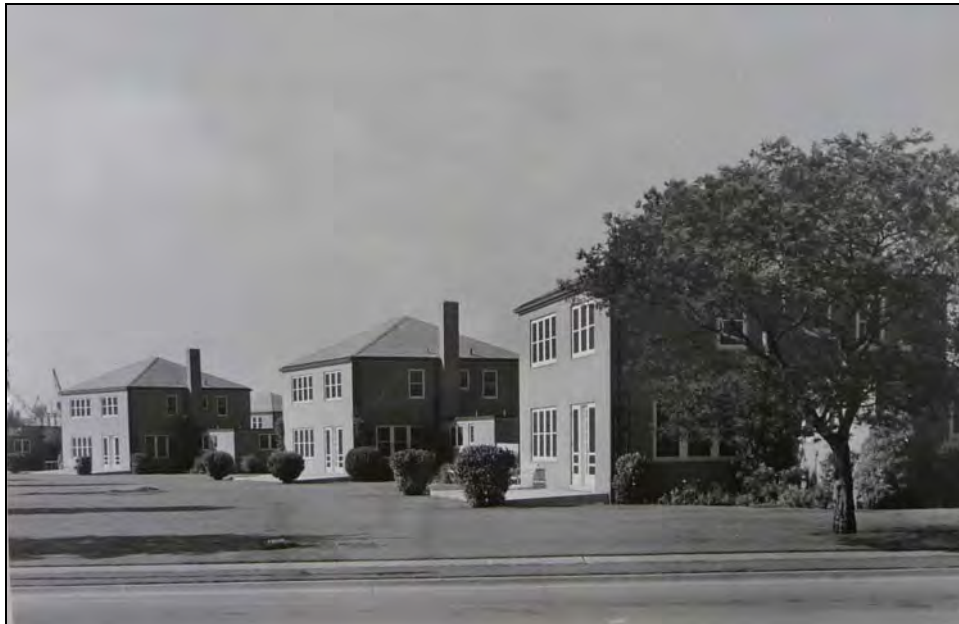
Photograph 6: May 1945 view of Officer’s Housing rear before sun porch additions, camera facing north. 2
