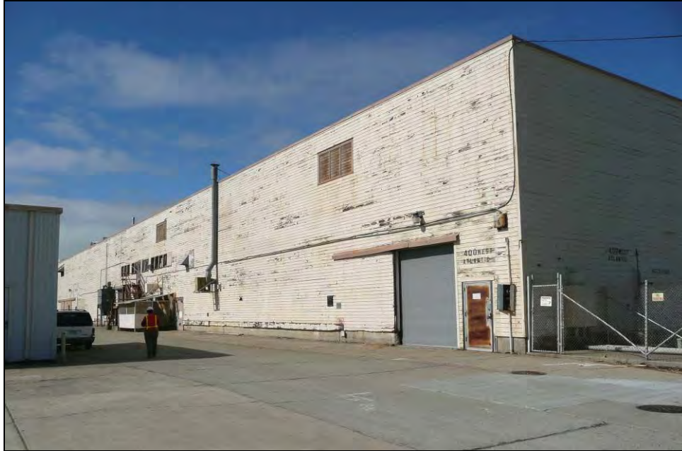
Photograph 8: South wall at southeast corner, camera facing northwest, October 15, 2009.
