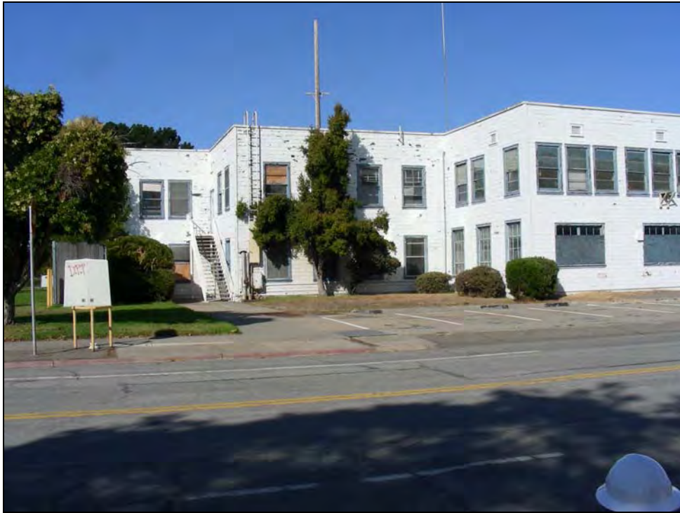
Photograph 4: Southwest setbacks, camera facing northeast, October 7, 2009.
