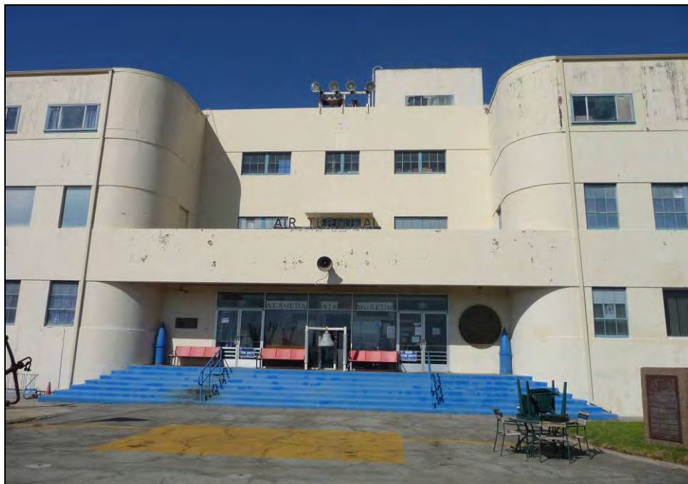
Photograph 2: South side entrance detail, camera facing north, October 8, 2009.
