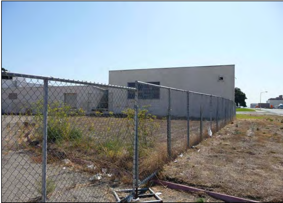
Photograph 13: Building 63, camera facing south, October 6, 2009.
