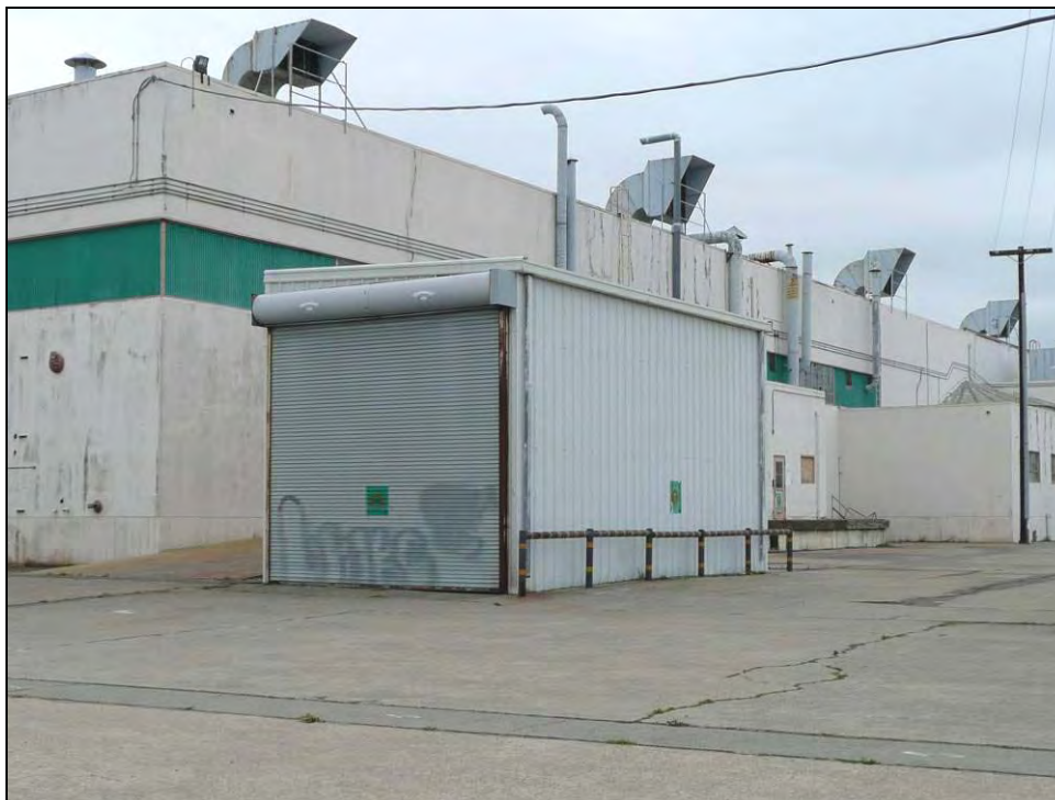
Photograph 5: Representative example of Buildings 360 A-D, at southwest corner of Building 360, camera facing southeast, October 15, 2009.
