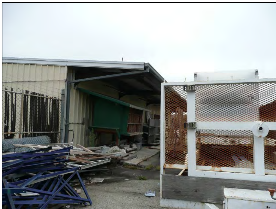
Photograph 2: Camera facing southeast, October 15, 2009.
