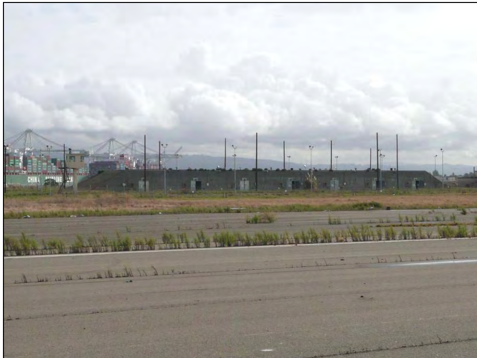
Photograph 7: Building 497, camera facing northeast, October 14, 2009.
