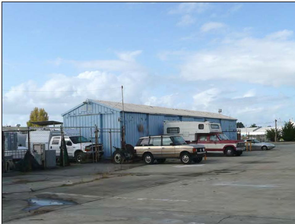
Photograph 3: Camera facing northwest, October 14, 2009.
