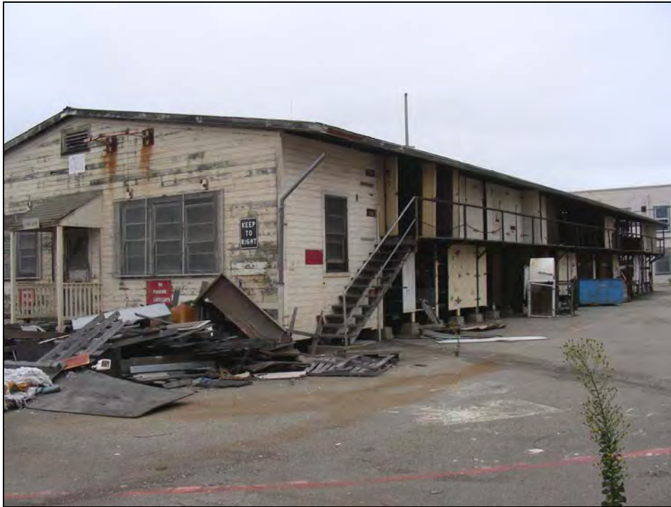
Photograph 4: Northeast corner, camera facing southwest, October 8, 2009.
