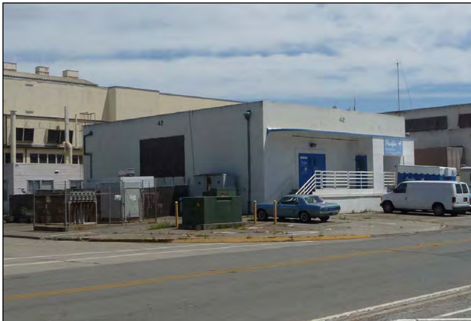
Photograph 1: Camera facing southeast, June 9, 2010.
