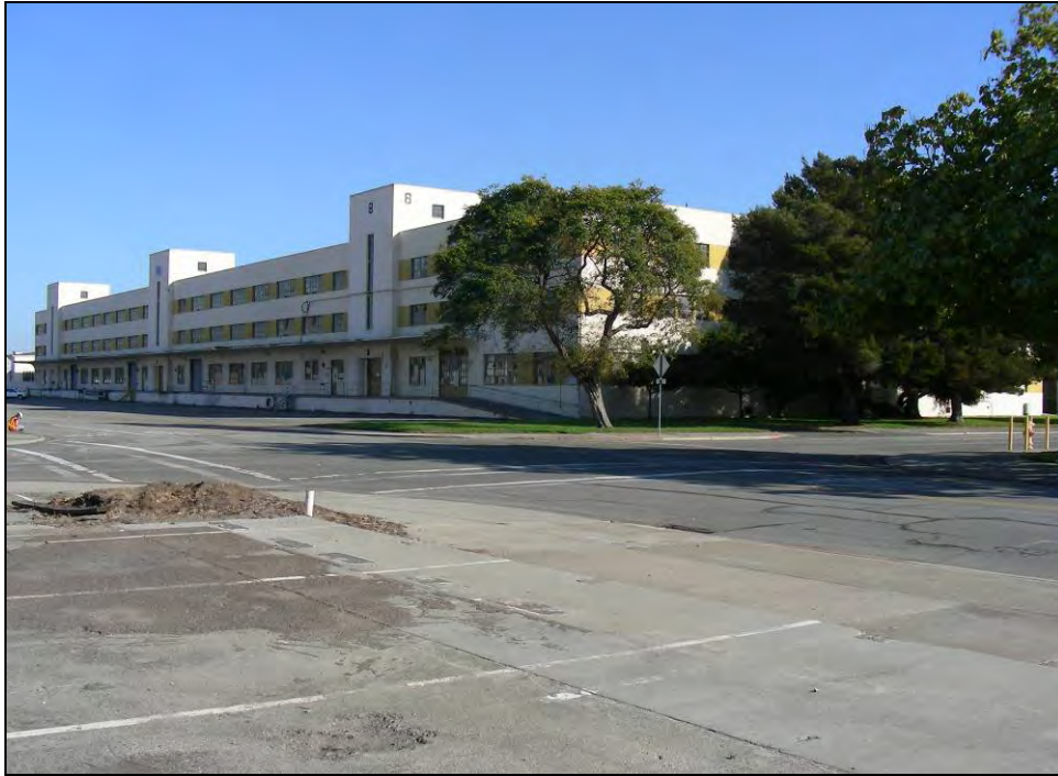
Photograph 1: Camera facing southeast, October 7, 2009.
