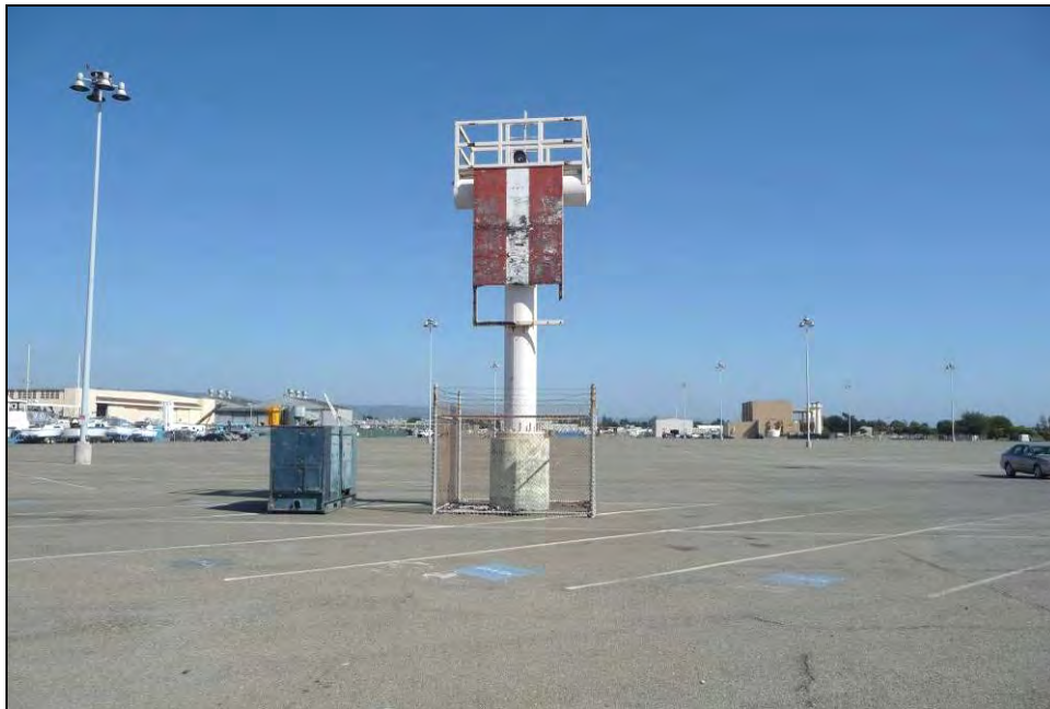
Photograph 60: Building 302W Navigation Range Light, October 8, 2009.
