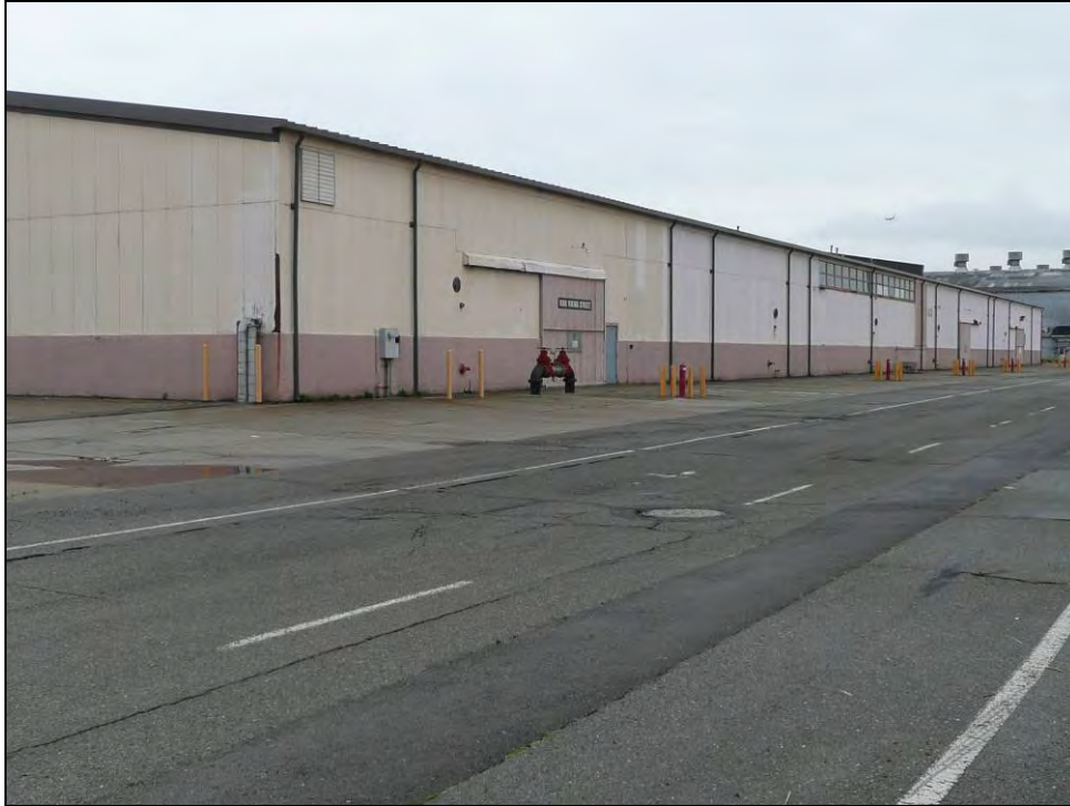
Photograph 2: Building 169, west side, camera facing southeast, October 14, 2009.
