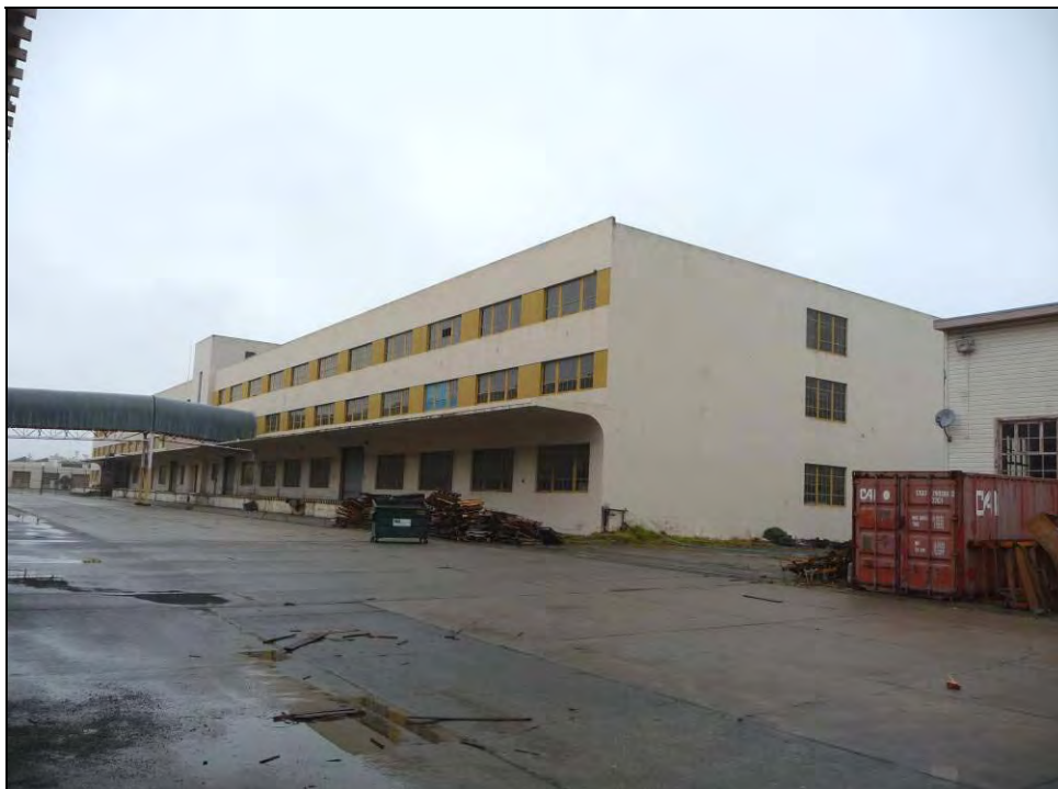
Photograph 2: South side of Building 8 with single tower, camera facing northwest, December 16, 2009.
