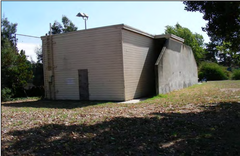
Photograph 3: Building 382, Squash Courts, facing southeast, September 29, 2009.
