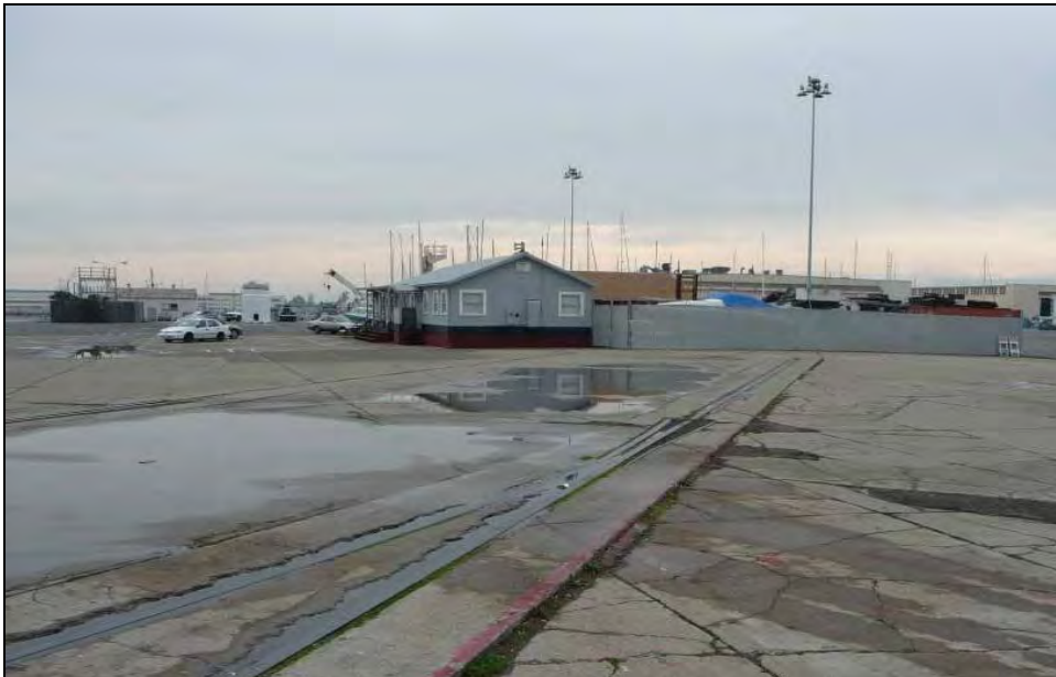
Photograph 3: Crane tracks, camera facing north, December 16, 2009.
