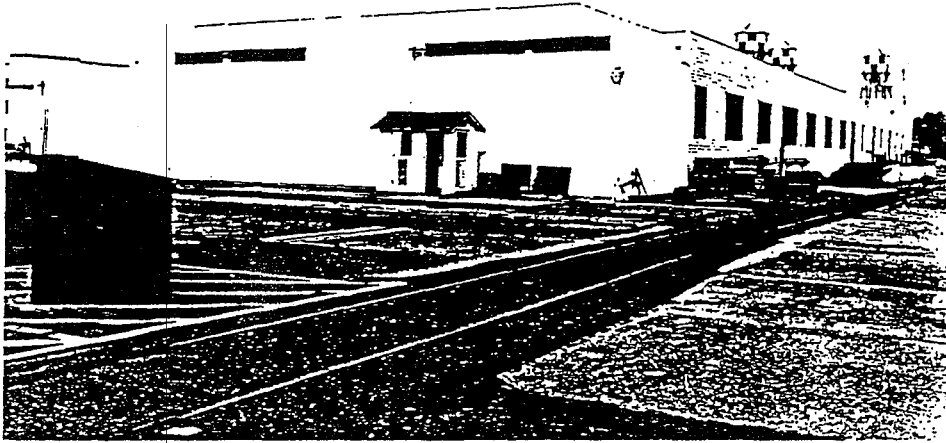
NAS ALAMEDA Building 13
