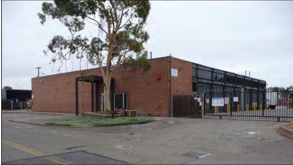
Photograph 2: Building 608, camera facing southeast, October 8, 2009.
