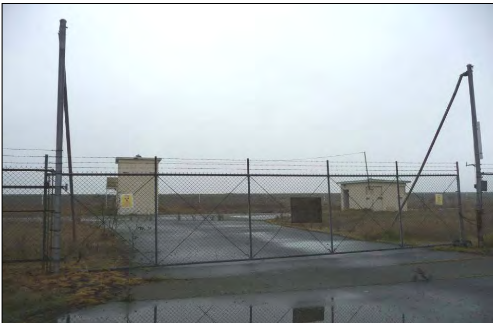
Photograph 3: Building 441 on right, Building 442 on left, camera facing south, December 16, 2009.
