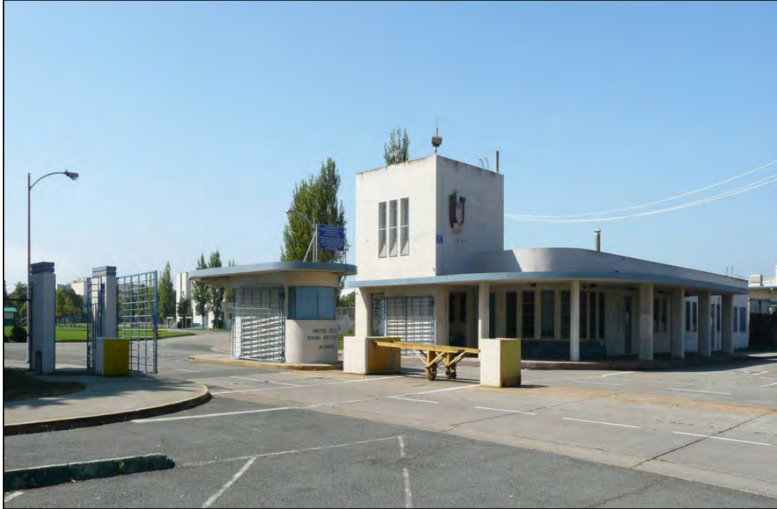
Photograph 1: Building 30 (right) and Building 31 (center), camera facing southwest, September 25, 2009.
