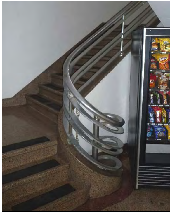
Photograph 10: Detail of curved staircase and metal railing, camera facing north, December 16, 2009.
