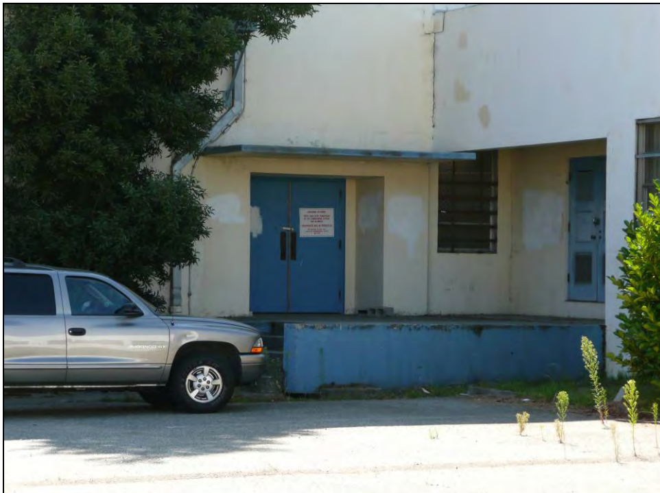
Photograph 2: Loading platform corner of theater and offices, camera facing southwest, September 25, 2009.
