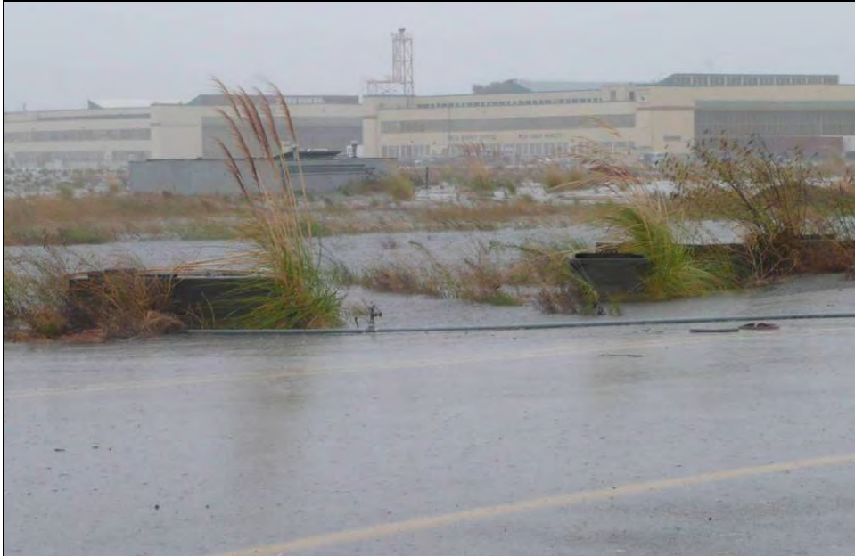
Photograph 24: Concrete boxes at the northwest corner outside of the structure, camera facing northeast, October 13, 2009.
