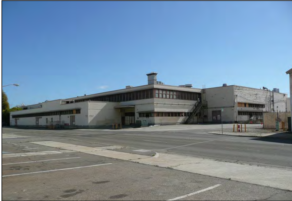
Photograph 1: Northwest corner, camera facing southeast, October 15, 2009.
