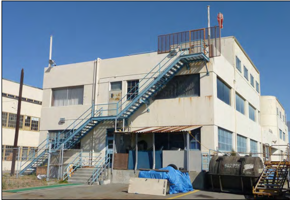
Photograph 3: West wall, camera facing northeast, October 8, 2009.
