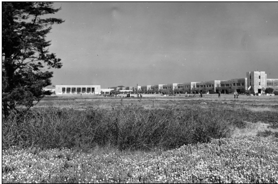
Photograph 7: View across the mall toward BEQ and Mess hall, 1945. 42
