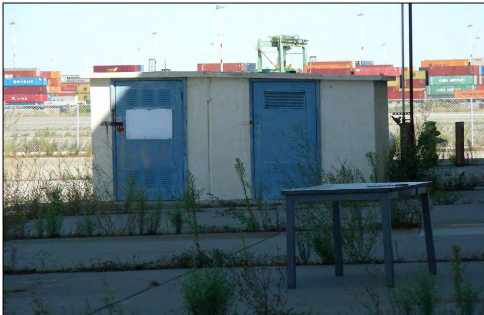
Photograph 4: Building 319, camera facing northwest, September 30, 2009.
