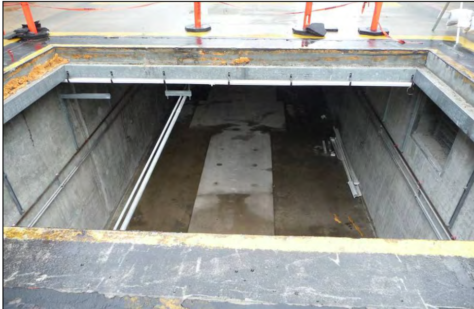
Photograph 7: Pier 2, preparation to move existing electrical transformers below deck, December 16, 2009.
