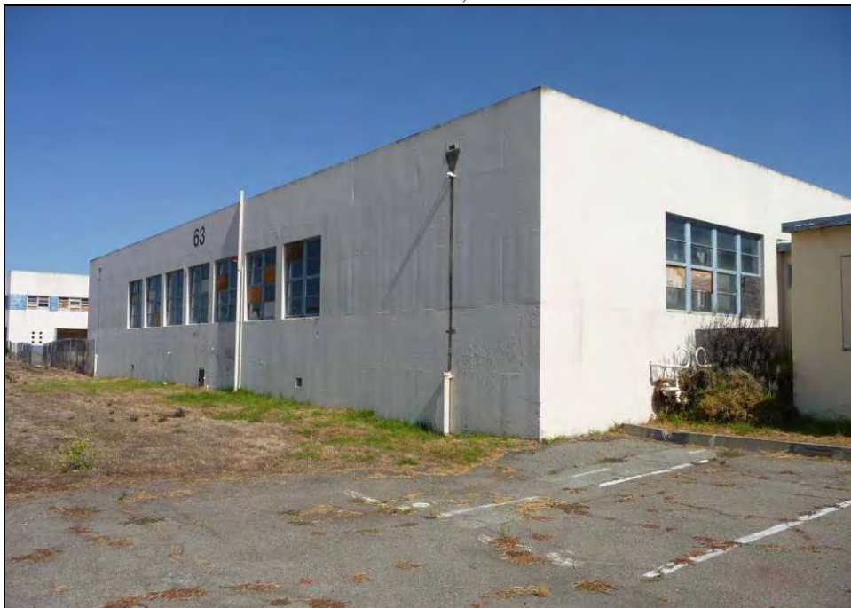
Photograph 12: Building 63, camera facing northeast, October 6, 2009.
