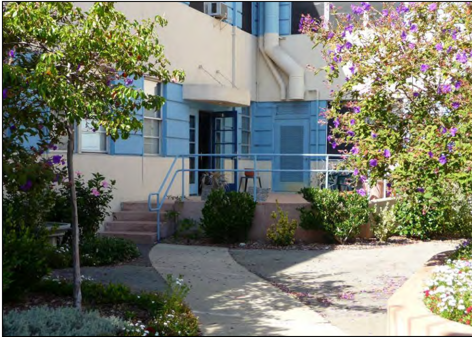
Photograph 6: Building 1, corner of south center wing (left) and north building (right), camera facing northwest, October 6, 2009.
