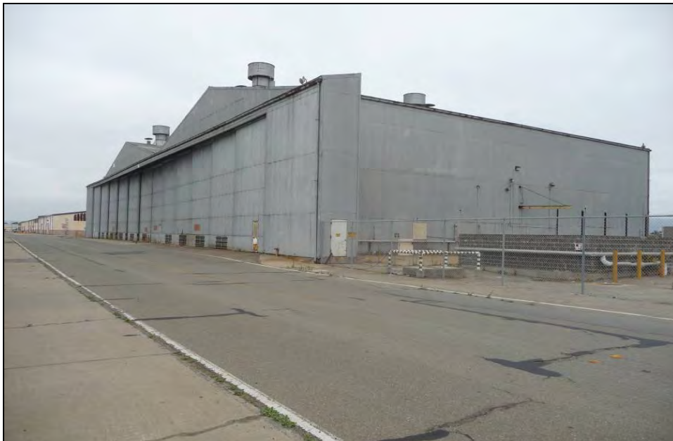
Photograph 3: Building 410, southwest corner, camera facing northeast, October 8, 2009.
