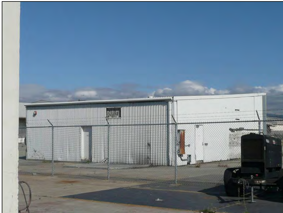
Photograph 2: Camera facing northeast, October 14, 2009.
