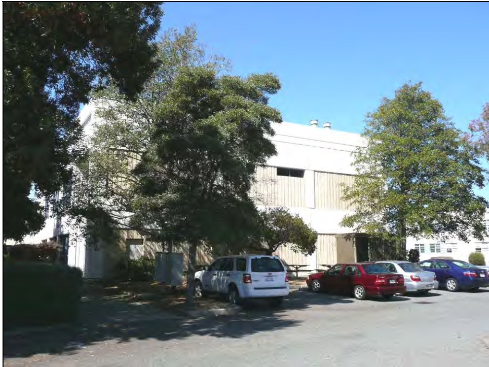
Photograph 3: Camera facing west, September 25, 2009.
