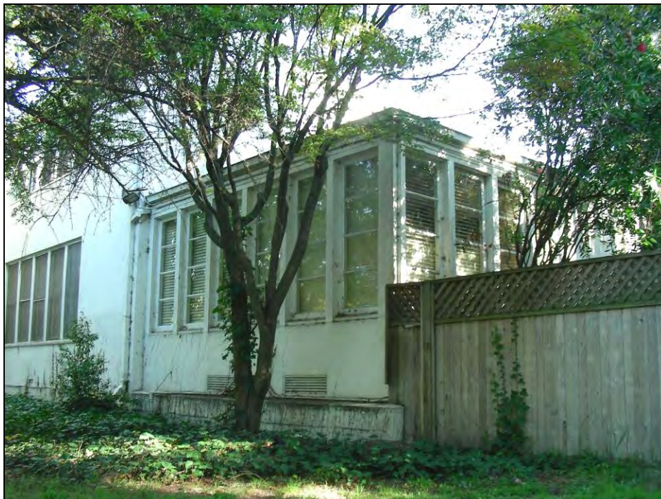
Photograph 4: Sun porch, camera facing southeast, November 12, 2009.
