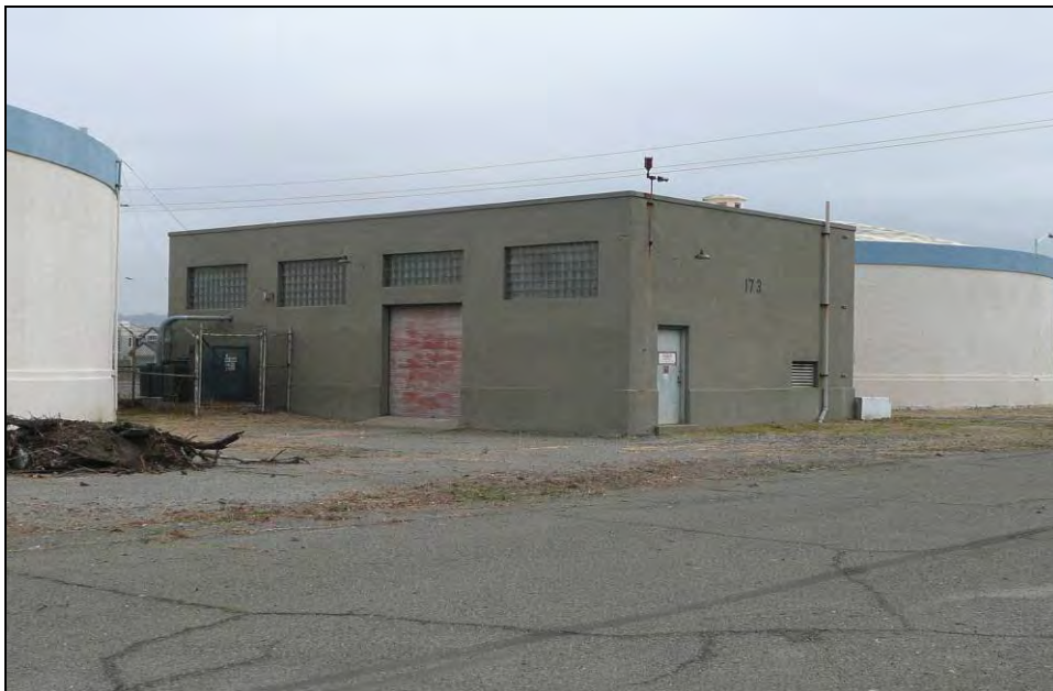
Photograph 2: Building 173, camera facing northeast, October 15, 2009.
