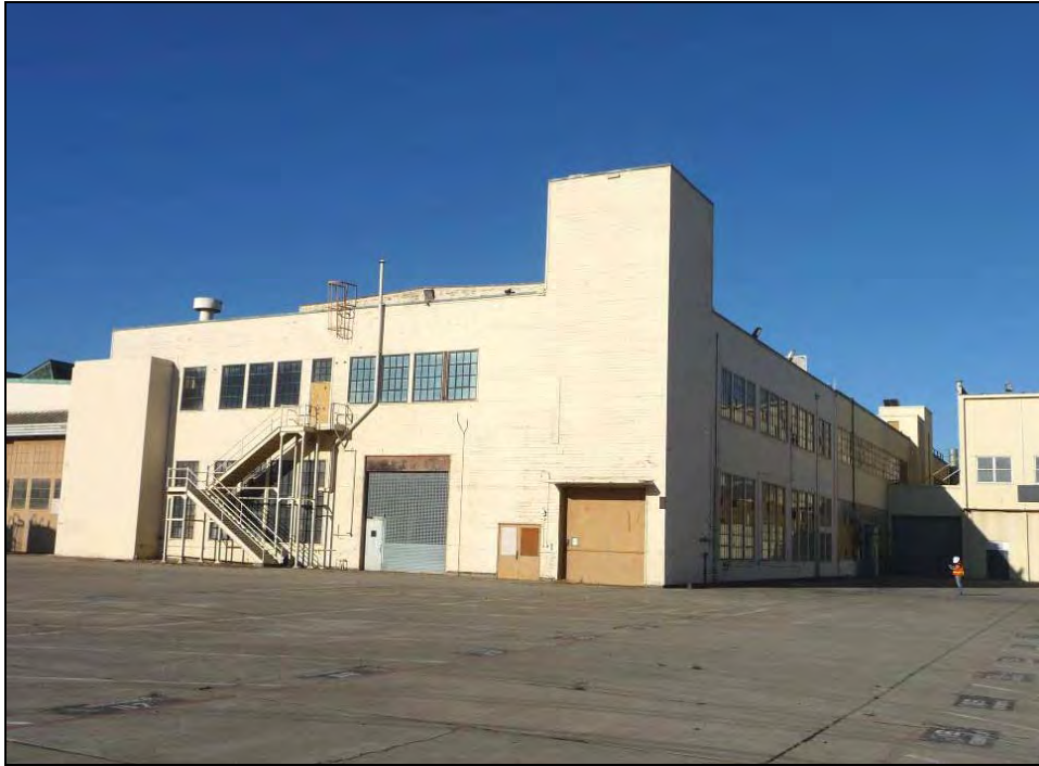
Photograph 13: Northeast Extension, camera facing southwest, October 1, 2009.
