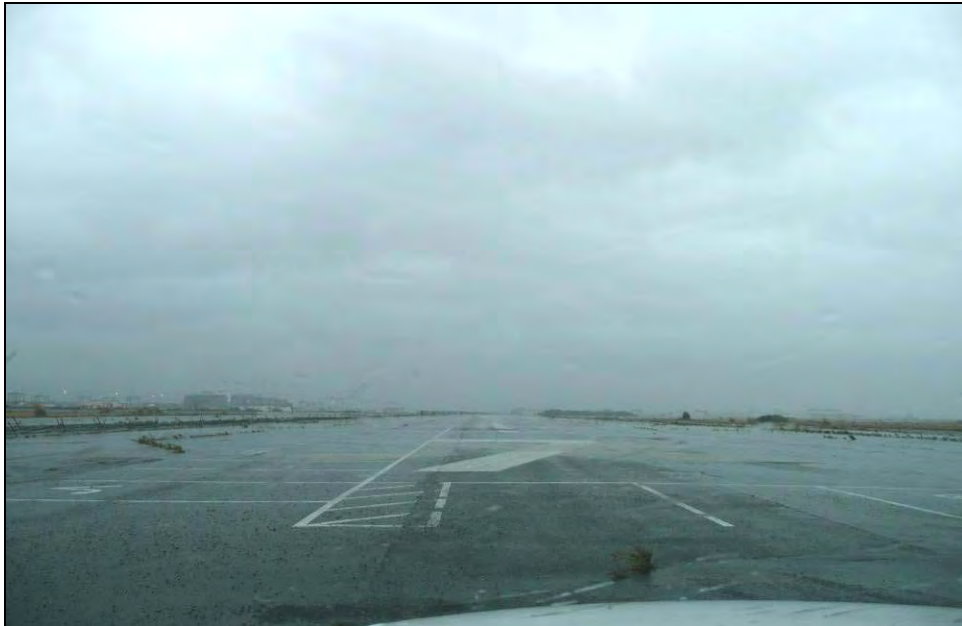
Photograph 4: Runway 7, camera facing east, October 13, 2009.
