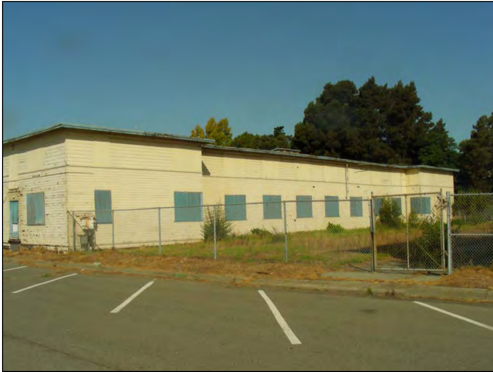
Photograph 3: Building 135, east wing, facing northwest, October 6, 2009.
