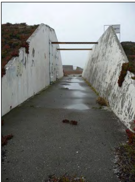
Photograph 2: Detail of Building 51 with Building 50 in background, camera facing west, December 16, 2009.
