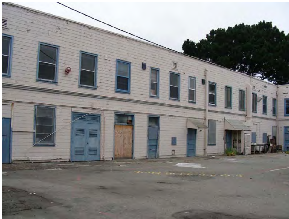
Photograph 6: East side of West Wing, camera facing northwest, October 8, 2009.
