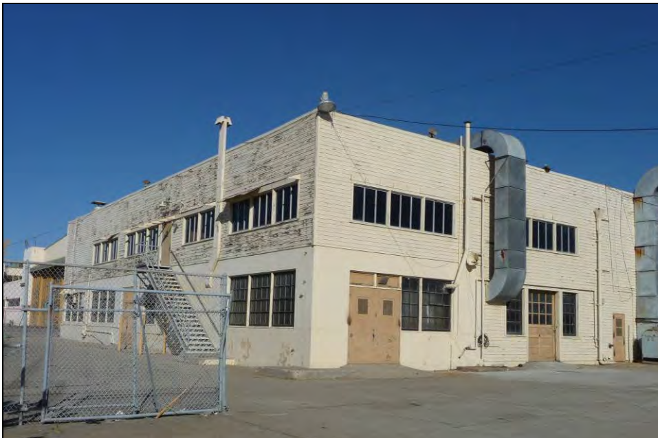
Photograph 14: Southeast corner Building 5, camera facing northwest, October 1, 2009.
