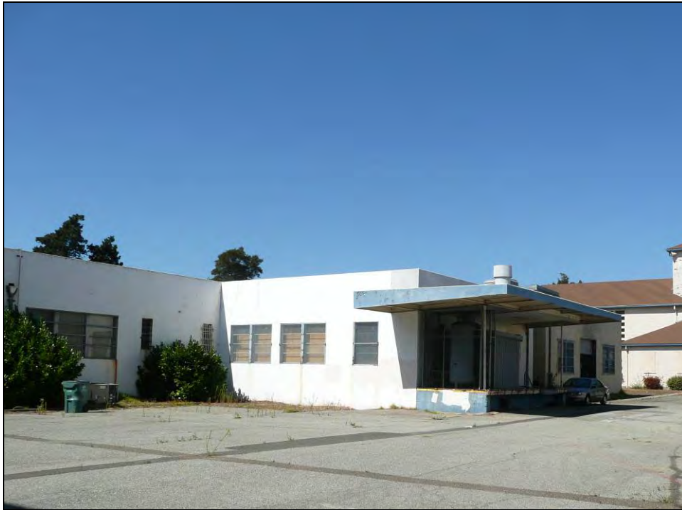
Photograph 3: Post office loading dock, camera facing northwest, September 25, 2009.
