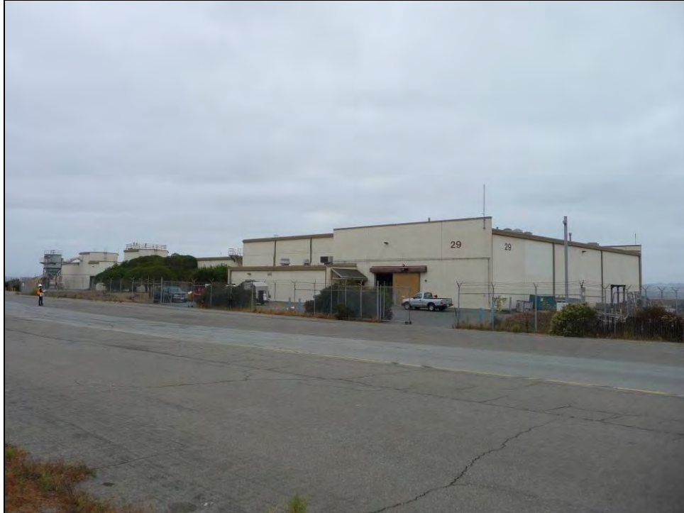
Photograph 2: Camera facing northwest, October 8, 2009.
