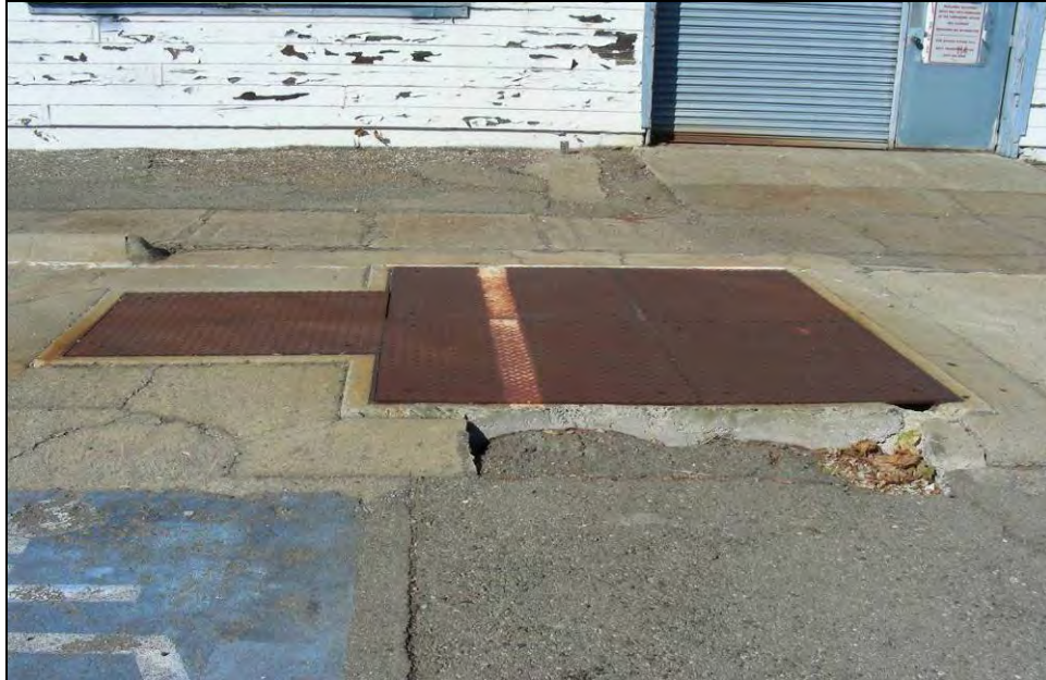
Photograph 8: Building 469 section 1, facing north, October 7, 2009.
