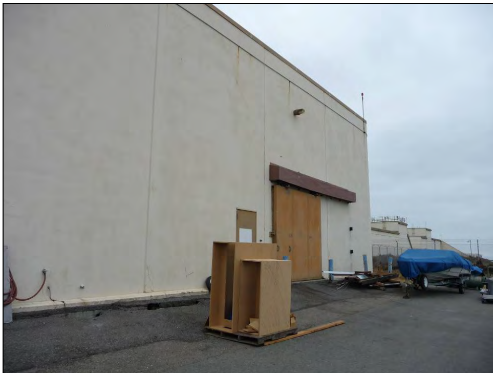
Photograph 12: North end of west side, camera facing southwest, October 8, 2009.
