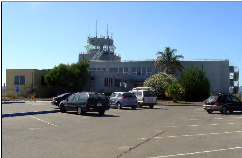
Photograph 4: Building 19, east side, camera facing west, September 30, 2009.
