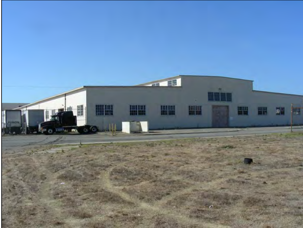
Photograph 1: Southeast corner, camera facing northwest, October 8, 2009.
