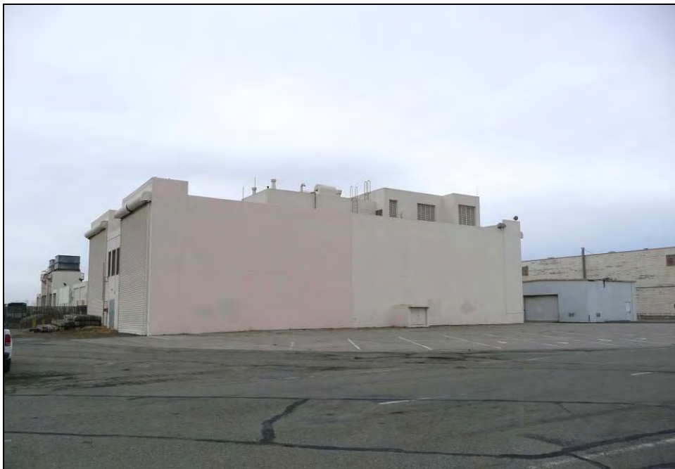
Photograph 3: Test Cells 11 and 12, camera facing northwest, October 15, 2009.
