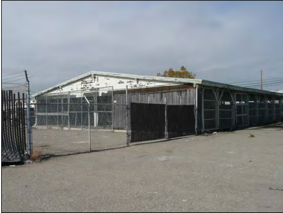
Photograph 3: South and east sides, camera facing northwest, October 15, 2009.
