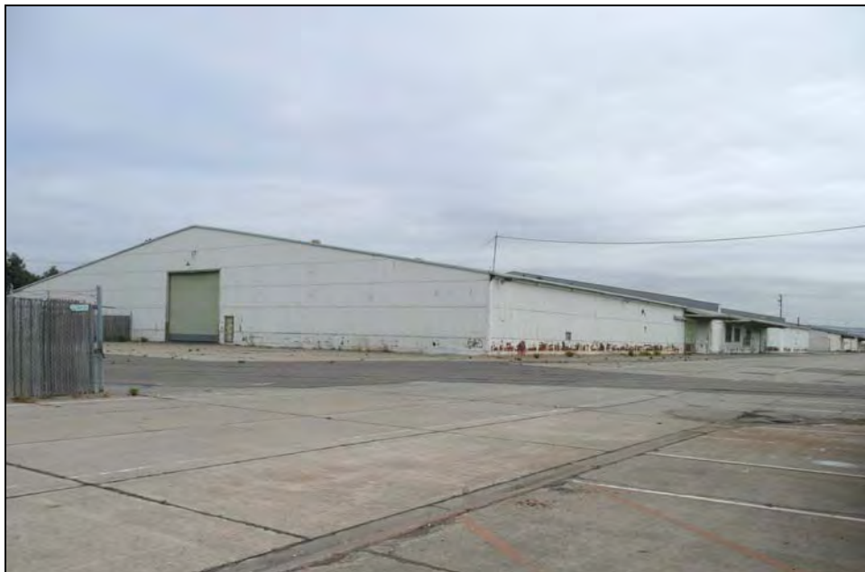
Photograph 49: Storehouse (Building 117), October 15, 2009.
