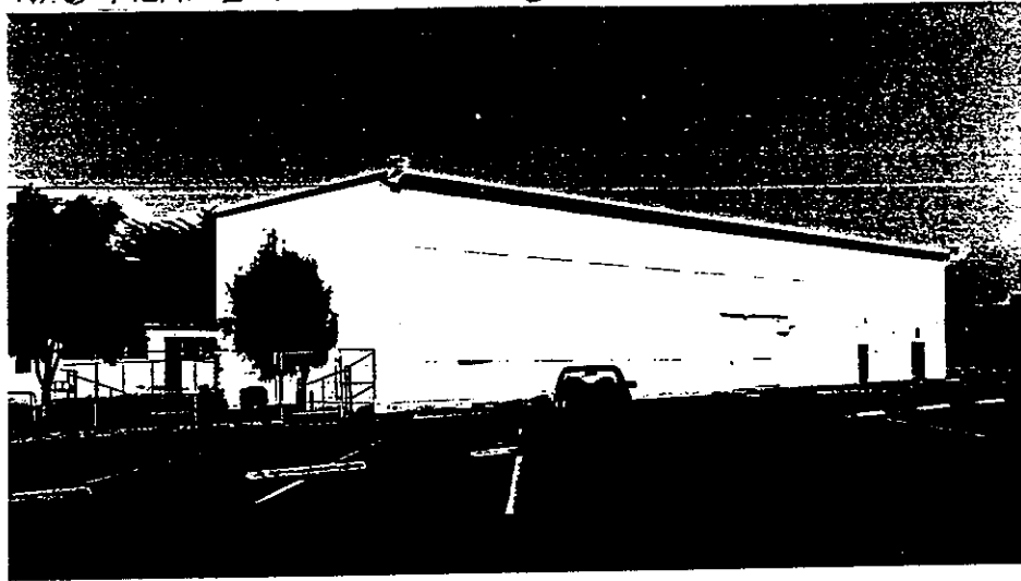
NAS ALAMEDA Building 137
