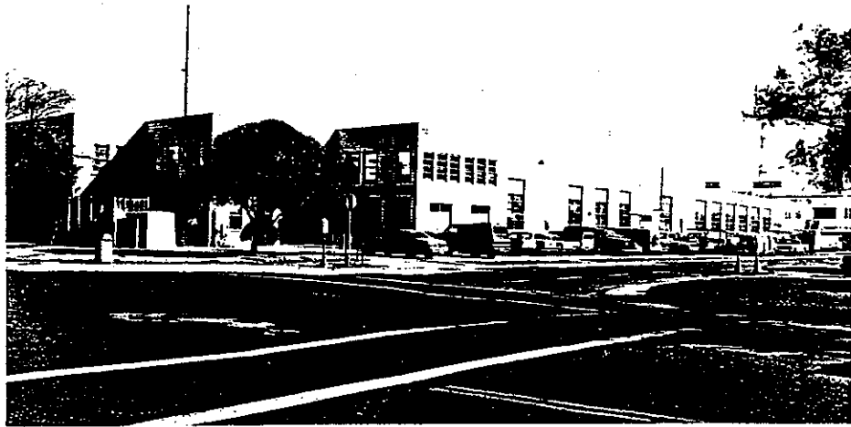
NAS ALAMEDA Building 114
