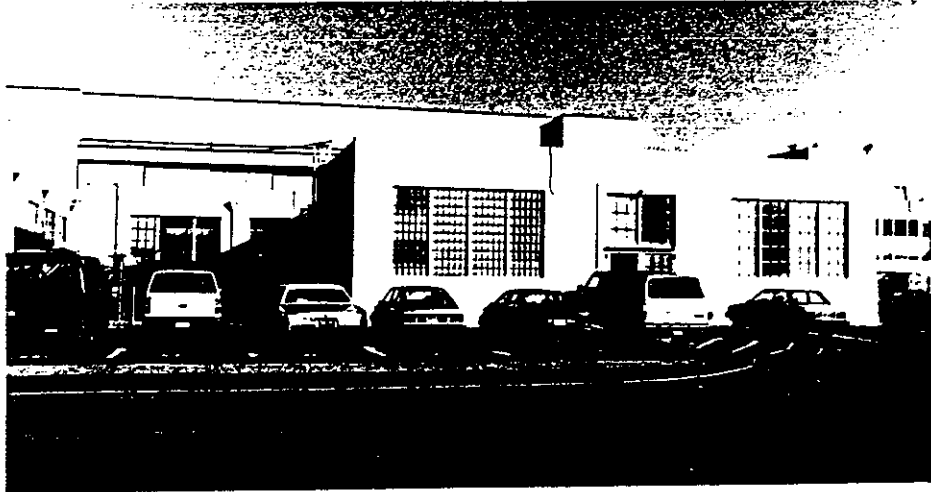
NAS ALAMEDA Building 44
