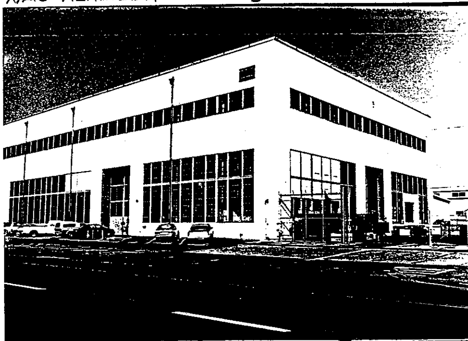
NAS ALAMEDA Building 9
