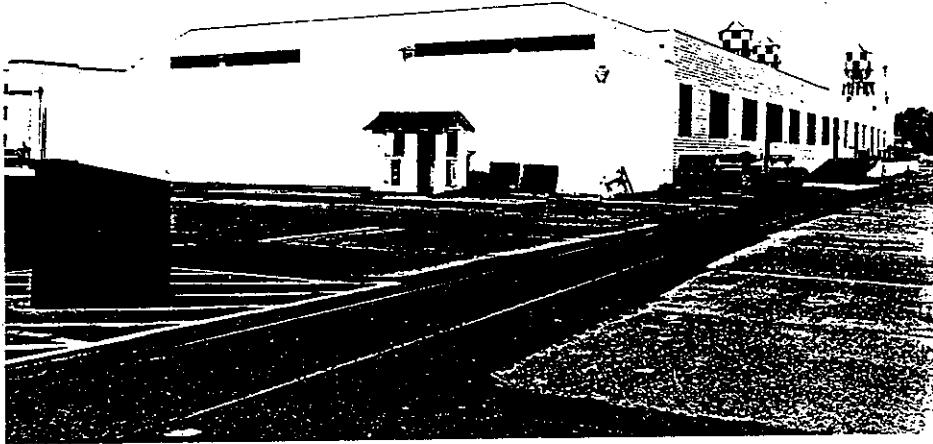
NAS ALAMEDA Building 13
