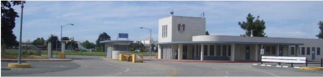
Figure 14. Main Gatehouse and Sentry House (Buildings 30 and 31), NAS Alameda, 2004.
