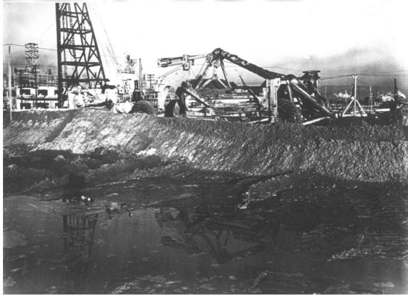
Figure 9. Filling underway at NAS Alameda, 1940. Courtesy of National Archives Pacific Region, San Bruno
