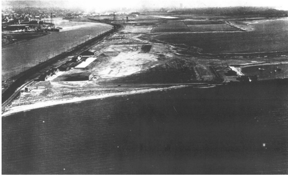
Figure 7. View of Alameda Municipal Airport, 1934. Courtesy National Archives Pacific Region, San Bruno
