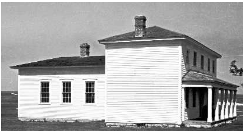
In a project at Fort Hays, Kansas, the wood frame officers' quarters were restored to the late 1860s—their period of significance. This included replacing a missing kitchen ell, chimneys, porch columns, and cornice, as well as closing a later window opening in the main block. The building and others in the museum complex is used to interpret frontier history. Photo: NPS files.
