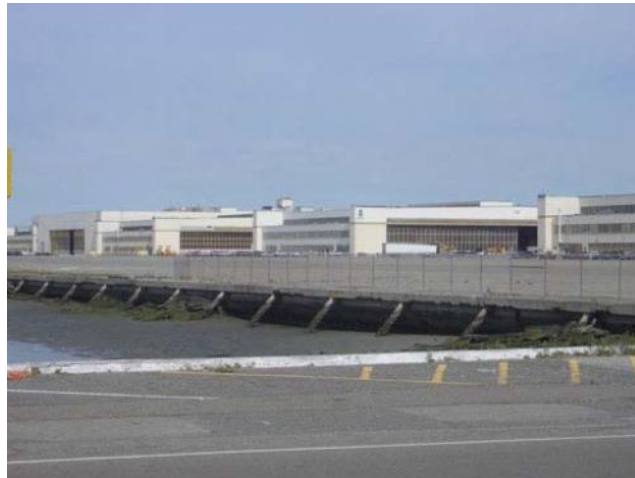
Figure 24. Seaplane Hangars north of Seaplane Lagoon, 2004
