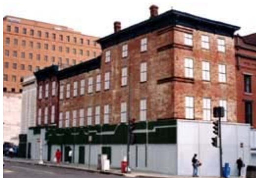
Urban buildings often need additional protection from unwanted entry and graffiti. This commercial building uses painted plywood panels to cover its glass storefronts. The upper windows on the street sides have been painted to resemble 19th century sash.
