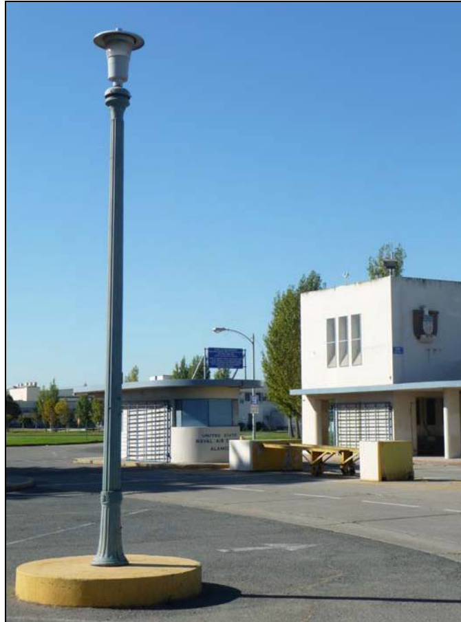
Photograph 87: Light pole in parking lot at Main Gate, sentry house (Building 31) and gate house (Building 30) in background.
