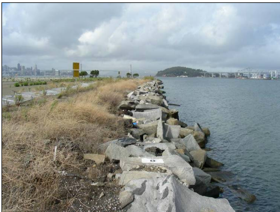
Photograph 139: Riprap along north edge of airfield, facing west.
