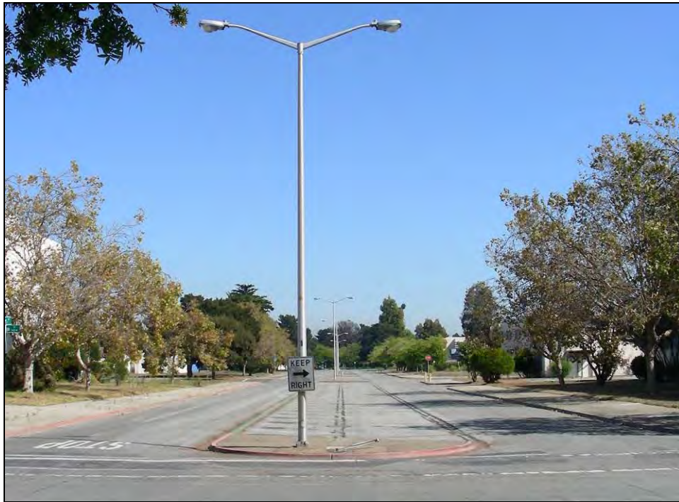
Photograph 27: Diagonal parking in the middle of West Essex Drive; new cobra lights offset north of the main east-west axis.
