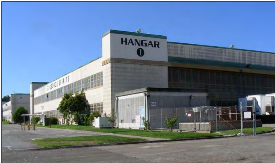
Photograph 62: Lawn panels along east side of landplane hangars. Building 21 in foreground and Building 22 in background.
