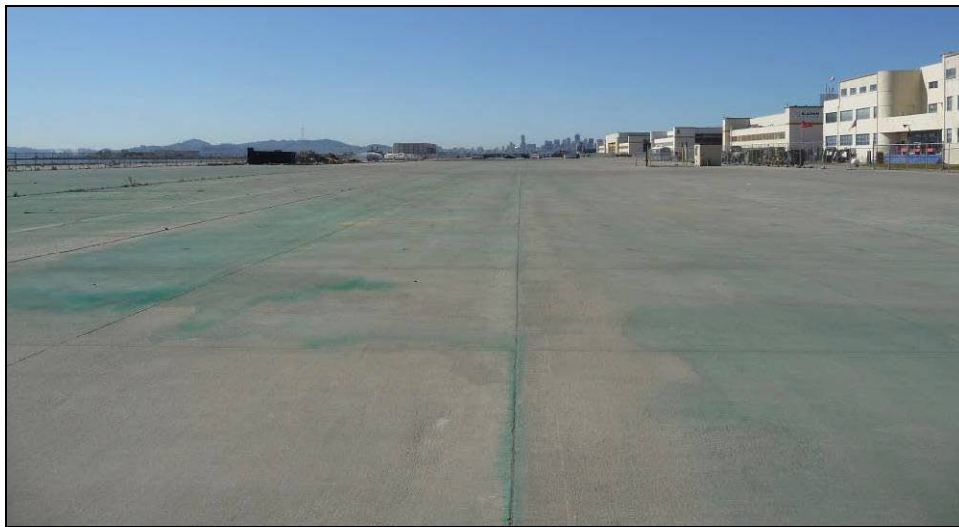
Photograph 113: Operations Area. Note aligned façades of seaplane hangars, Buildings 39, 40, 11, 12, 400, and large expanse of pavement; Building 77 at far right.
