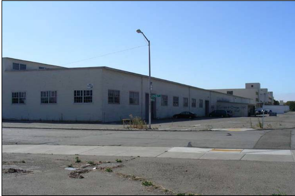
Photograph 93: Most of the Shops Area is paved; view showing Building 92 at the intersection of Pan Am Way and West Ranger Avenue.
