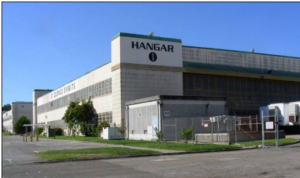
Photograph 117: Lawn panels along east side of landplane hangars. Building 21 in foreground and Building 22 in background.
