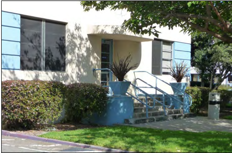
Photograph 33: Example of trapezoidal-shaped free-standing concrete pots found in the Administrative Core; south side of Building 1.
