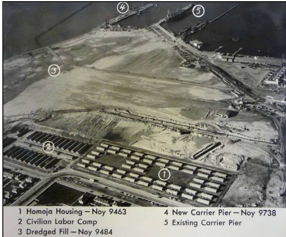
Photograph 21: November 1944. Newly dredged and filled southeast portion of the station. This area was outside the original station plan, and outside the original planting plan. (Numbers and labels from original photo identification.) 87
