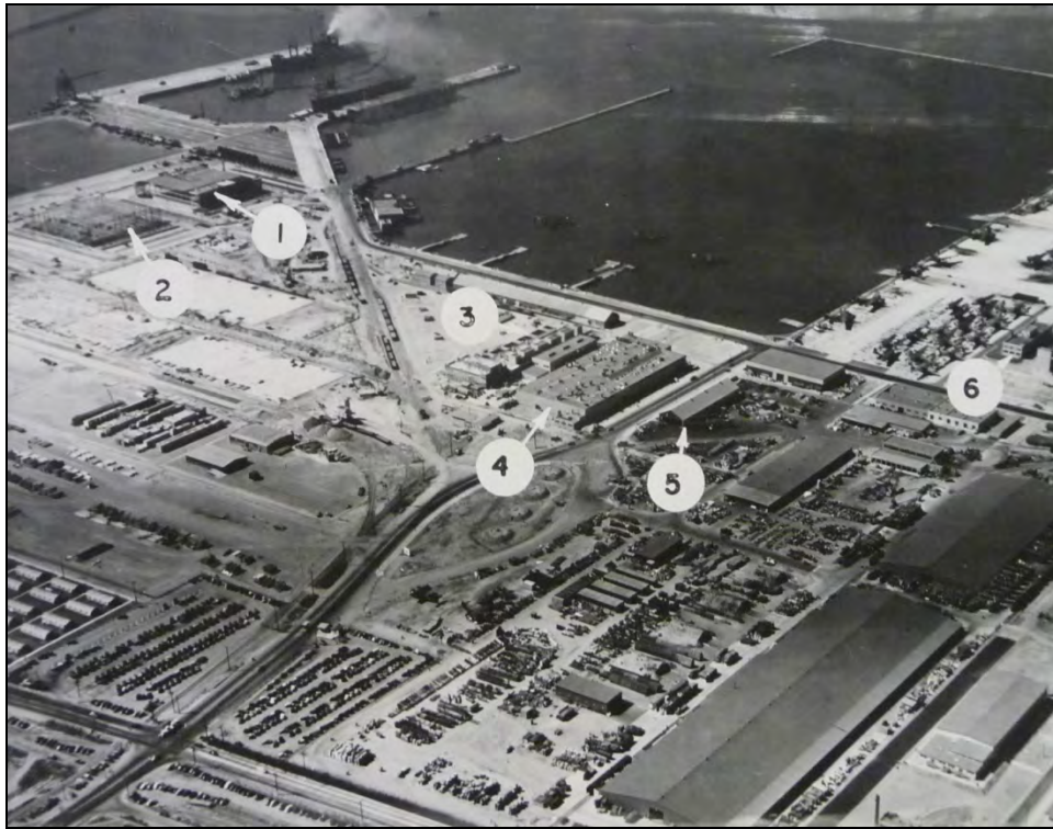
Photograph 51: September 1945. Southeast portion of the station retained a utilitarian appearance throughout World War II, distinct from the formal design of the core of the station. (Numbers from original photo identification.) 78
