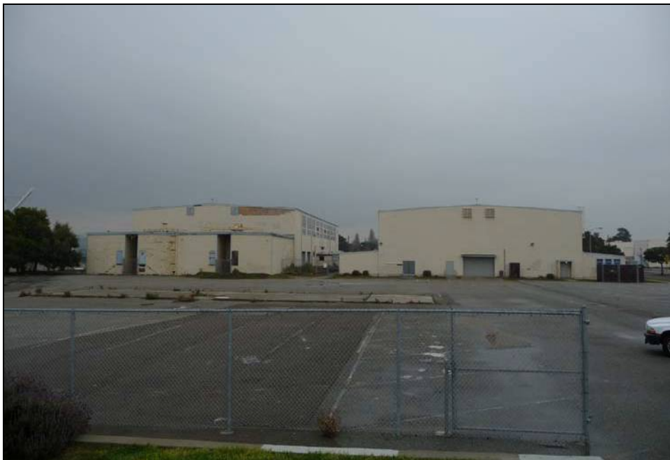
Photograph 120: Large open paved area west of Buildings 76 and 134.
