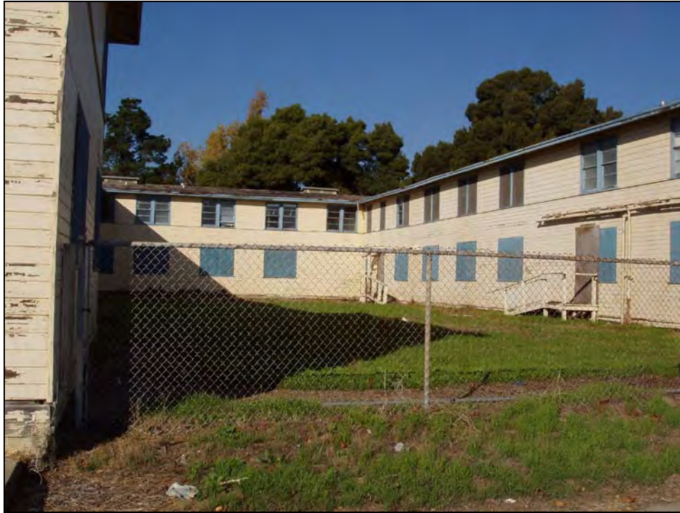
Photograph 7: Typical courtyard found in Administrative Core, Building 135; facing north.
