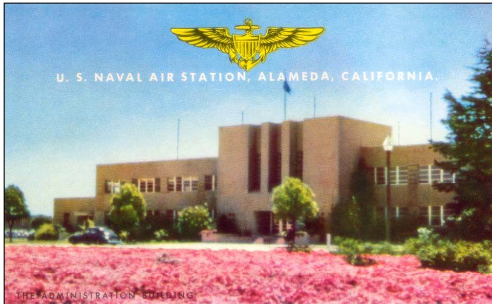
Photograph 29: Period postcard depicting Building 1, circa 1943. Colorized postcard exaggerated the vibrancy of ice plant in entry mall.
