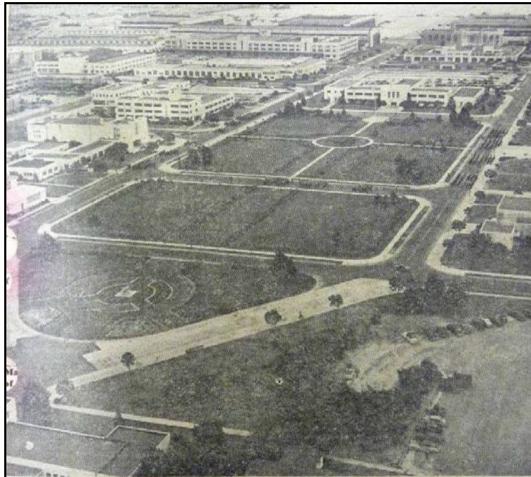
Photograph 38: Oblique aerial photograph, 1950. 121 Entry mall, facing south. Planting plan has been altered from original design to include the lines of plantings running north-south through the entry mall. Also note installation of new planting around monument in triangle.
