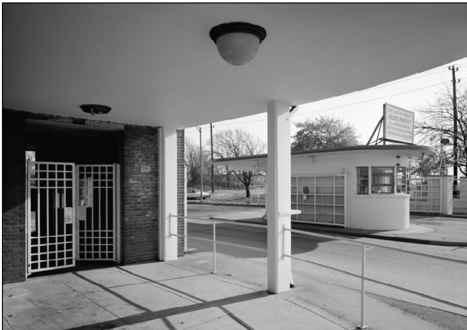
Photograph 45: Buildings 10 and 850, NAS Quonset Point, RI, 1979. 53
