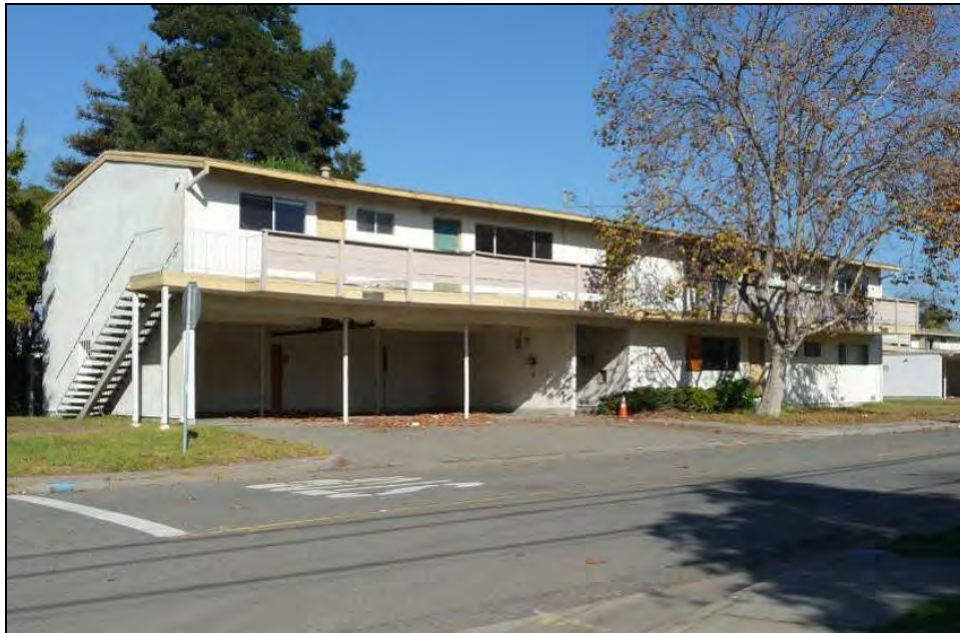
Photograph 79: Typical Capehart multiple family unit, Building 754, camera facing northeast, November 12, 2009.
