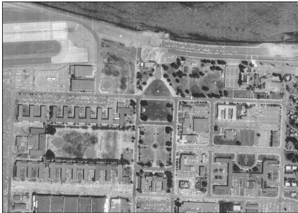
Photograph 75: Aerial Photograph, 1985. Only two temporary barracks remain in block north of the BOQ (Building 17). 127
