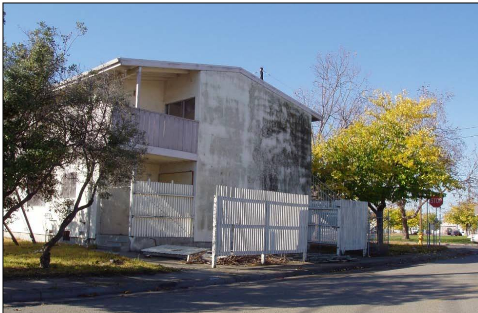
Photograph 135: Fenced drying yard.
