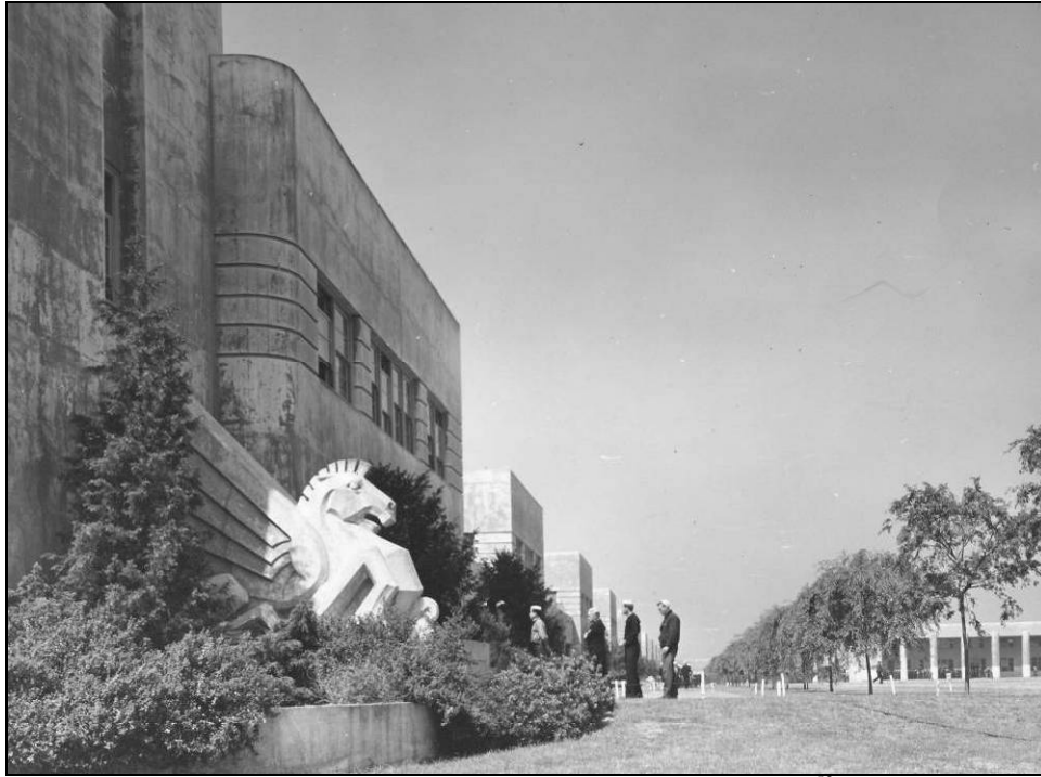
Photograph 8: East end of Building 2, May 1945. 52
