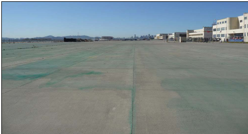
Photograph 58: Operations Area. Note aligned façades of seaplane hangars, Buildings 39, 40, 11, 12, 400, and large expanse of pavement; Building 77 at far right.
