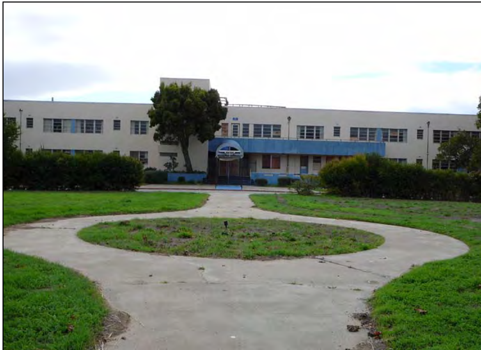
Photograph 30: Curved path on the north side of BOQ Building 17.
