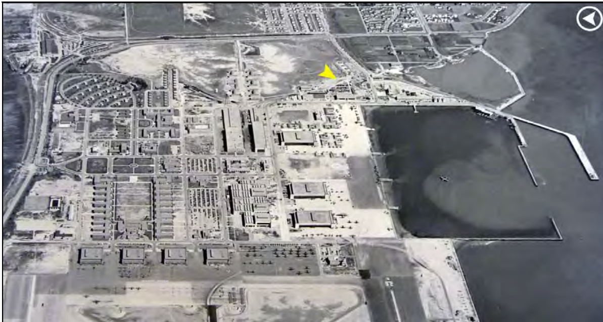
Photograph 49: June 1943. Triangular area east of Seaplane Lagoon (area indicated with yellow arrow) was secondary to the station plan. As the Supply Department expanded during the war, the area developed a utilitarian layout and landscape. 69
