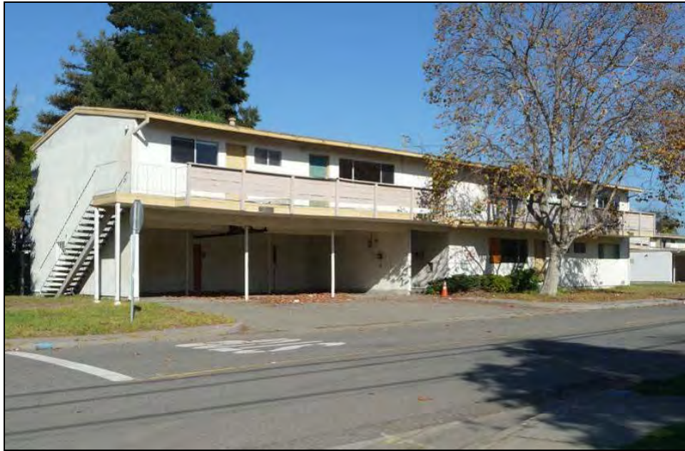
Photograph 113: Typical Capehart multiple family unit, Building 754, camera facing northeast, November 12, 2009.
