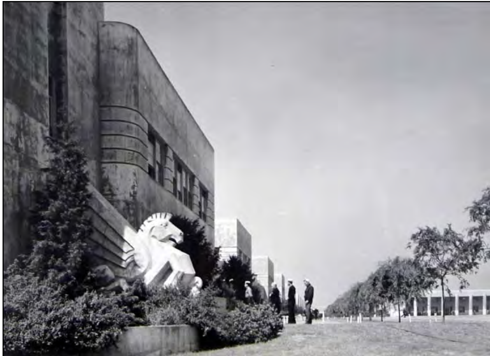
Photograph 97: 1945. Building 4 at left, camera facing west. The tree line depicted in the planting plan had been executed (right), and like other buildings in the Administrative Core, Building 4 had foundation shrubbery. 105
