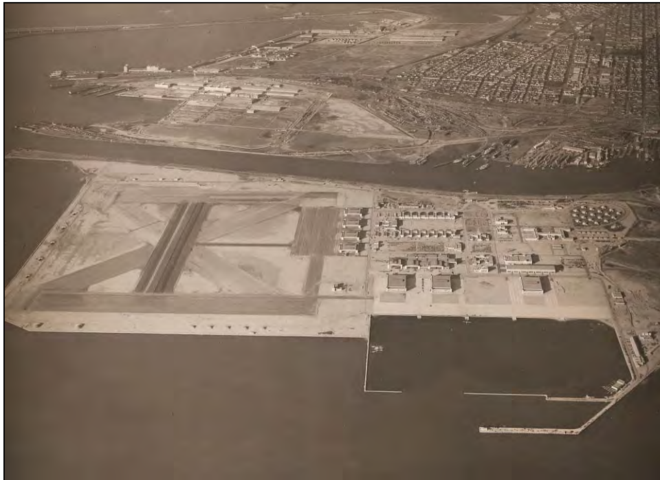
Photograph 34: Aerial Photograph of NAS Alameda November 12, 1941, showing infill and construction progress within the year. 27
