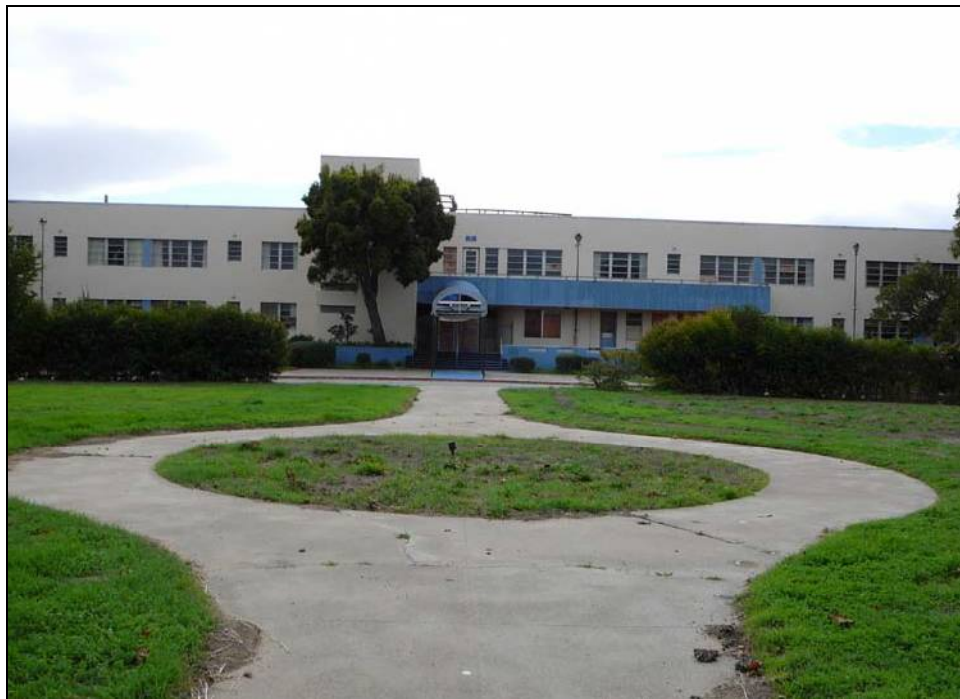
Photograph 85: Curved path on the north side of BOQ Building 17.
