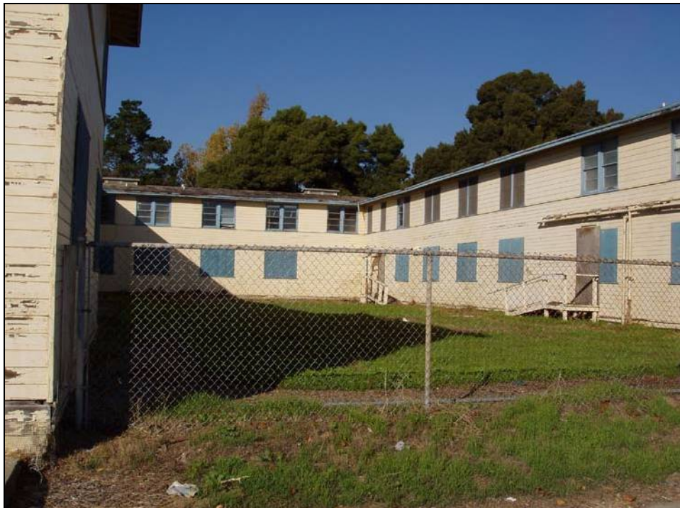
Photograph 62: Typical courtyard found in Administrative Core, Building 135; facing north.
