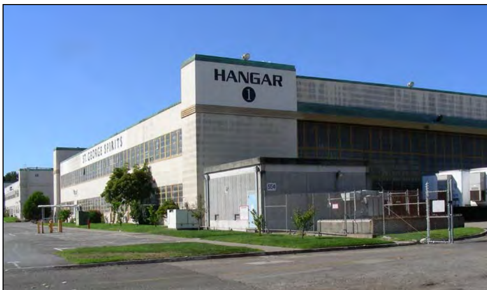
Photograph 62: Lawn panels along east side of landplane hangars. Building 21 in foreground and Building 22 in background.
