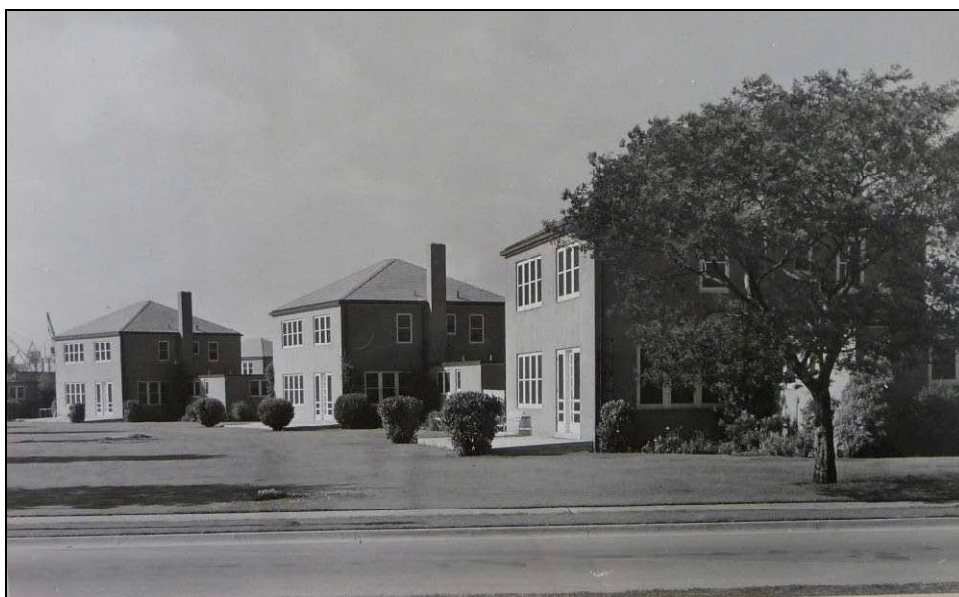
Photograph 27: Housing for married officers circa 1945 as seen from back (southwest side). Implemented landscaping included foundation plantings and shrubs and street trees. 103
