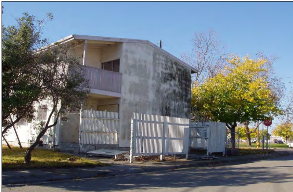
Photograph 18: Fenced drying yard.
