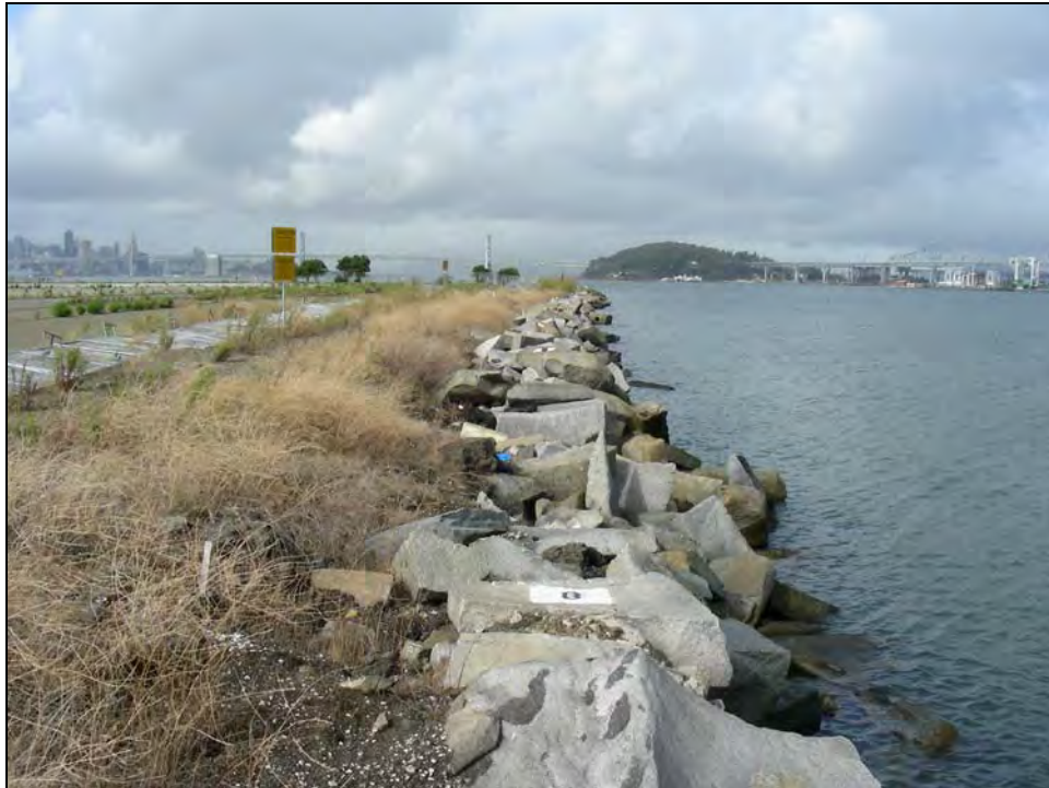
Photograph 22: Riprap along north edge of airfield, facing west.
