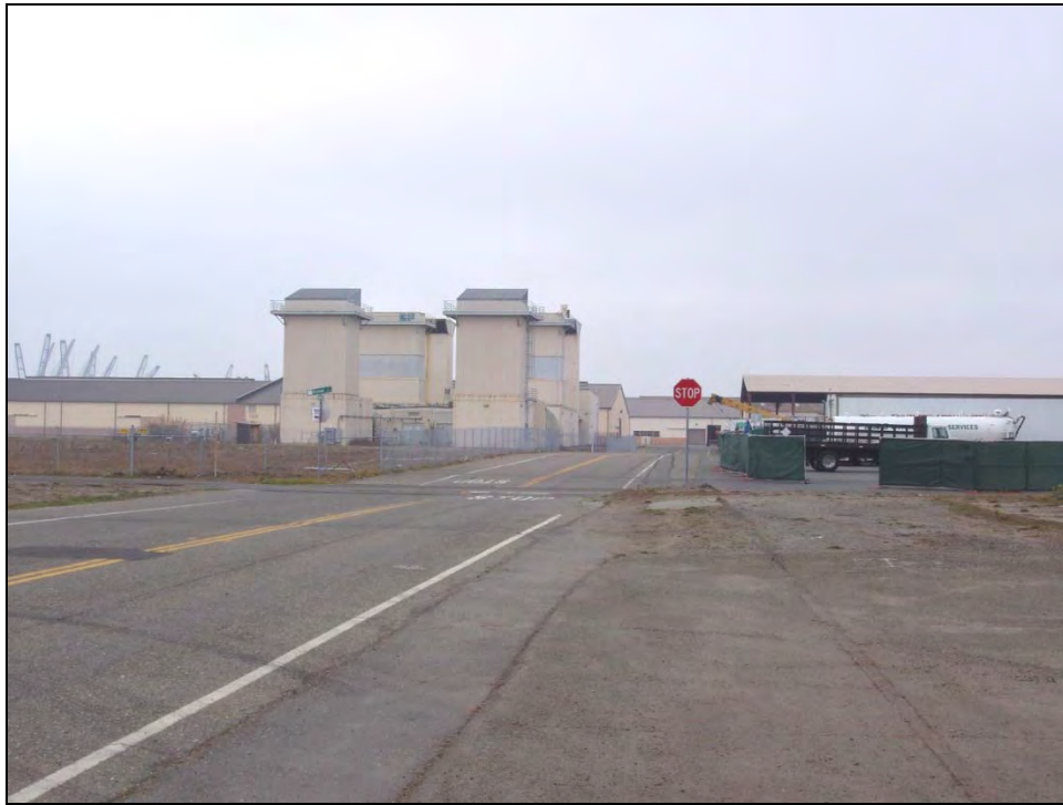
Photograph 4: Buildings in the Southeast area are not a strong spatial organizer. Also note lack of curbing. Camera facing west at intersection of Skyhawk Street and West Pacific Avenue.
