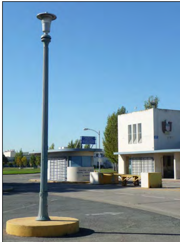
Photograph 32: Light pole in parking lot at Main Gate, sentry house (Building 31) and gate house (Building 30) in background.
