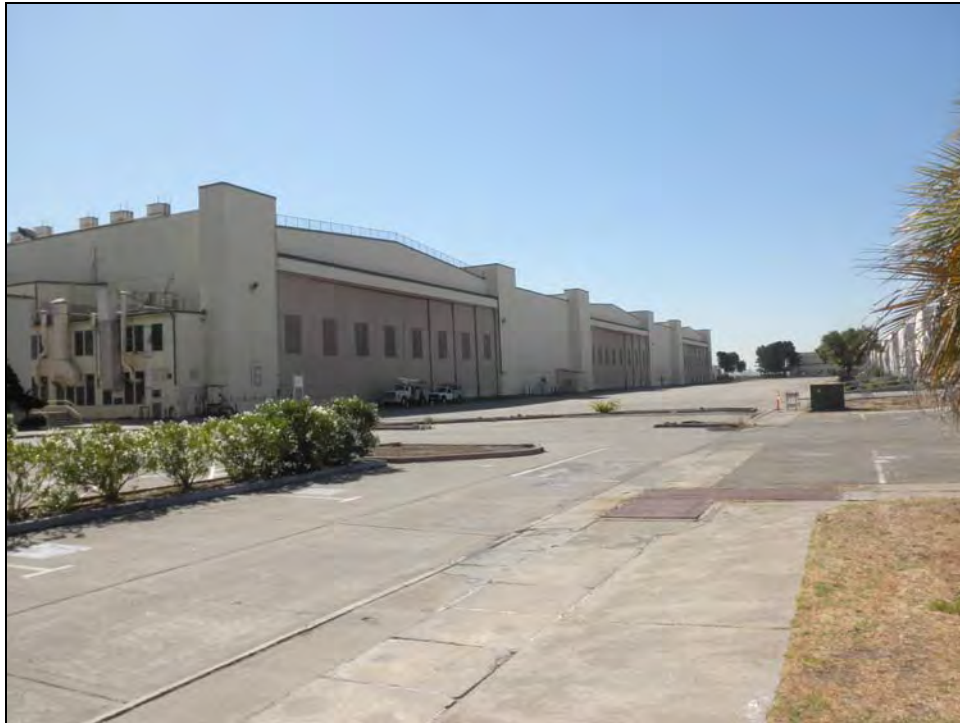
Photograph 37: Space between north side of Building 5 and Building 2.
