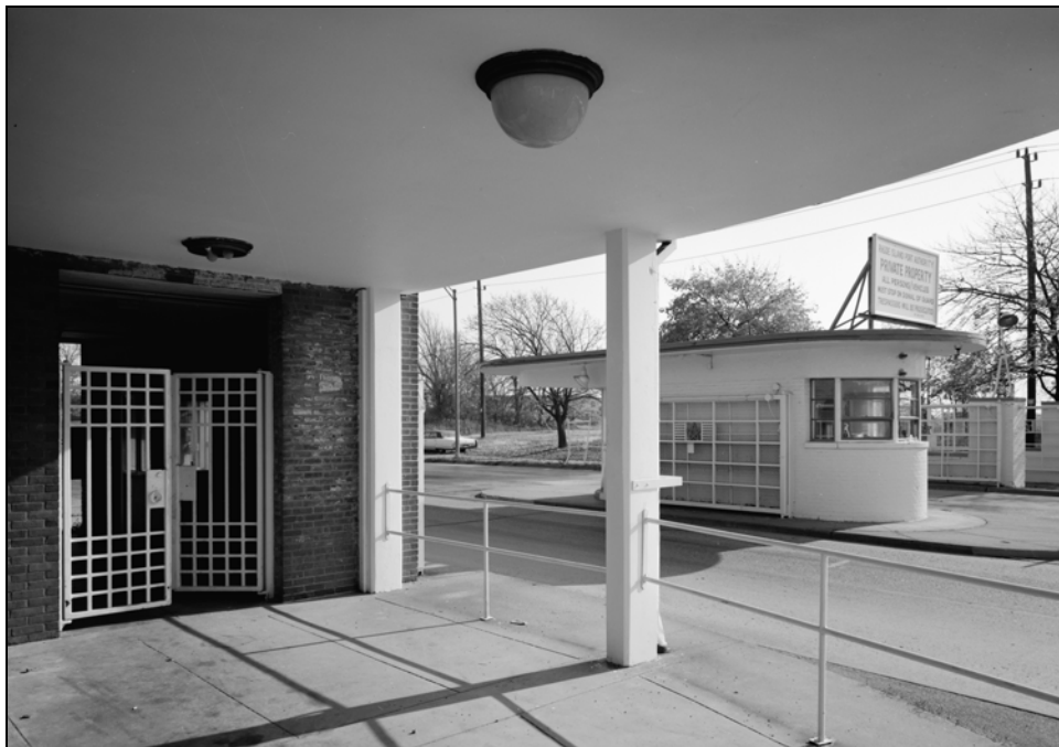
Photograph 79: Buildings 10 and 850, NAS Quonset Point, RI, 1979. 59
