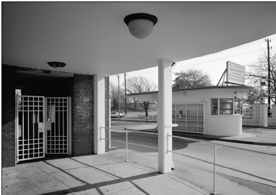
Photograph 45: Buildings 10 and 850, NAS Quonset Point, RI, 1979. 53
