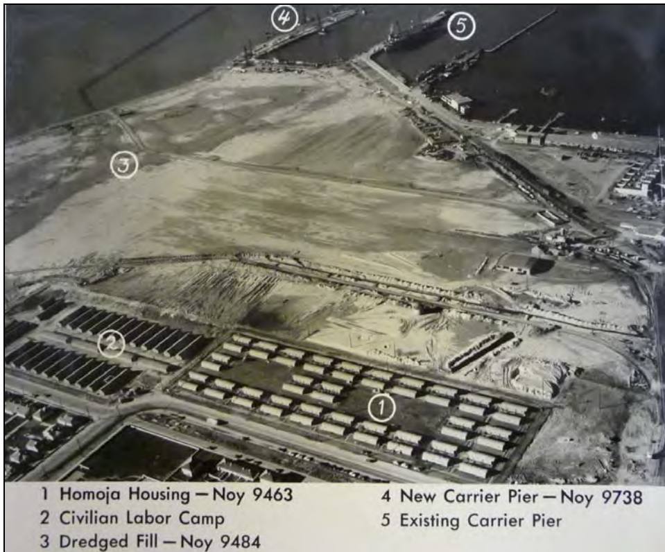
Photograph 50: November 1944. Newly dredged and filled southeast portion of the station. This area was outside the original station plan, and outside the original planting plan. (Numbers and labels from original photo identification.) 76
