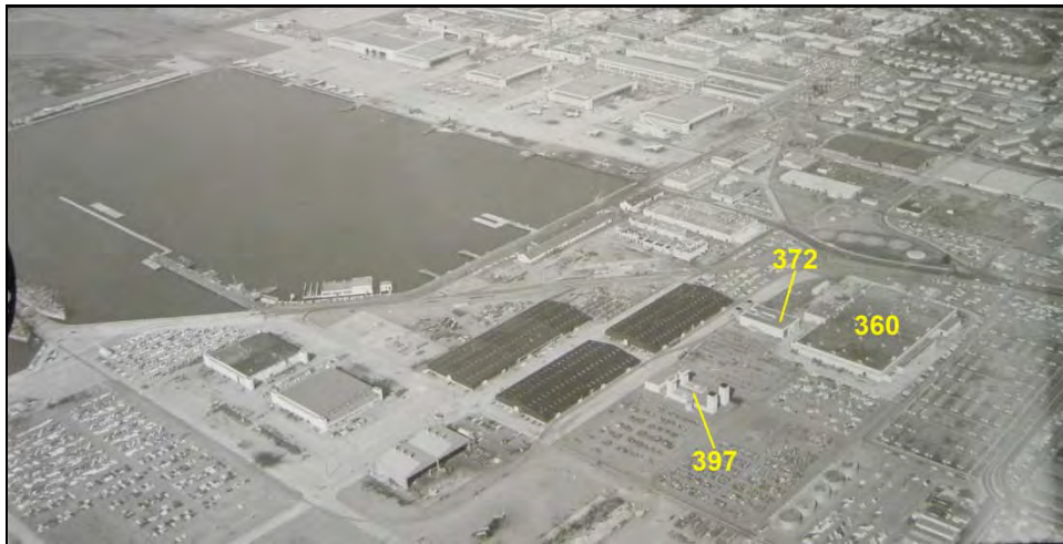
Photograph 111: Aerial view, 1960s. Buildings 360, 372, and 297 have been built in the southeast portion of the station in the additional Shops Area. 146
