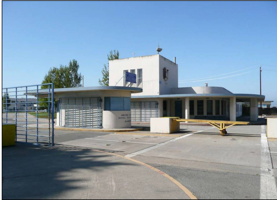
Photograph 15: Buildings 30 and 31, NAS Alameda, 2009.
