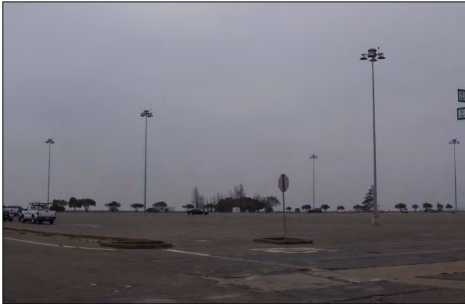
Photograph 28: Asphalt parking lot in waterfront area, note curved curbing; camera facing southwest.
