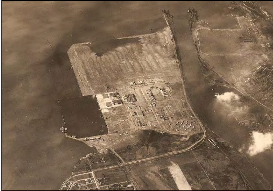
Photograph 66: Aerial Photograph of NAS Alameda January 20, 1941. Note the rows of dredged materials on what is now the Airfield. 31
