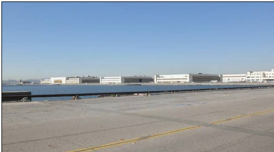
Photograph 114: Seaplane hangars aligned with straight line of Seaplane Lagoon, facing northwest.
