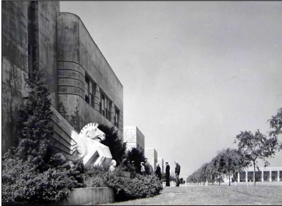
Photograph 34: 1945. Building 4 at left, camera facing west. The tree line depicted in the planting plan had been executed (right), and like other buildings in the Administrative Core, Building 4 had foundation shrubbery. 110
