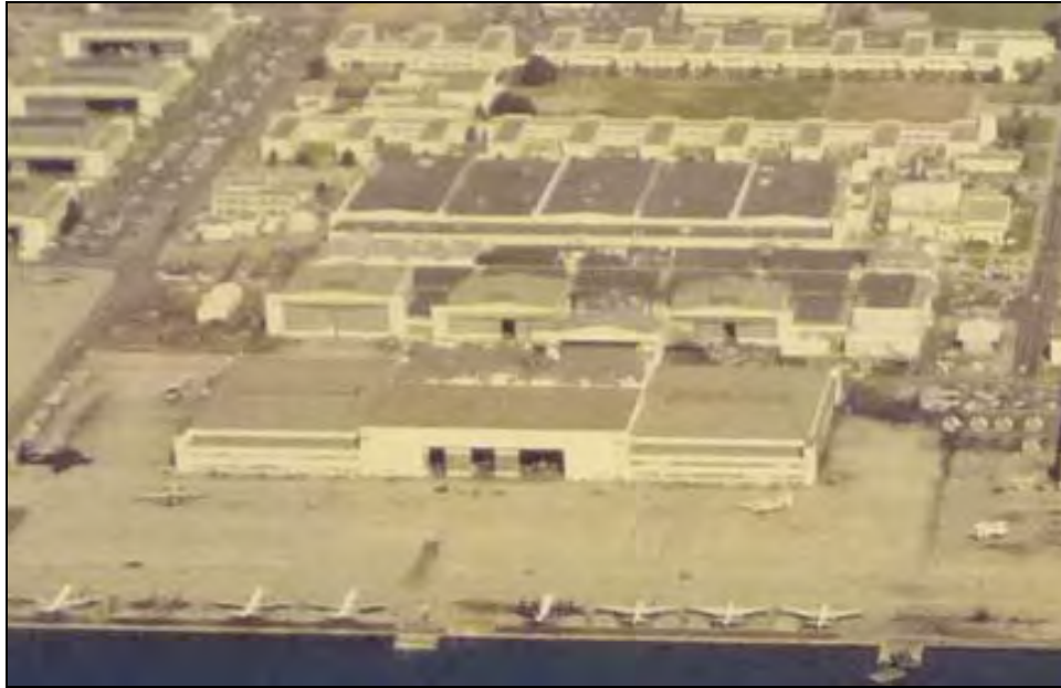
Photograph 118: 1960s oblique aerial showing Building 400 in the foreground, located between Hangars 11 and 12. 170
