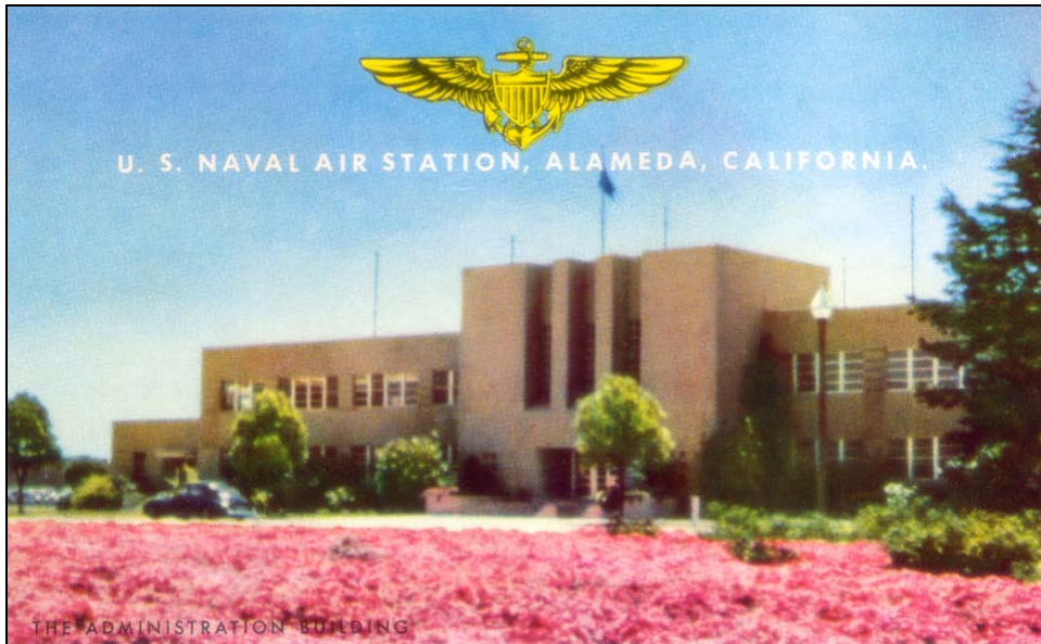
Photograph 92: Period postcard depicting Building 1, circa 1943. Colorized postcard exaggerated the vibrancy of ice plant in entry mall.
