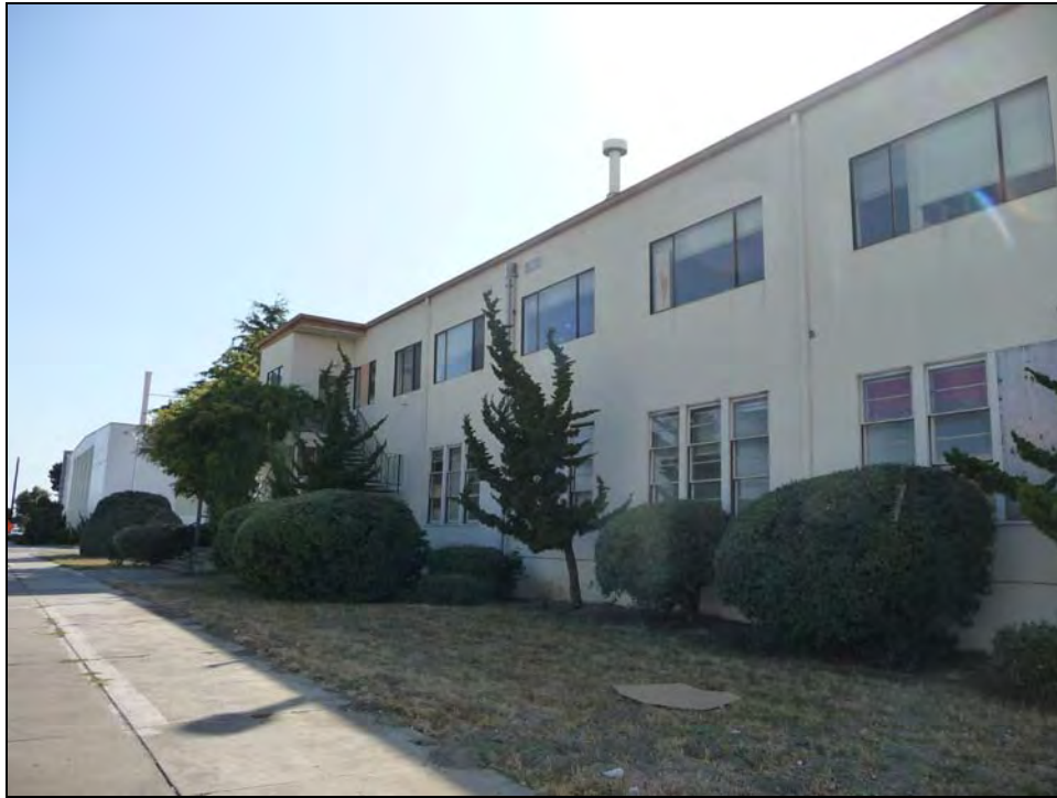
Photograph 41: Vegetation on the north side of Building 62 along West Midway Avenue.
