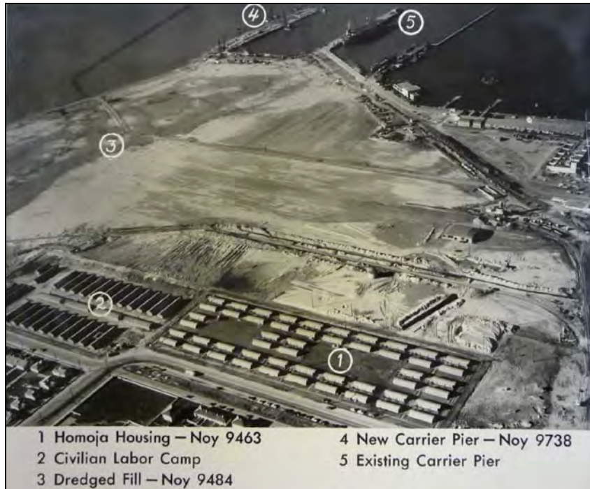
Photograph 84: November 1944. Newly dredged and filled southeast portion of the station. This area was outside the original station plan, and outside the original planting plan. (Numbers and labels from original photo identification.) 83
