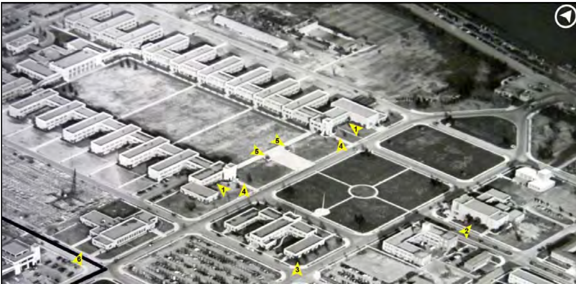
Photograph 96: 1944. In addition to the plantings present by January 1942, this photograph indicates the presence of foundation shrubbery around the east ends of Buildings 2 and 4 (1), and on the south side of Building 18 (2). Street trees are present around Building 1 (3). Also present are paired plantings flanking the pathways approaching the east ends of Buildings 2 and 4 (4) and the BEQ quadrangle (5). Parts of the Shops Area also had formal plantings, as seen here at Building 62 (6). 104
