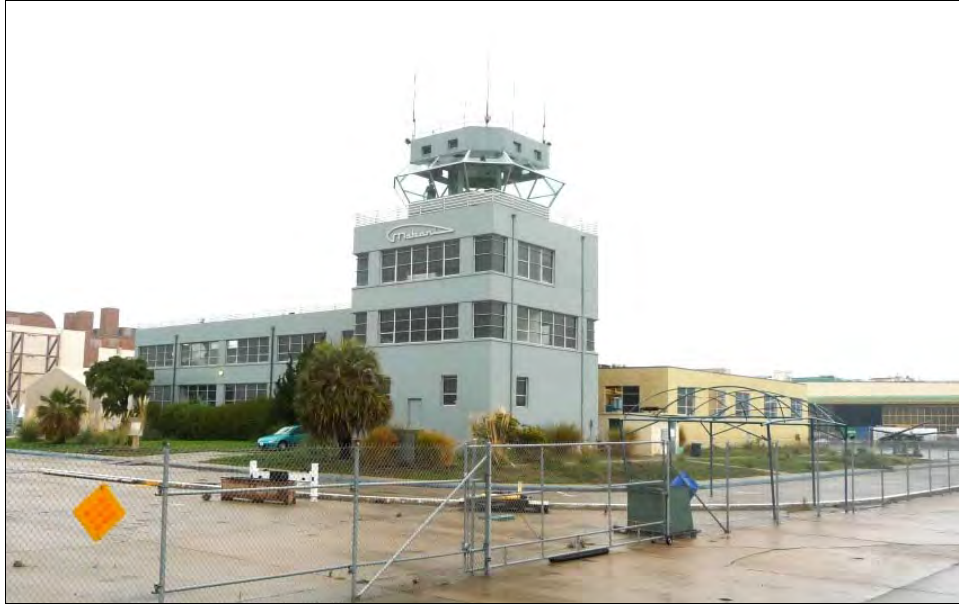
Photograph 63: Wide lawn panels with foundation shrubs around Building 19 (Control Tower).
