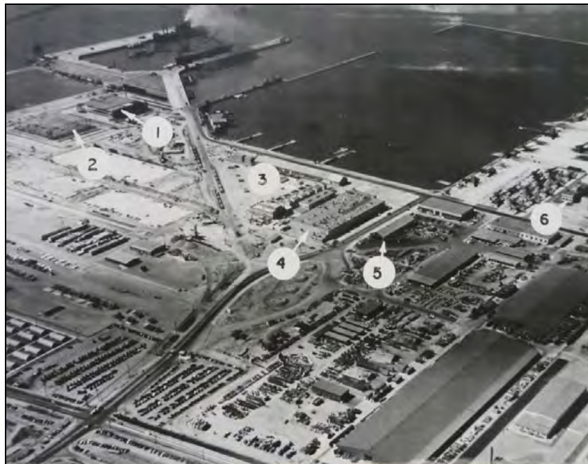
Photograph 85: September 1945. Southeast portion of the station retained a utilitarian appearance throughout World War II, distinct from the formal design of the core of the station. (Numbers from original photo identification.) 84
