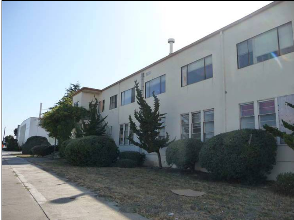
Photograph 96: Vegetation on the north side of Building 62 along West Midway Avenue.
