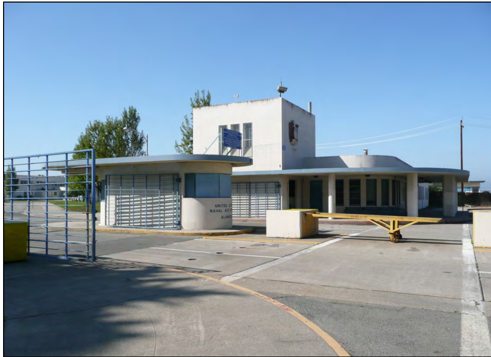
Photograph 44: Buildings 30 and 31, NAS Alameda, 2009.
