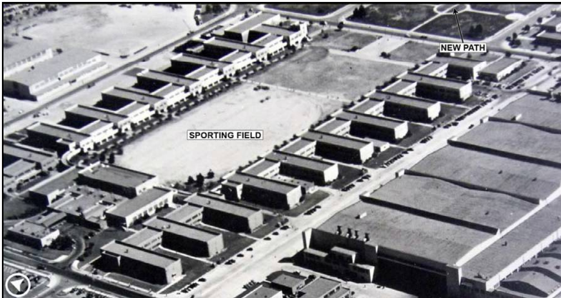
Photograph 36: September 1945. The western pathway bisecting the BEQ quadrangle was removed to make room for a sporting field. Also note the extension of the path through the circular area in the center of the entry mall. 112
