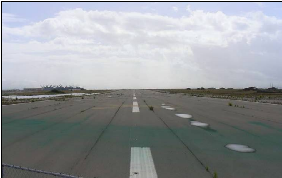
Photograph 138: Runways are a strong spatial organizer in the Airfield; north end of Runway 13-31 facing southeast.
