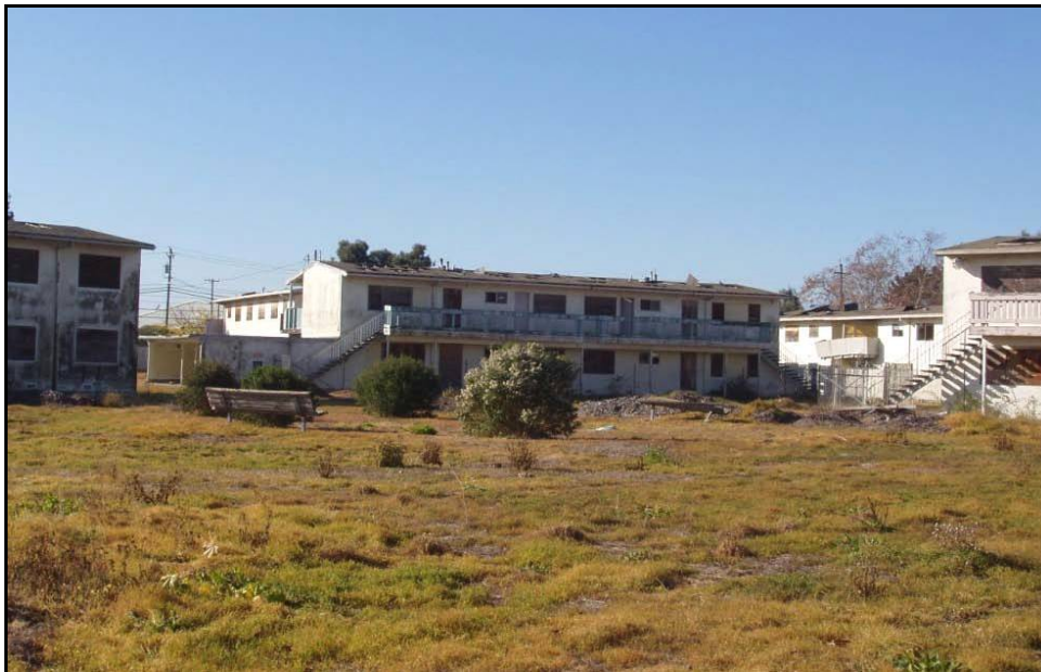
Photograph 127: Organization of multi-family area between Tower Avenue and Stardust; camera facing northwest.
