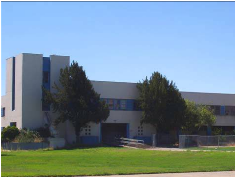
Photograph 73: Example of trees flanking building entries in the Administrative Core; cypresses at Wing 1, Building 2.
