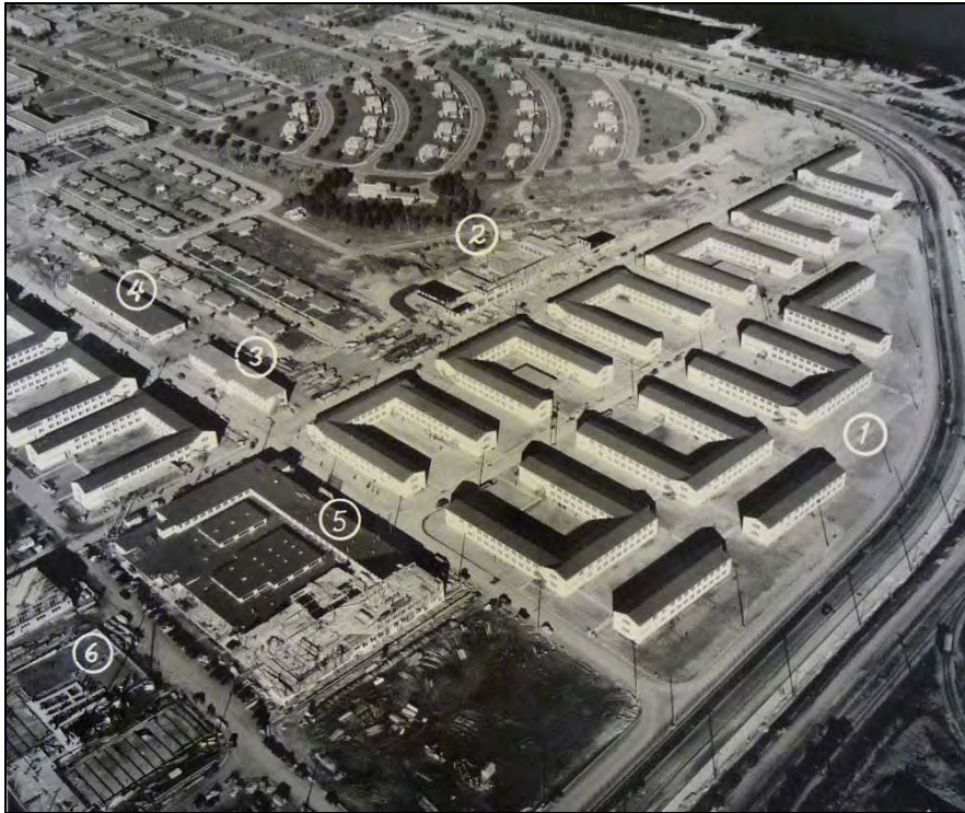
Photograph 86: Construction of temporary style barrack on east end of NAS Alameda, 1944. Numbers indicated specific projects on original photograph. 92
