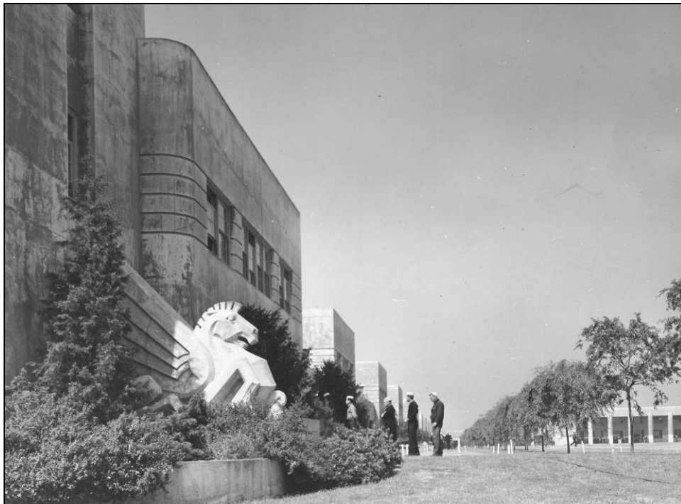
Photograph 71: East end of Building 2, May 1945. 45
