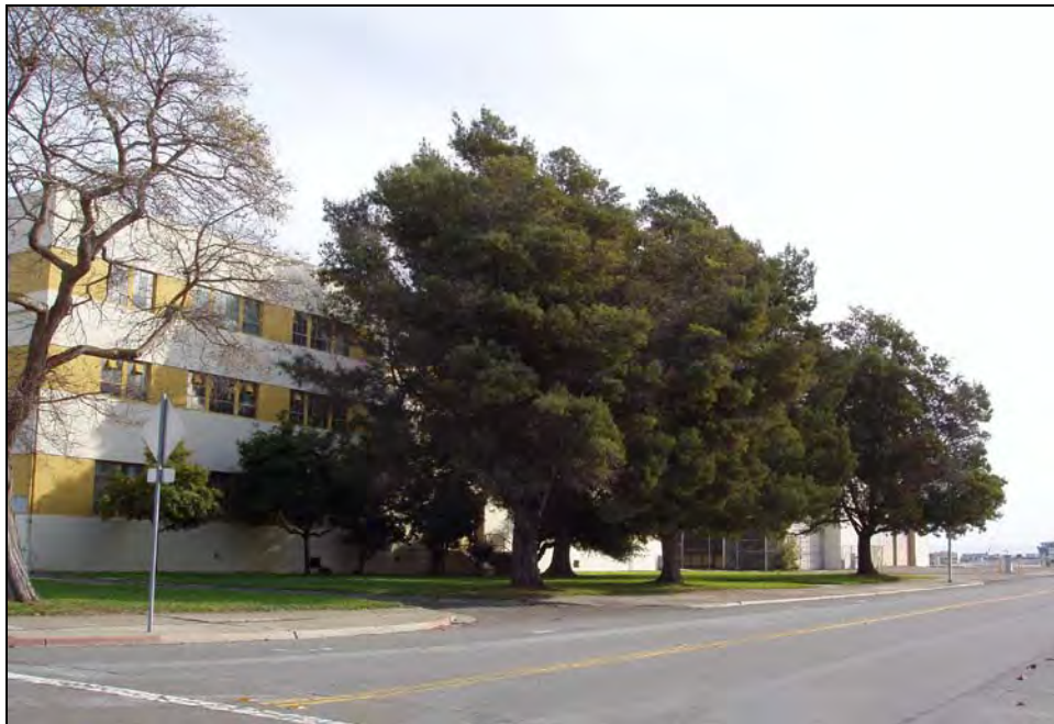
Photograph 40: Vegetation on west side of Building 8, along Lexington Street.
