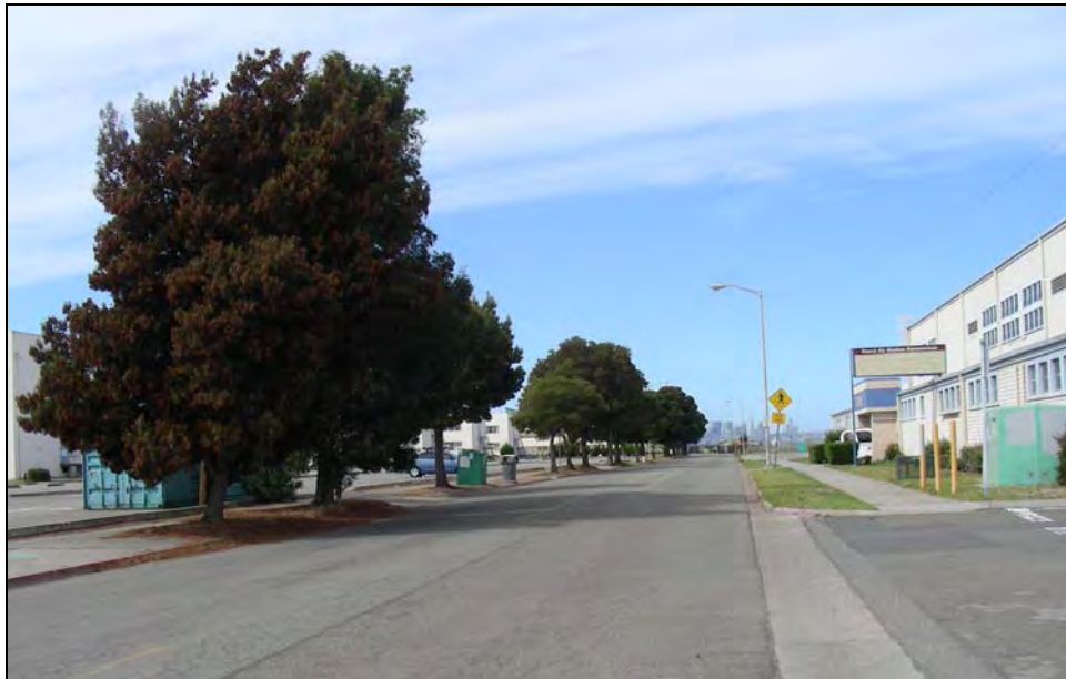
Photograph 2: West Red Line Avenue Building 134 at right, view of San Francisco in background.
