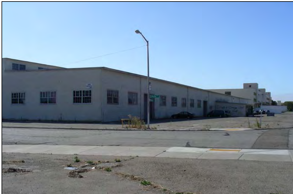
Photograph 38: Most of the Shops Area is paved; view showing Building 92 at the intersection of Pan Am Way and West Ranger Avenue.
