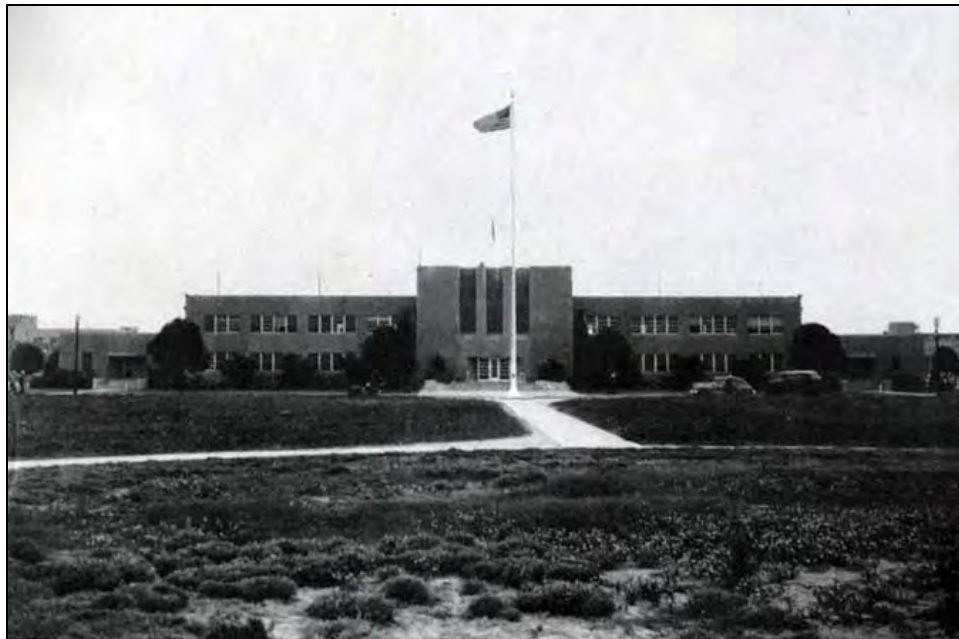
Photograph 61: 1945. Building 1, facing south from circular space in the center of the entry mall. 95
