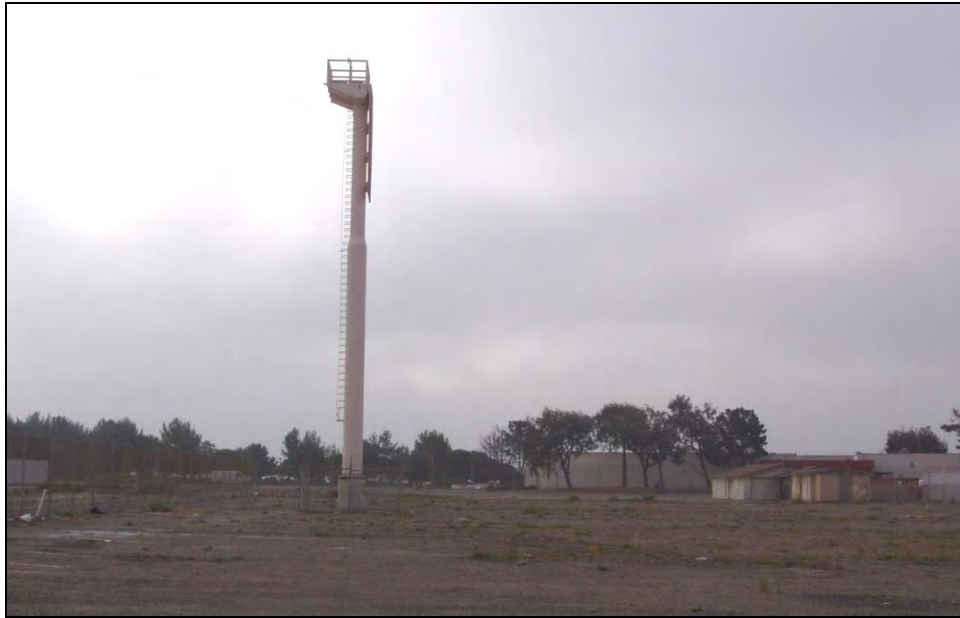
Photograph 30: Navigation range light in fallow area south of Building 530; facing south.
