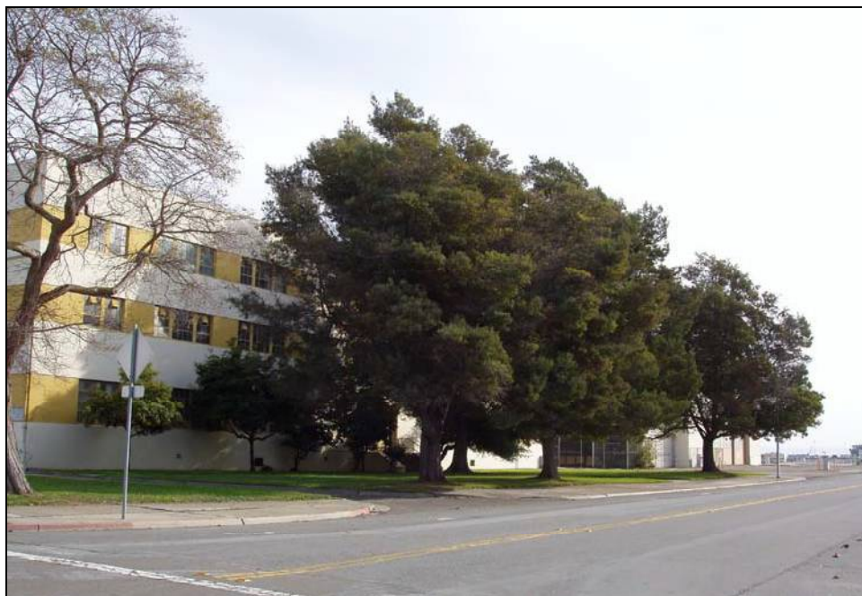
Photograph 95: Vegetation on west side of Building 8, along Lexington Street.
