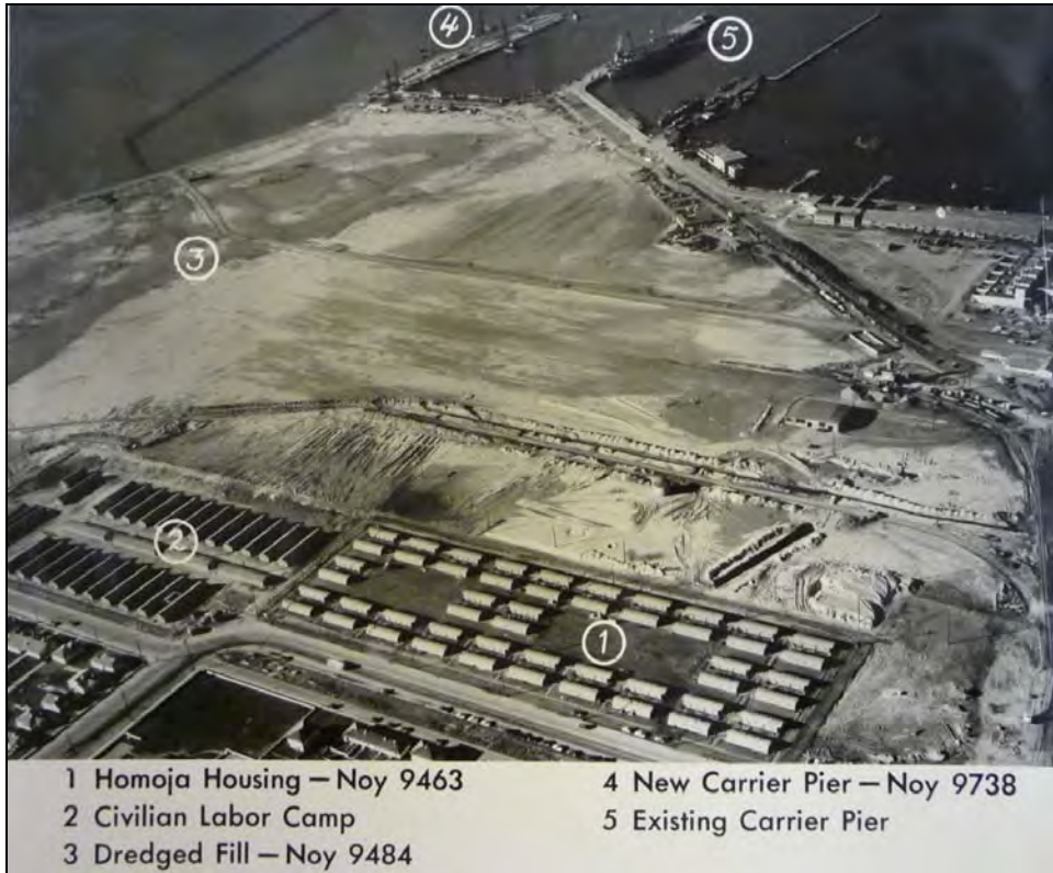
Photograph 50: November 1944. Newly dredged and filled southeast portion of the station. This area was outside the original station plan, and outside the original planting plan. (Numbers and labels from original photo identification.) 76
