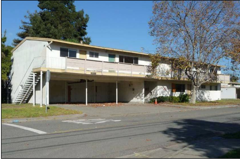
Photograph 50: Typical Capehart multiple family unit, Building 754, camera facing northeast, November 12, 2009.
