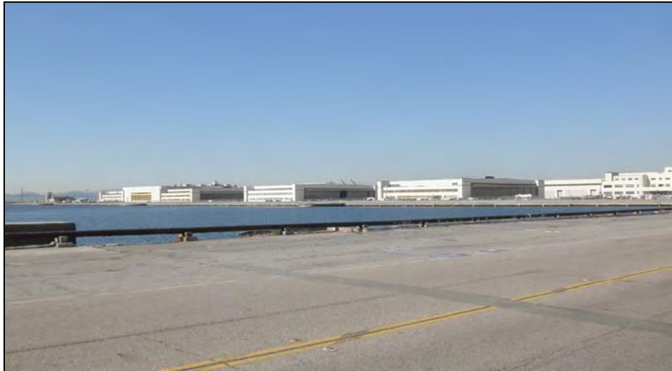
Photograph 59: Seaplane hangars aligned with straight line of Seaplane Lagoon, facing northwest.
