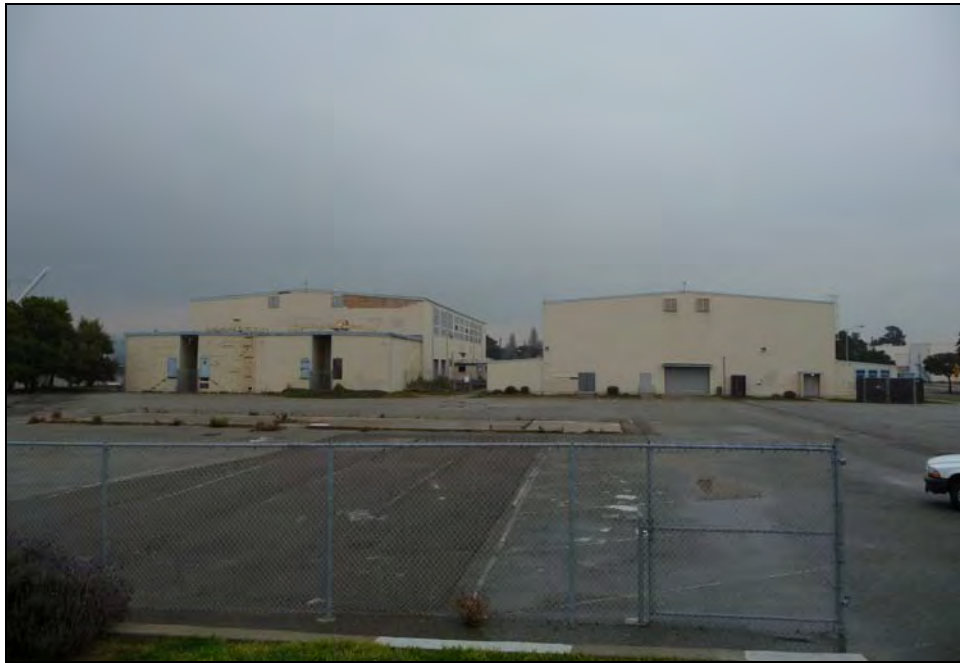
Photograph 3: Large open paved area west of Buildings 76 and 134.
