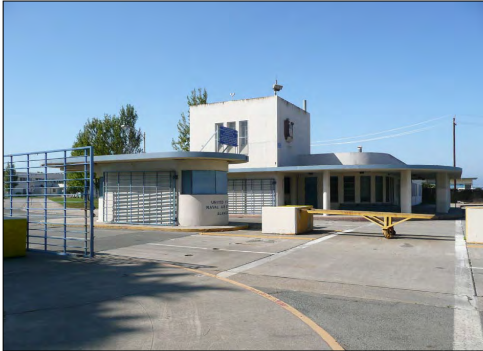
Photograph 78: Buildings 30 and 31, NAS Alameda, 2009.
