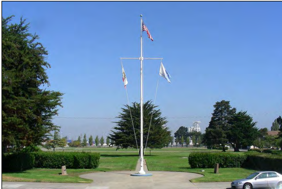
Photograph 9: View looking north from Building 1; monuments in foreground, Monterey cypress tree at center, and crane in background at right.
