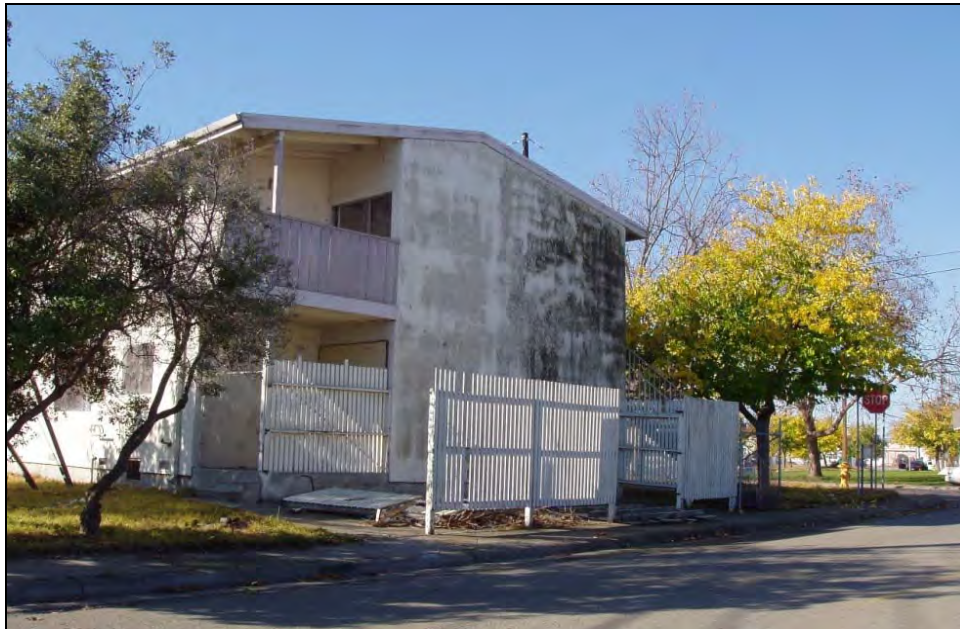
Photograph 18: Fenced drying yard.
