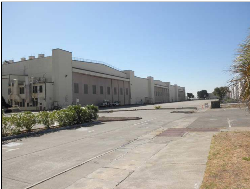
Photograph 92: Space between north side of Building 5 and Building 2.
