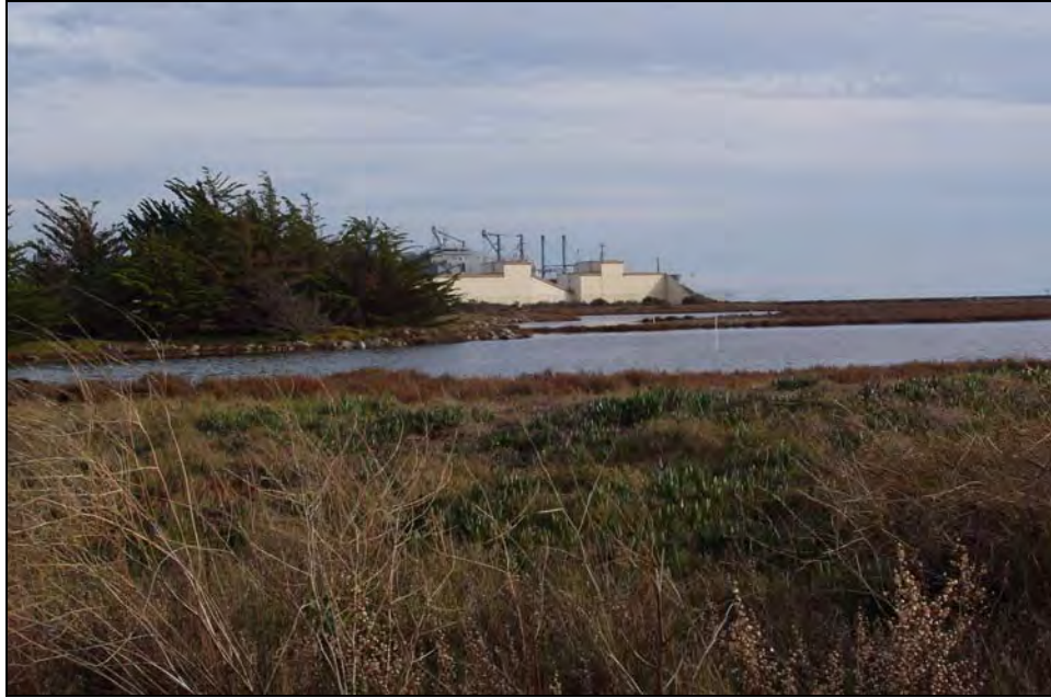
Photograph 20: Marsh at southeast corner of Airfield, Building 29 in background; facing southeast.
