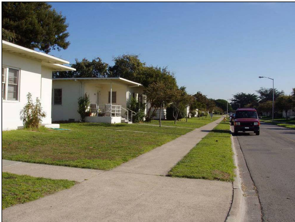
Photograph 103: CPO Housing showing straight alignment of roads, density of development, and uniformity of siting from street and from one another; also note planted parking strip.
