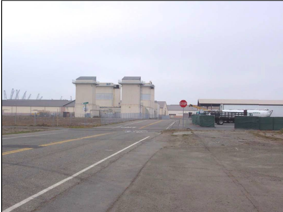
Photograph 121: Buildings in the Southeast area are not a strong spatial organizer. Also note lack of curbing. Camera facing west at intersection of Skyhawk Street and West Pacific Avenue.
