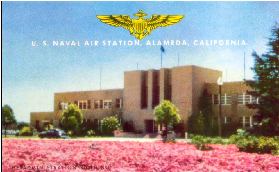
Photograph 58: Period postcard depicting Building 1, circa 1943. Colorized postcard exaggerated the vibrancy of ice plant in entry mall.
