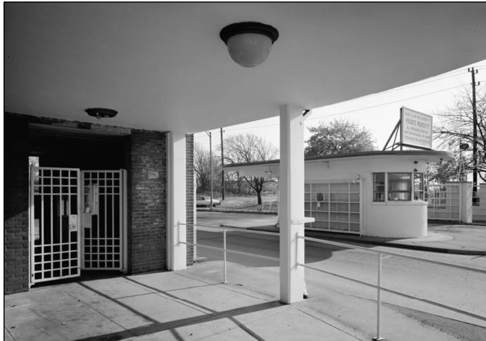
Photograph 16: Buildings 10 and 850, NAS Quonset Point, RI, 1979. 64
