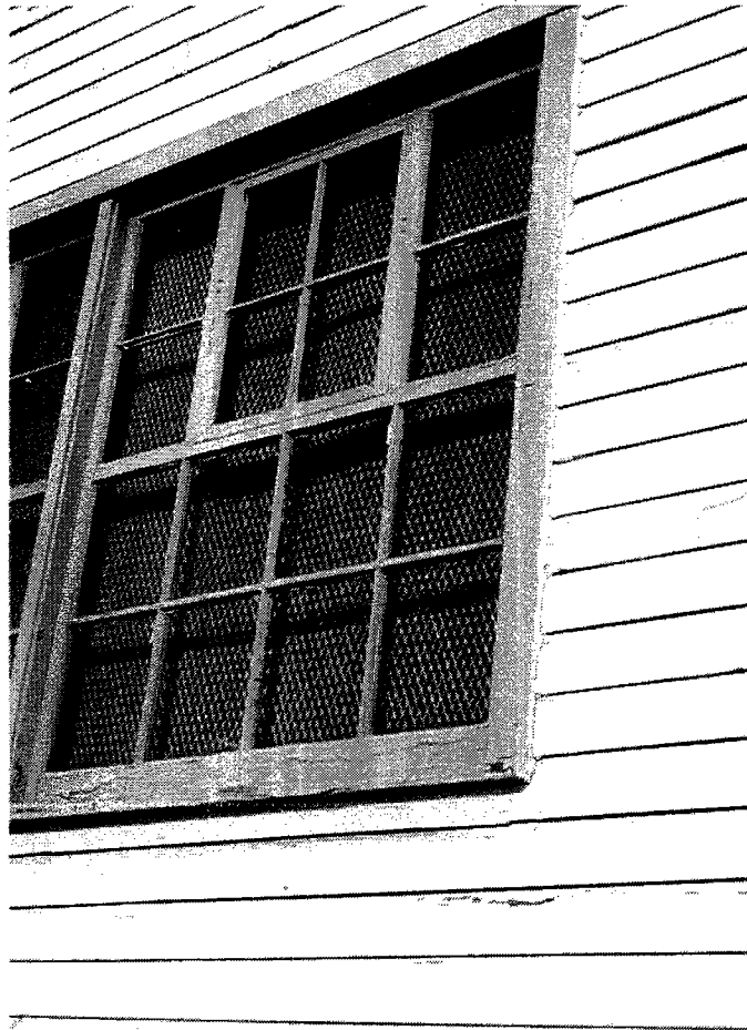
Photograph 51. Wooden industrial sash in Building 92.
