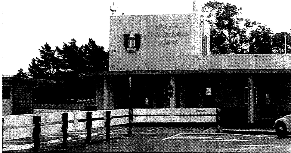
Photograph 33. Gate House, Building 30.
