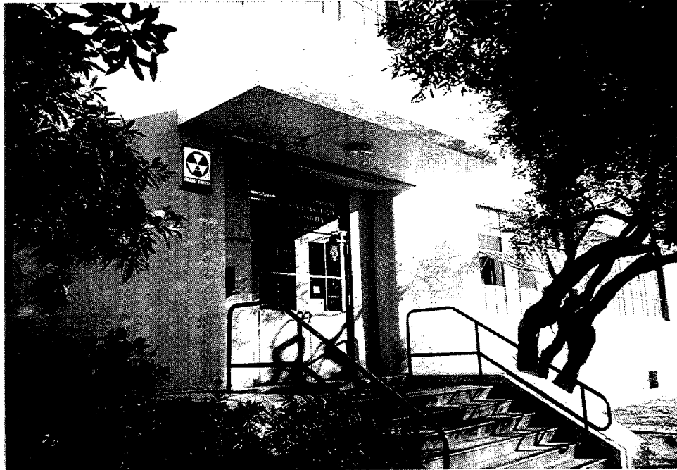
Photograph 54. Original steel personnel door, Building 8.
