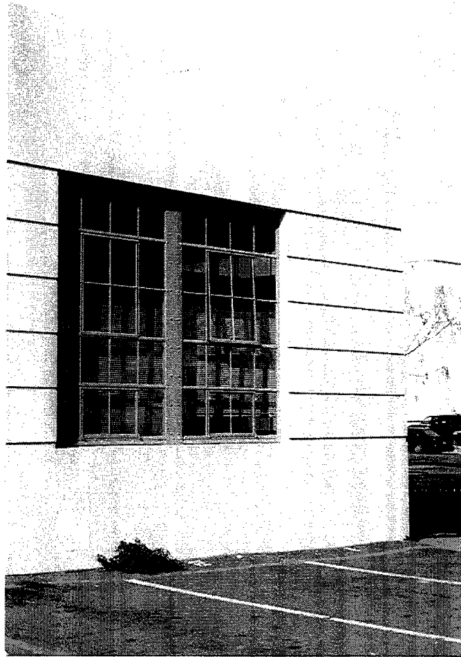
Photograph 52. Steel sash in Building 6.
