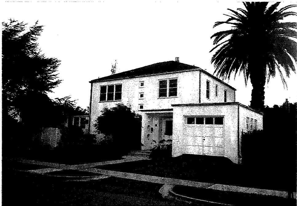
Photograph 58. Typical Officers' Quarters building.
