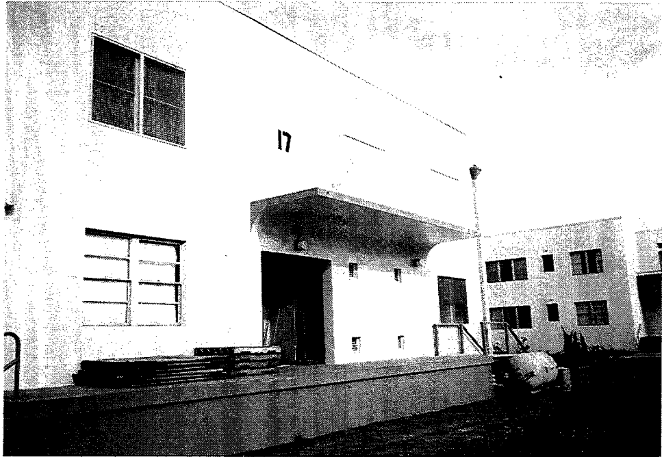
Photograph 32. Concrete canopy over loading dock of Building 17.
