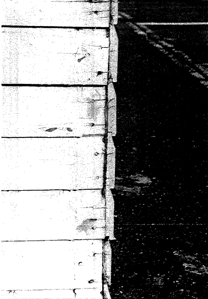
Photograph 43. Drop siding on Building 91.
