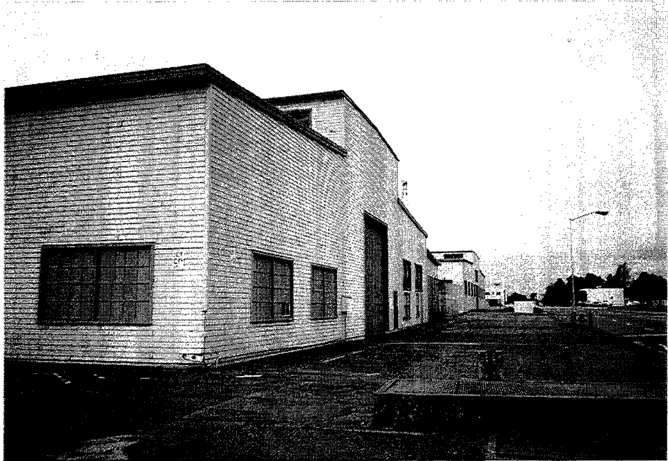
Photograph 42. East sides of Buildings 91 and 92, wood frame warehouses.
