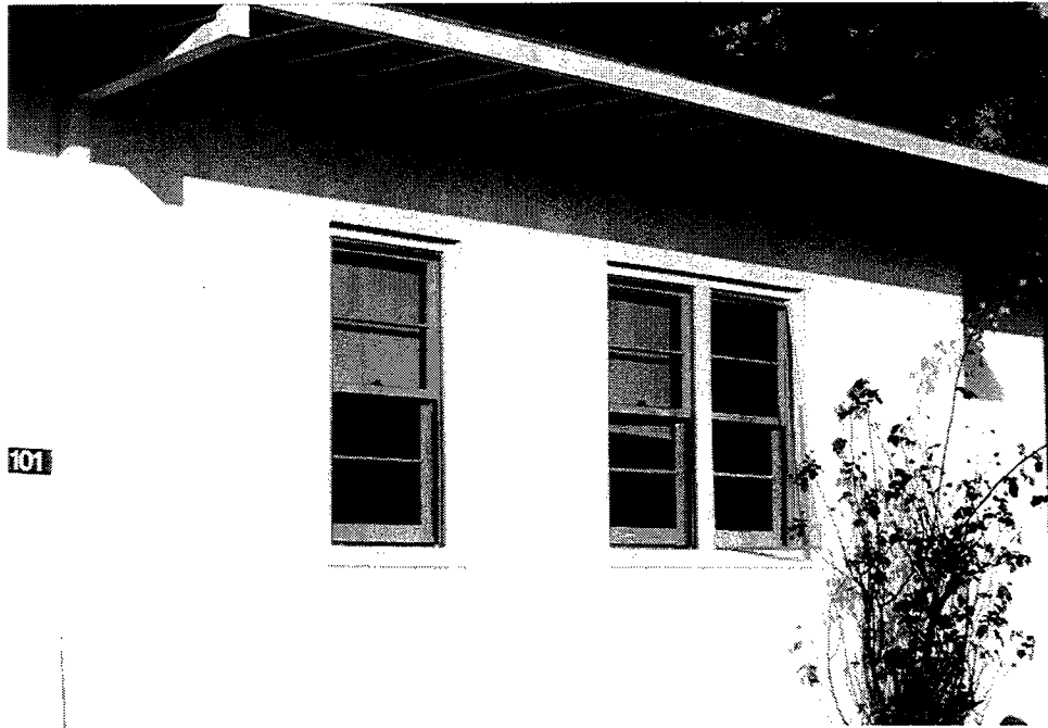
Photograph 61. Window detail, NCO Quarters.
