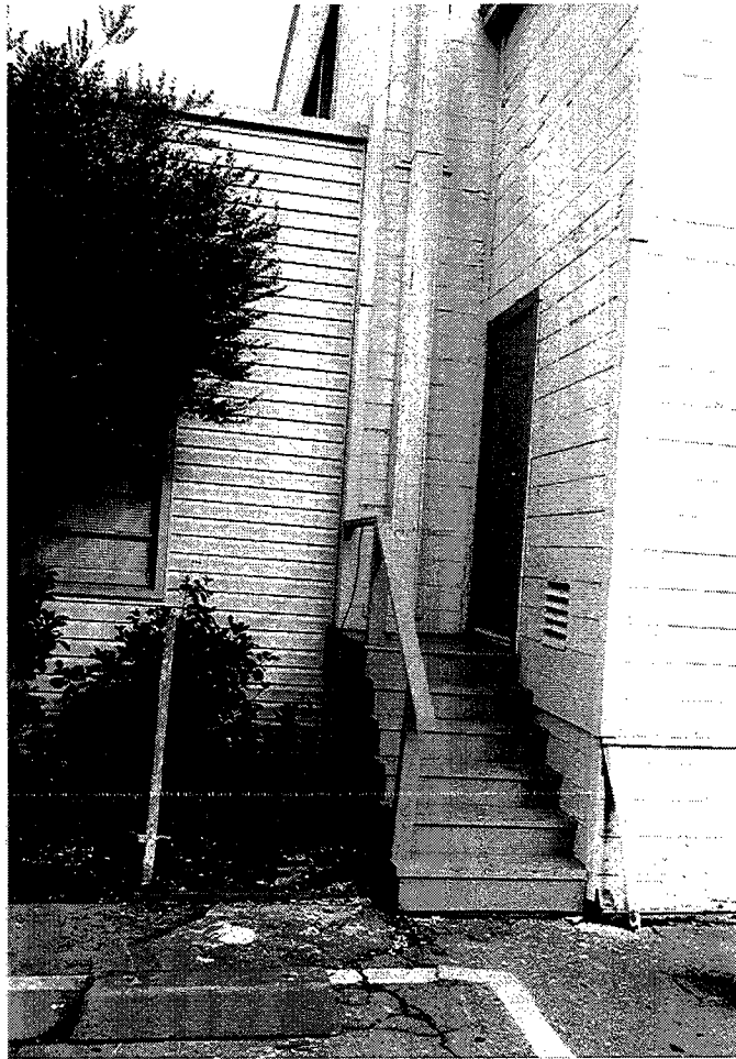
Photograph 45. New vinyl siding on office wing of Building 101.
