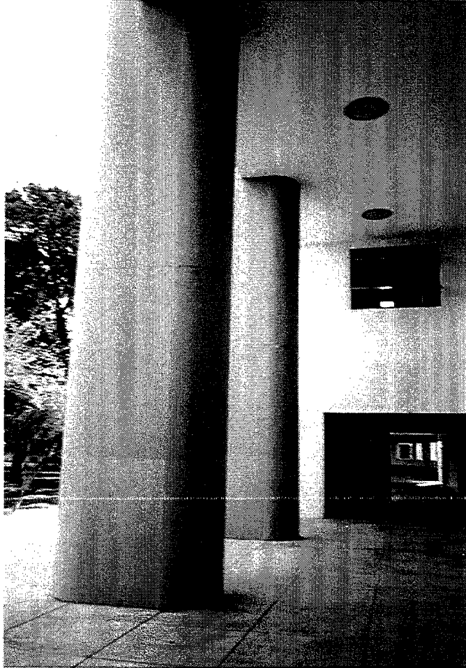
Photograph 18. Massive columns, Building 3.
