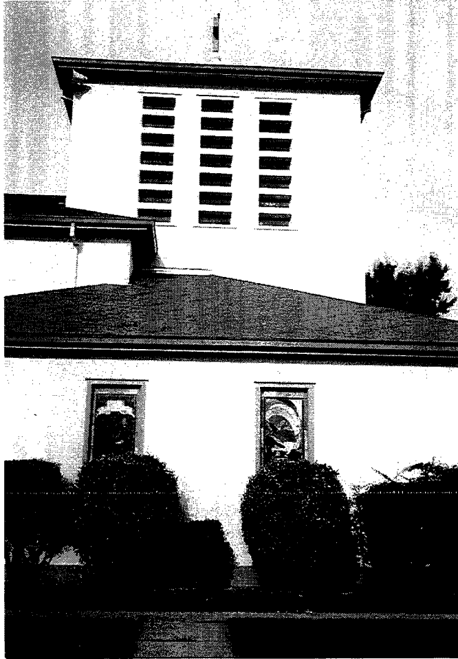
Photograph 27. Stacked openings in belfry of Building 94.
