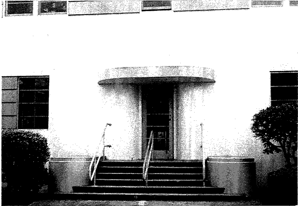
Photograph 11. Five-light door, concrete canopy, concrete planters, and steel railings are rounded to go with the other rounded forms, Building 1.
