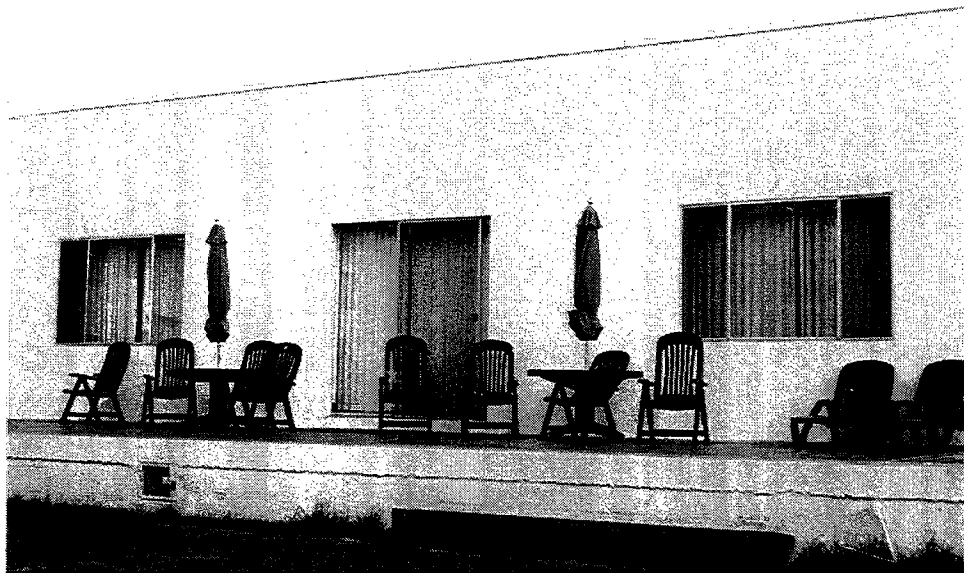
Photograph 9. Inappropriate windows and doors in Building 17.
