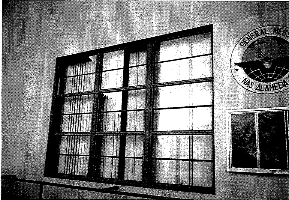
Photograph 10. Steel awning windows in Building 3.
