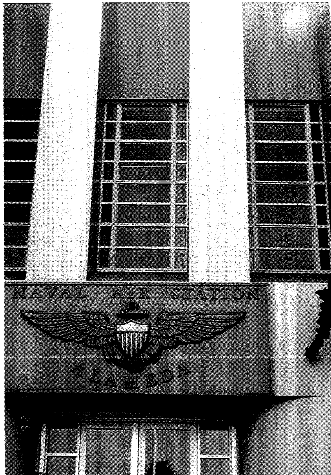
Photograph 25. Stacked windows in entry pavilion of Building 1.
