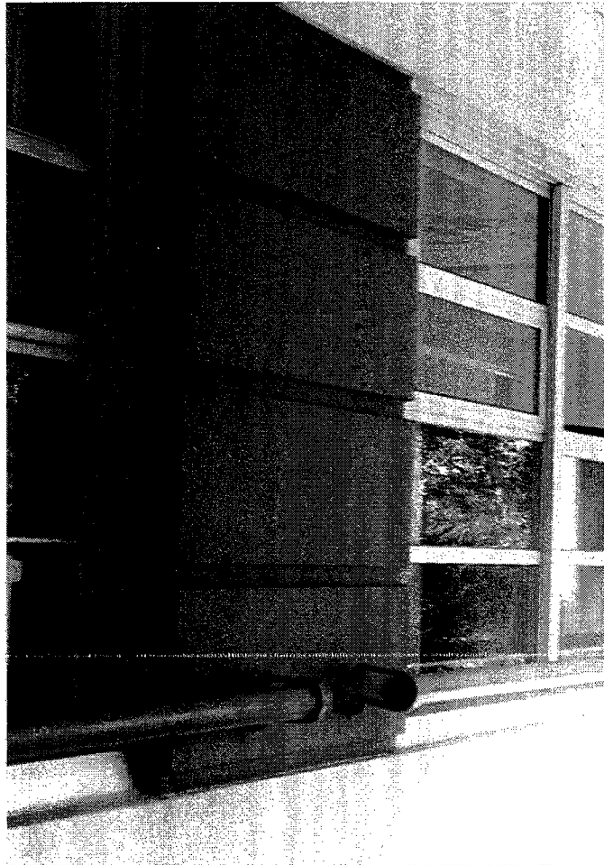
Photograph 14. Quoin-like features in Building 4; also illustrates replacement windows with wide muntins.
