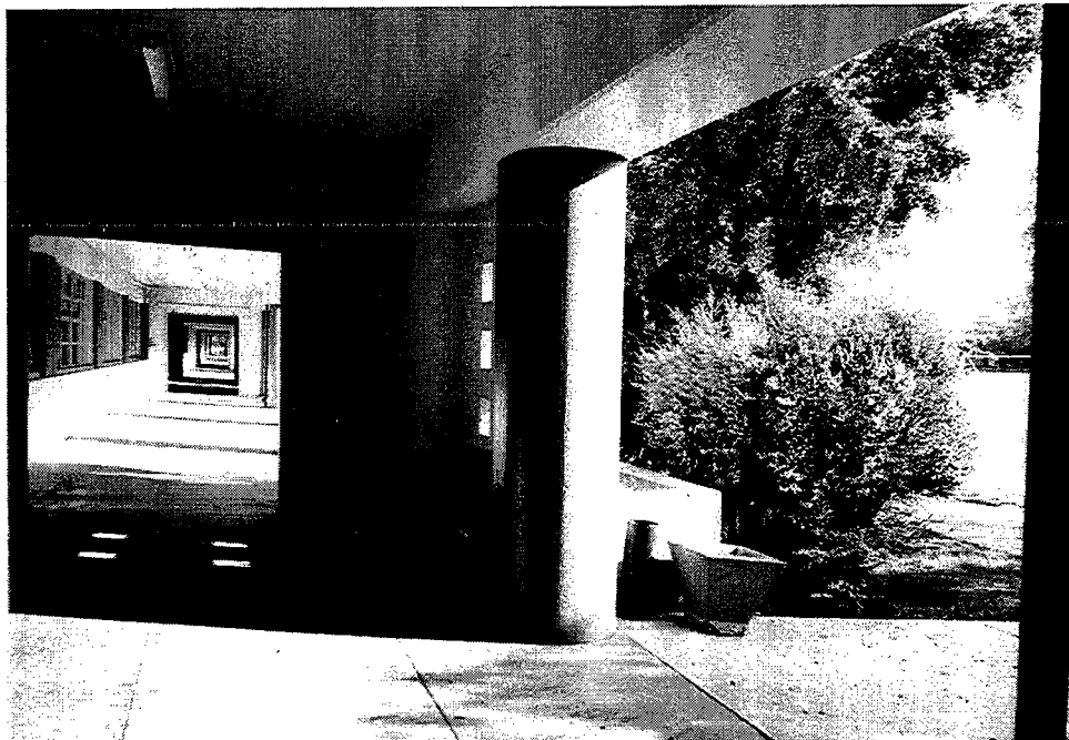
Photograph 17. Oval columns, arcade, Building 2.
