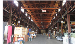
Interior View of Packing-Shipping Storehouse
