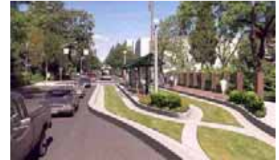
Busway under construction in Eugene, OR Station and median views
